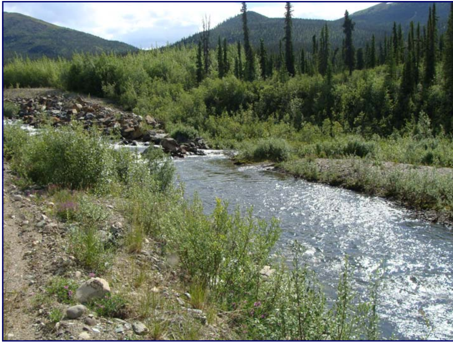
July: view of the lower weir section, this is where Severin Creek enters the Diversion Canal.
