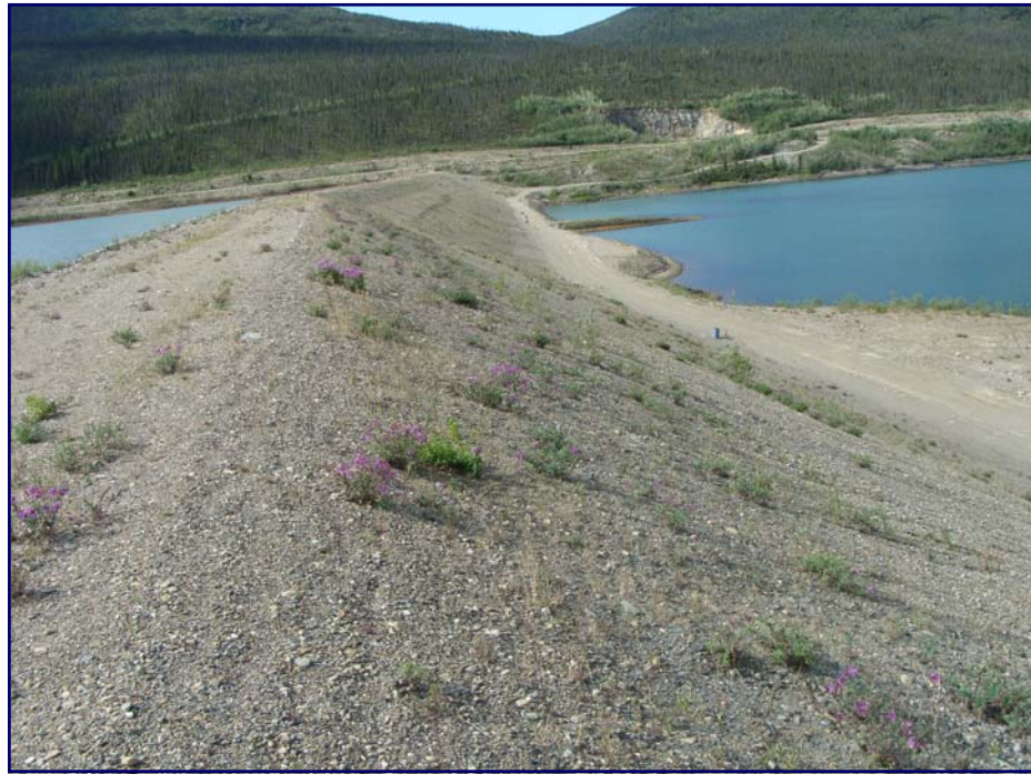
July: showing a view looking south along the downstream dam face.
