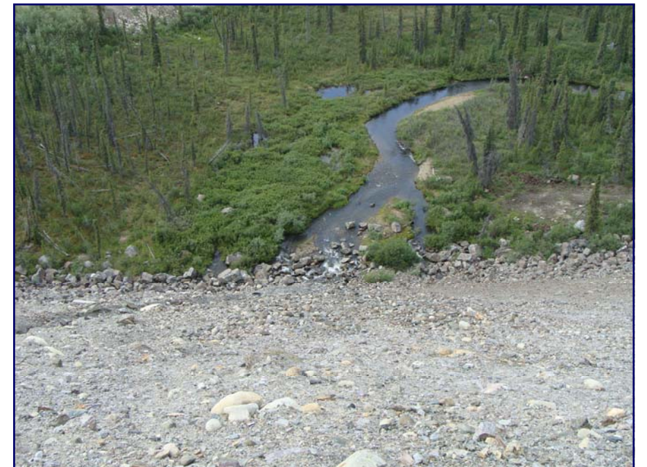
July: Looking at the downstream drain from the crest.
