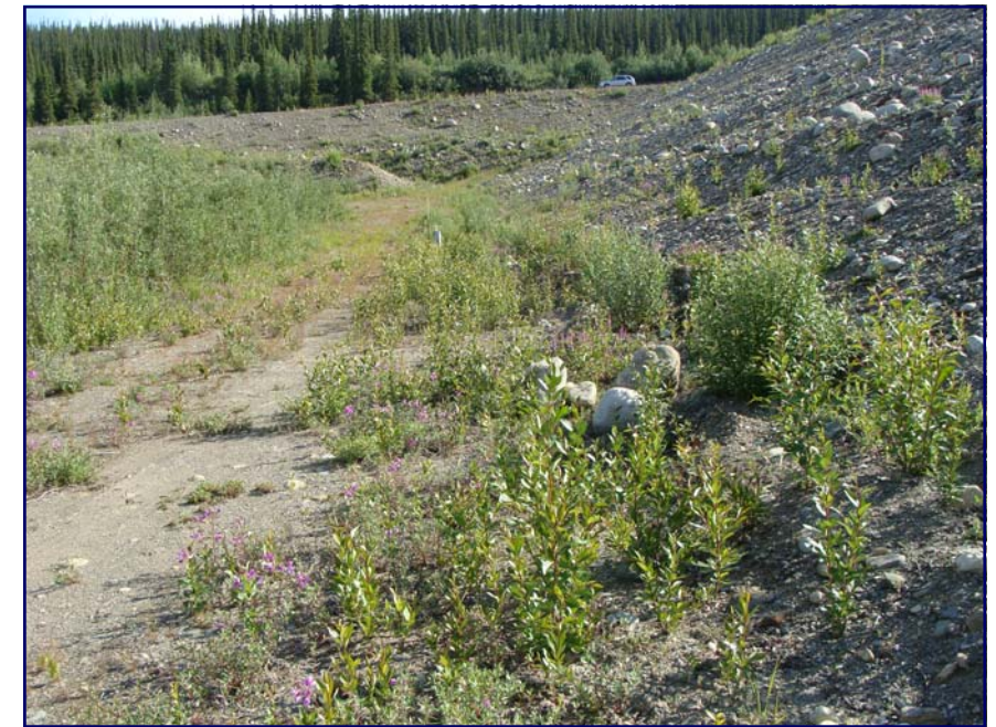
July: view of the wet location located on the right side of the dam toe.
