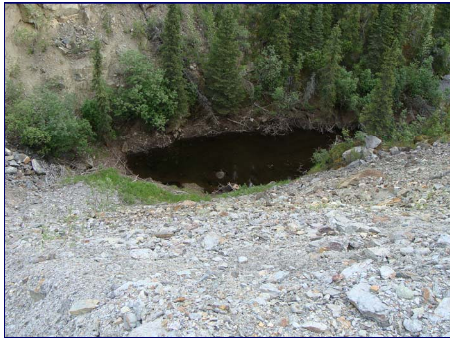
June: a view looking down the upstream face of the rock drain at the upstream pond.
