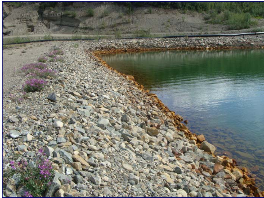
July: shows a view of the riprap near the spillway.
