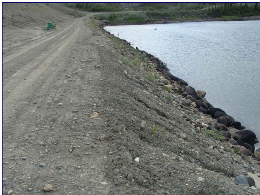
July: shows a view of the edge of the polishing pond. Note that some rilling and wave erosion is evident.
