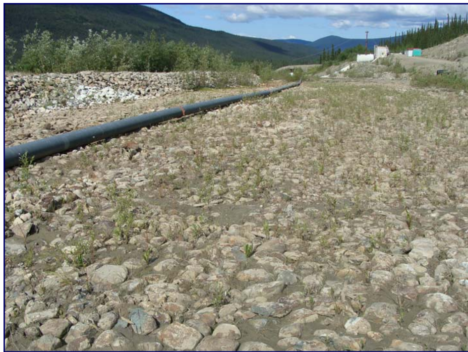
July: looking downstream in the spillway.
