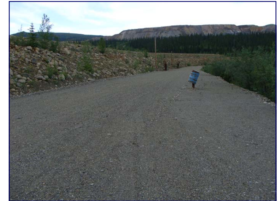
July: shows the downstream face of the Secondary Dam.
