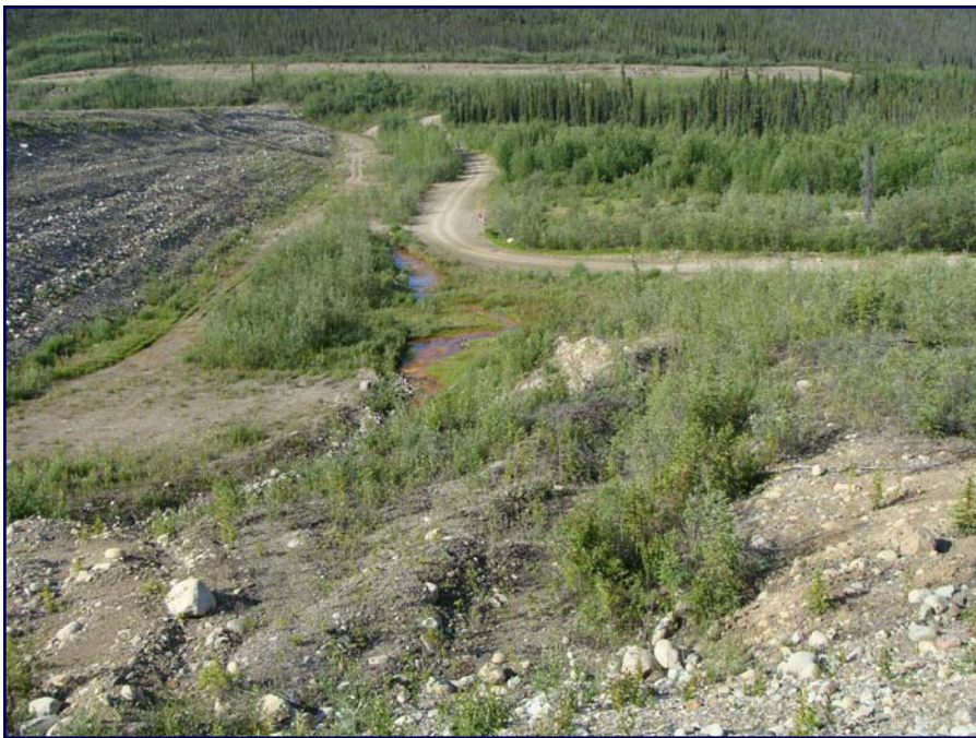
July: Overview of the downstream toe area of the dam.
