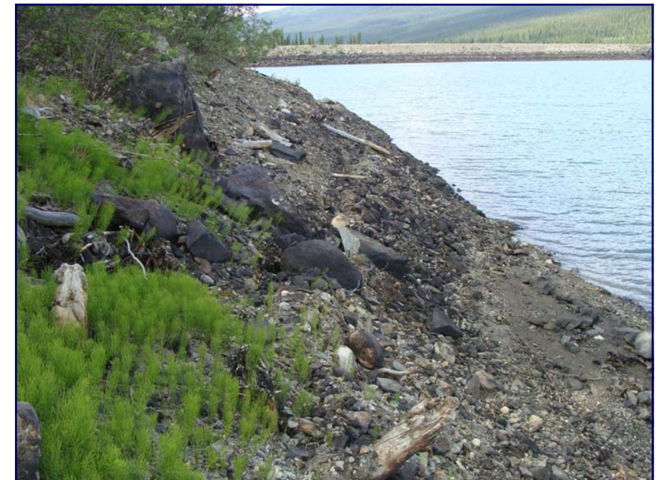
July: shows ice plucking damage to shoreline.
