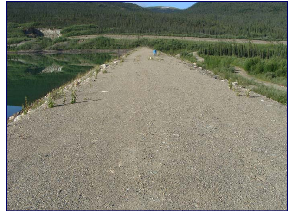
July: shows a view of the crest of the dam.
