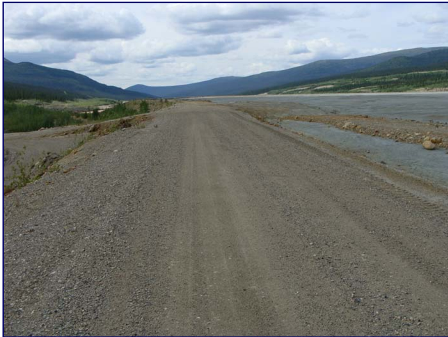
July: shows the crest of the Secondary Dam.
