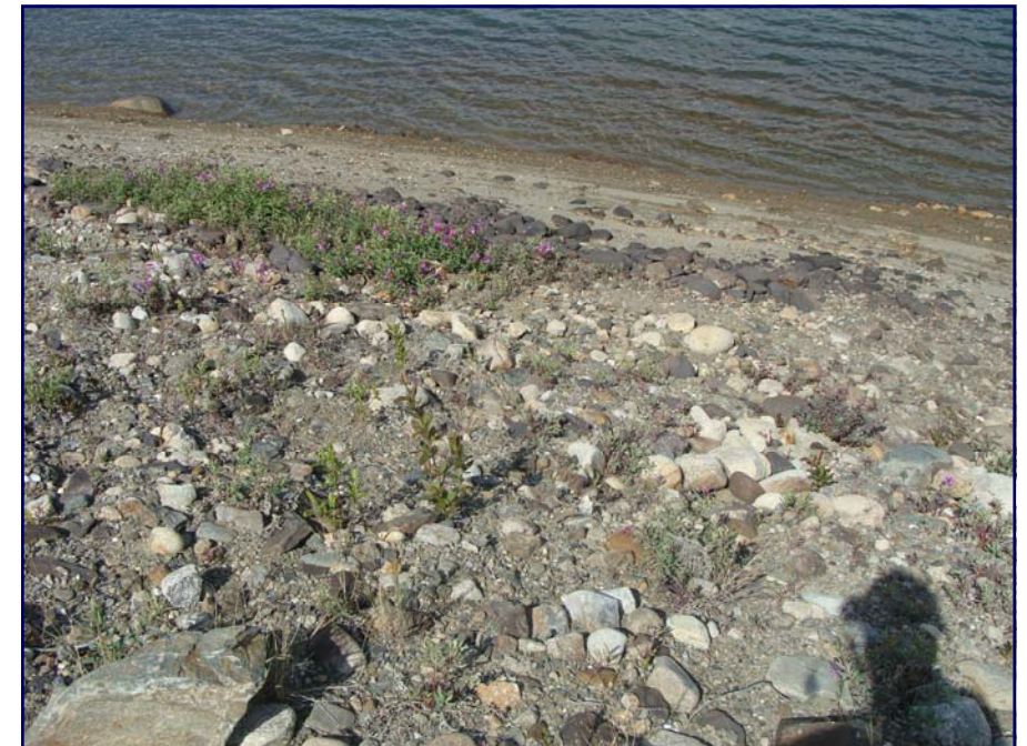
July: a view of the edge of the polishing pond, note some ice plucking damage to the riprap.
