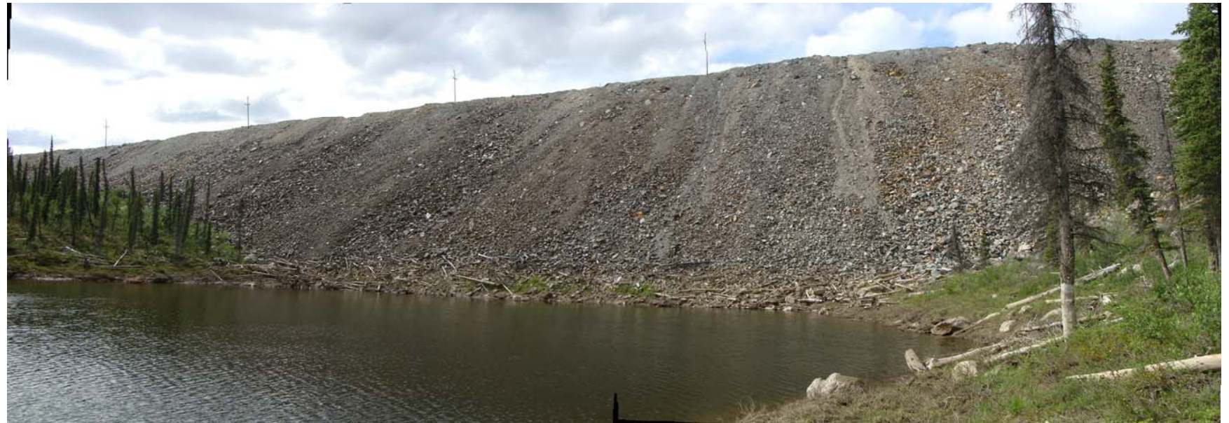
June: shows a panorama view of the upstream side of the North Fork Rock Drain
