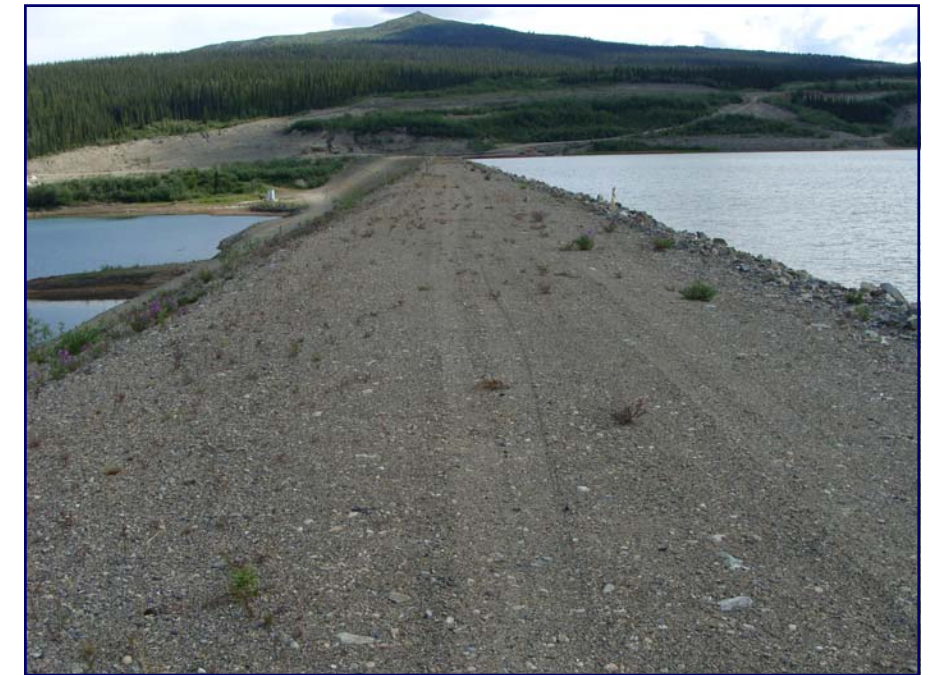
July: a view looking south along the crest of the dam.
