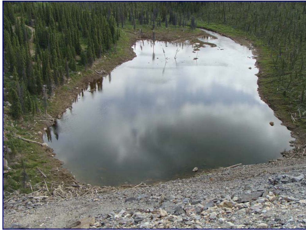
June: shows a view of the upstream head pond of the North Fork Rock Drain. Note that the pond level is higher than for the same flow 4 years ago. This appears to be due to beaver activity on the upstream face of the rock drain.
