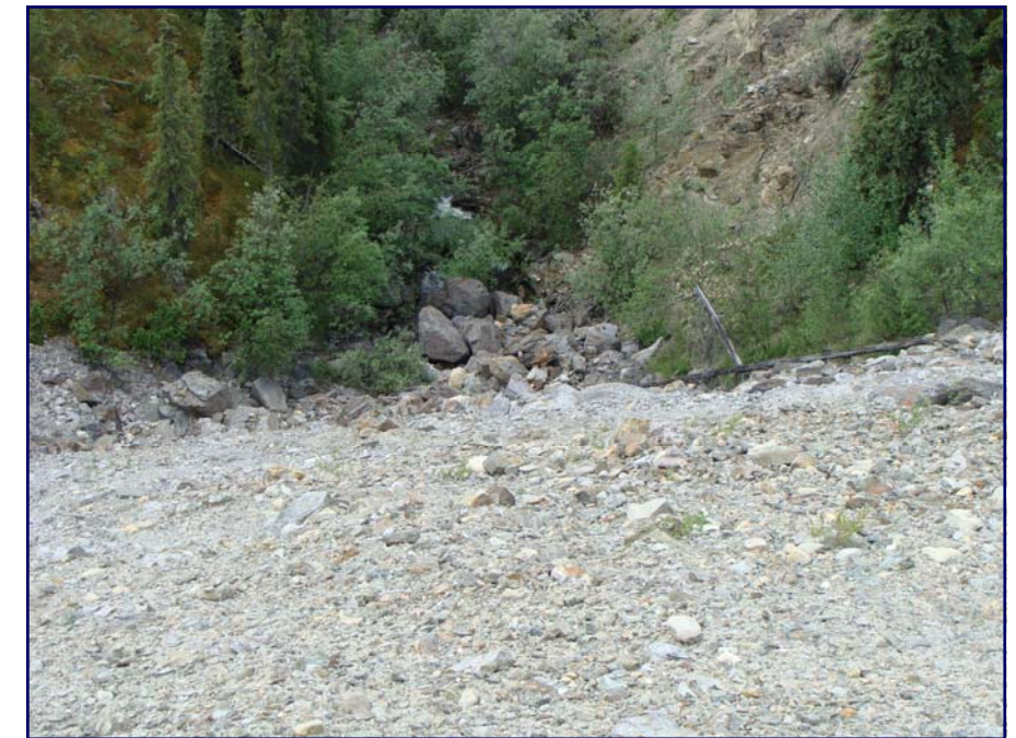
June: shows the downstream face of the rock drain with water flowing clearly from the toe.
