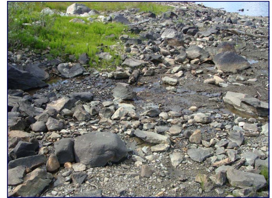
July: view of one of the larger seepage points in the spoil toe.
