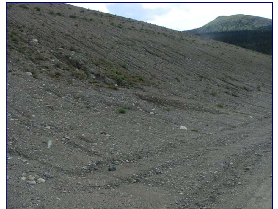
July: a view of the downstream face of the Intermediate Dam Note the appearance of the erosion rills on the face.
