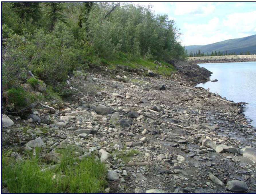
July: view of the polishing pond shoreline, which is formed by the spoil pile base. Note that this is an area of slumping and seepage.
