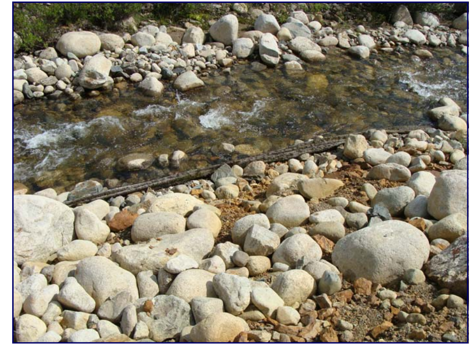
June: shows a view of an area with geotextile exposure.
