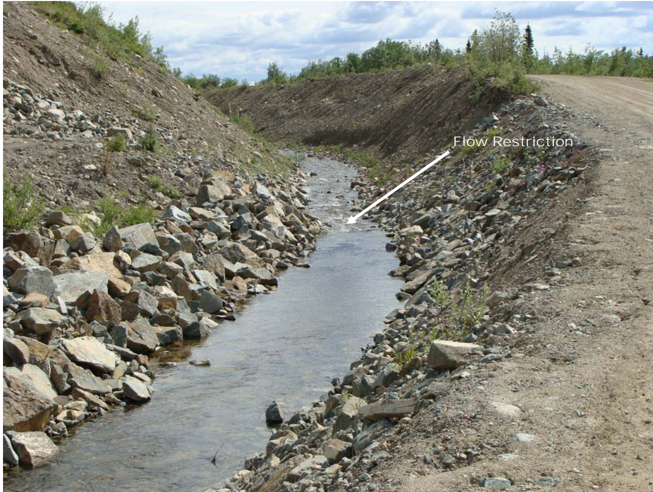
June: a view of the repaired slough area which was caused partially by over steepened banks. The area is still restricting the flow through the channel. Repaired in July 2009 by site staff.
