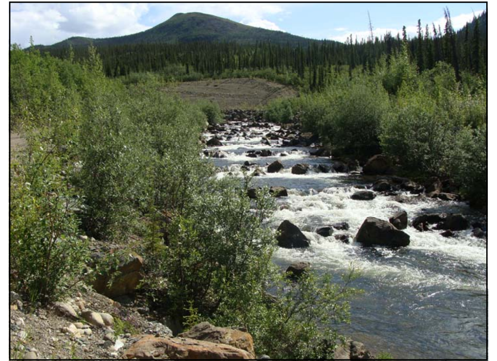
July: shows an upstream view of the upper weir section of the canal, looking towards Cornish Creek.
