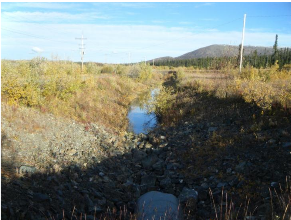
Photo 77 Interceptor Ditch upstream of Fresh Water Supply Pond - looking upstream (September 20, 2012)
