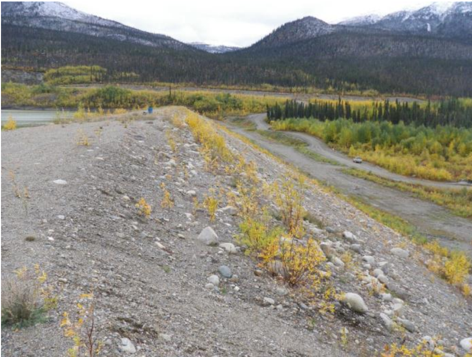
Photo 40 Crest and downstream slope - looking southwest (September 11, 2012)
