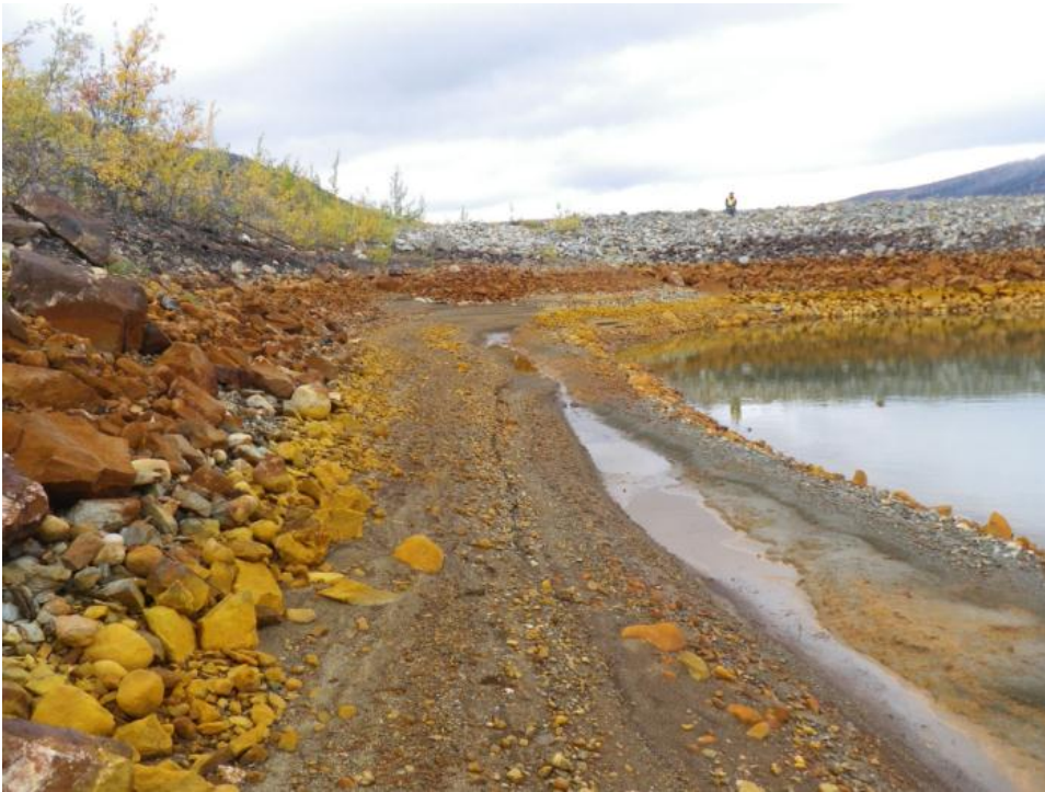
Photo 31 Northeast abutment of upstream slope (September 11, 2012)
