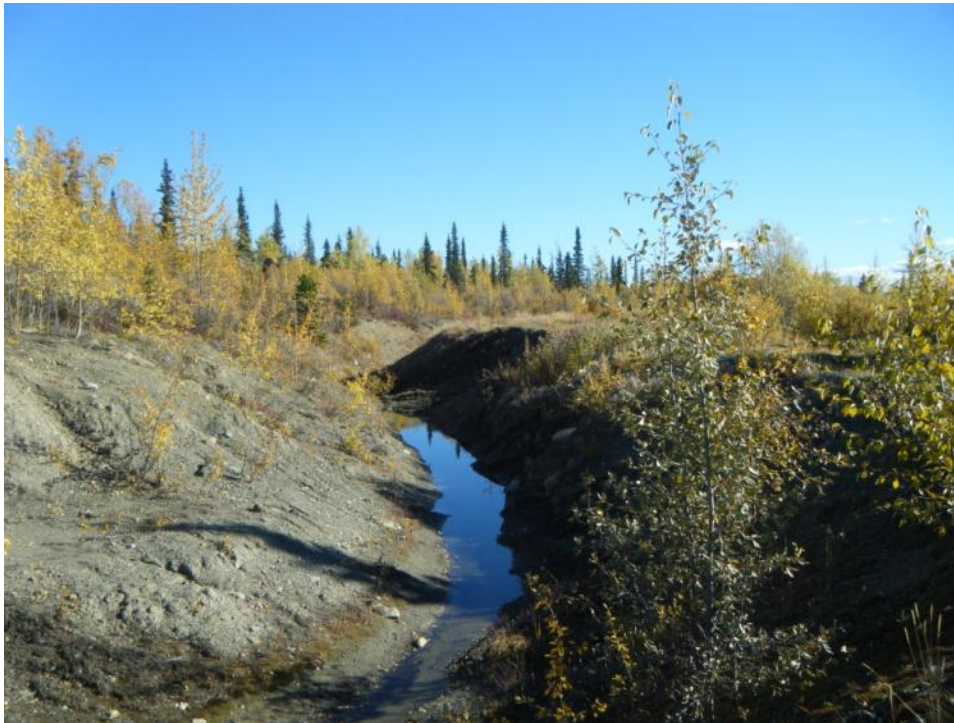
Photo 82 Interceptor Ditch – looking downstream (September 20, 2012)
