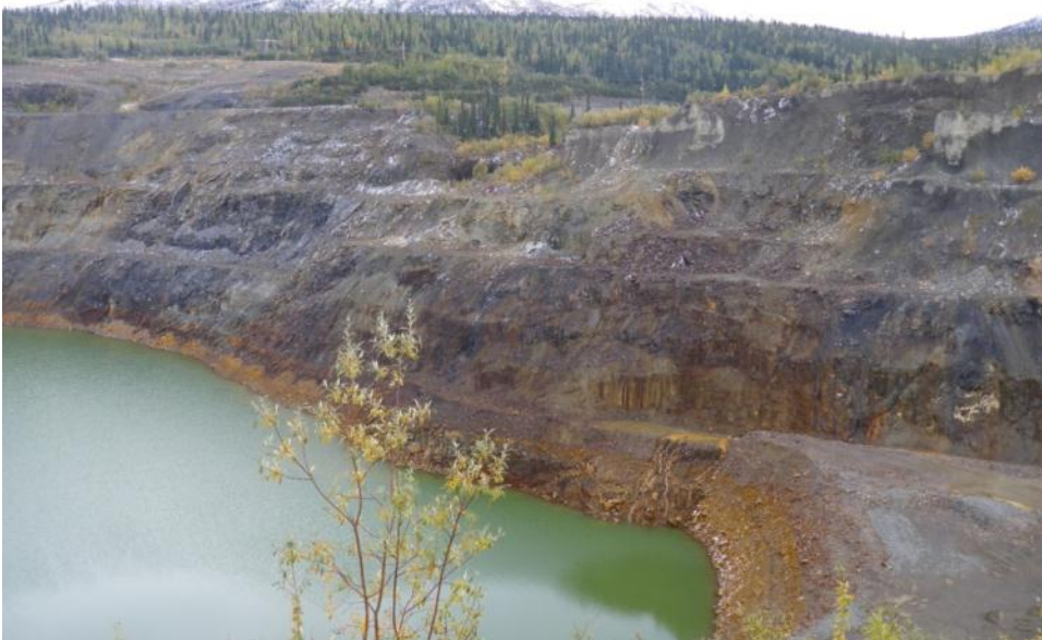
Photo 57 Pit southeast wall (September 12, 2012)
