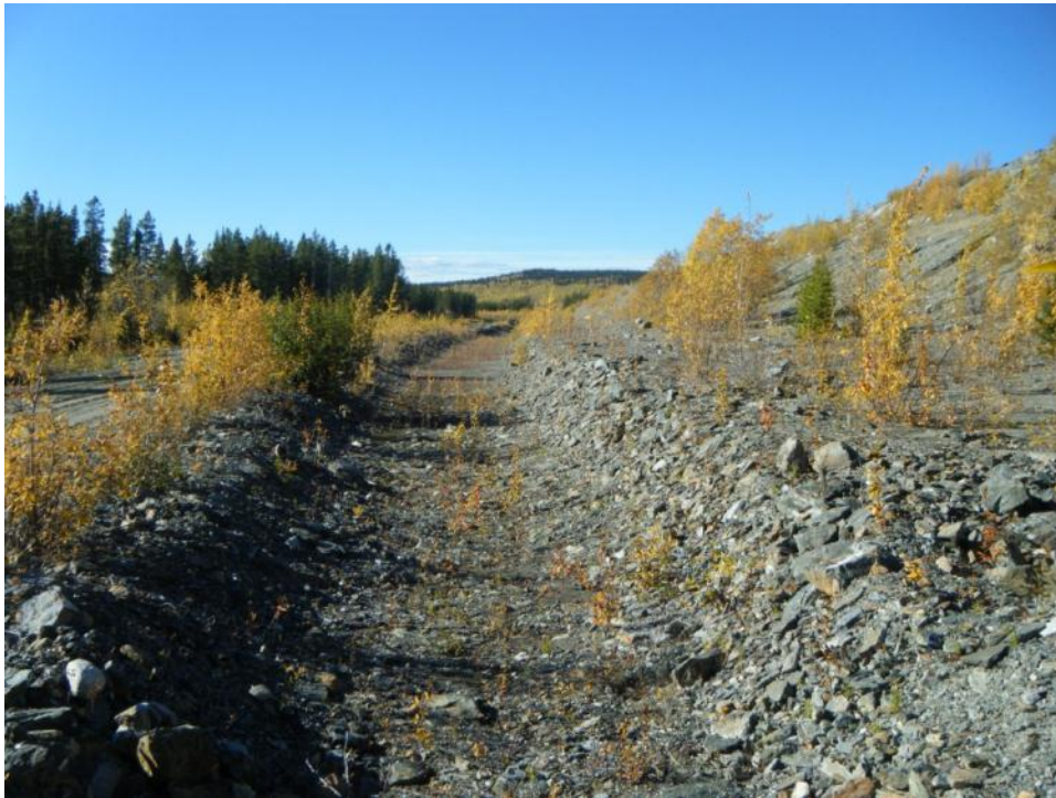
Photo 80 Interceptor Ditch near its upstream end – looking upstream (September 20, 2012)
