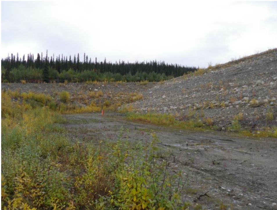
Photo 48 Downstream slope and berm – looking towards northeast (September 11, 2012)
