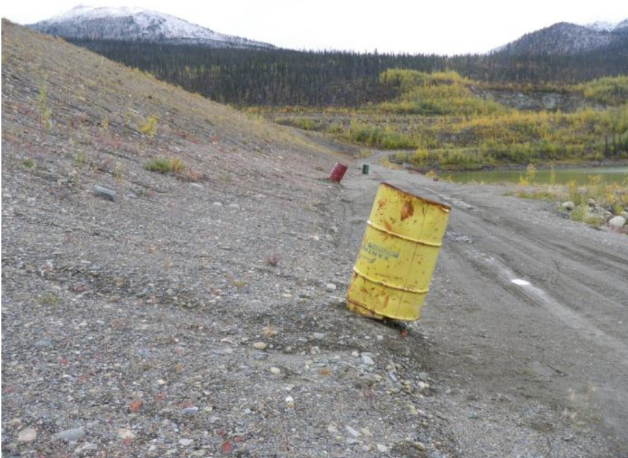
Photo 37 Southwest portion of downstream slope – note rill erosion at toe and tilted instrument-protection barrel (September 11, 2012)
