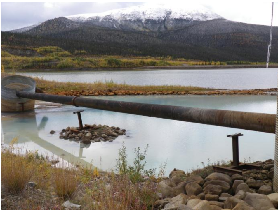
Photo 38 Discharge pipeline of treated water – note separation of pipeline and its intermediate supports)
