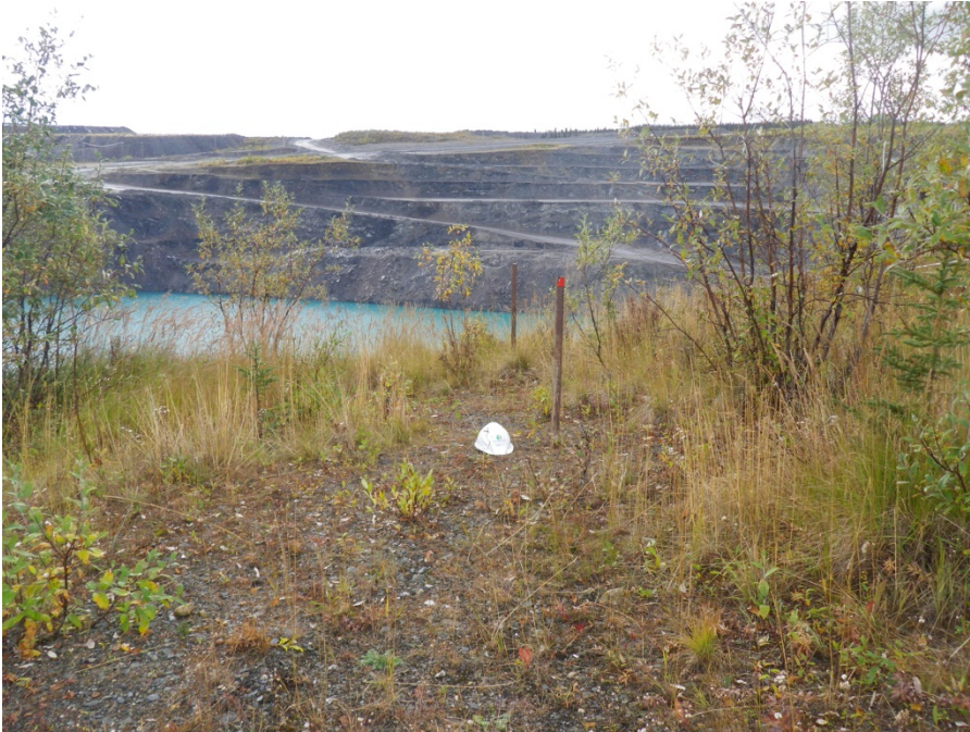
Photo 52 Reference Rods NP-1 and NP-2 along north array – crack noted at hard-hat location near NP-2 (September 12, 2012)
