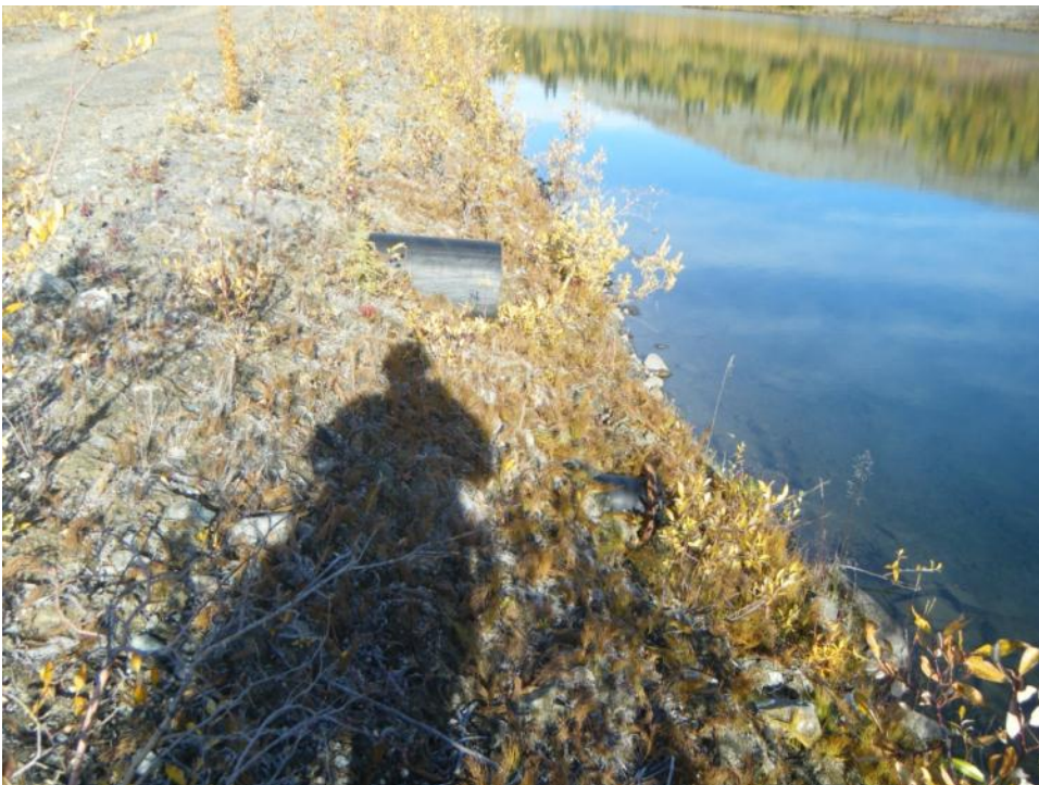
Photo 111 Culvert spillway for Lower Sheep Pad Pond (September 20, 2012)
