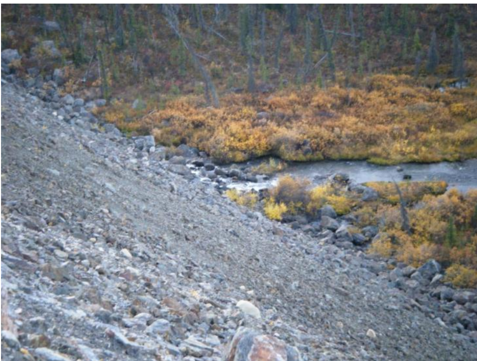
Photo 18 North Fork Drain outlet - downstream slope of access road between Faro and Vangorda Plateau (September 20, 2012)
