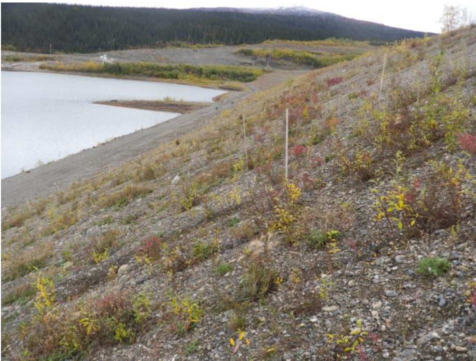
Photo 32 Rill erosion along lower portion of downstream slope (September 11, 2012)
