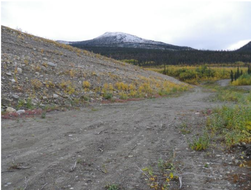
Photo 49 Downstream slope and berm – looking southwest (September 11, 2012)
