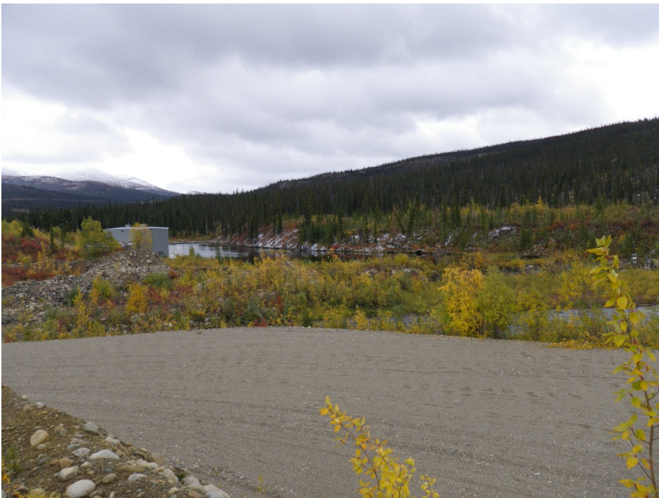
Photo 22 Downstream berm surface at southeast corner of Secondary Tailings Dam (September 11, 2012)
