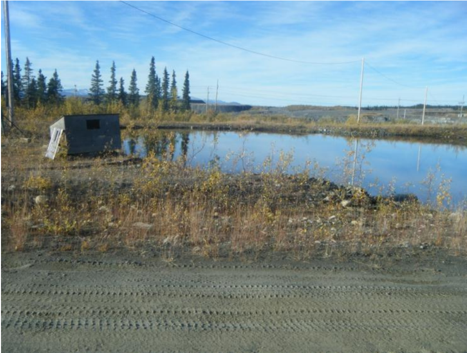
Photo 112 Grum Settling Pond (September 20, 2012)
