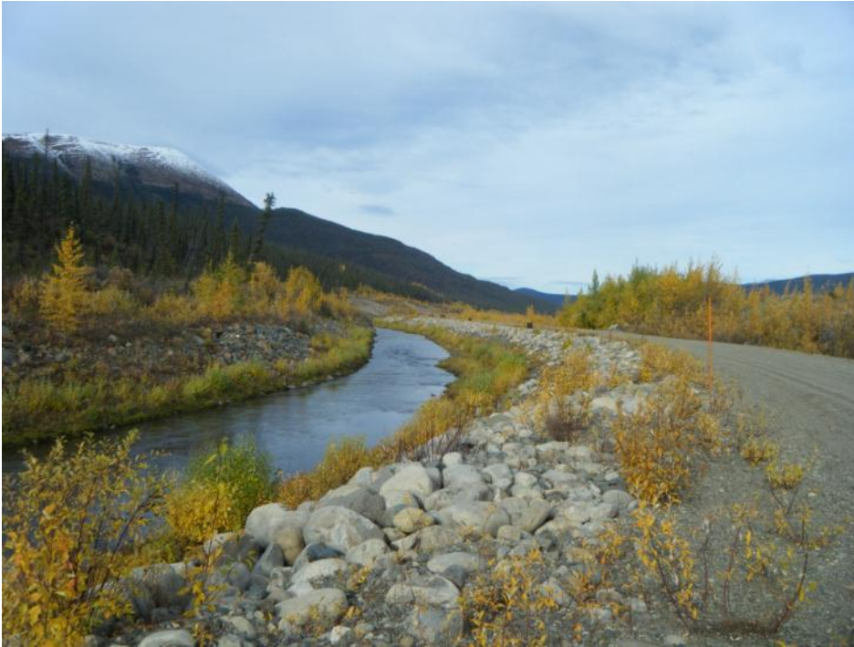
Photo 13 Rose Creek Diversion Channel adjacent to tailings impoundment (September 19, 2012)
