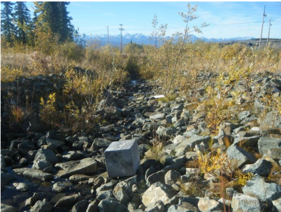
Photo 113 Pond spillway channel, looking downstream towards Grum Interceptor Ditch (September 20, 2012)
