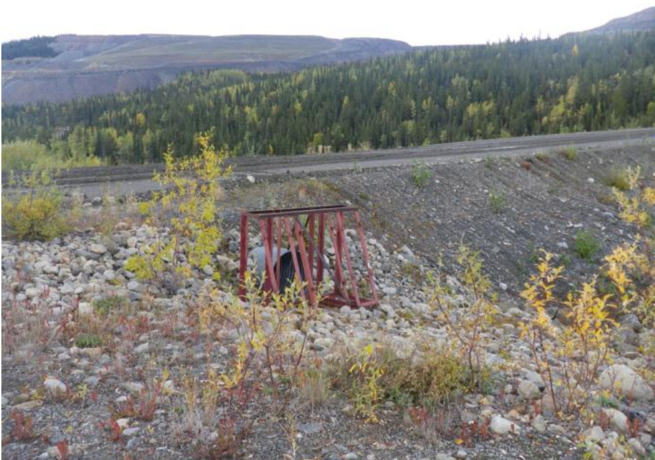
Photo 101 Upstream end of culvert emergency spillway at left (south) abutment (September 13, 2012)
