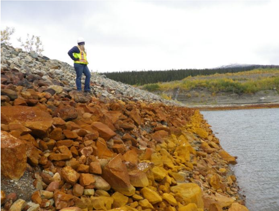
Photo 29 Wave erosion zone on upstream slope – note third marker rod installed by Brodie in 2010 in the foreground (September 11, 2012)
