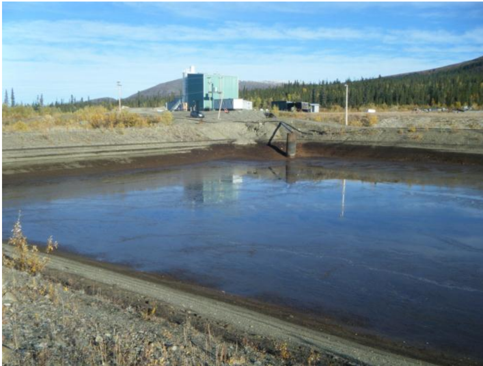
Photo 122 Grum Sludge Pond (September 20, 2012)
