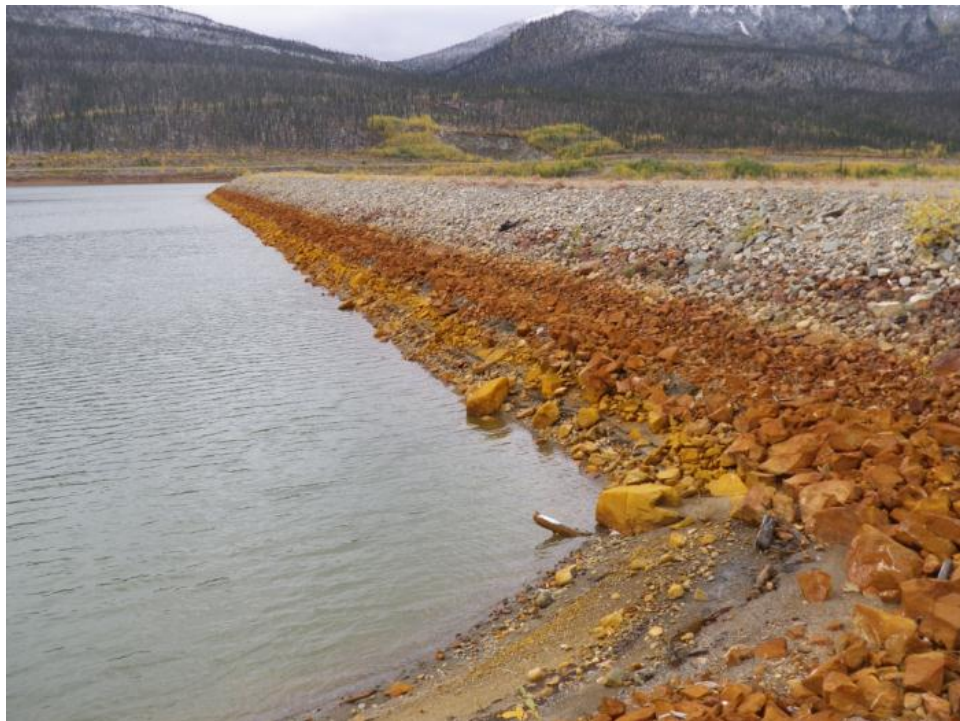
Photo 25 Upstream slope of Intermediate Dam – looking southwest (September 11, 2012)
