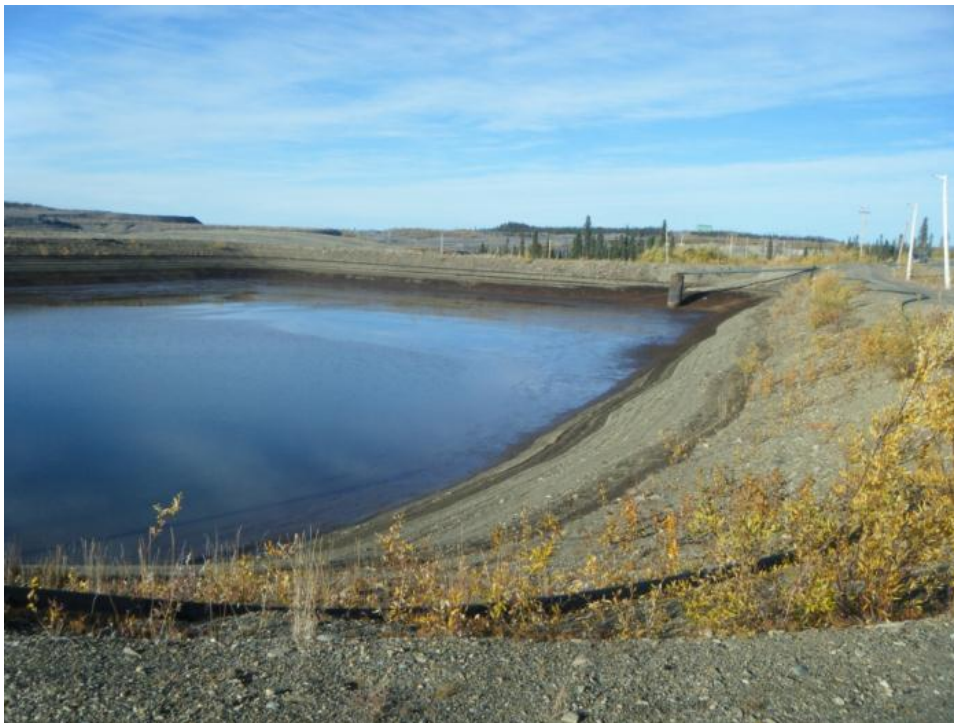
Photo 123 Grum Sludge Pond (September 20, 2012)
