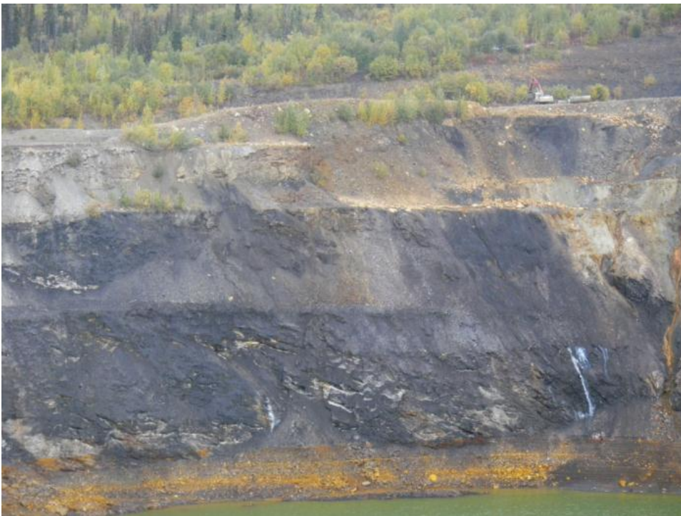
Photo 55 Pit north wall (September 12, 2012)
