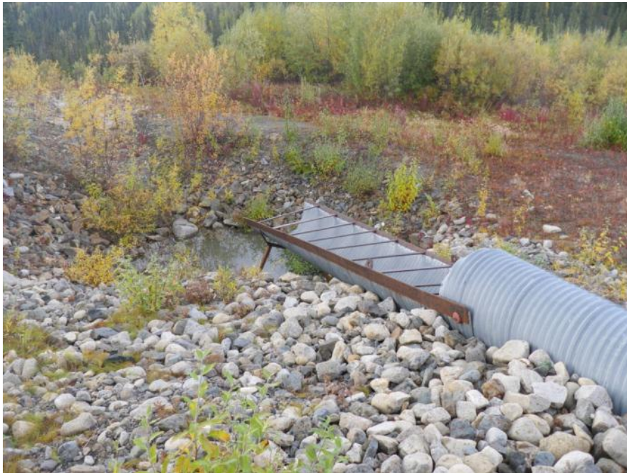
Photo 102 Downstream end of culvert spillway (September 13, 2012)
