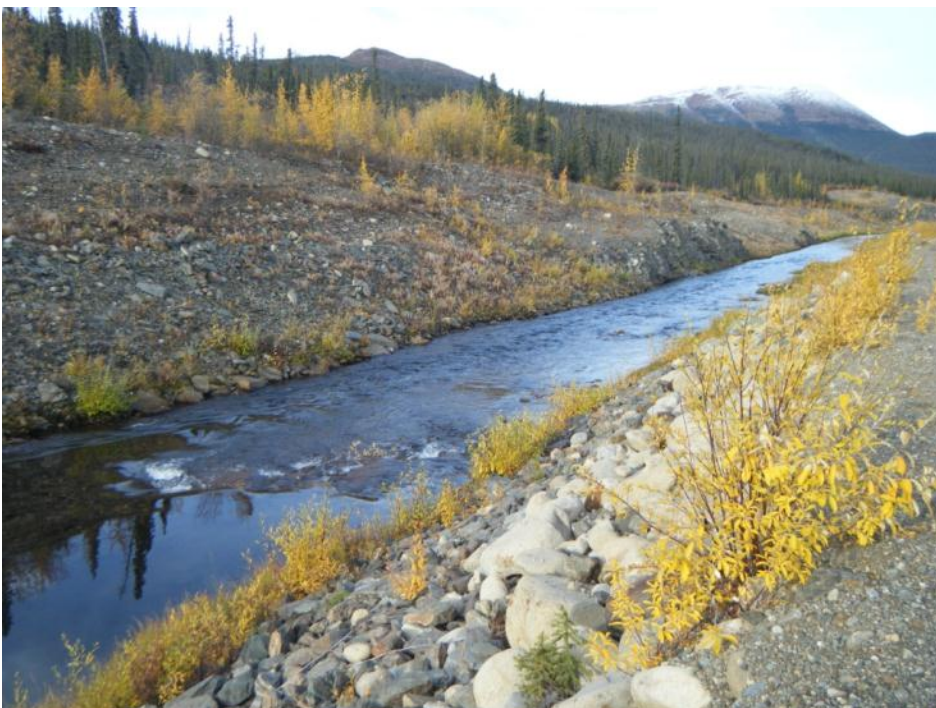
Photo 12 Rose Creek Diversion Channel downstream of fuse plug (September 19, 2012)
