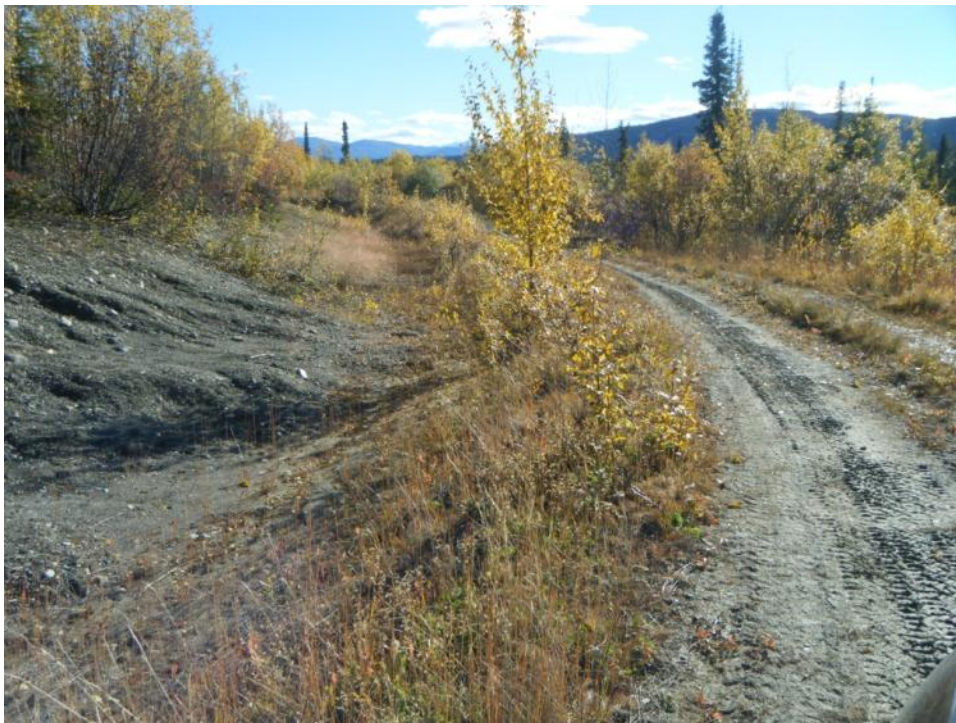
Photo 81 Interceptor Ditch – looking downstream (September 20, 2012)
