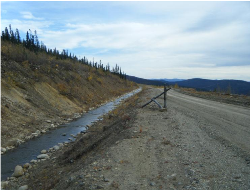
Photo 4 Faro Creek Diversion Ditch above Faro Pit, looking downstream (September 19, 2012)
