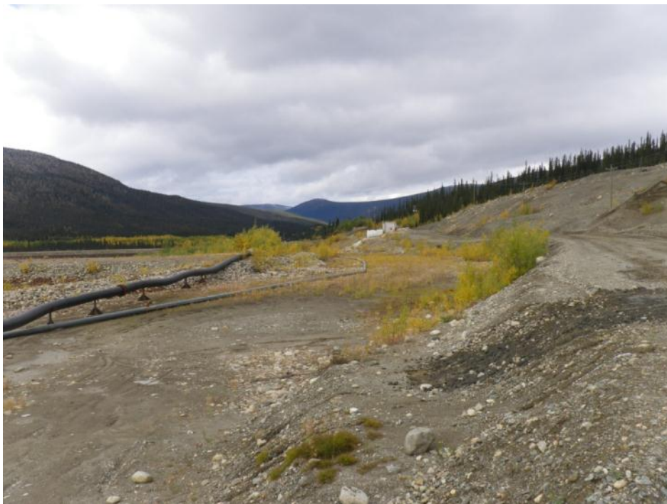
Photo 24 Spillway channel – looking downstream (September 11, 2012)
