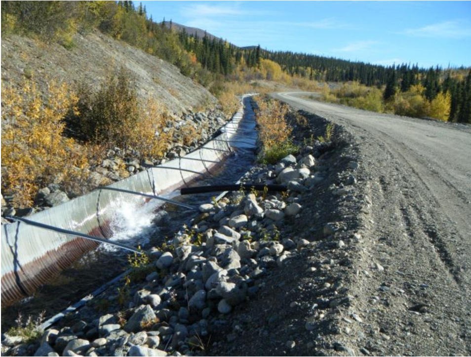
Photo 90 Pumped inflow of intercepted runoff collected below access road (September 20, 2012)
