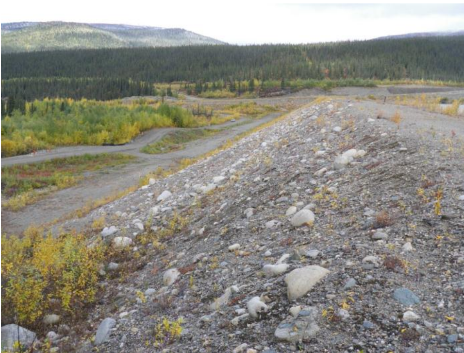
Photo 43 Crest and downstream slope - looking northeast (September 11, 2012)
