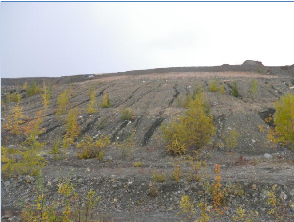
Photo 65 Waste Dump slope with rill erosion (September 13, 2012)
