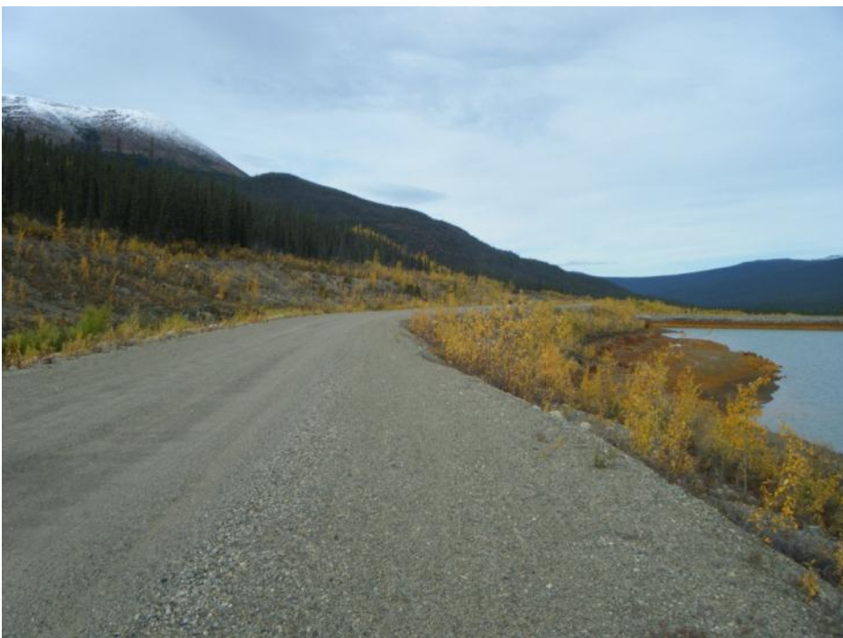
Photo 14 Rose Creek Diversion Channel (canal) dyke adjacent to Intermediate Dam (September 19, 2012)
