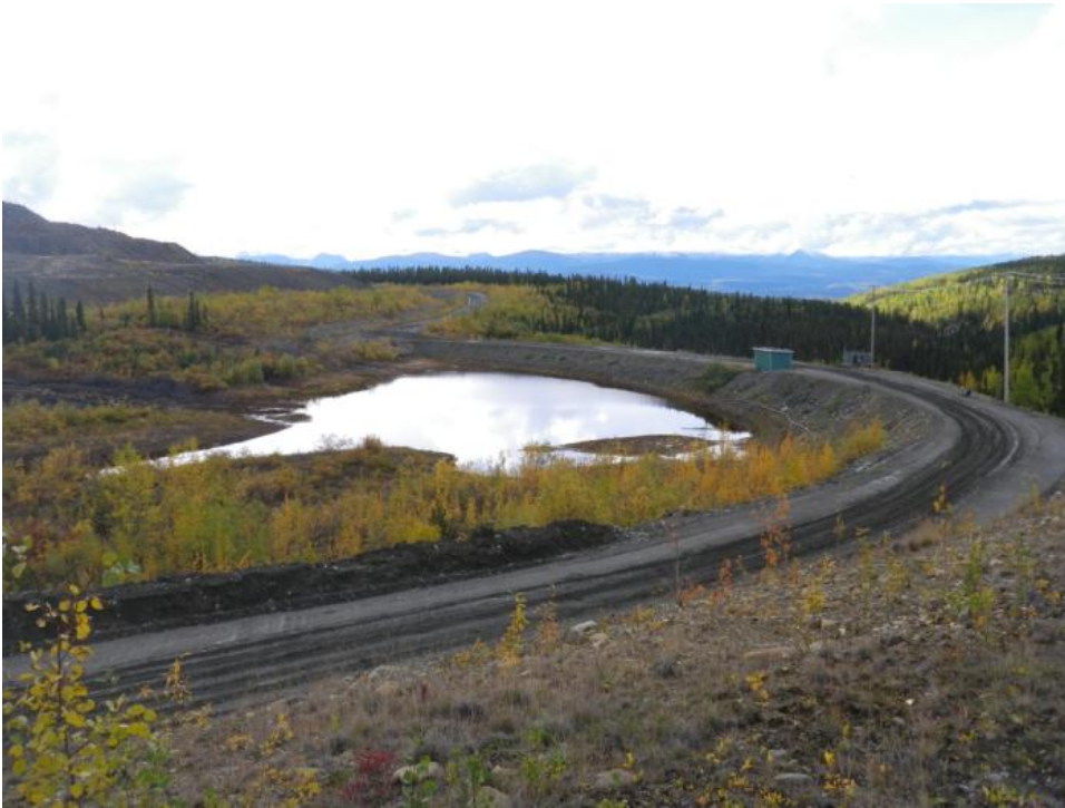
Photo 96 Dam crest/upstream slope and pond (September 13, 2012)
