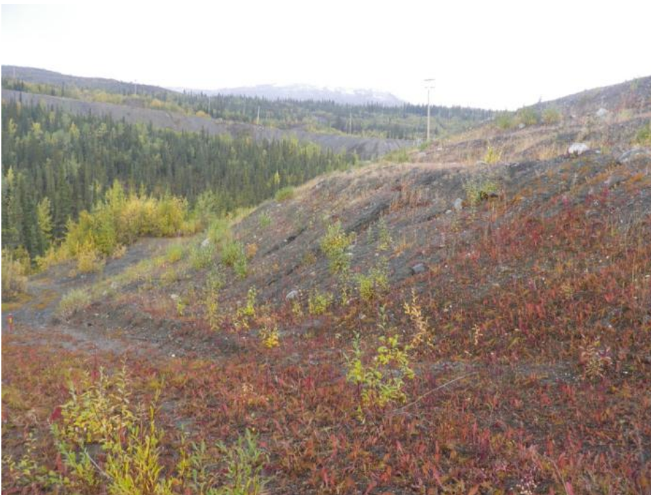
Photo 107 Downstream dam slope and berm – note piezometer at toe (September 13, 2012)
