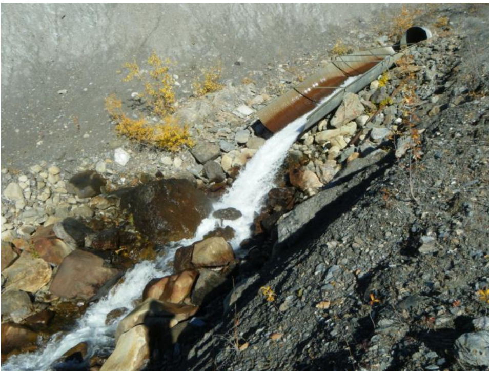
Photo 95 Vangorda Creek Diversion outfall at Vangorda Creek downstream of drop box (September 20, 2012)
