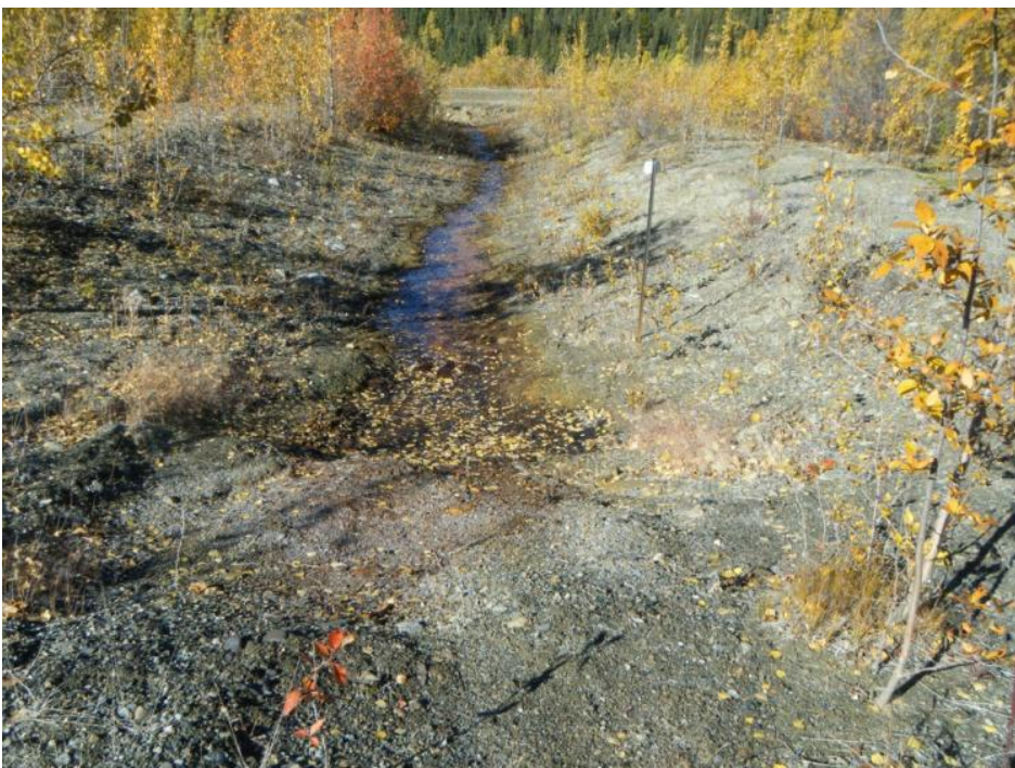
Photo 69 Vangorda Waste Dump Drain No. 4 looking downstream - no weir at this drain (September 20, 2012)
