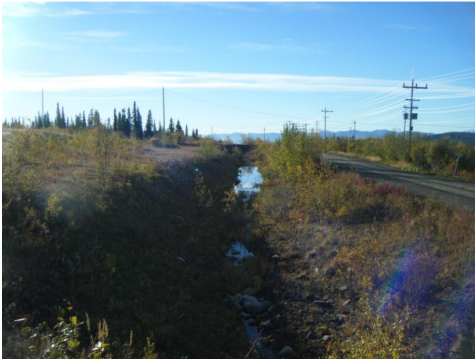
Photo 78 Interceptor Ditch near Fresh Water Supply Pond - looking downstream (September 20, 2012)
