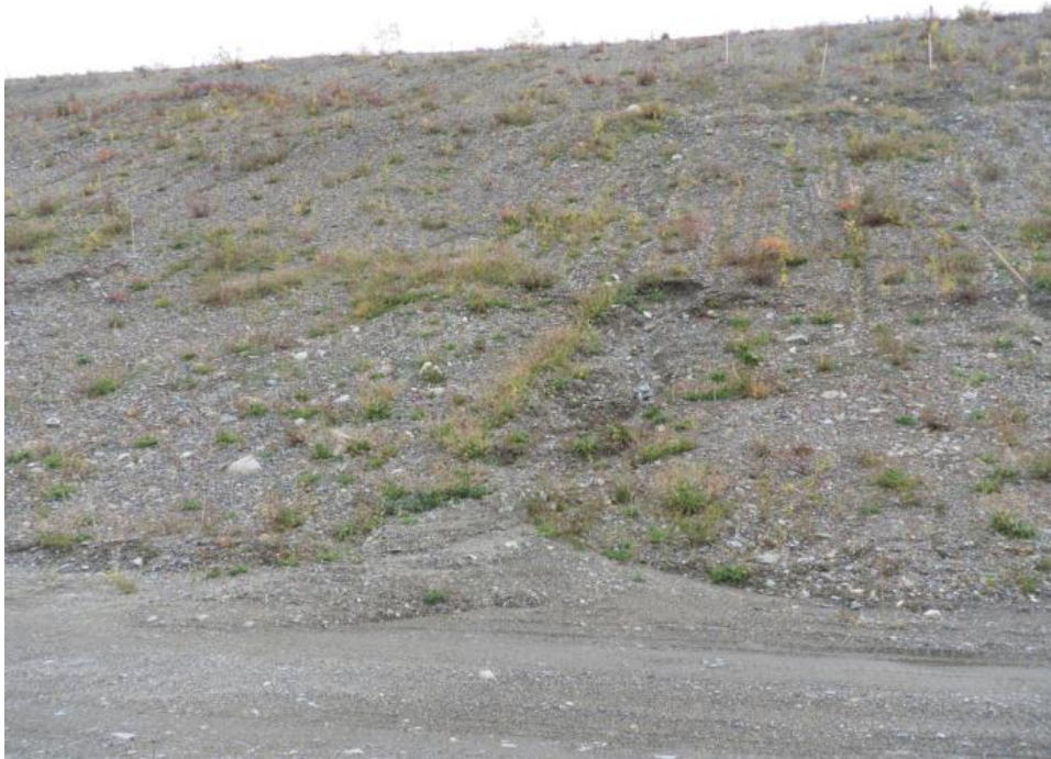
Photo 35 Downstream dam slope – looking up from downstream berm (September 11, 2012)
