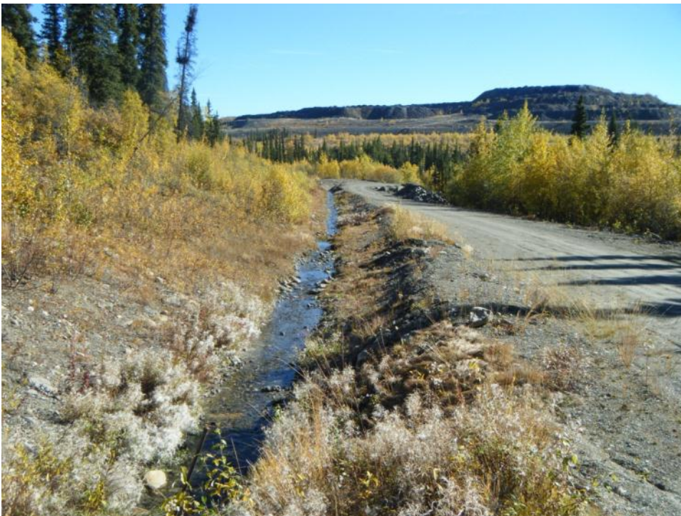
Photo 117 V-15 Diversion Ditch looking downstream towards Moose Pond (September 20, 2012)
