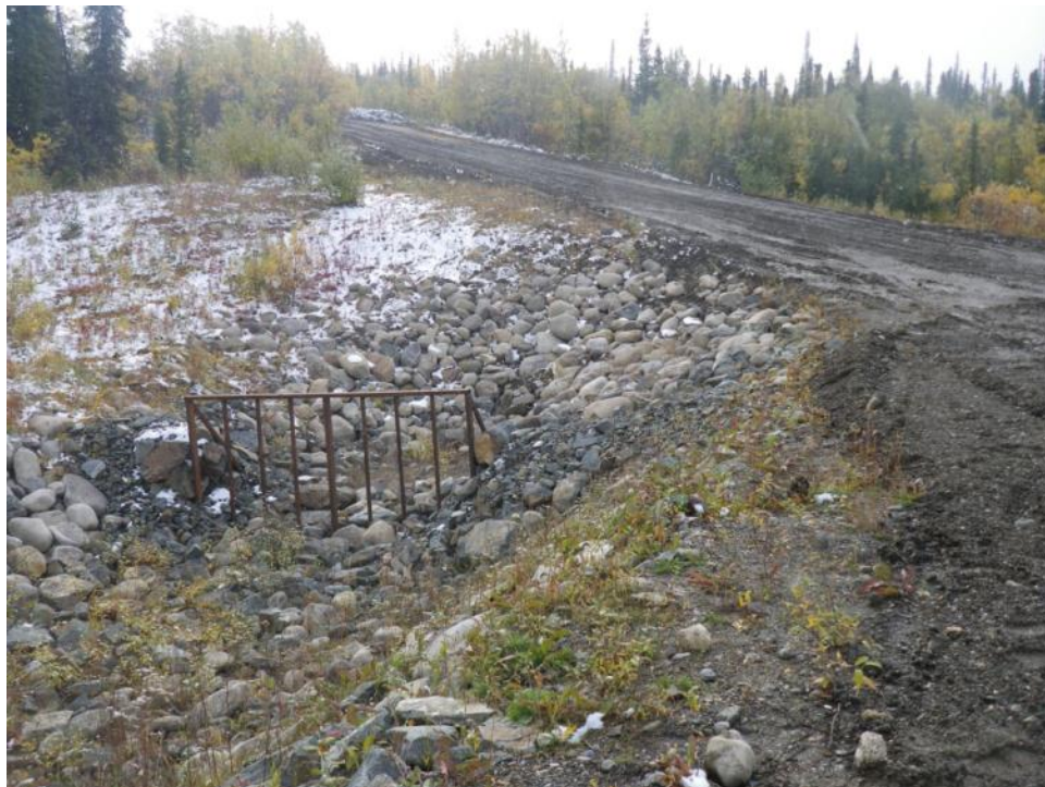
Photo 84 Flume emergency spillway intake culverts (behind trash rack) (September 12, 2012)
