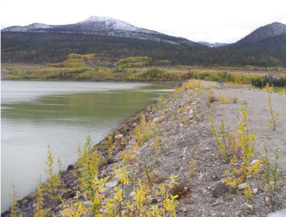
Photo 41 Crest and upstream slope – looking southwest (September 11, 2012)
