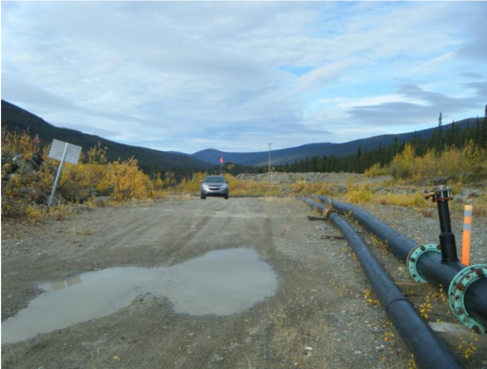
Photo 46 Cross Valley Pond siphon pipeline on spillway channel (September 19, 2012)
