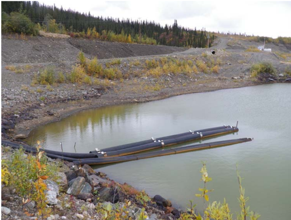
Photo 44 Cross Valley Pond siphon pipelines intake (September 11, 2012)
