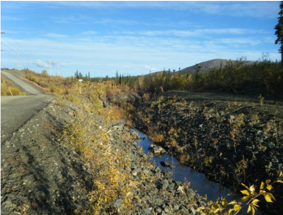
Photo 76 Interceptor Ditch near upstream end – looking upstream (September 20, 2012)
