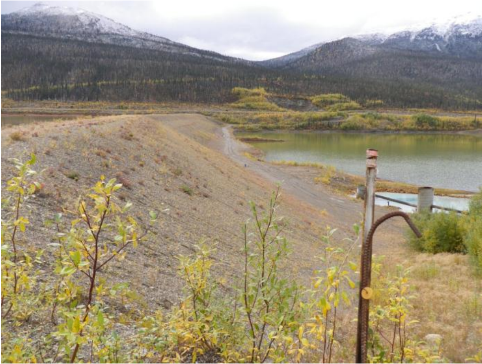
Photo 39 Downstream dam slope – looking from northeast abutment (September 11, 2012)
