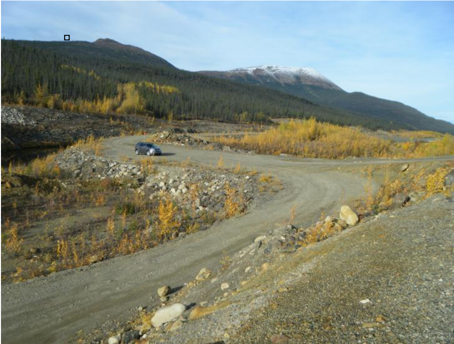
Photo 11 Rose Creek Diversion Channel fuse plug - looking towards Canal Dyke from Secondary Dam (September 19, 2012)
