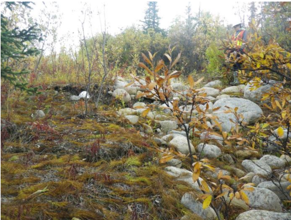
Photo 105 Spillway channel downstream end – note deep crack perpendicular to channel (September 13, 2012)
