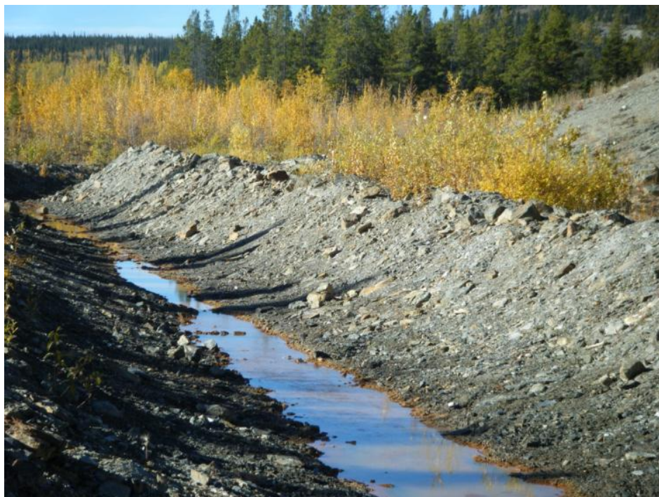
Photo 73 Seepage Collection Ditch downstream of Drain No. 3 - looking downstream (September 20, 2012)
