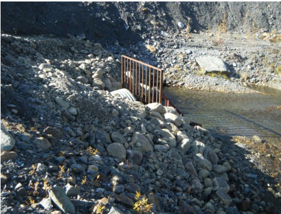
Photo 93 Flume plunge pool and culvert to drop box (September 20, 2012)
