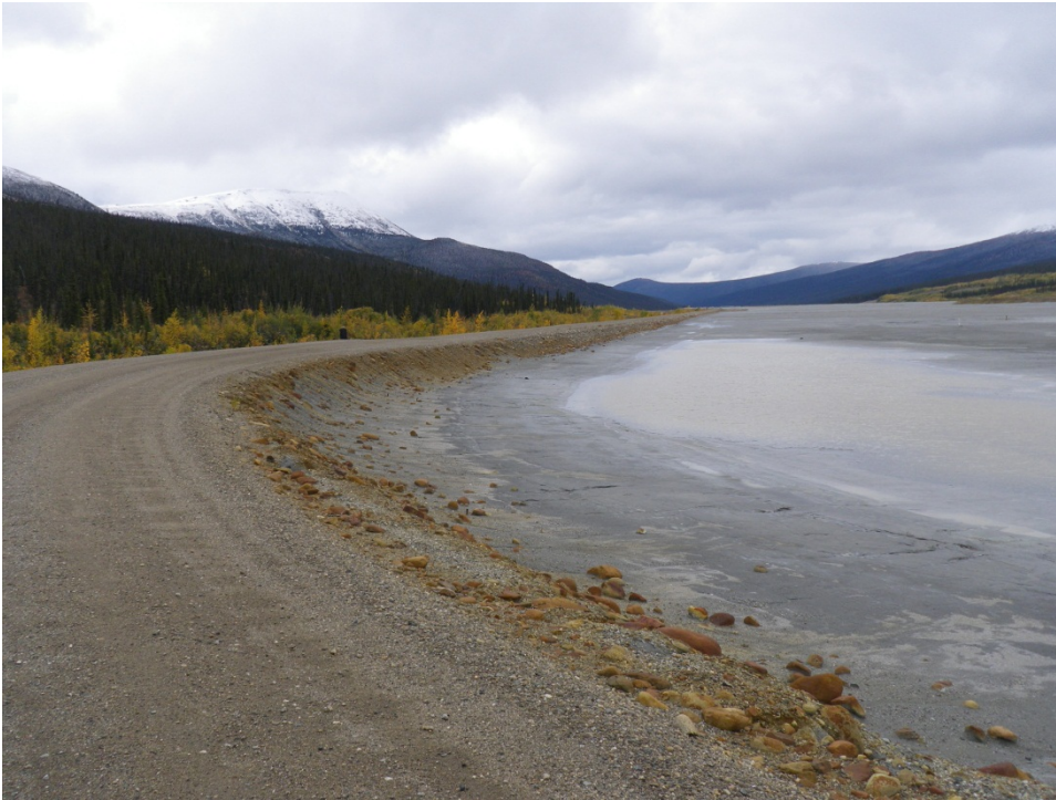
Photo 21 Southeast corner of Secondary Dam (September 11, 2012)
