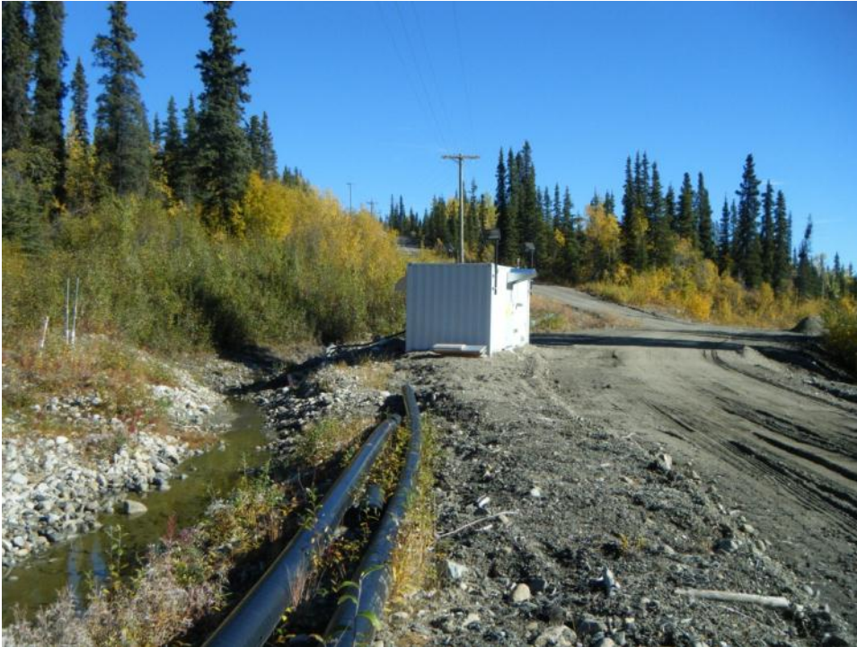
Photo 116 V-15 Pumphouse (September 20, 2012)
