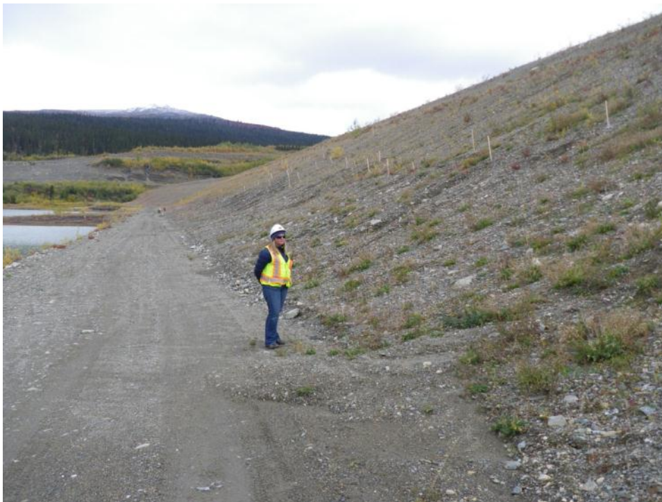
Photo 34 Downstream dam slope – looking northeast along toe (September 11, 2012)
