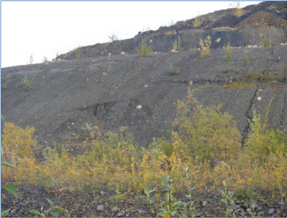
Photo 64 Waste Dump slope with old scarp and rill erosion (September 13, 2012)
