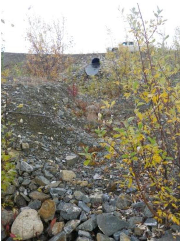
Photo 103 Spillway channel with relatively flat invert – looking upstream (September 13, 2012)
