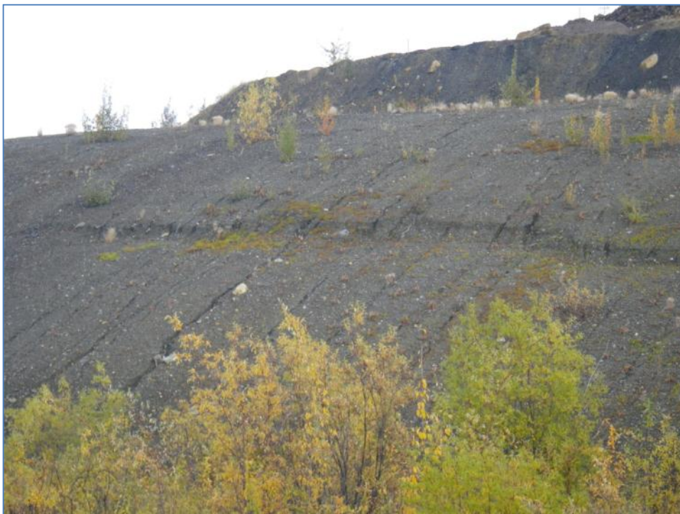
Photo 63 Waste Dump slope with old scarp and rill erosion (September 13, 2012)
