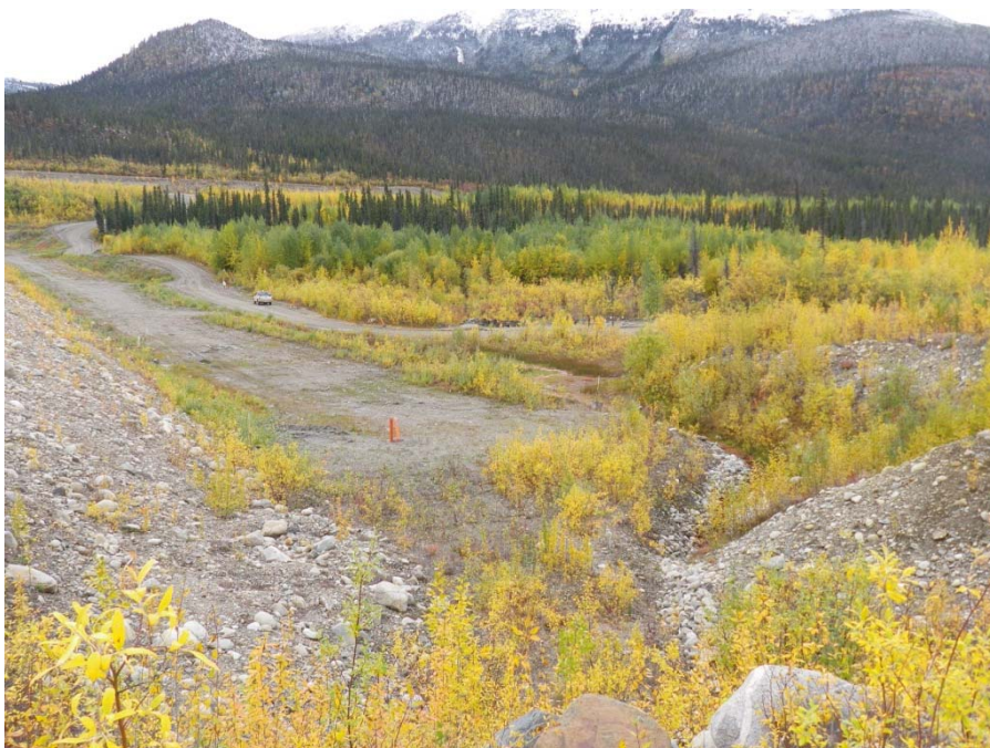
Photo 45 Downstream slope and berm – looking from northeast abutment (September 11, 2012)
