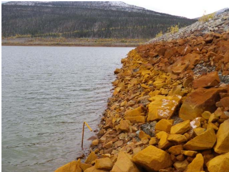
Photo 27 Wave erosion zone on upstream slope – note second marker rod installed by Brodie in 2010 in the foreground (September 11, 2012)
