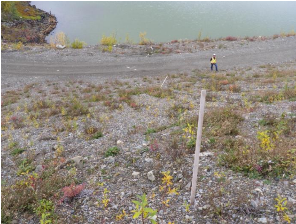
Photo 33 Lower portion of downstream slope – looking downslope (September 11, 2012)
