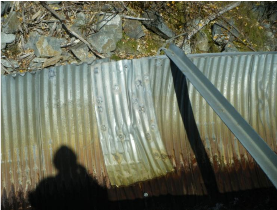
Photo 92 Repaired flume segment (September 20, 2012)
