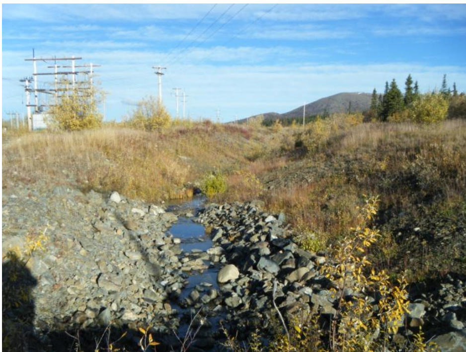
Photo 79 Interceptor Ditch near Grum Water Treatment Plant - looking upstream (September 20, 2012)
