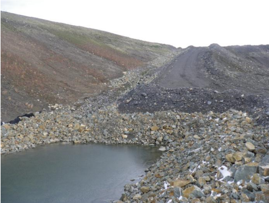
Photo 60 Dump side slope, water retention pond on bench and access ramp (September 12, 2012)
