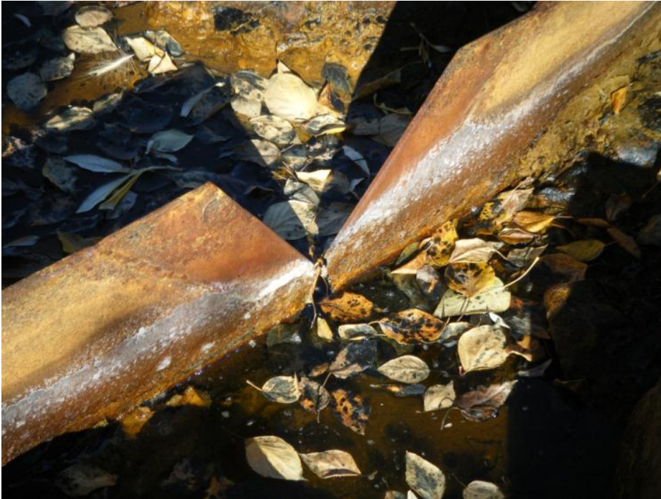
Photo 68 Vangorda Waste Dump Drain No. 5. Weir – weir plate split into two pieces at the V-notch (September 20, 2012)
