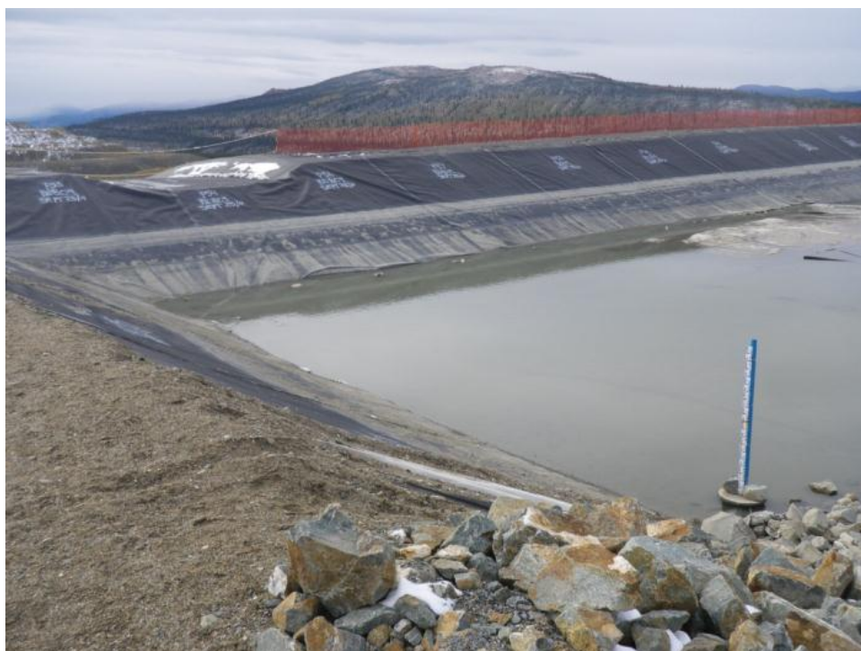
Photo 59 Grum Sulphide Cell water storage pond – side view (September 12, 2012)
