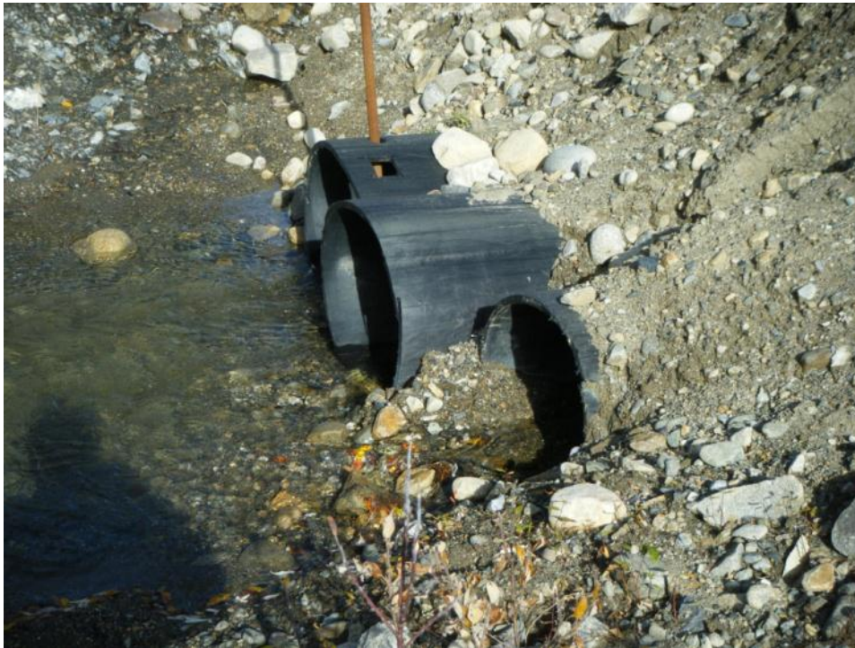
Photo 7 Downstream end of culverts at well access road (September 19, 2012)
