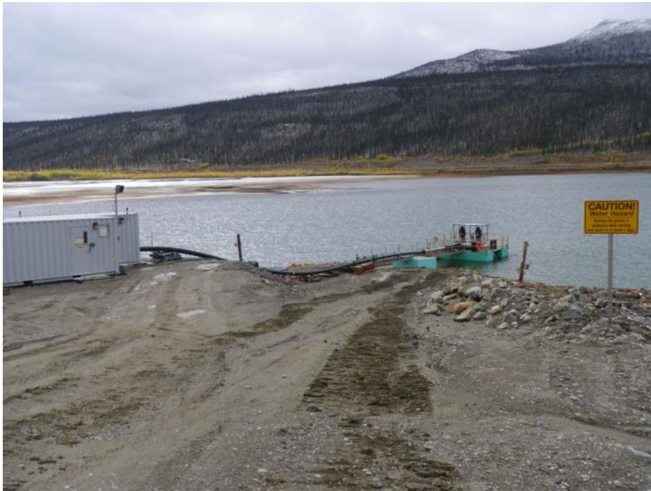
Photo 23 Upstream pump barge at northeast abutment (September 11, 2012)
