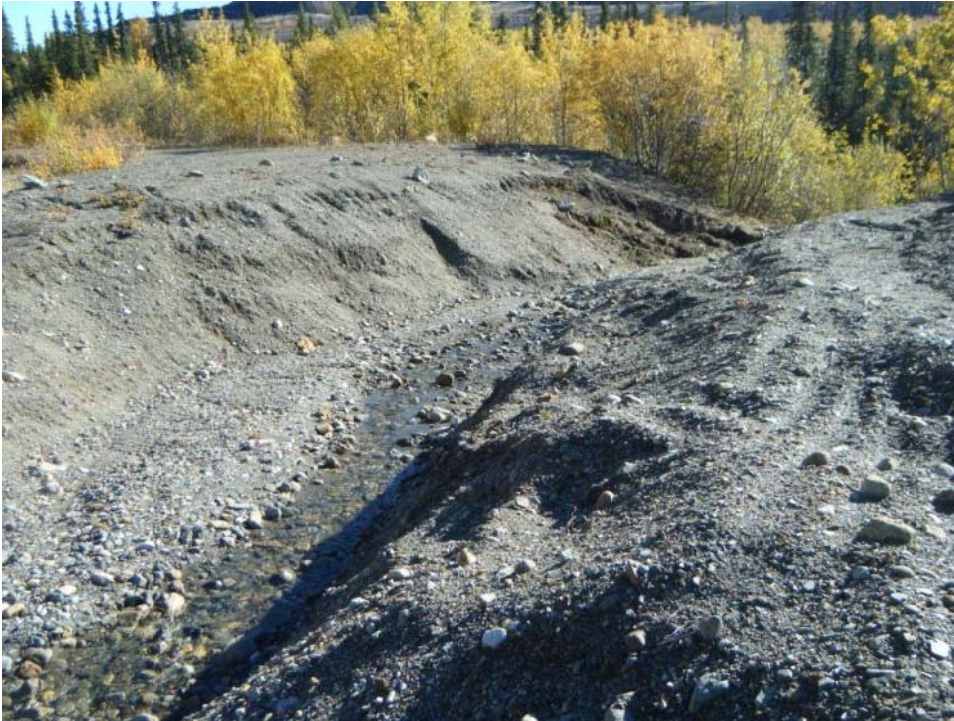
Photo 118 V-15 Diversion Ditch at its downstream end near Moose Pond (September 20, 2012)
