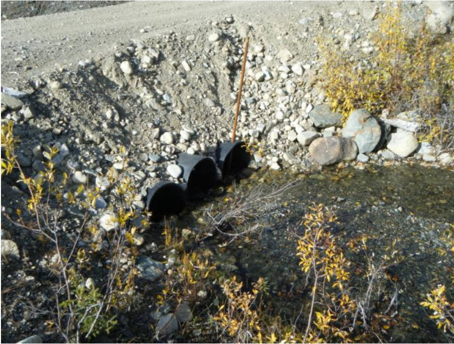
Photo 5 Interceptor Ditch upper reach at access road to potable water well upstream end of culverts (September 19, 2012)
