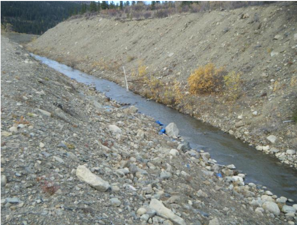
Photo 3 Faro Creek Diversion Ditch above Faro Pit, looking upstream (September 19, 2012)
