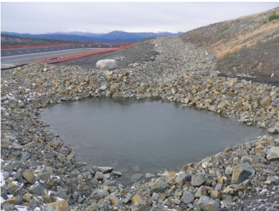
Photo 61 Water retention pond on bench – Grum Sulphide Cell in background (September 12, 2012)
