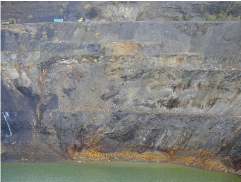
Photo 56 Pit northeast wall (September 12, 2012)
