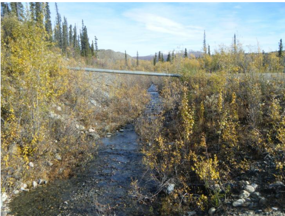
Photo 6 Upper reach of Interceptor Ditch looking upstream from well access road. (September 19, 2012)
