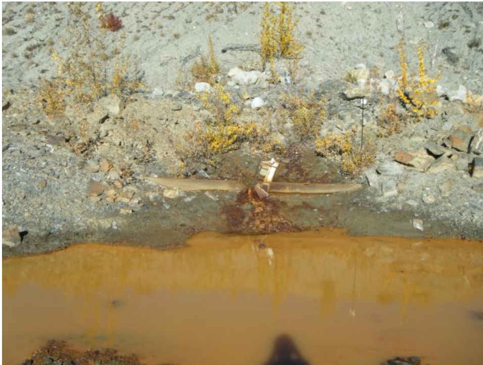
Photo 70 Vangorda Waste Dump Drain No. 3 weir (September 20, 2012)
