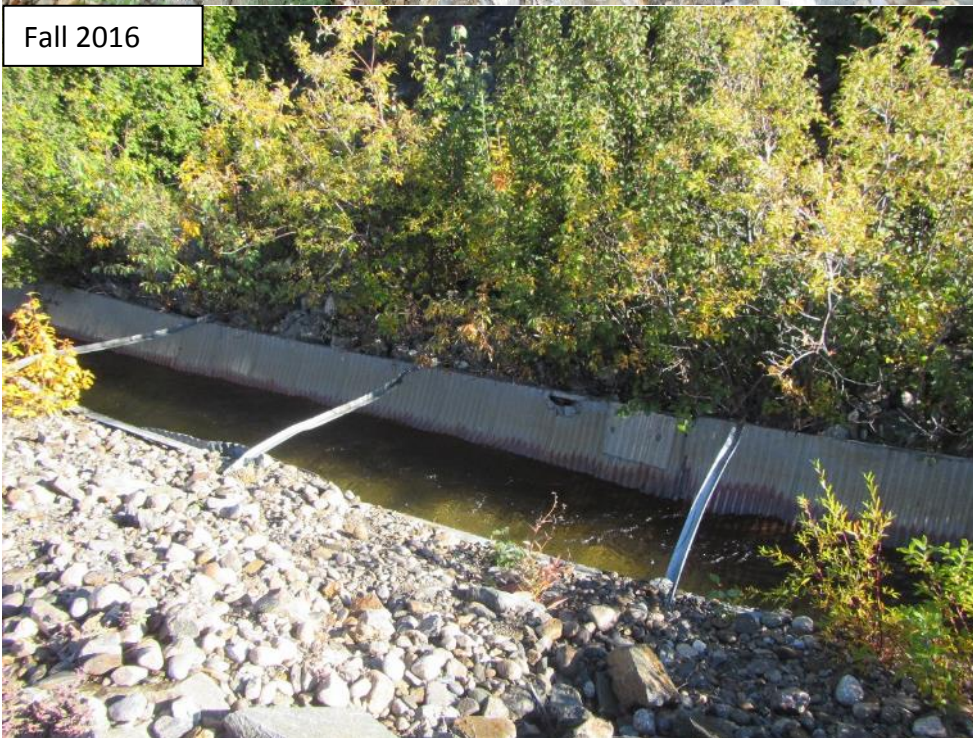
Photograph 51 Flat slope section, overtops during high flow
