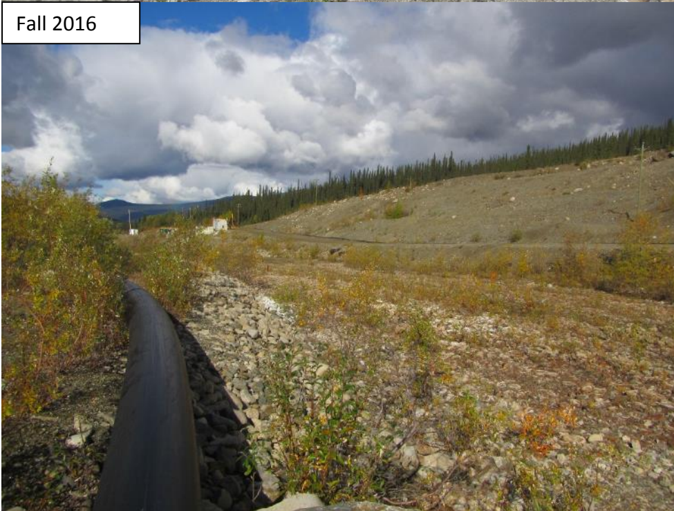
Photograph 28 Spillway, looking downstream. Pipeline in the spillway was removed in Fall 2016.
