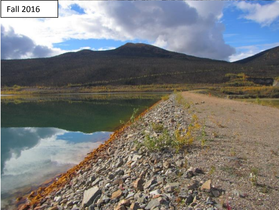
Photograph 25 Intermediate Dam from access road, looking south. Satisfactory conditions.
