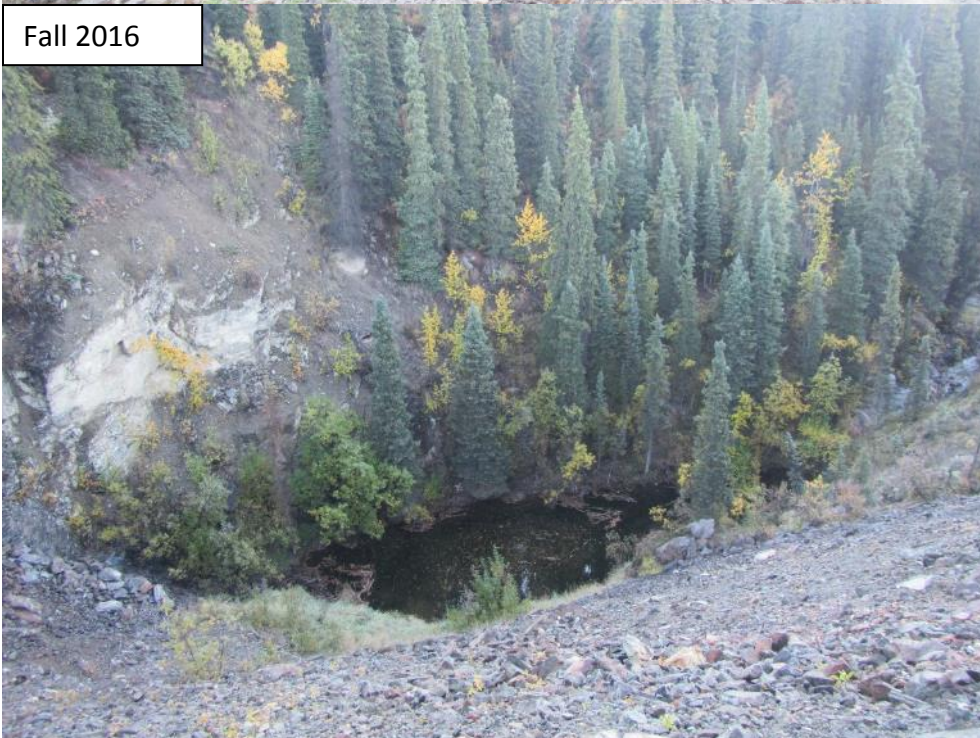
Photograph 21 K8 Rock Drain upstream pool. Satisfactory conditions.
