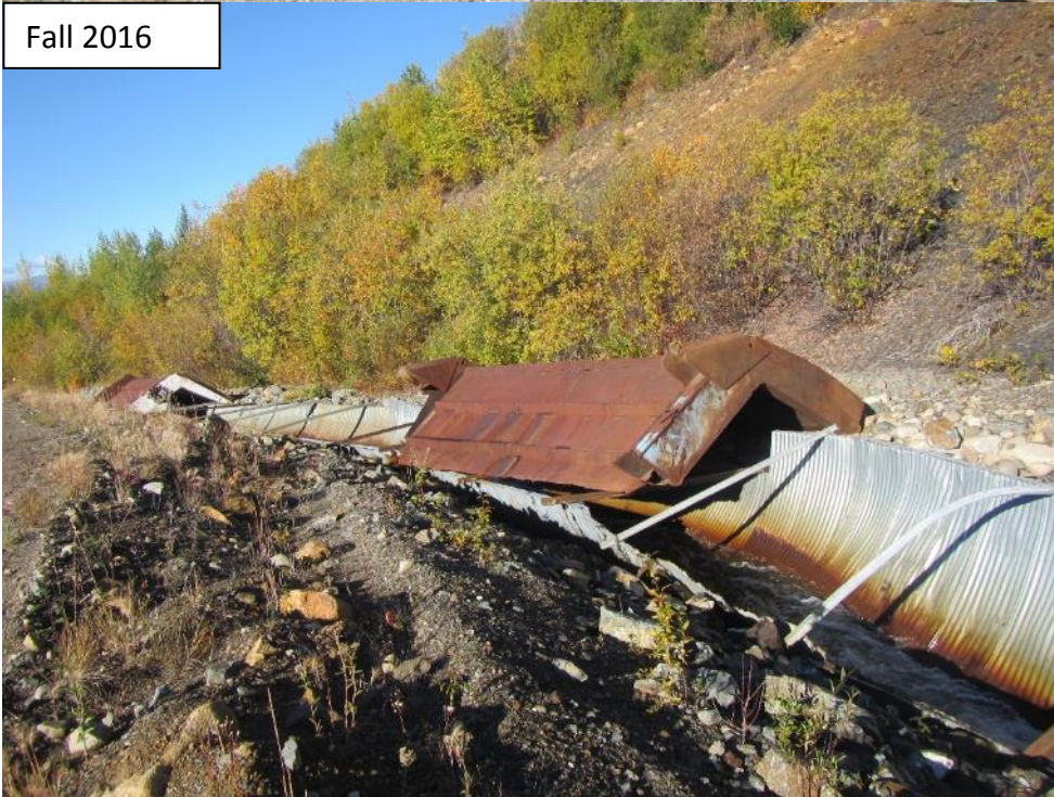
Photograph 49 Weight added to flume for anchoring
