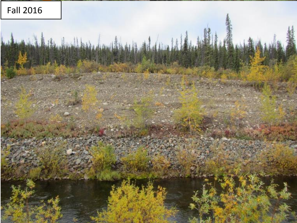
Photograph 17 Rose Creek Diversion Channel Proposed Back Slope Observation Location C. Conditions similar in spring and fall.
