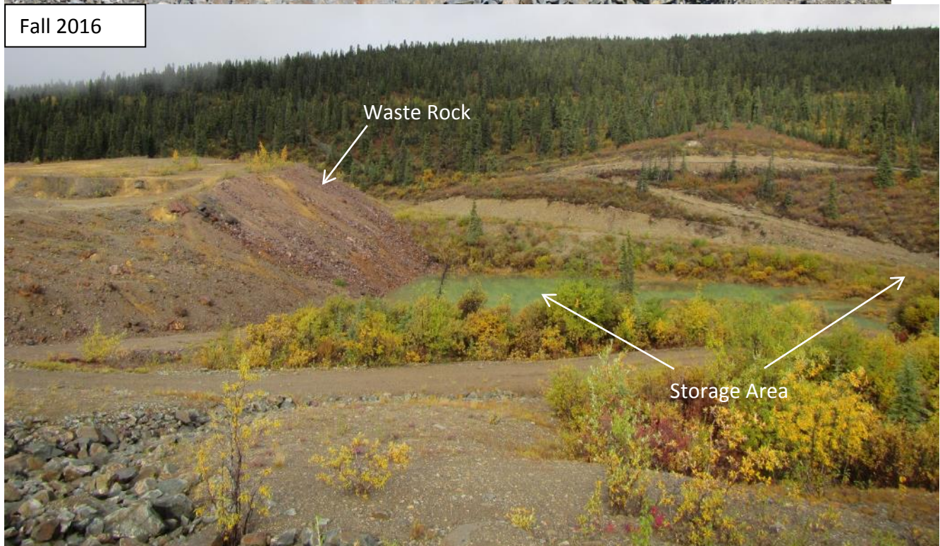
Photograph 3 Faro Creek Diversion Overflow (FCO) Sump (looking west)
