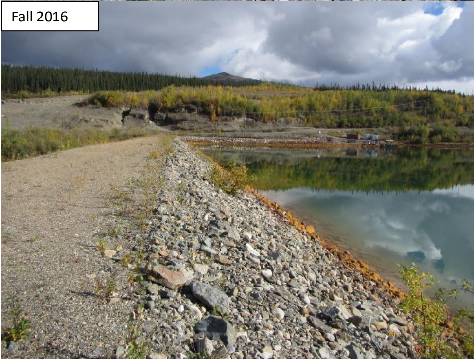
Photograph 26 Intermediate Dam crest and upstream slope, looking north. Satisfactory Conditions.
