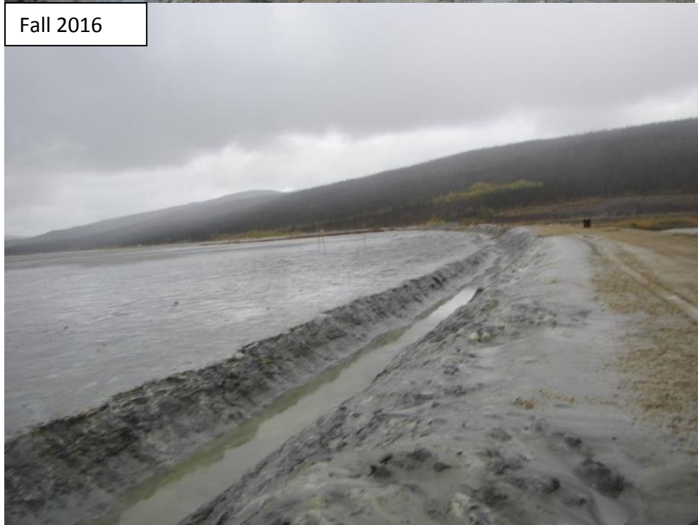
Photograph 23 Secondary Tailings Dam upstream ditch looking south. Ditch appears deeper since spring.
