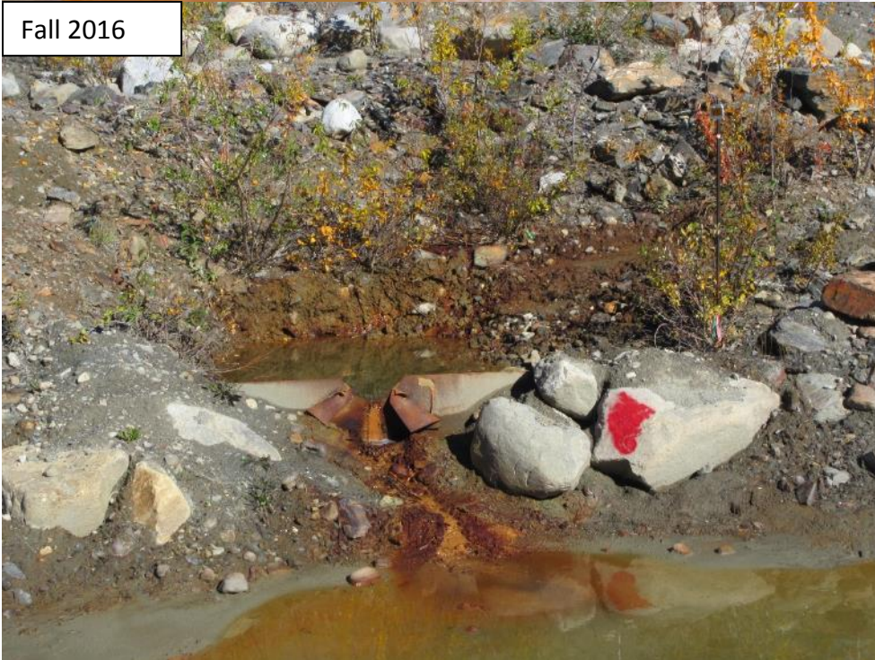
Photograph 37 Drain No. 3 (V30). Satisfactory conditions.
