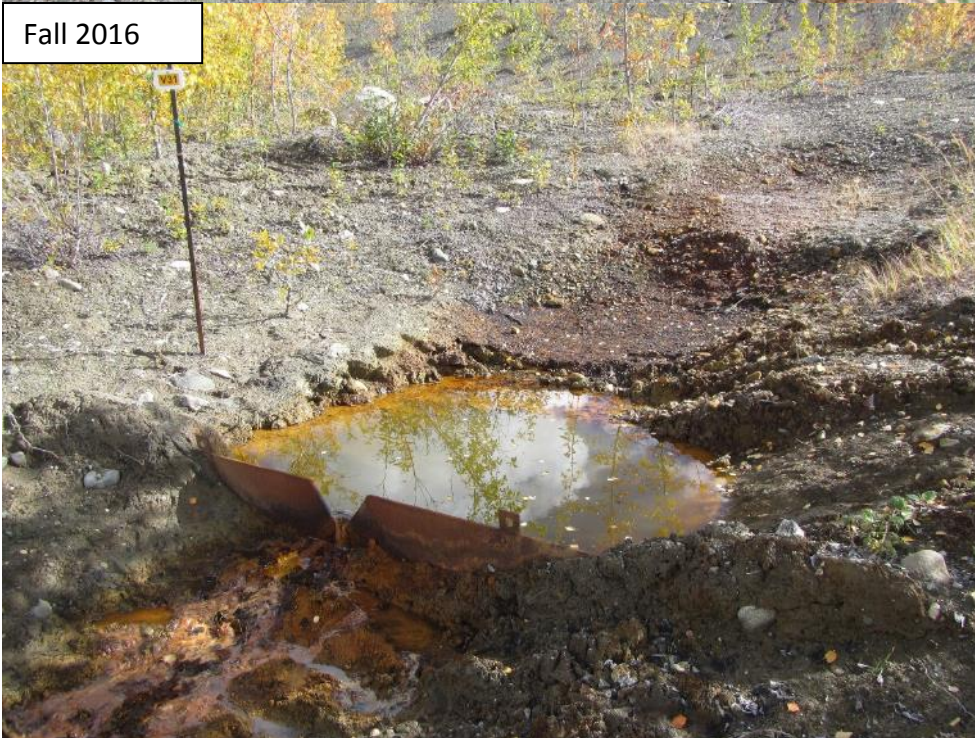
Photograph 38 Drain No. 4 (V31). Satisfactory conditions.
