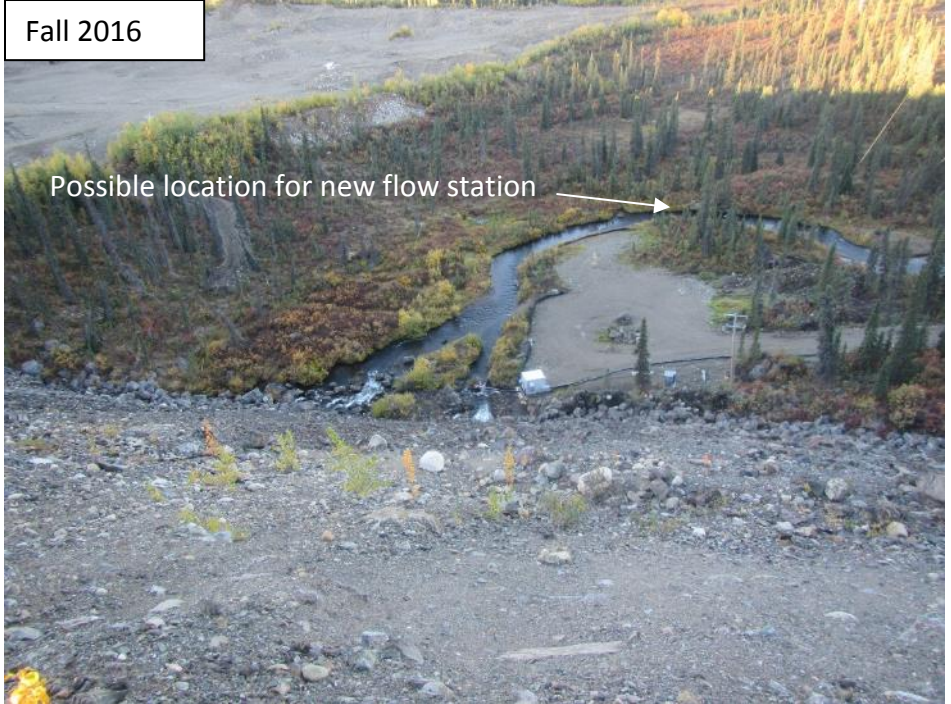
Photograph 20 North Fork Rock Drain outlet, looking downstream. Satisfactory conditions. Possible location of new flow station shown.
