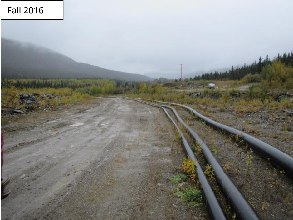
Photograph 32 Siphon pipelines in spillway, looking downstream
