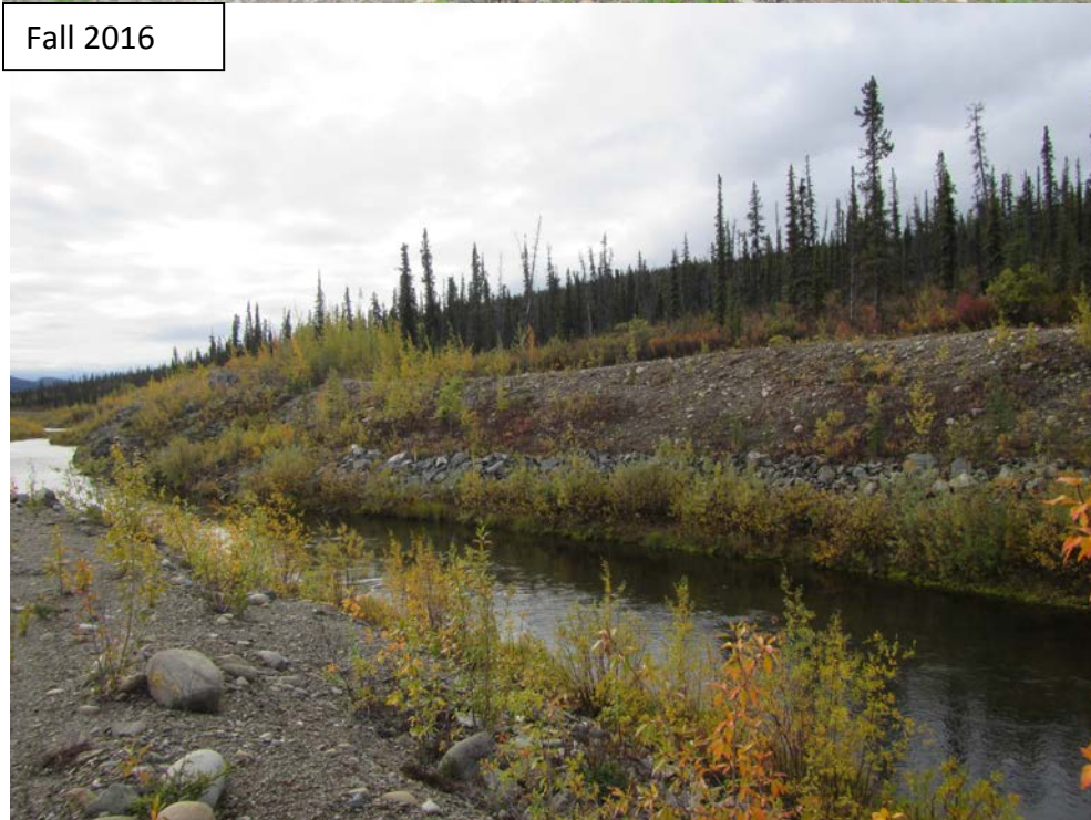
Photograph 15 Rose Creek Diversion Channel Back Slope Observation Location A.
