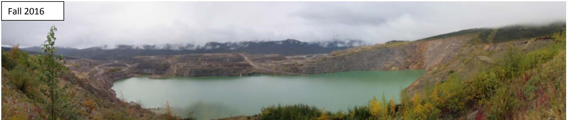
Photograph 2 Faro Pit Northwest Wall and West Wall (from the Faro Creek Diversion Channel). Similar conditions in spring and fall.
