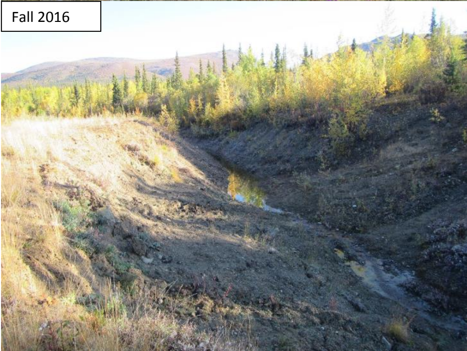
Photograph 45 Slumping of side slopes. Similar conditions in spring and fall.
