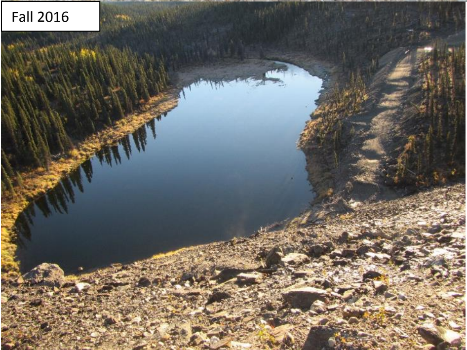
Photograph 19 North Fork Rock Drain upstream pool at access road. Satisfactory condition.
