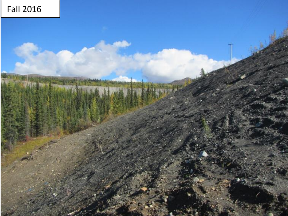
Photograph 57 Rill erosion on downstream berm slopes. To be graded in the fall and revegetated in the spring.
