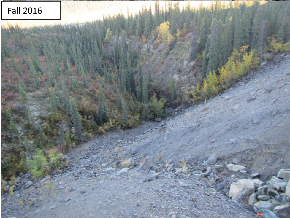
Photograph 22 K8 Rock Drain downstream outlet, looking down. Satisfactory conditions.
