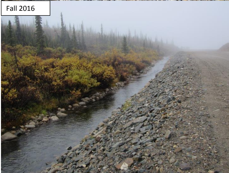
Photograph 4 Upper Faro Creek Diversion. Satisfactory conditions.
