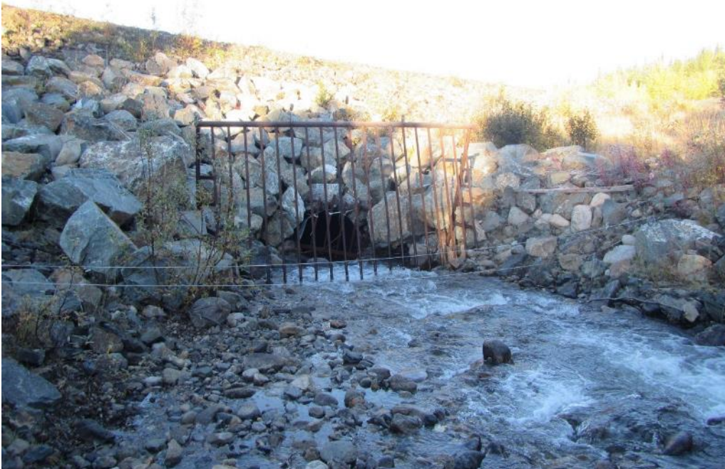
Photograph 47 Vangorda Flume intake culvert upstream trashrack. Satisfactory conditions.
