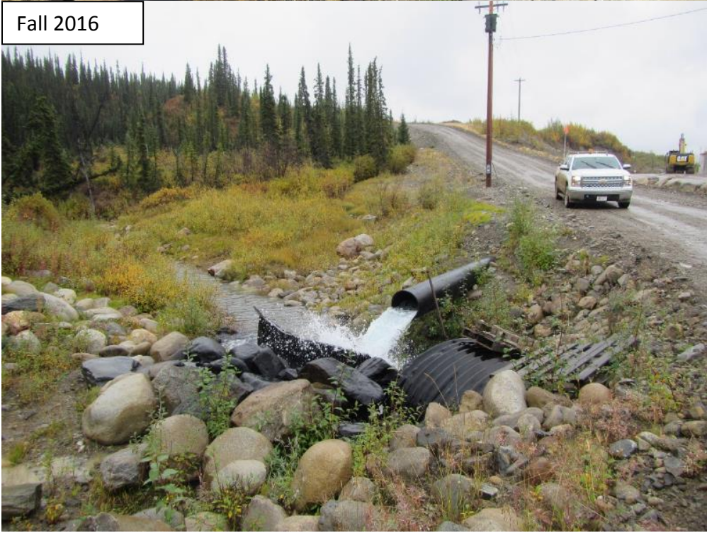
Photograph 11 Culvert between middle reach to lower reach of ditch – water treatment release pipeline. Direct discharge in fall. Approximately 2600 m from the diversion inlet.
