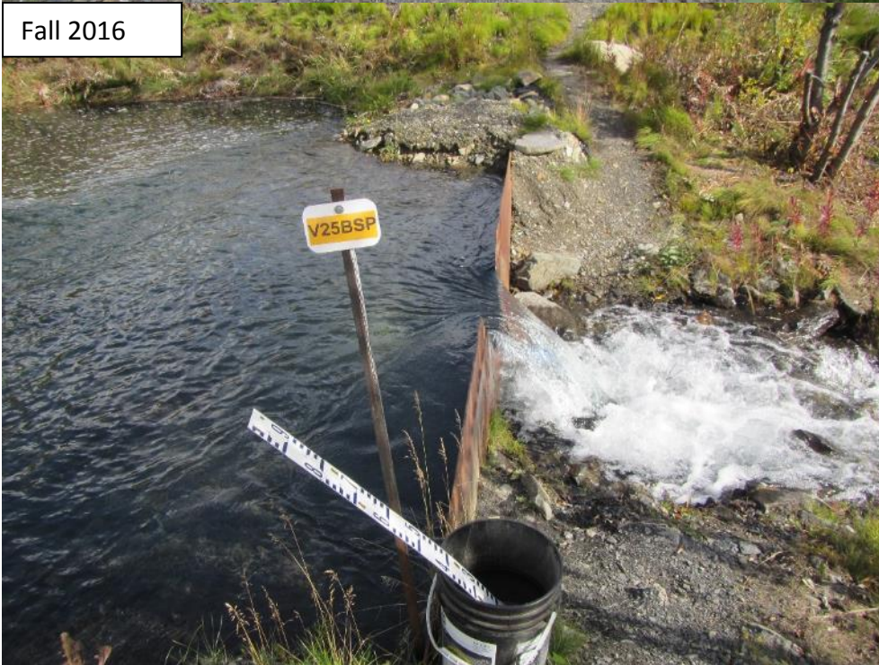
Photograph 60 Outflow of Sediment Pond upstream of Plunge Pool. Satisfactory conditions.
