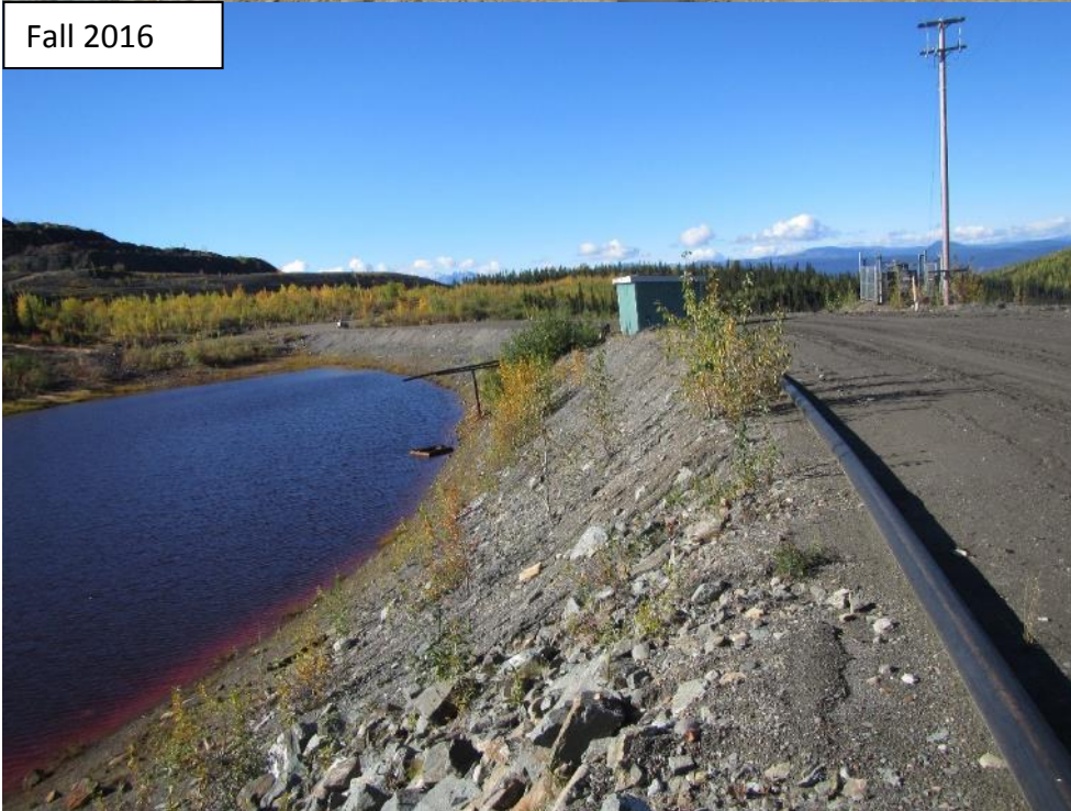
Photograph 53 Little Creek Dam from the access road (looking west). Satisfactory conditions.
