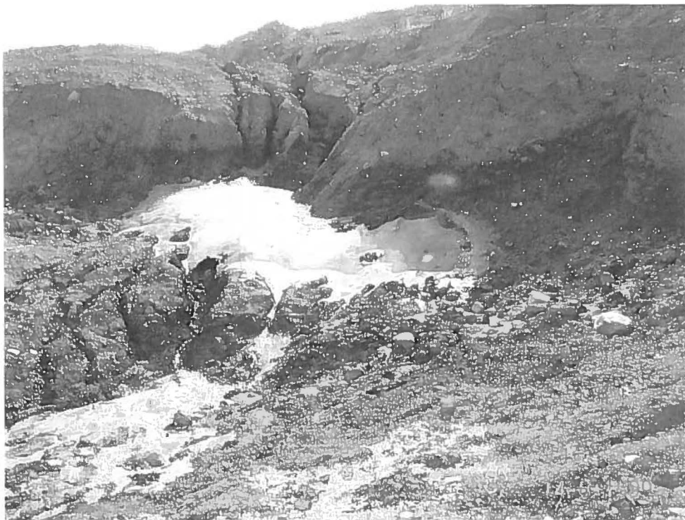
Photo 4: Erosion above Weir 6
