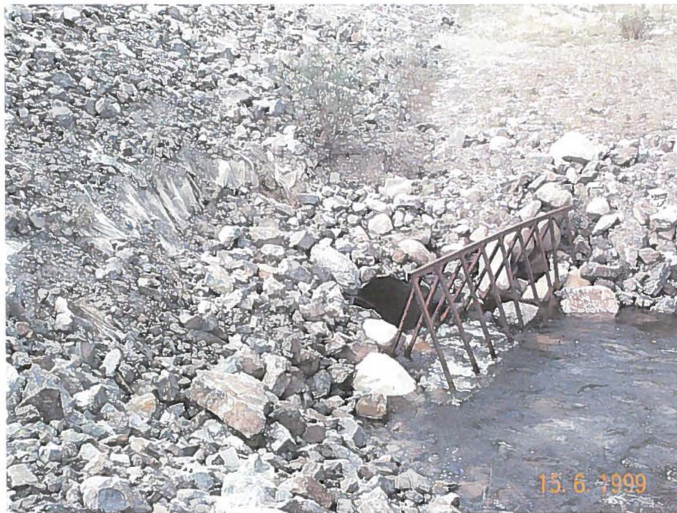
Photo 22: Headworks of the Vangorda Creek Diversion
