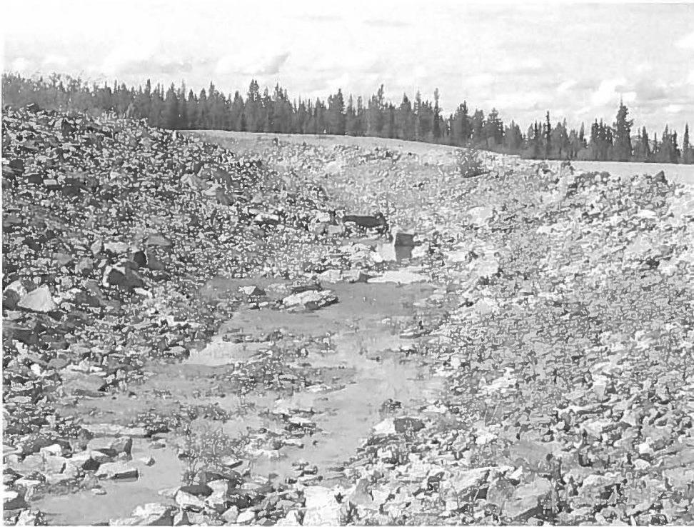
Photo 7: Seepage Collection Ditch on Northside of Waste Dump
