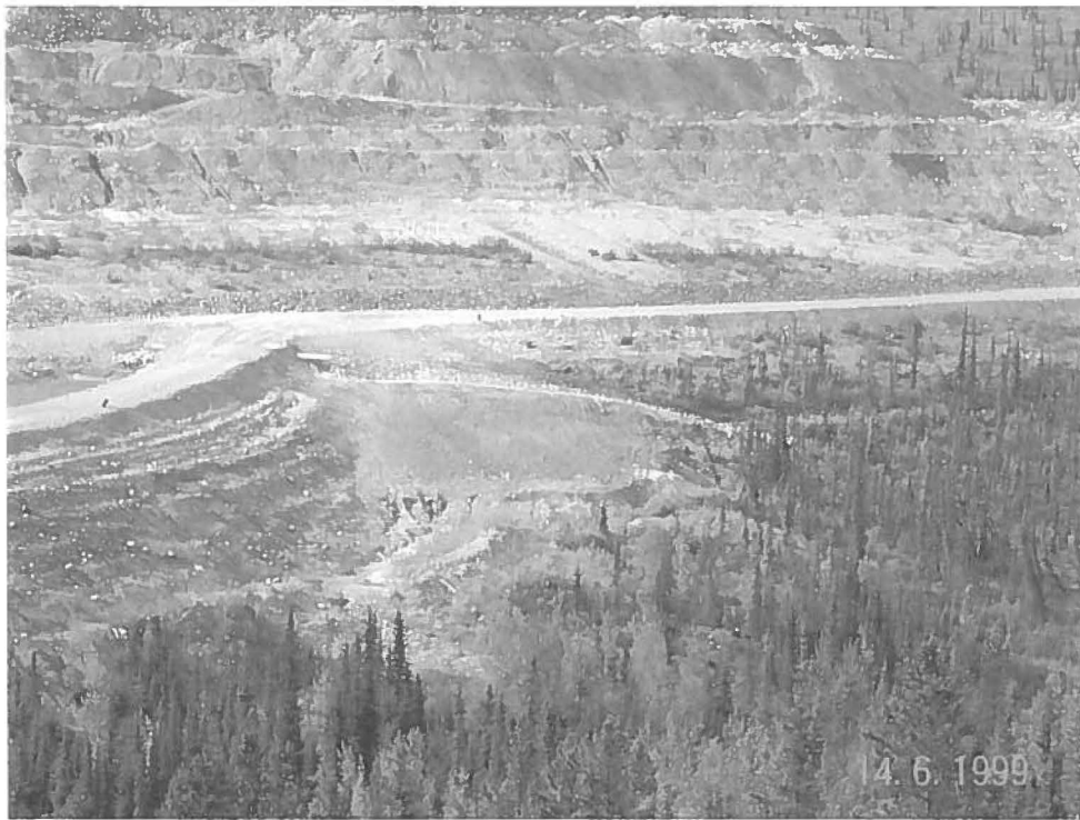
Photo 8: CSP Culvert Spillway in Little Creek Dam
