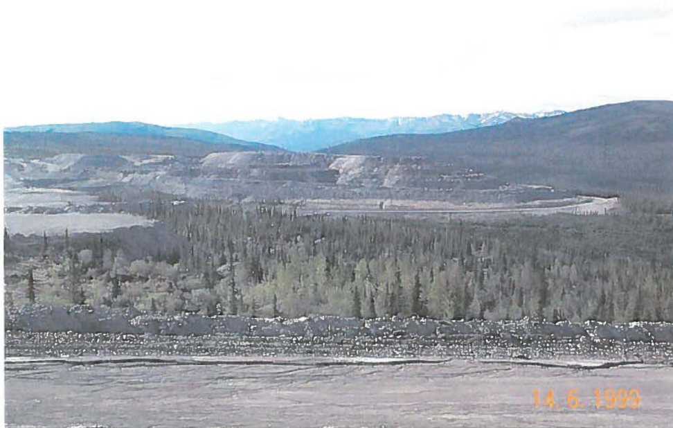
Photo 1: A view overlooking the Vangorda Waste Dump and the Seepage Collection Ditch
