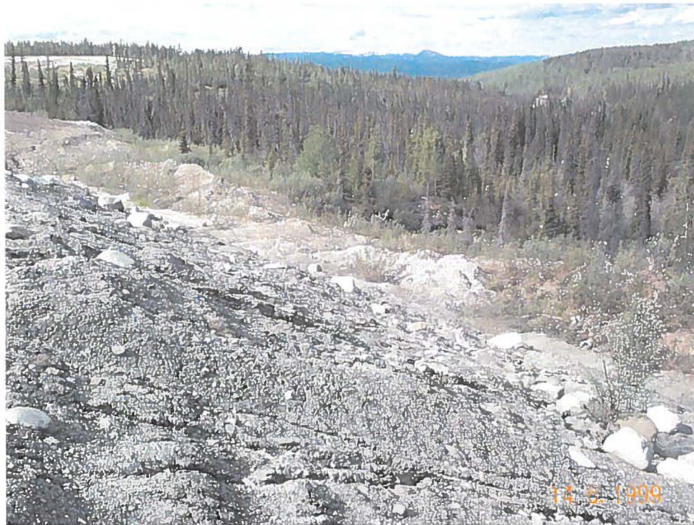
Photo 14: Downstream Face of Little Creek Dam
