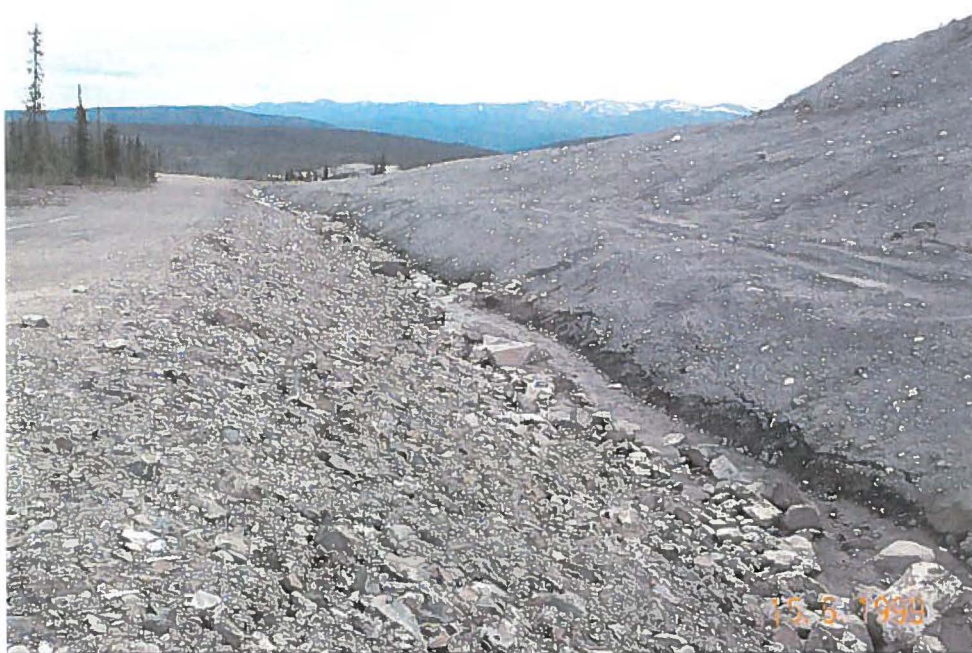
Photo 30: Grum Interceptor Ditch
