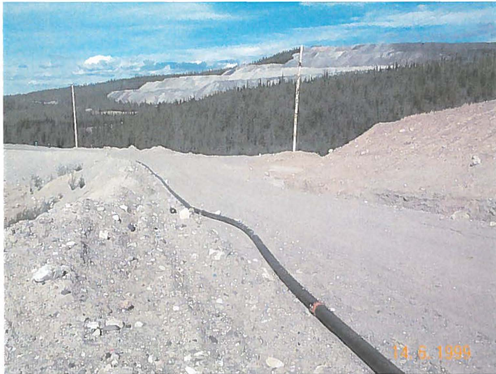
Photo 11: Approach Road to Little Creek Dam after Pipeline Return to Treatment Plant on side of Road
