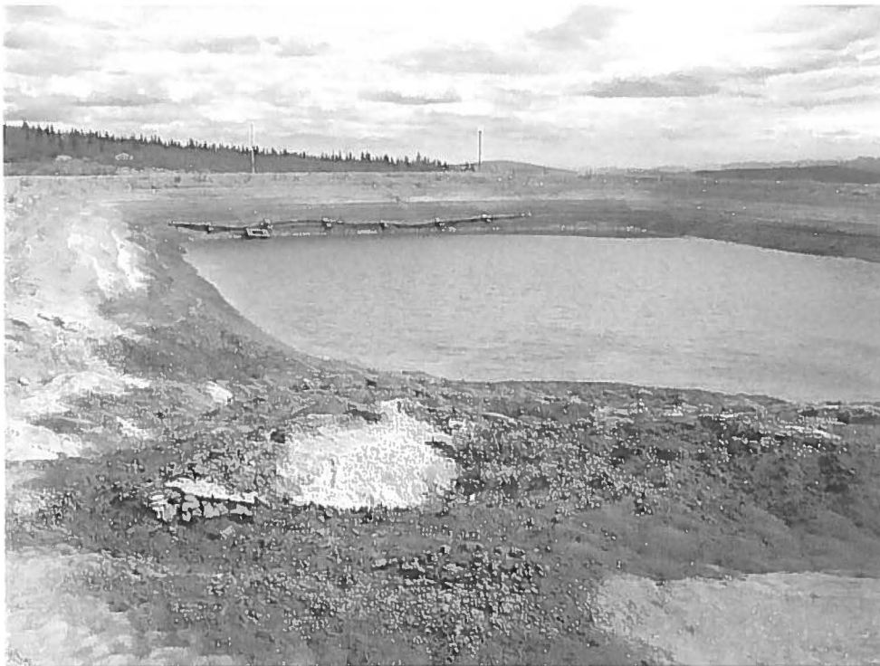
Photo 26: Sludge Pond at the Treatment Plant
