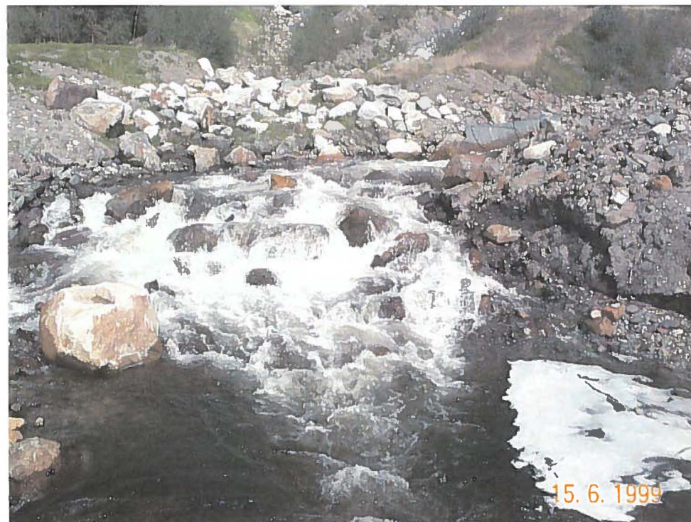
Photo 24: Outlet of the Vangvorda Creek Diversion
