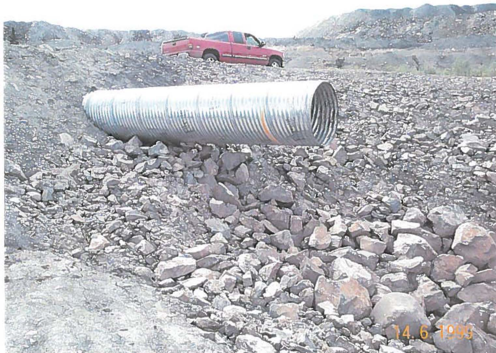
Photo 17: View South of Outlet end of Spillway in June 1999
