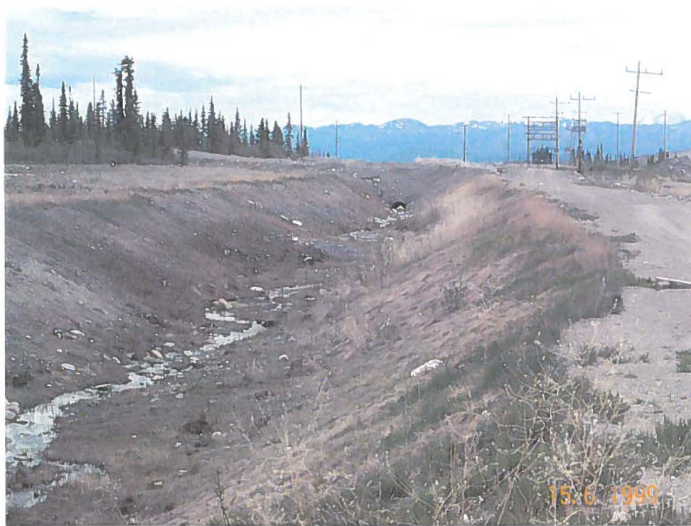
Photo 28: Grum Interceptor Ditch above Treatment Plant
