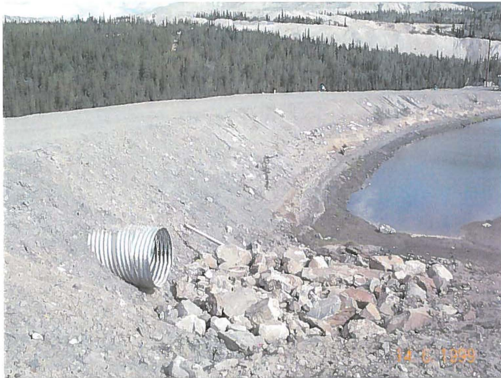
Photo 15: Inlet of Culvert Spillway at South end of Little Creek Dam
