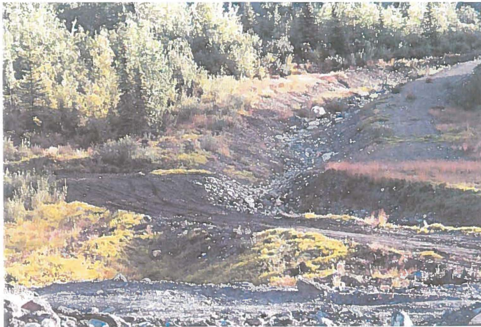
Photo 30: View of removed culvert at the end of the GID
