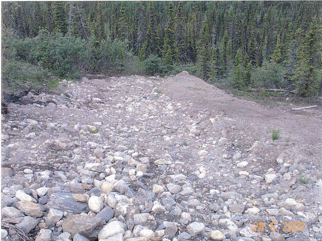
Photo 17 Exit Channel below Plunge pool at Little Creek Dam Spillway
