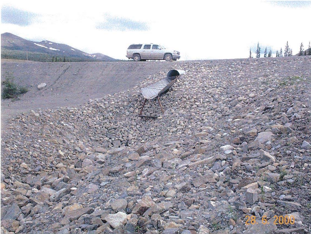
Photo 15 Emergency Spillway Culvert and chute at Little Creek Dam
