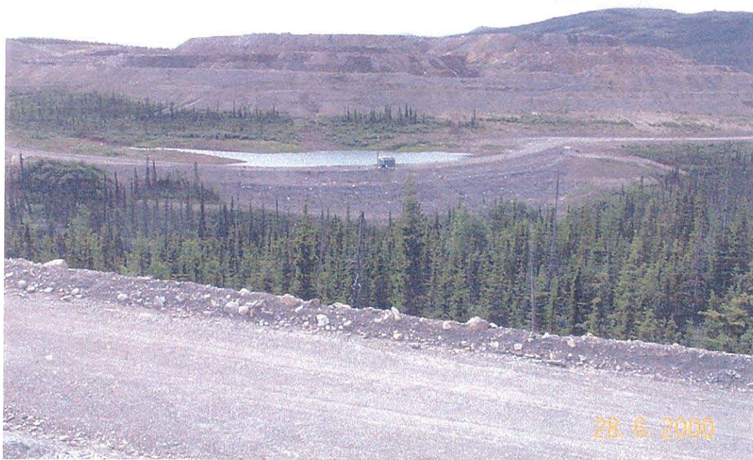
Photo 1 A view overlooking the Vangorda Waste Dump with Little Creek Pond in the foreground
