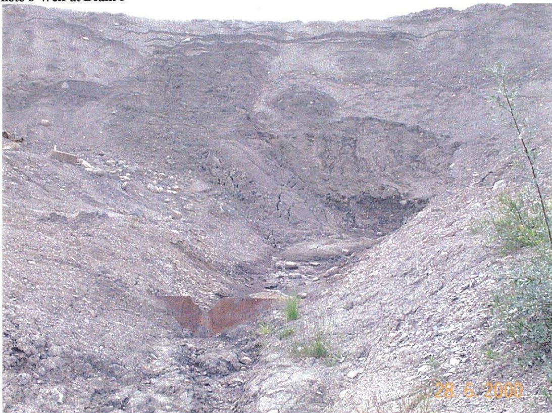
Photo 4 Weir at Drain 6
