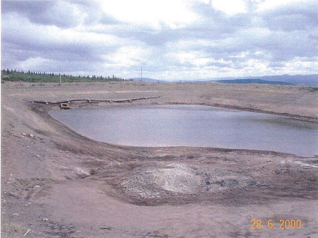
Photo 23 Sludge Pond at the Treatment Plant
