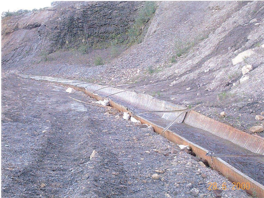
Photo 19 Lower Reaches of Vangorda Creek Diversion
