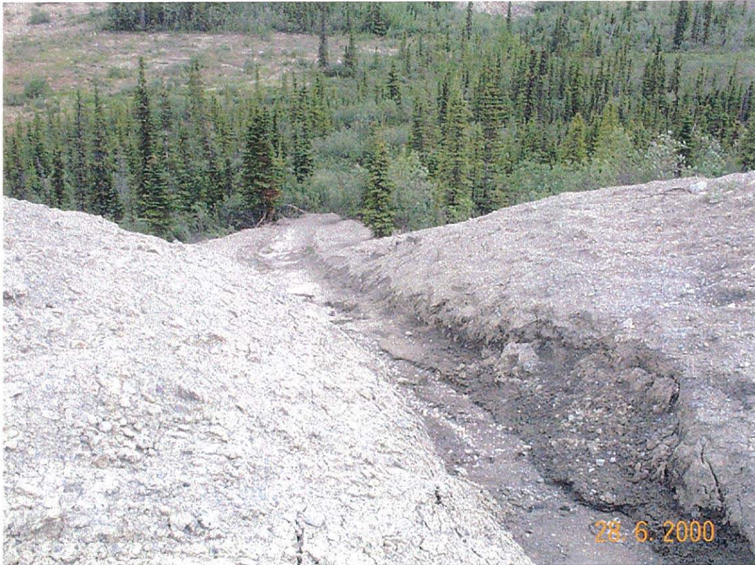
Photo 7 Exit reach of the diversion ditch
