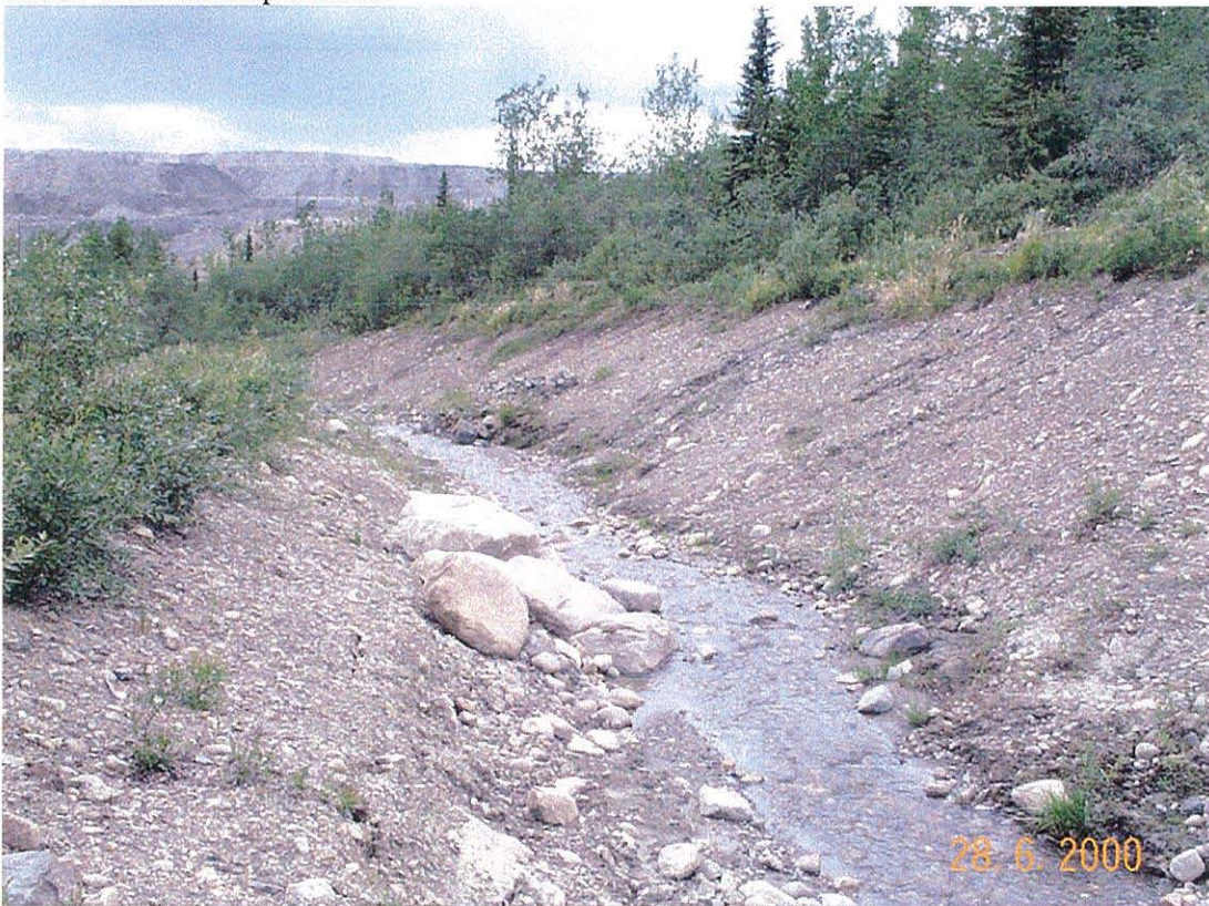
Photo 28 Subsidence in the lower reaches of the GID
