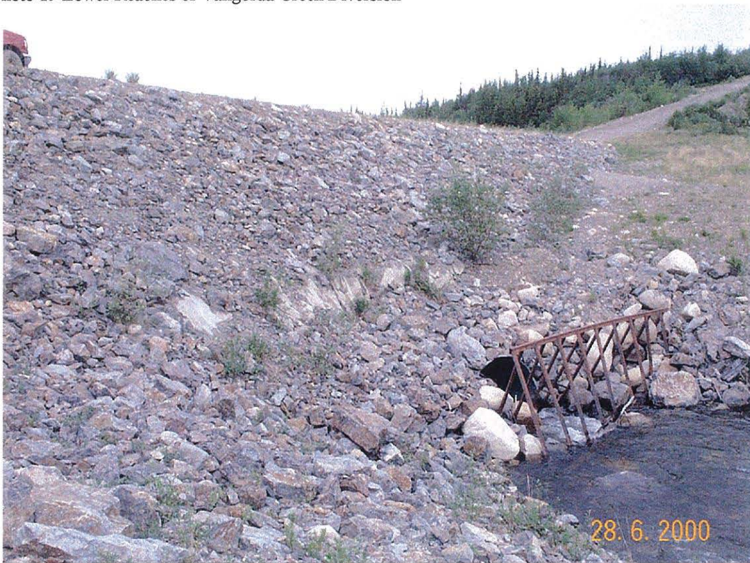
Photo 20 Headworks of the Vangorda Creek Diversion
