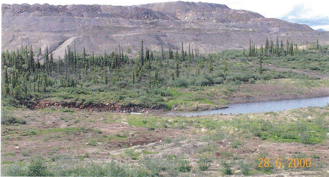
Photo 5 View of the Starter Dyke Diversion Ditch
