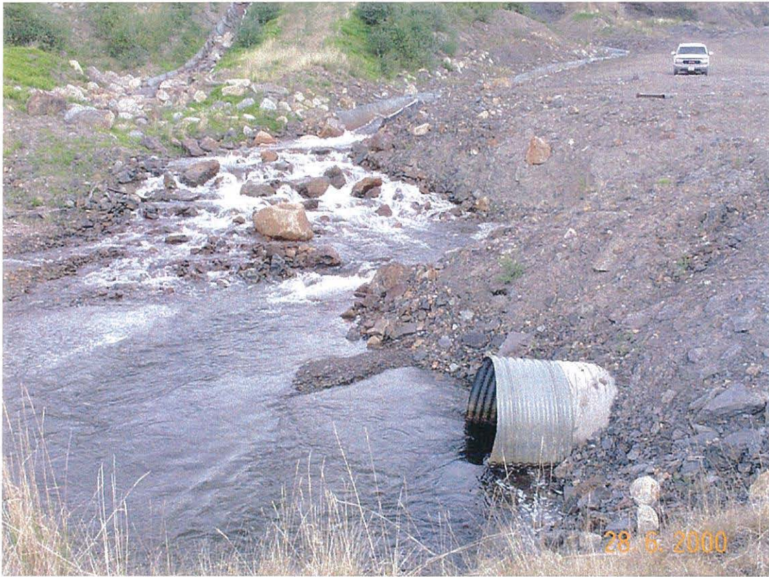
Photo 21 Plunge pool at base of Vangorda Creek Diversion
