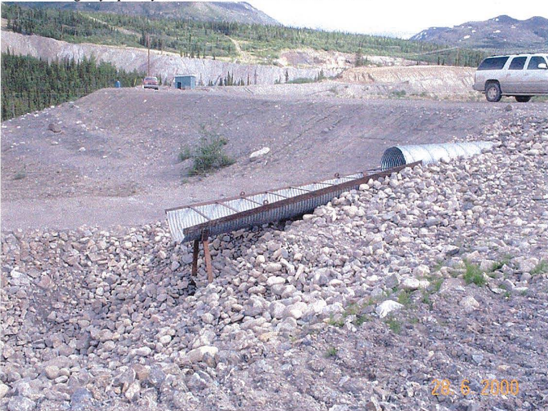
Photo 16 Emergency Spillway at Little Creek dam
