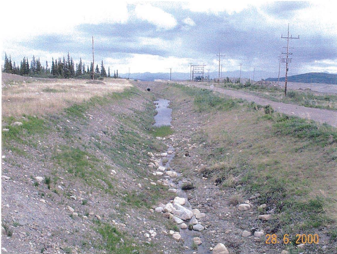
Photo 27 Grum Interceptor Ditch
