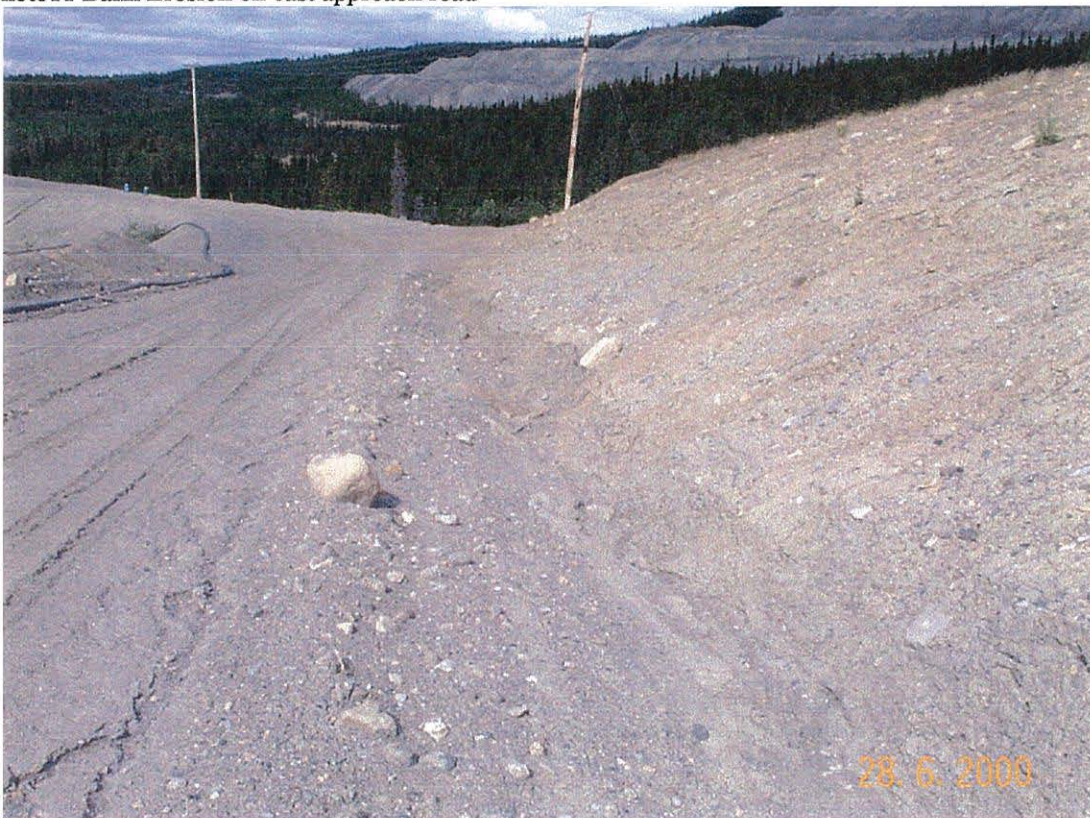
Photo 12 Drainage ditch on the Approach road to Little Creek Dam
