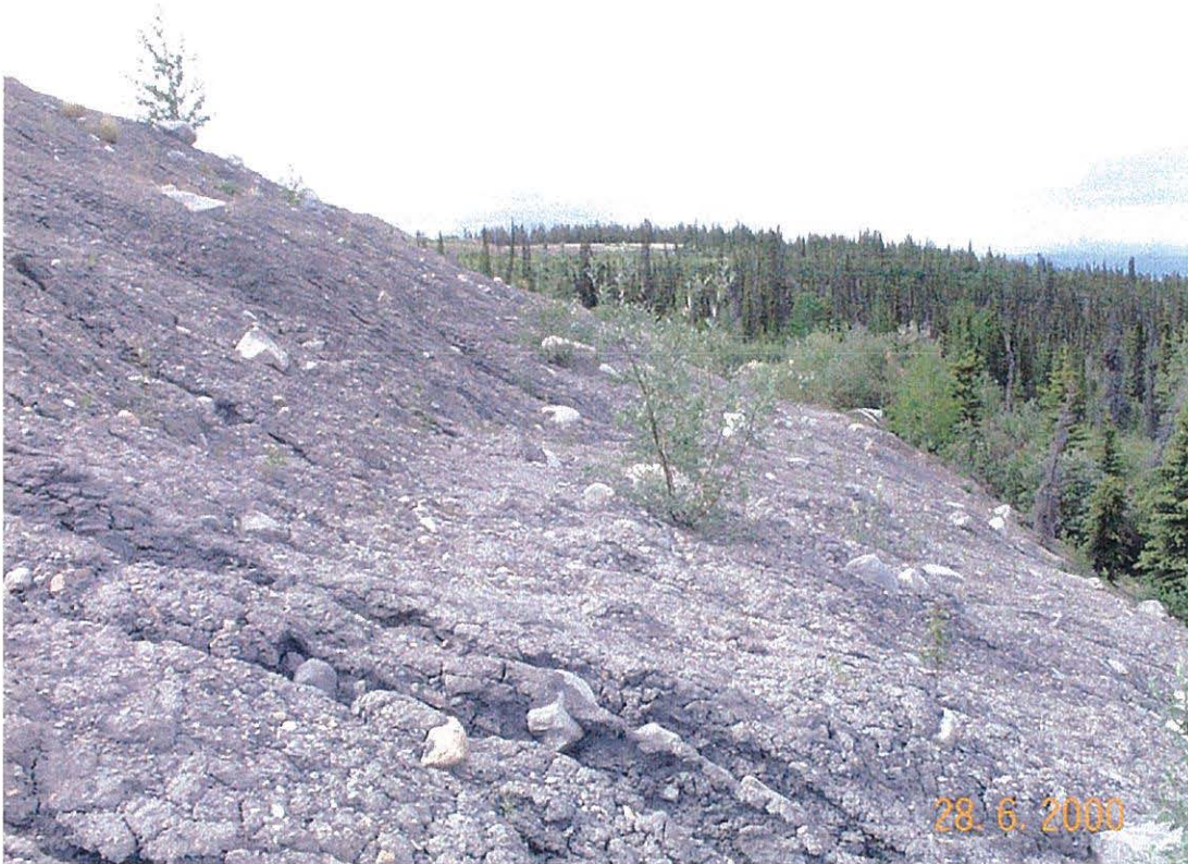
Photo 14 Downstream face of Little Creek Dam
