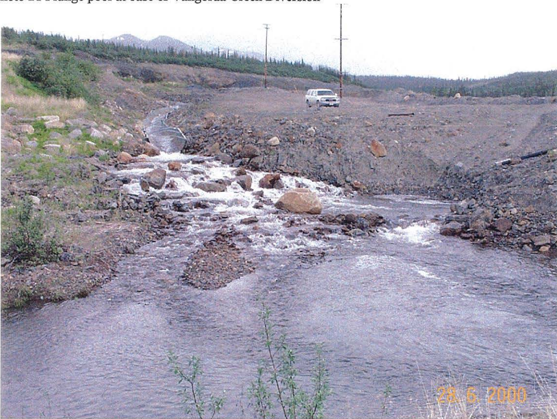
Photo 22 Plunge pool at base of Vangorda Creek Diversion
