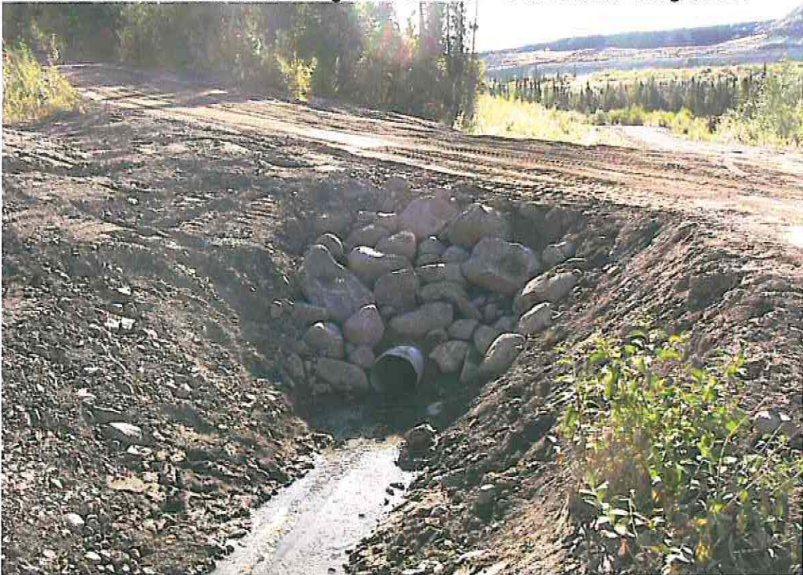
Photo 26: New culvert (2007) below V-notch Weir on Grum Creek and new diversion
