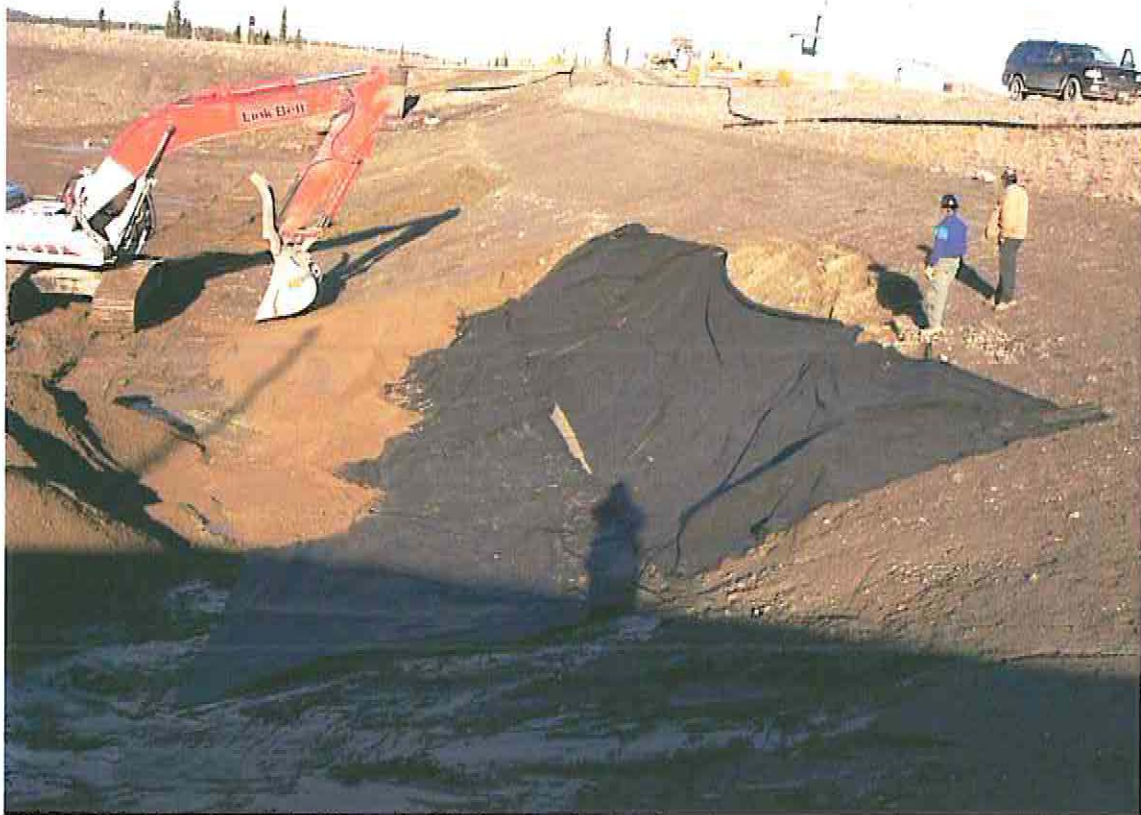
Photo 29: Repair to subsidence in Sludge Pond at Vangorda
