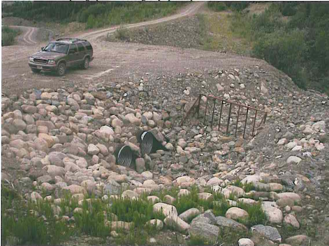
Photo 14: Emergency Spillway at the headworks of Vangorda Creek Diversion
