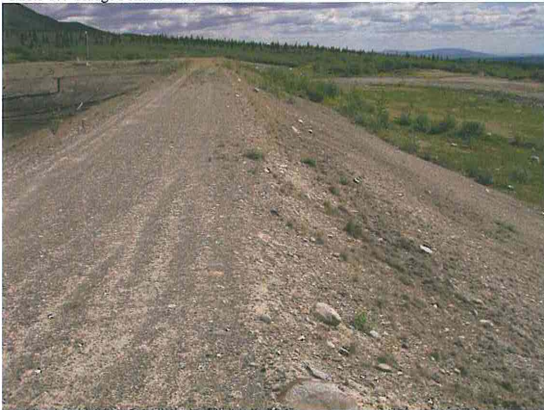
Photo 18: Till Embankment around the Sludge Pond
