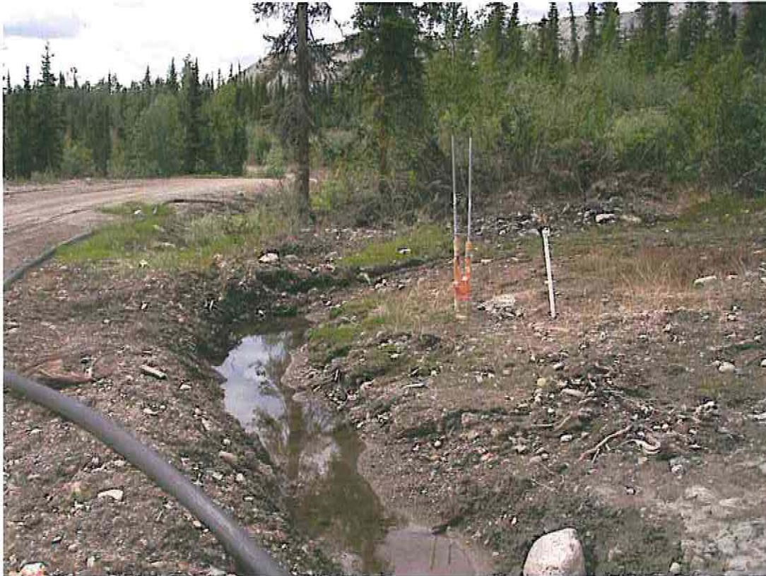
Photo 3: Seepage collection ditch below groundwater wells.
