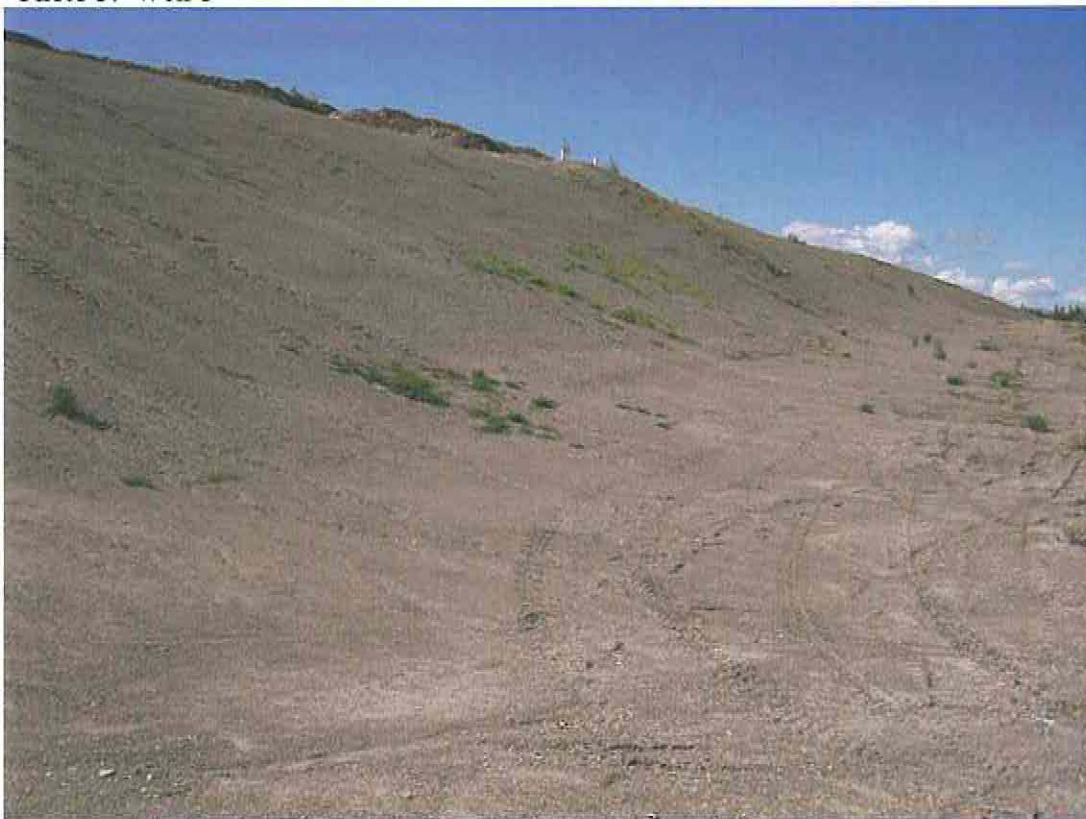
Photo 4: Till Slope above Weirs #5 and #6
