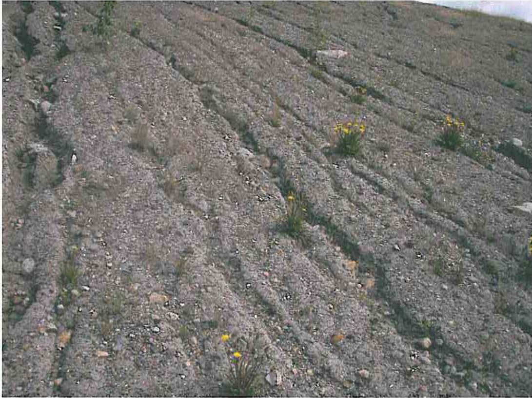
Photo 9: Erosion Gullies in the till cover on Vangorda Dump
