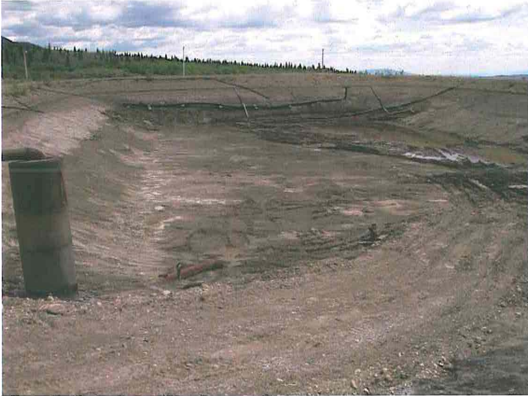
Photo 17: Sludge Pond at Water Treatment Plant
