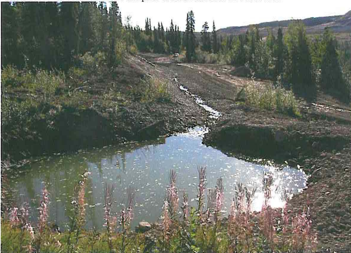
Photo 24: V-15 Sedimentation Pond after construction
