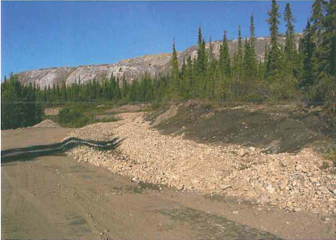
Photo 25: Runoff diversion ditch along haul road from V-15 constructed in August 2007
