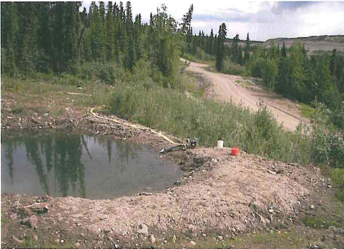
Photo 23: V-15 Sedimentation Pond prior to construction of diversion ditch
