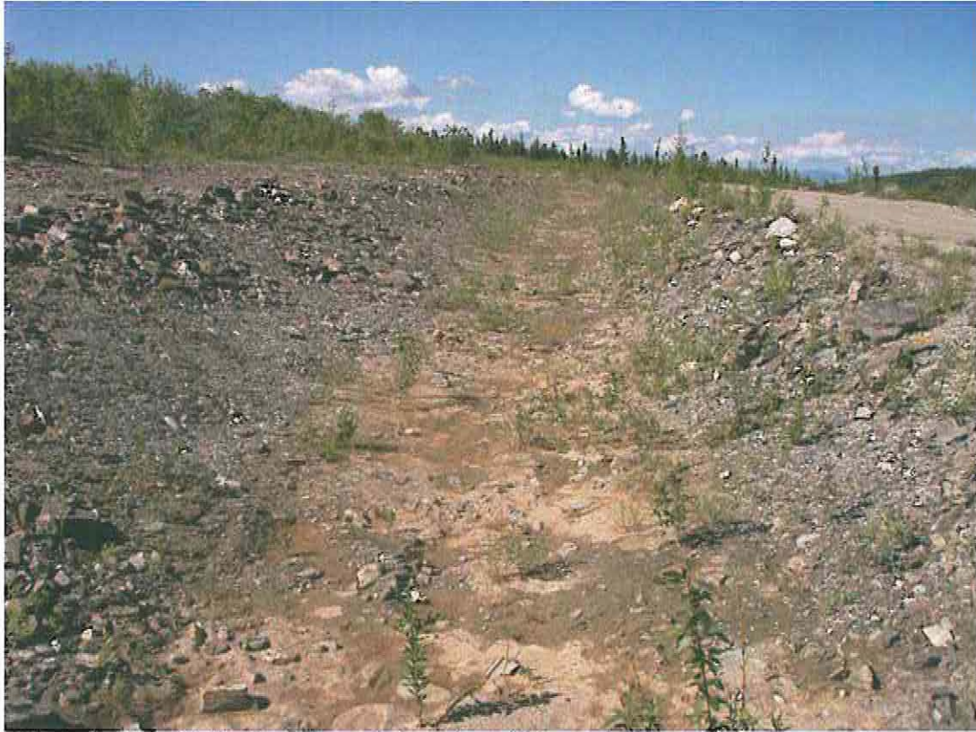
Photo 5: Seep Collection Channel along toe of Vangorda Waste Dump
