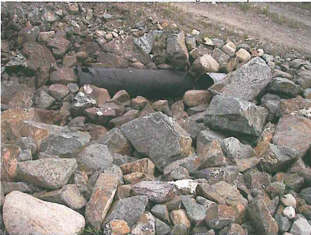
Photo 22: Culvert entrance just above Sheep Pad Pond
