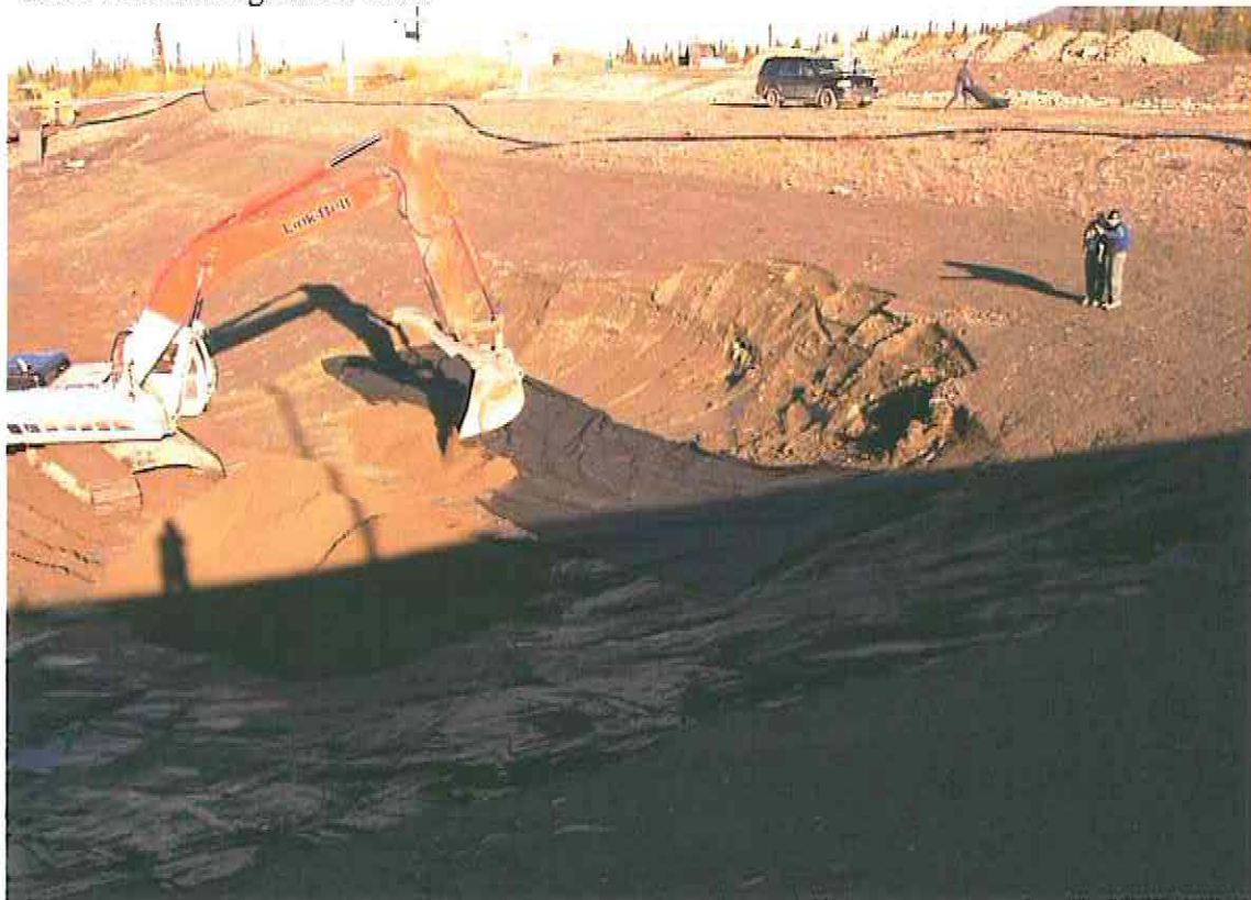
Photo 28: Repair to subsidence in Sludge Pond at Vangorda
