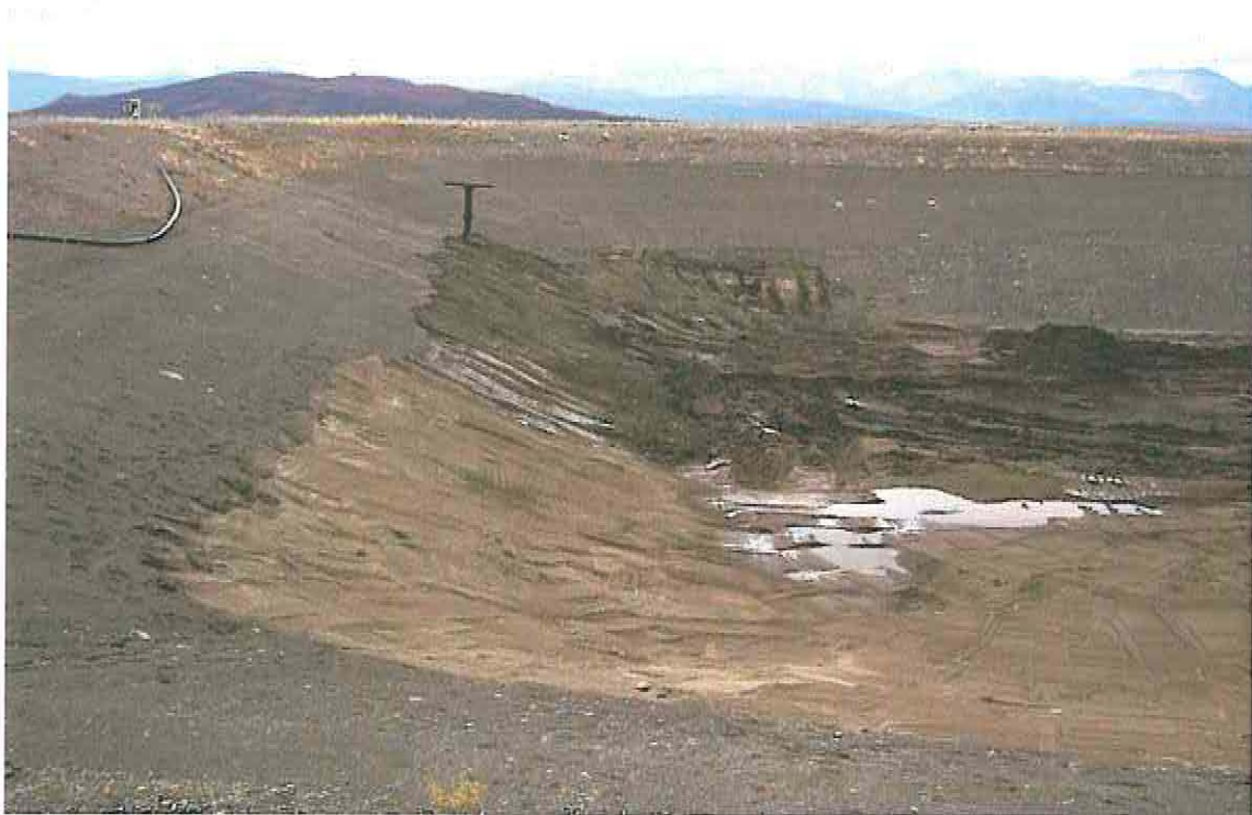
Photo 30: Completed remediation to subsidence in Sludge Pond at Vangorda
