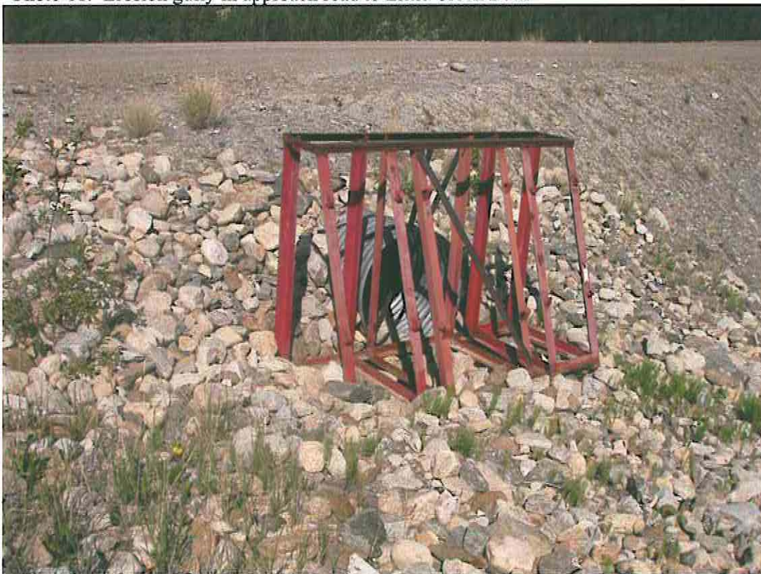
Photo 12: Emergency culvert (inlet) at Little Creek Pond
