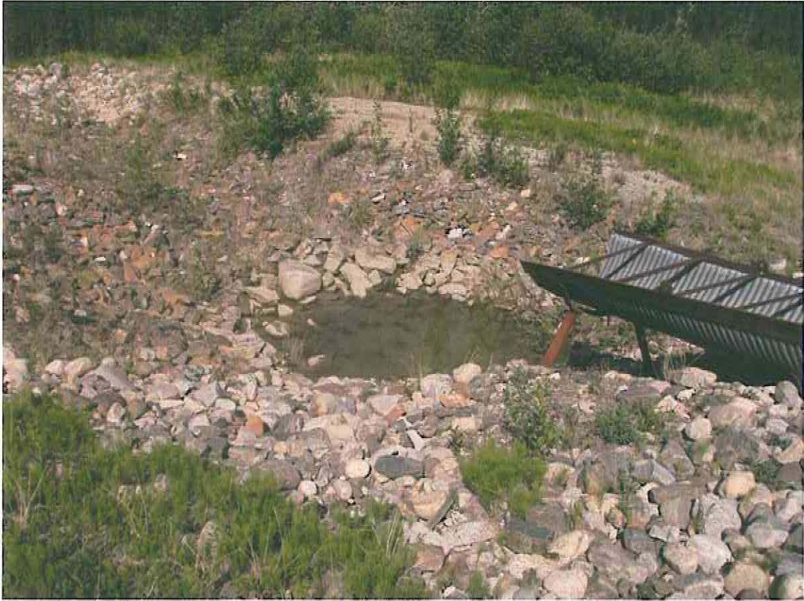
Photo 13: Outlet to plunge pool of emergency spillway at Little Creek Dam
