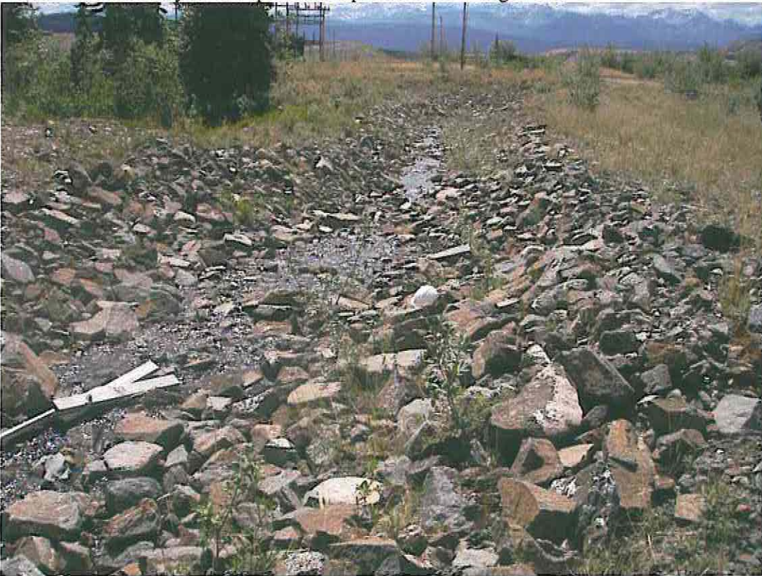
Photo 20: Grum Interceptor Ditch
