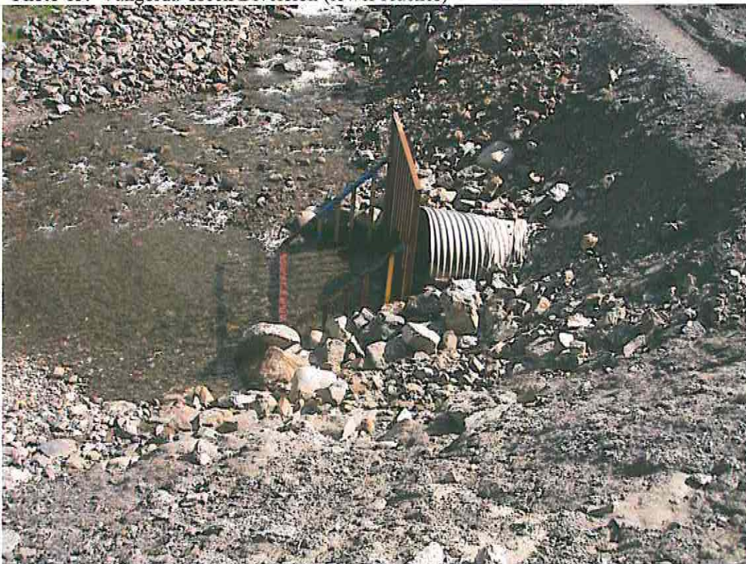
Photo 16: Inlet to the 2m dia CMP at the Vangorda diversion plunge pool
