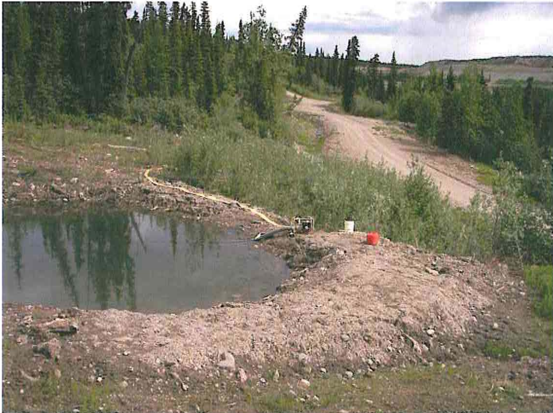
Photo 1: V-15 Sedimentation Pond looking east towards location of V-notch weir on Grum Creek.
