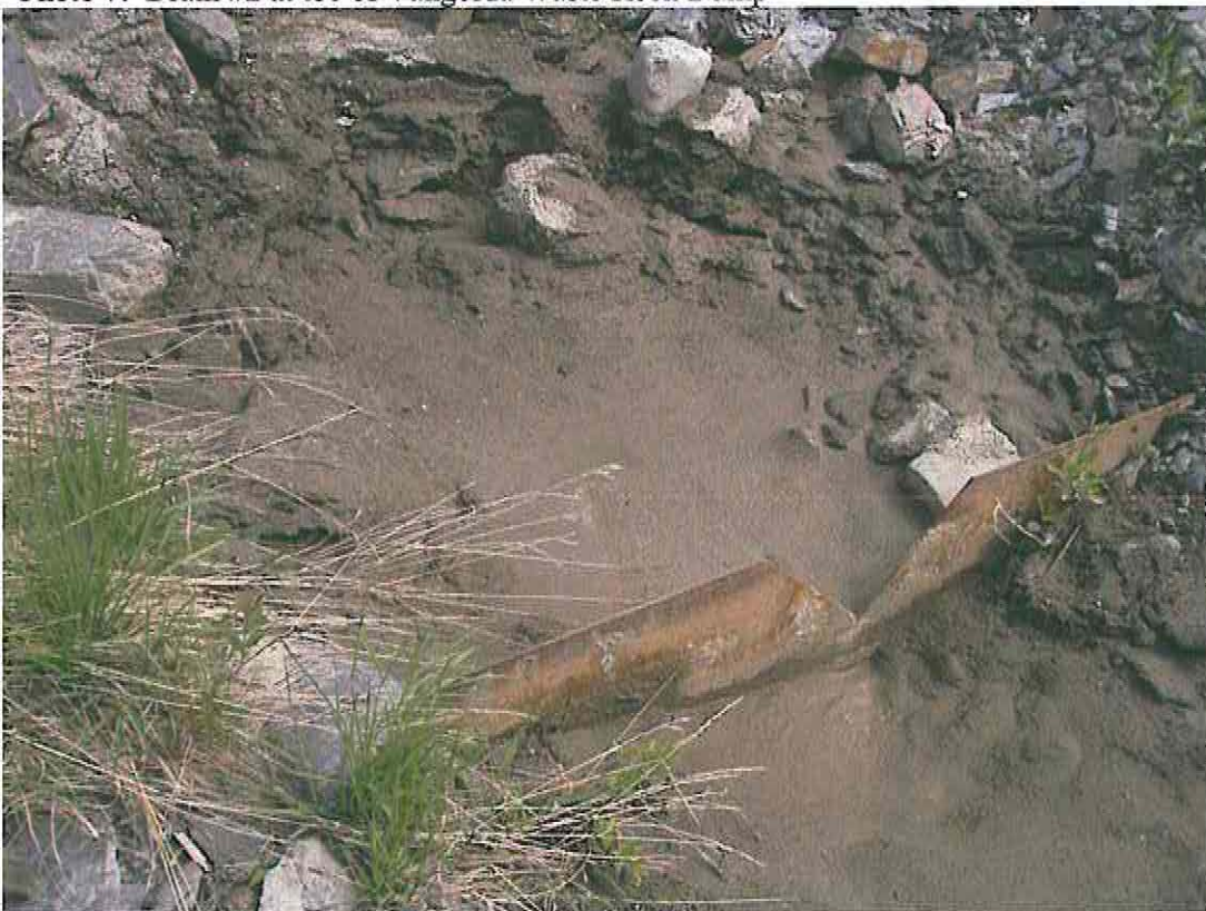
Photo 8: Close-up of Drain #2
