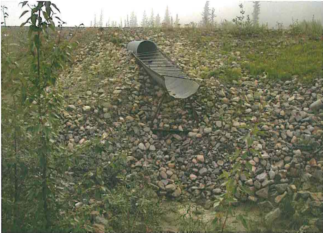
Photo 13: Outlet to plunge pool of emergency spillway at Little Creek Pond
