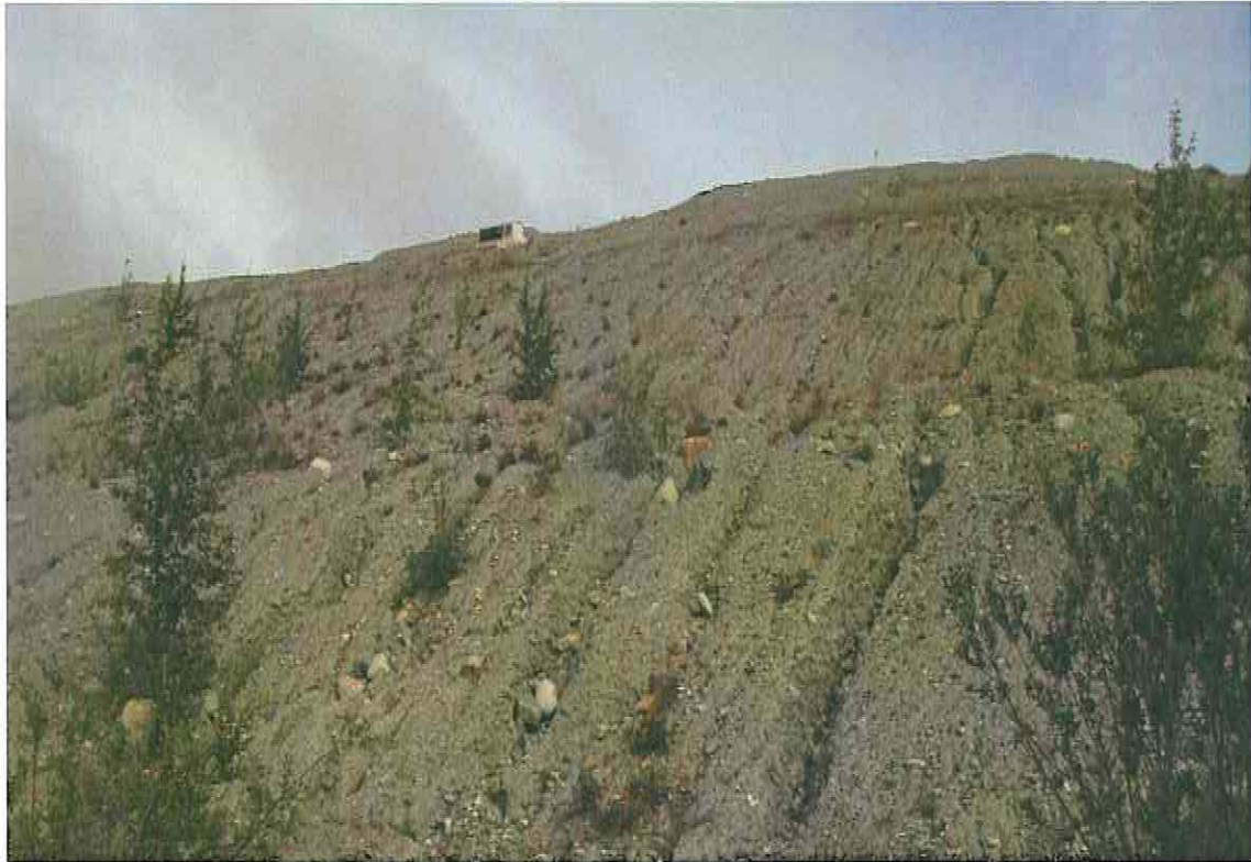
Photo 9: Erosion Gullies in the till cover on Vangorda Dump
