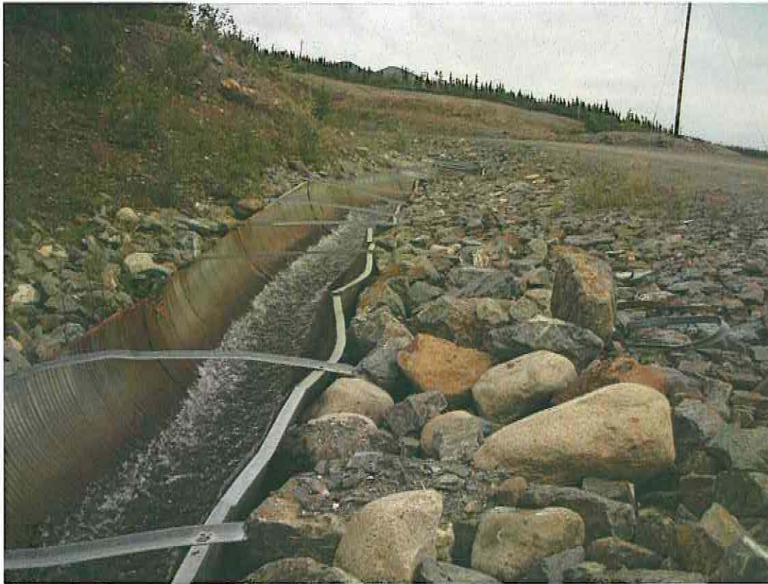
Photo 15: Vangorda Creek Diversion (lower reaches)
