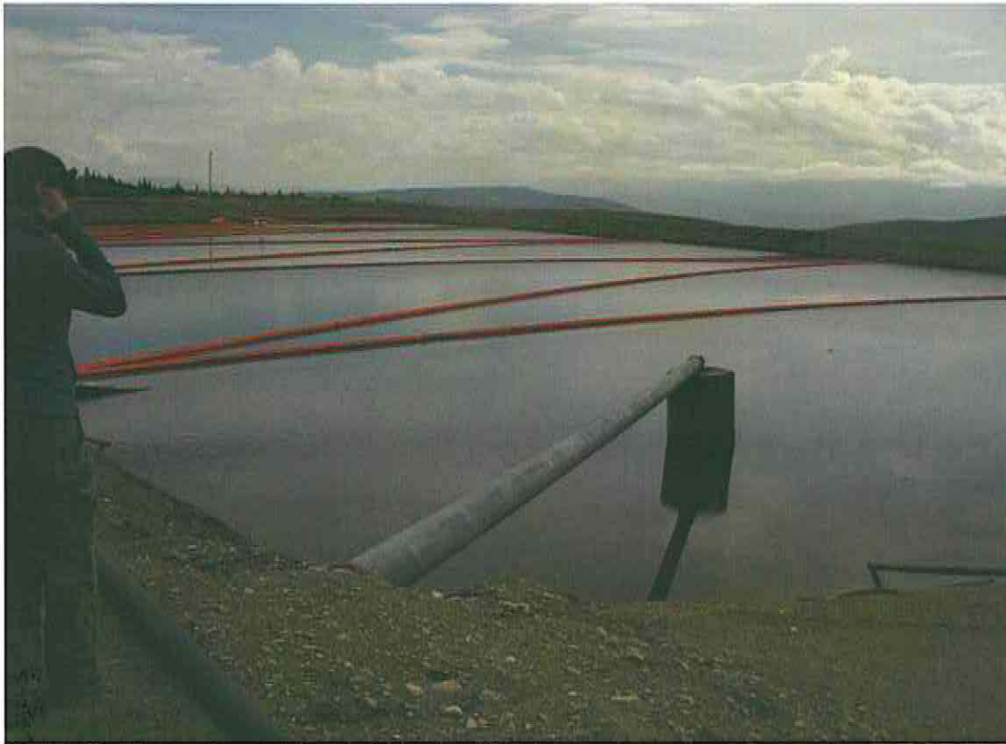
Photo 17: Sludge Pond at Water Treatment Plant
