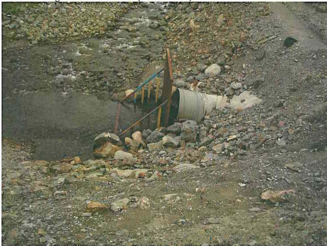
Photo 16: Inlet to the 2m dia CMP at the Vangorda Creek diversion plunge pool
