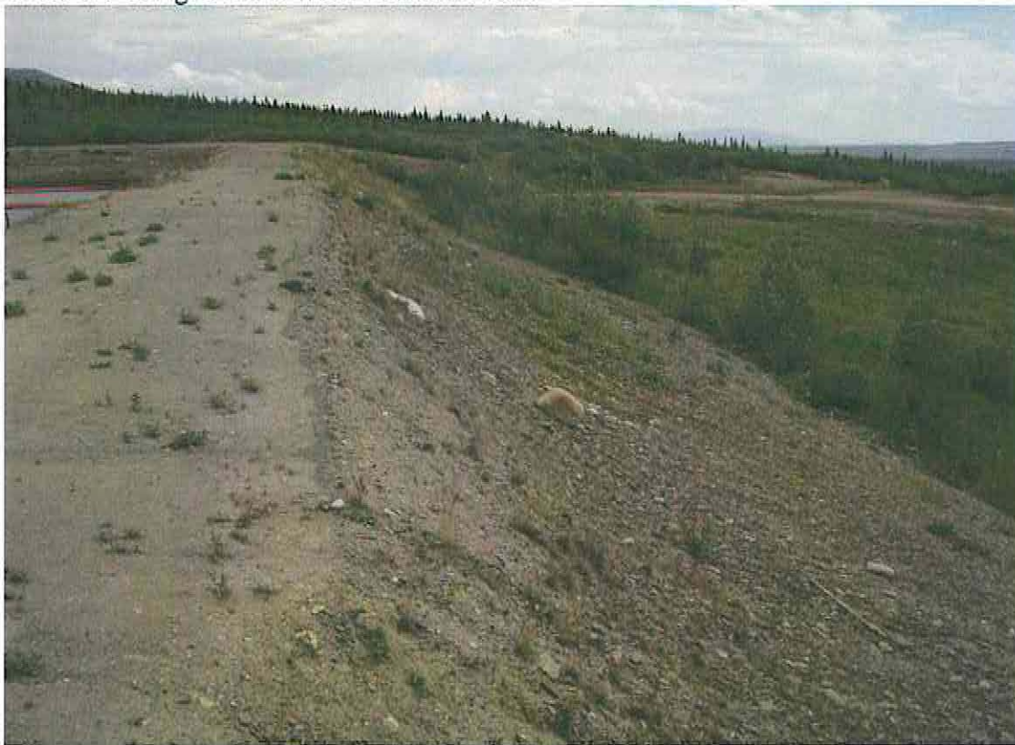
Photo 18: Till Embankment around the Sludge Pond
