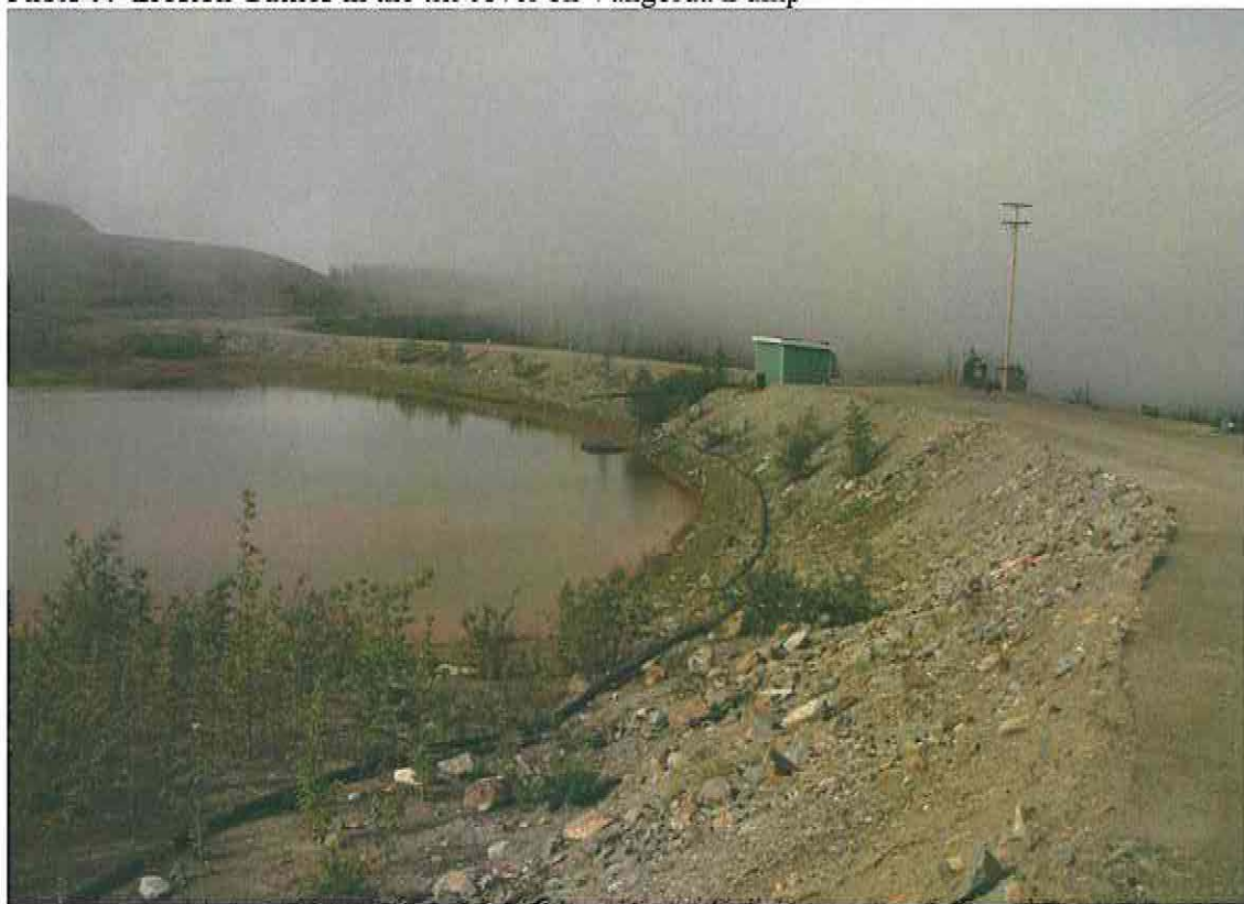
Photo 10: Little Creek Pond Dam
