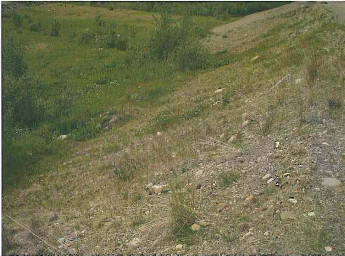
Photo 19: Downstream slope of the dyke around the Sludge Pond
