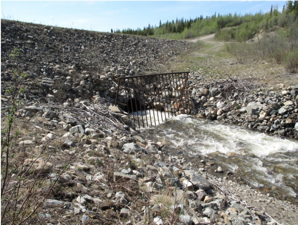
Photo 16: Trash rack at inlet to Vangorda Creek Diversion
