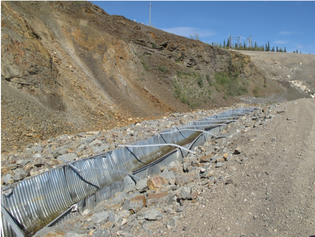
Photo 20: Flume in the Vangorda Creek Diversion
