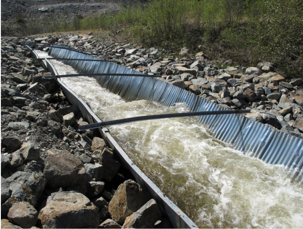
Photo 19: Half round culvert flume in Vangorda Creek Diversion
