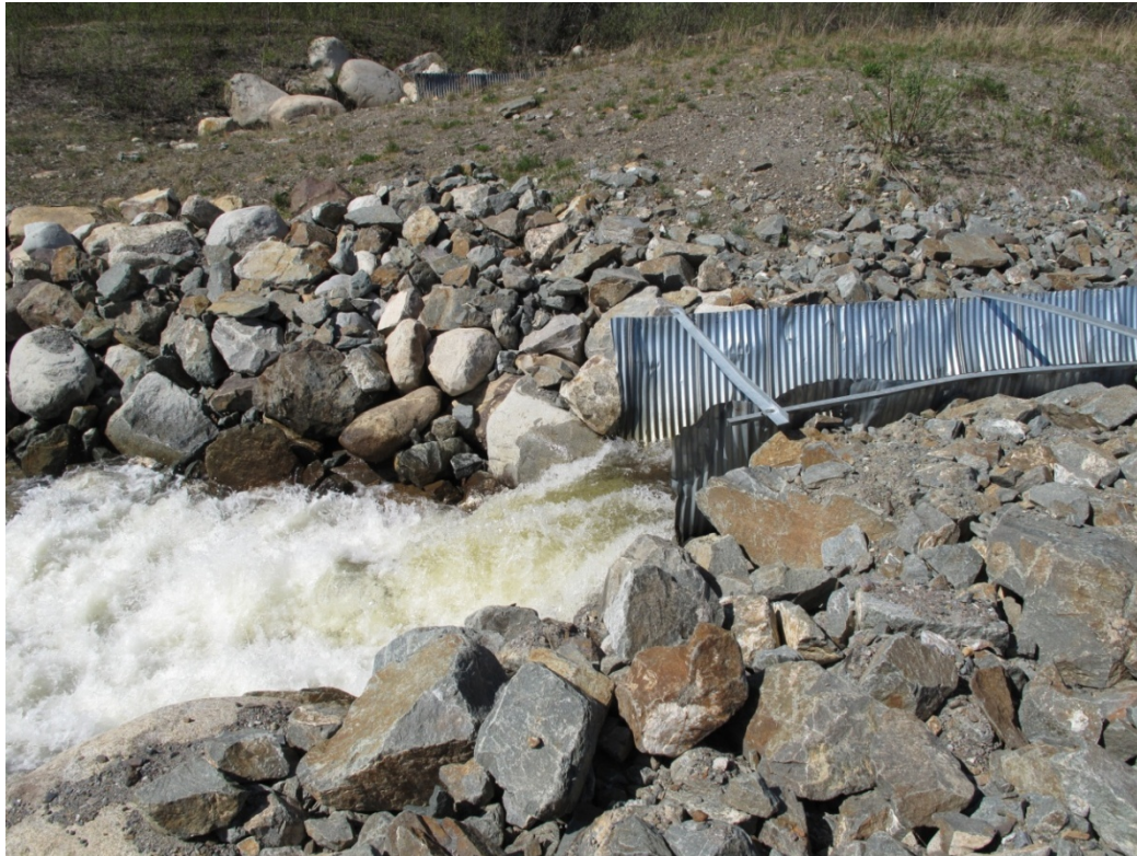
Photo 18: Outlets of the Vangorda Creek Diversion into Plunge Pool
