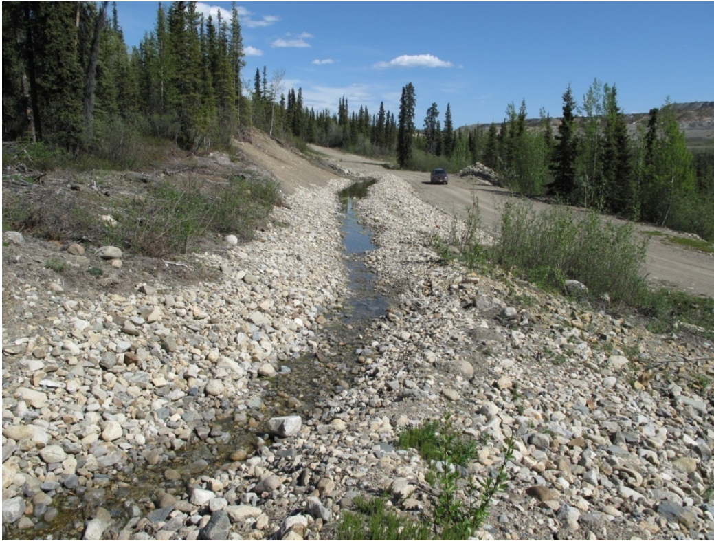
Photo 27: Bentamat lined Diversion ditch from V-15 to main stem of Grum Creek
