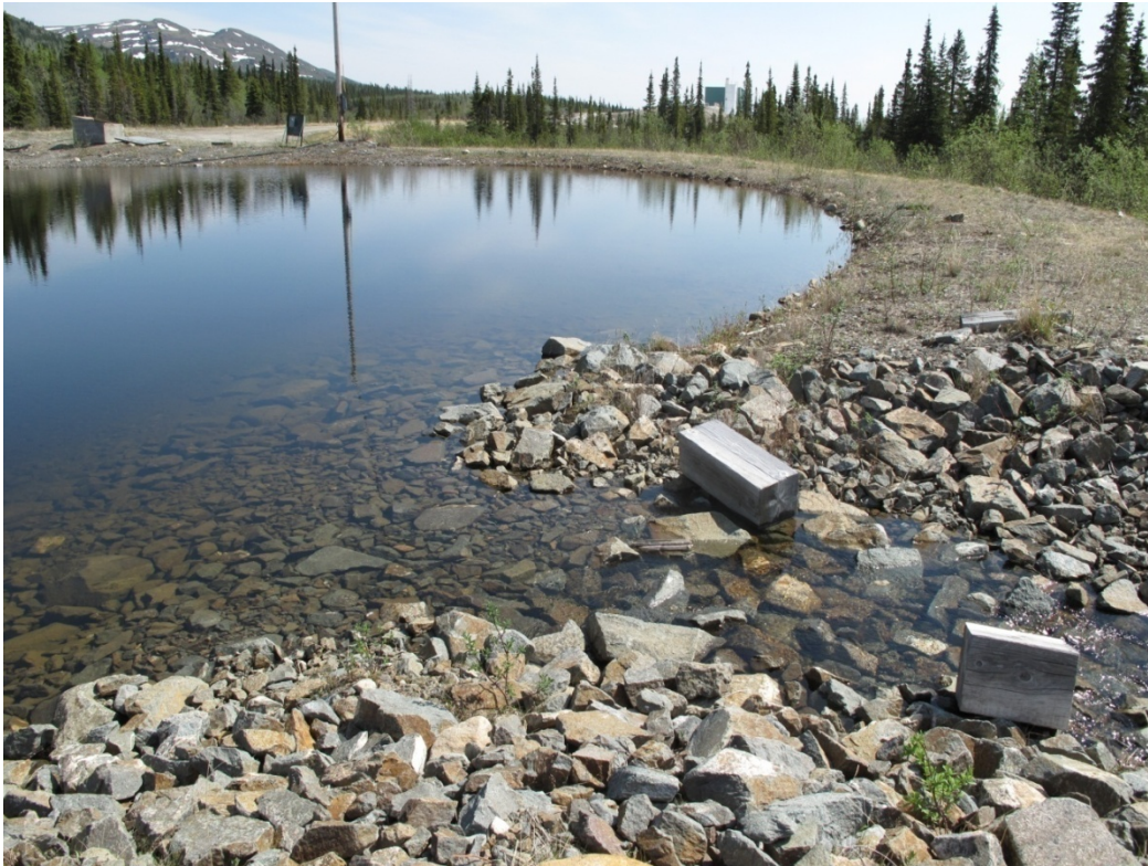
Photo 30: Grum Settling Pond (Groucho Pond) – Spillway Entrance
