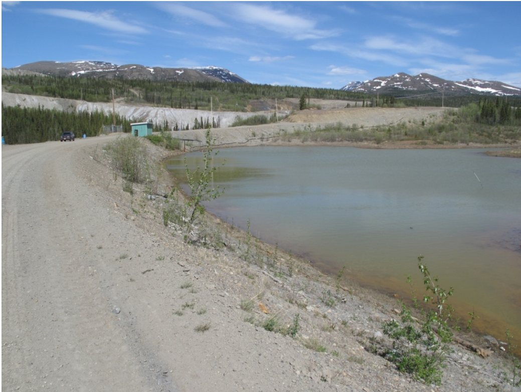
Photo 12: Upstream slope of Little Creek Dam
