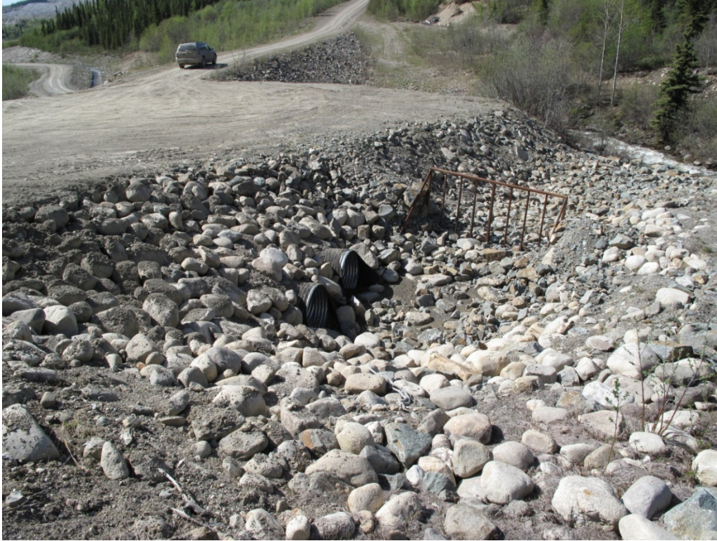
Photo 15: Entrance to emergency spillway on Vangorda Creek Diversion
