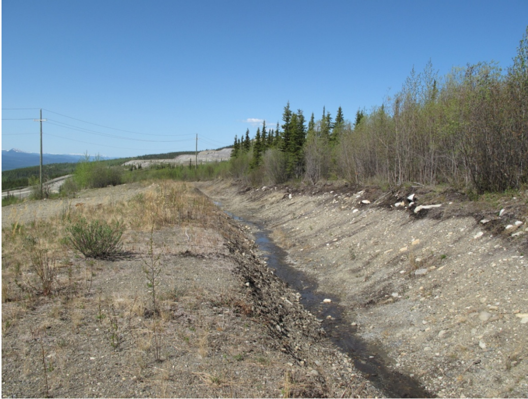
Photo 25: Middle reach of the Grum Interceptor ditch (above WTP)
