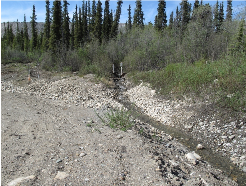
Photo 29: V-notch Weir on main stem of Grum Creek
