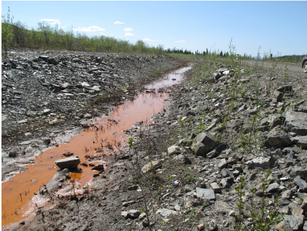
Photo 6: Seepage Collection Channel along toe of Vangorda Waste Dump
