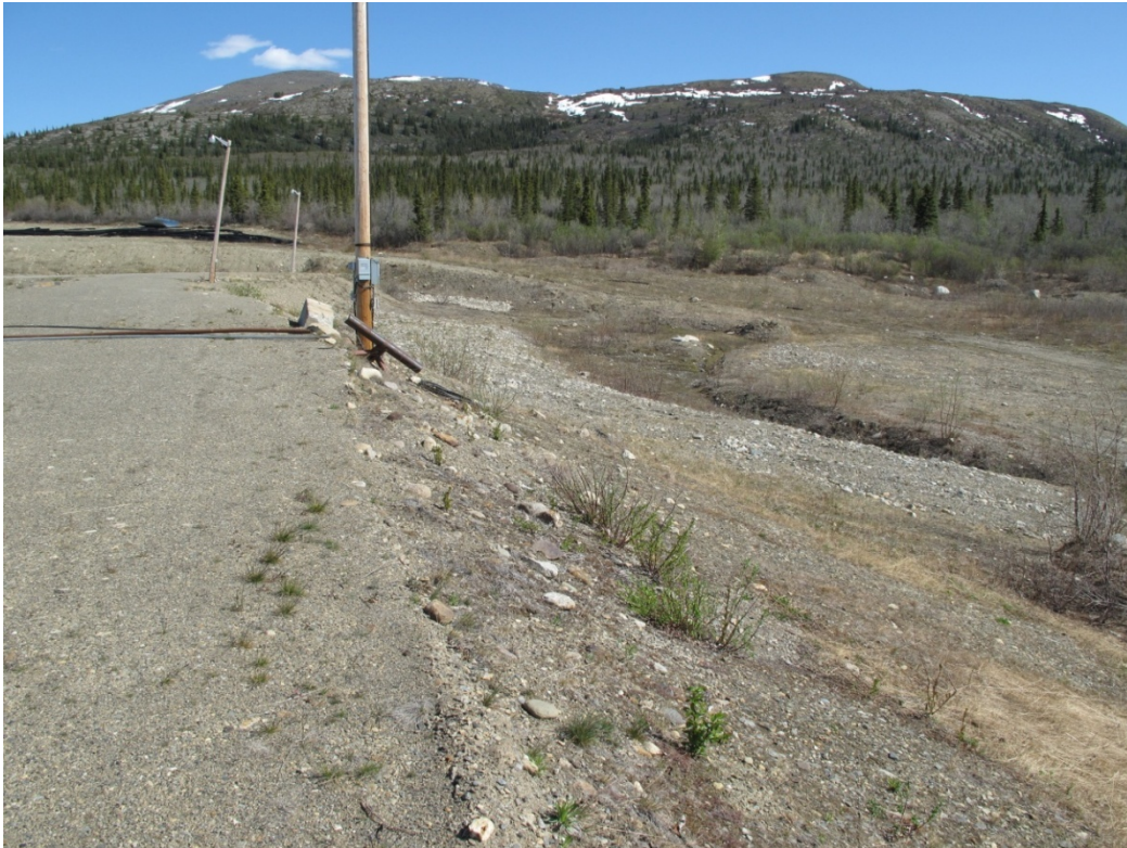
Photo 22: Downstream slopes of Dyke around Sludge Pond at Vangorda (south end)
