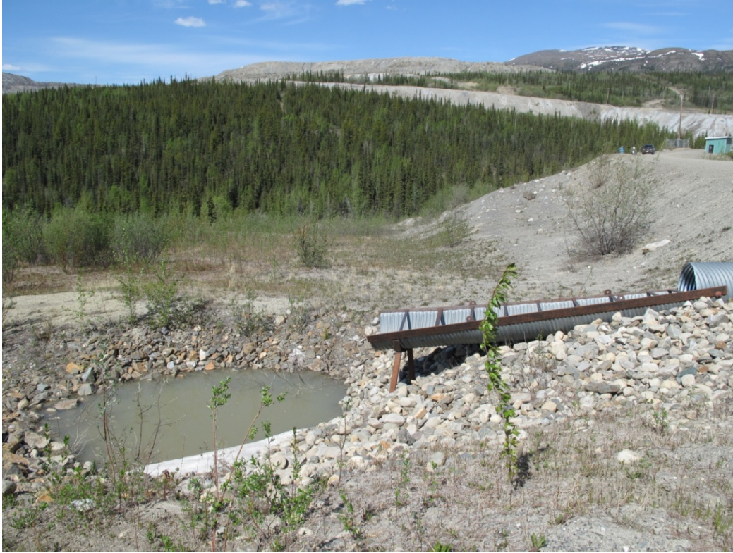
Photo 13: Emergency Spillway (outlet) from Little Creek Pond
