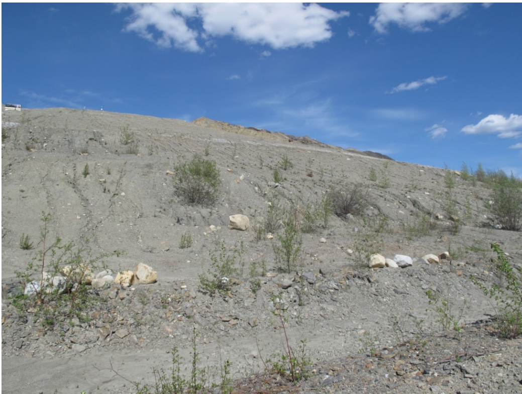
Photo 10: Erosion Gullies in the till cover on Vangorda Dump
