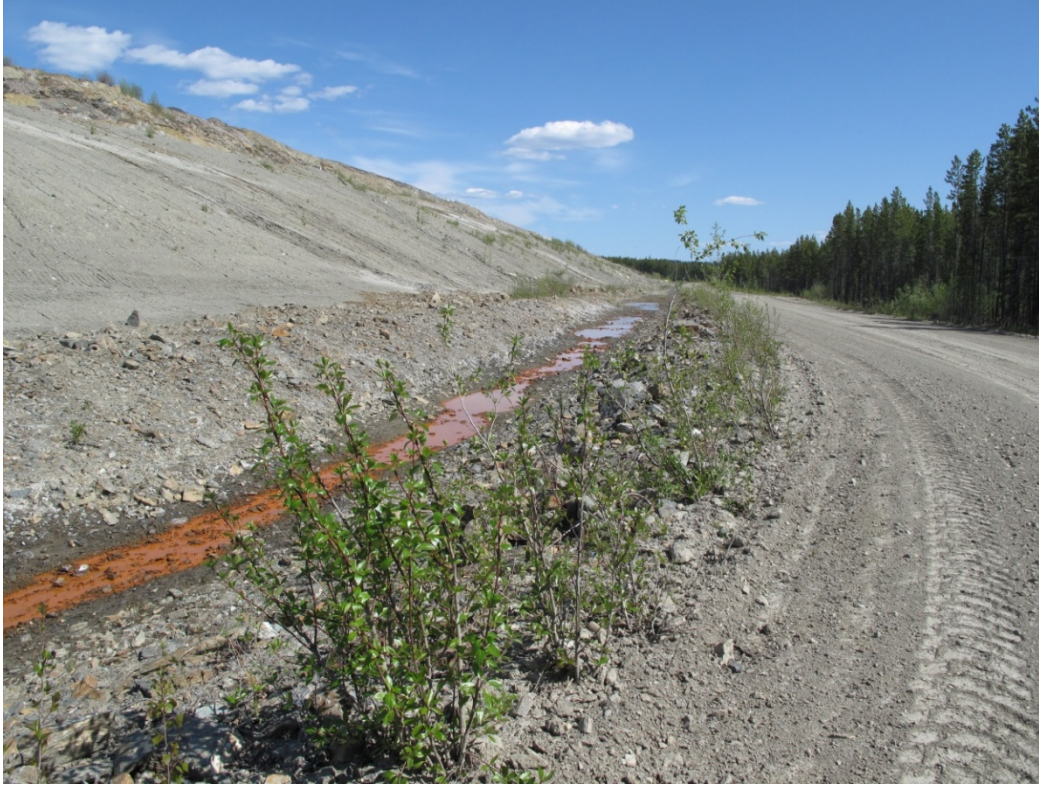
Photo 7: Seepage Collection Ditch along south toe of Vangorda Waste Rock Dump
