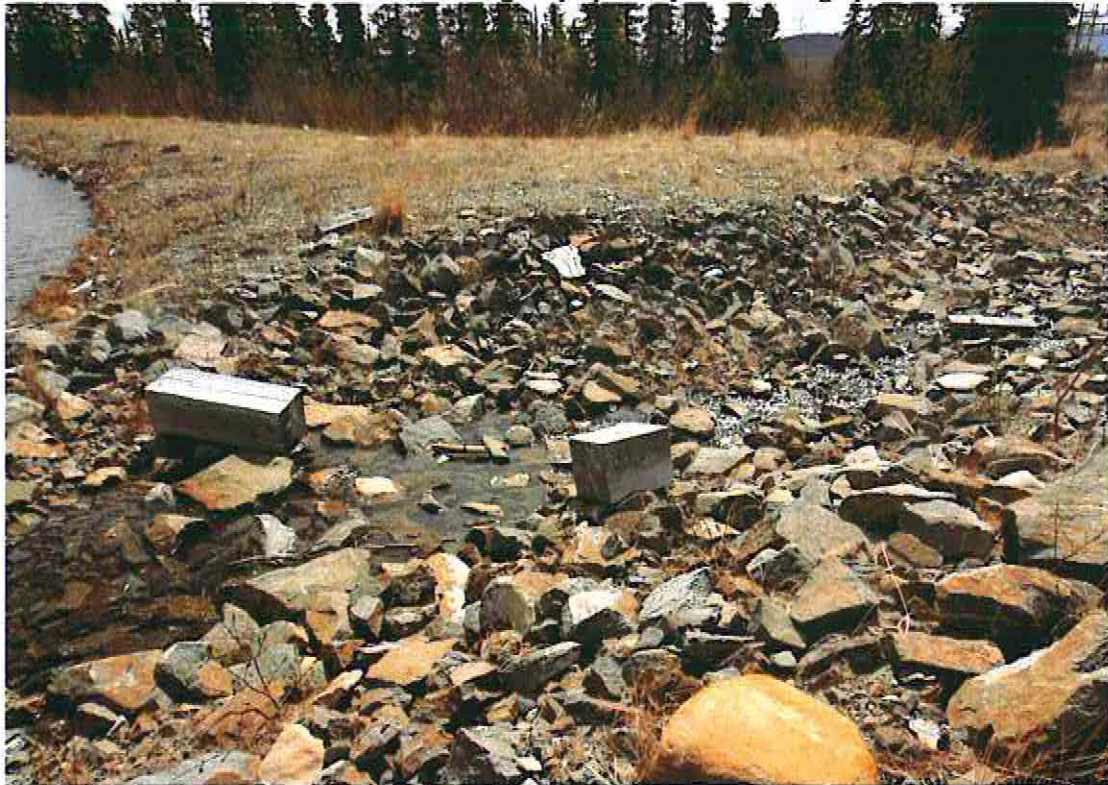
Photo 24: Spillway from Grum Settling Pond to GID
