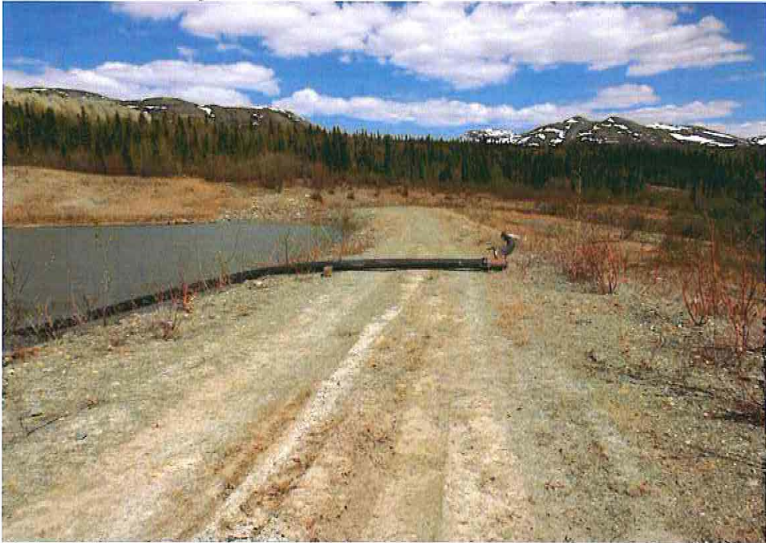
Photo 26: Sheep Pad Pond perimeter dyke
