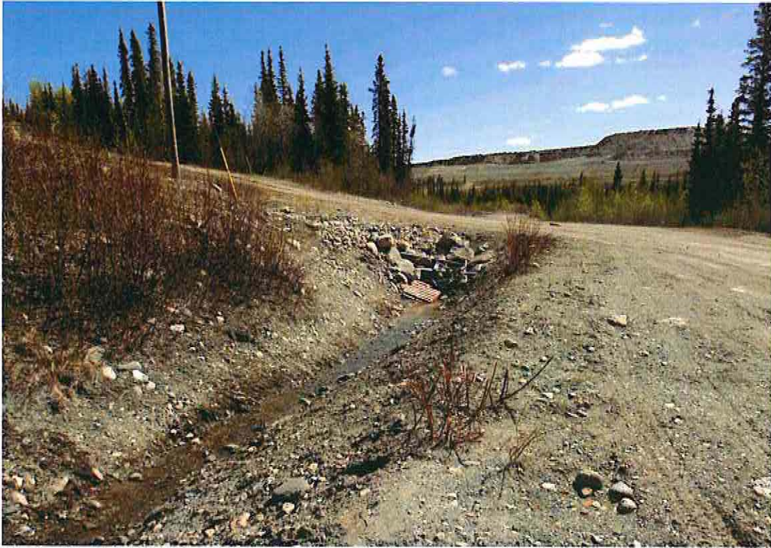
Photo 29: Culvert below V-notch weir on Grum creek
