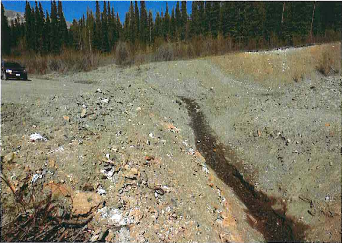
Photo 30: Diversion ditch to Moose Pond below V2A
