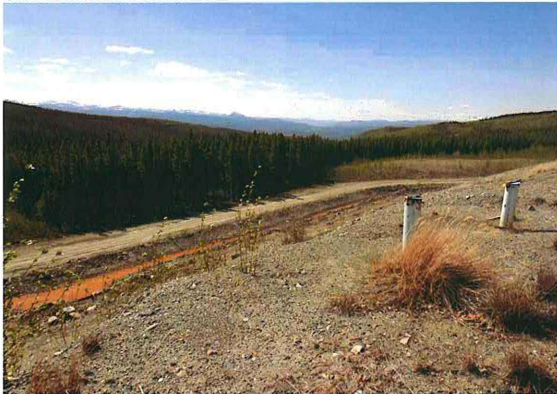
Photo 14: Piezometers P94-1A and 1B
