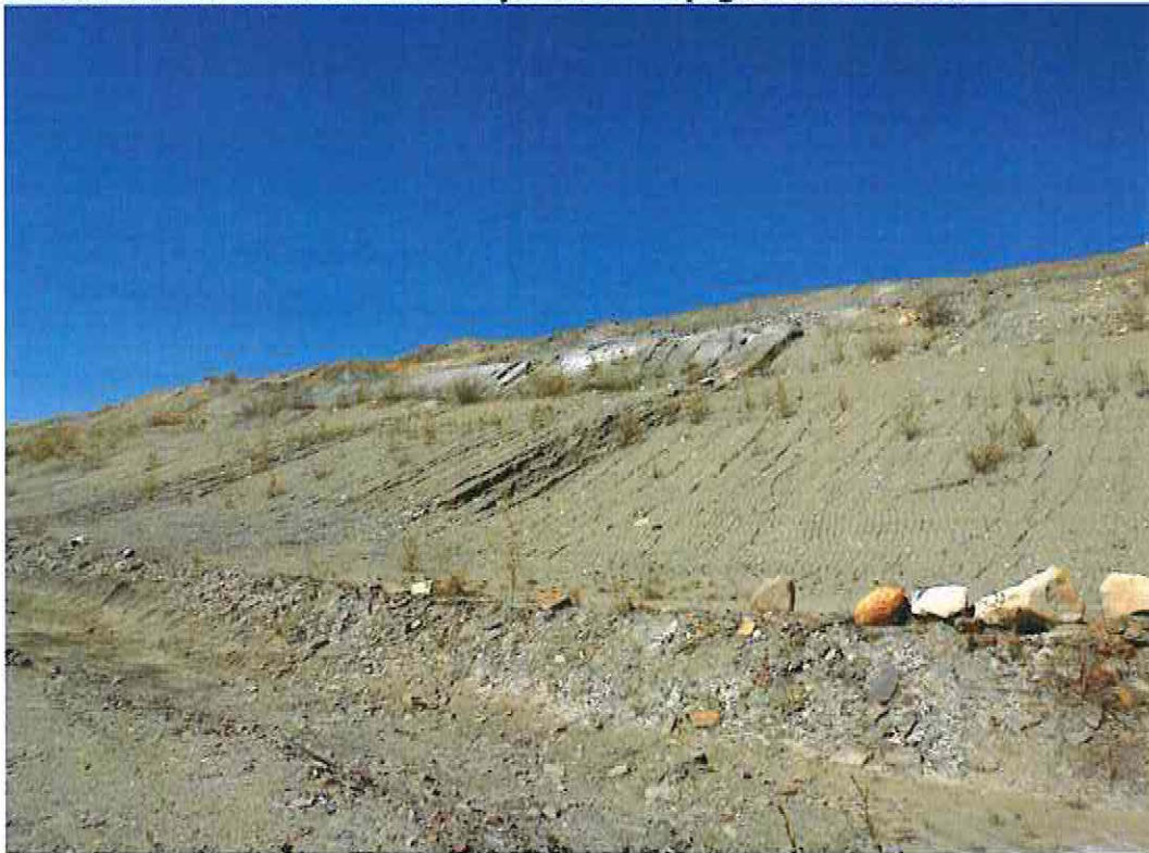
Photo 10: Erosion on the till dyke below cover trials
