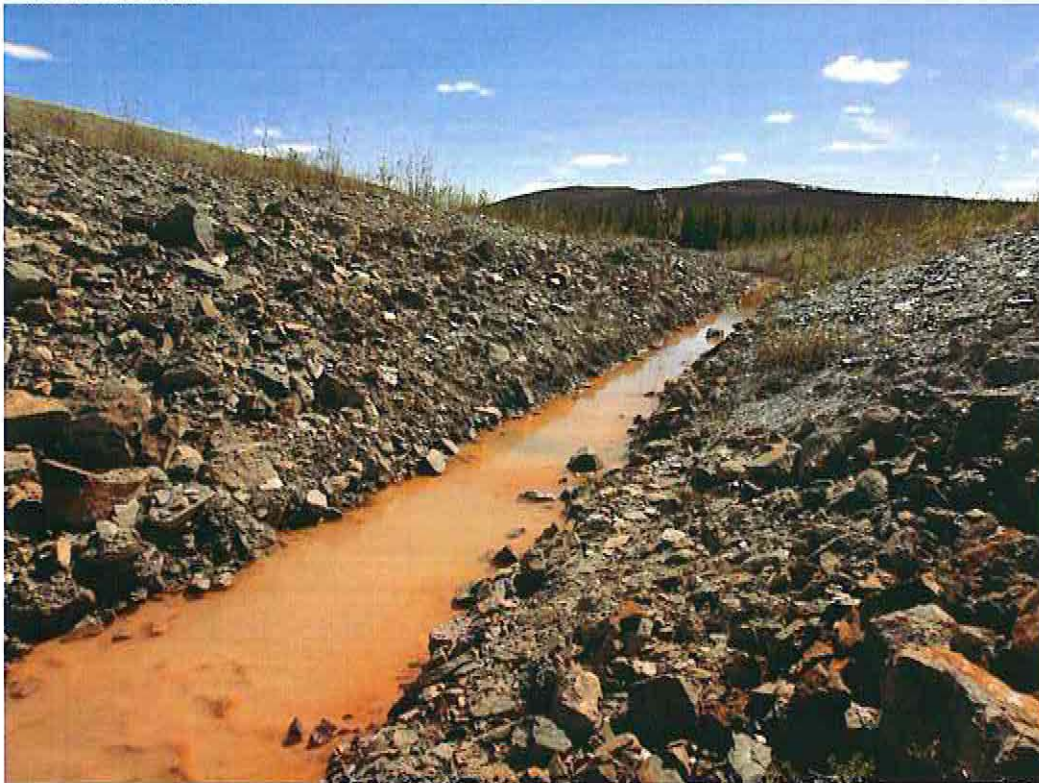
Photo 6: Seepage Collection looking back towards Drain #3
