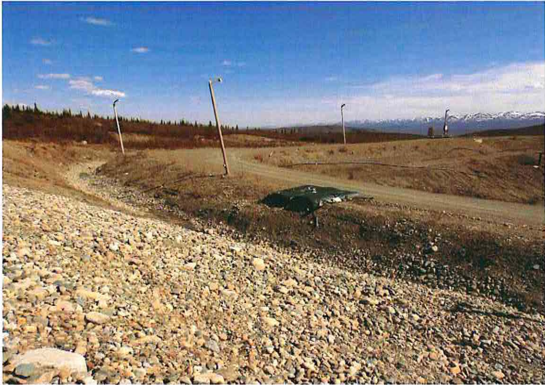
Photo 23: Proposed location of the emergency spillway at the sludge pond
