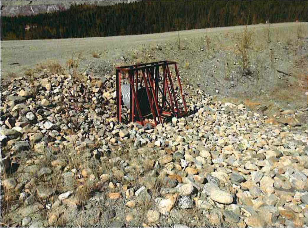
Photo 17: Inlet to the Emergency spillway at The Little Creek Pond
