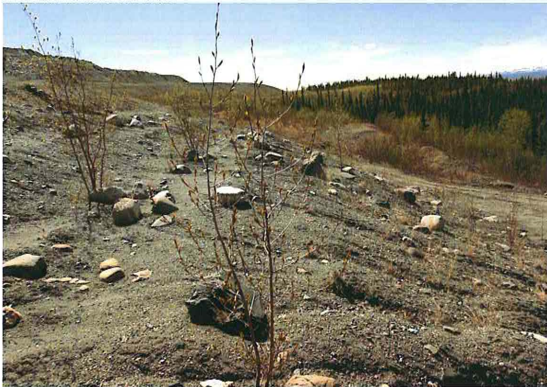
Photo 16: Downstream face of Little Creek Pond
