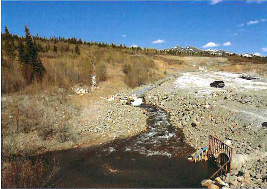
Photo 21: Plunge Pool at base of Vangorda Creek Diversion
