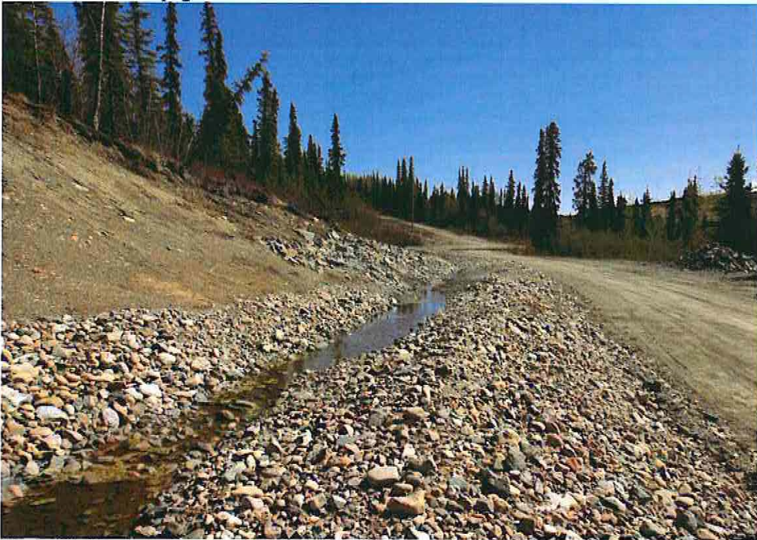
Photo 28: Bentomat Lined Ditch from V-15
