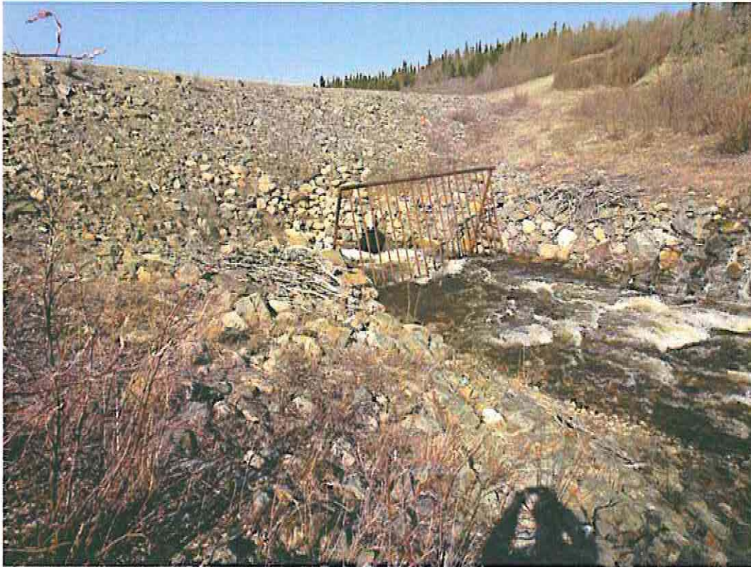
Photo 15: Trashrack at Headworks of Vangorda Creek Diversion
