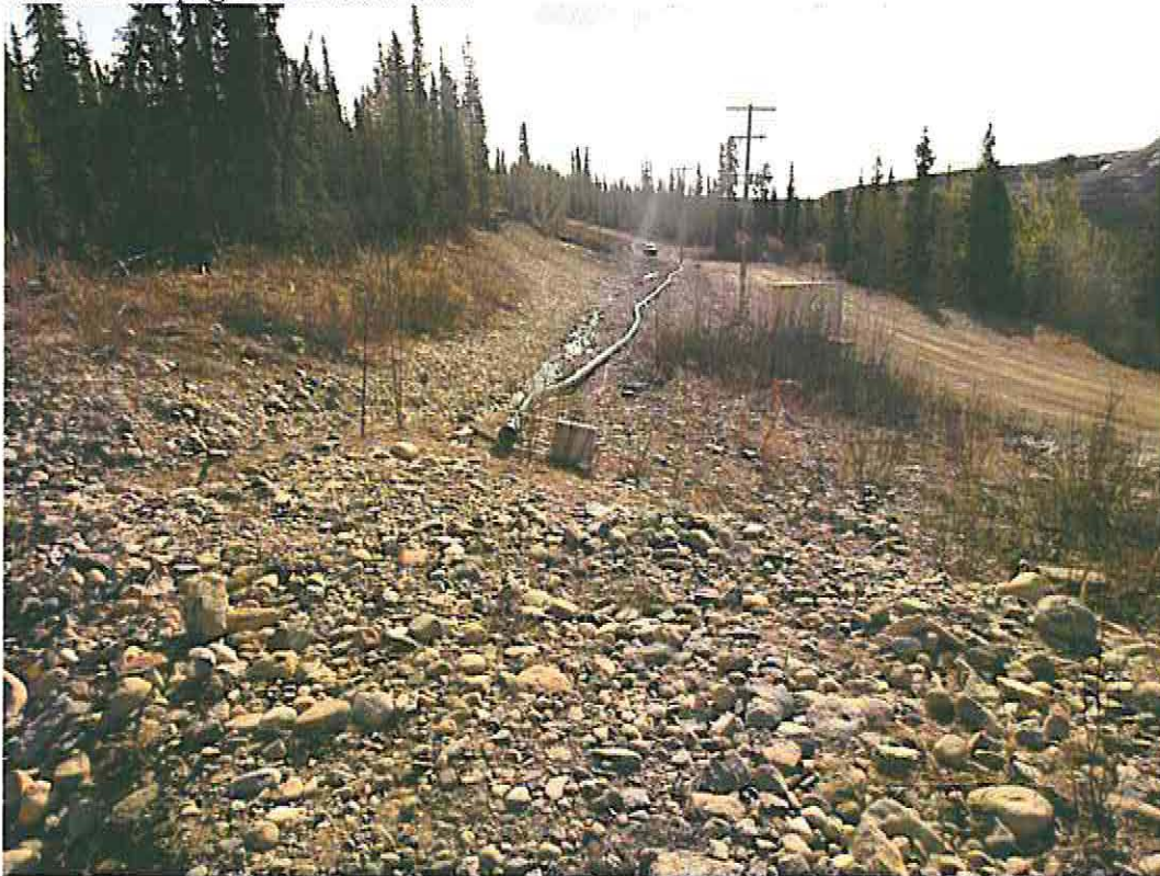
Photo 24: Bentomat Lined Ditch from V-15
