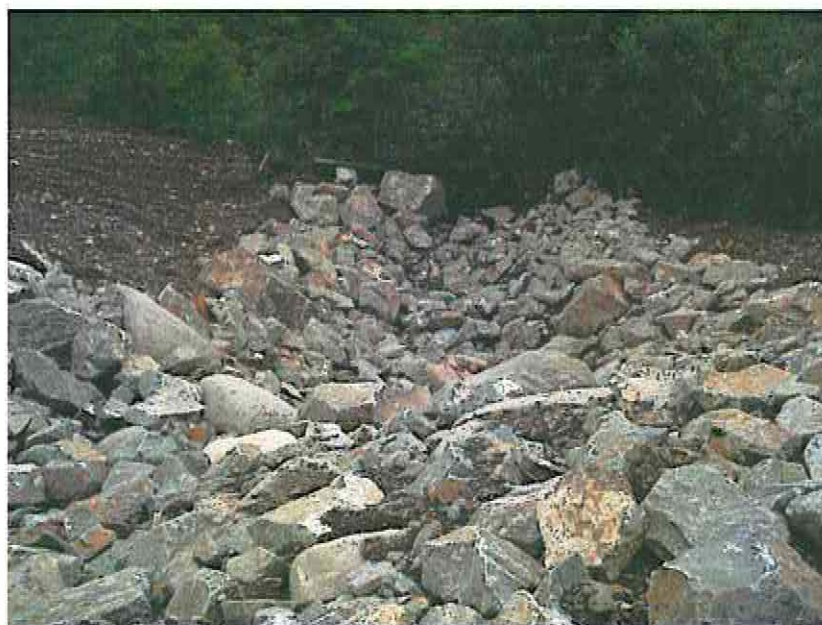
Photo 6: Rip rap on temporary flow path constructed mid-May (not in use at time of photo) (June 26, 2011)
