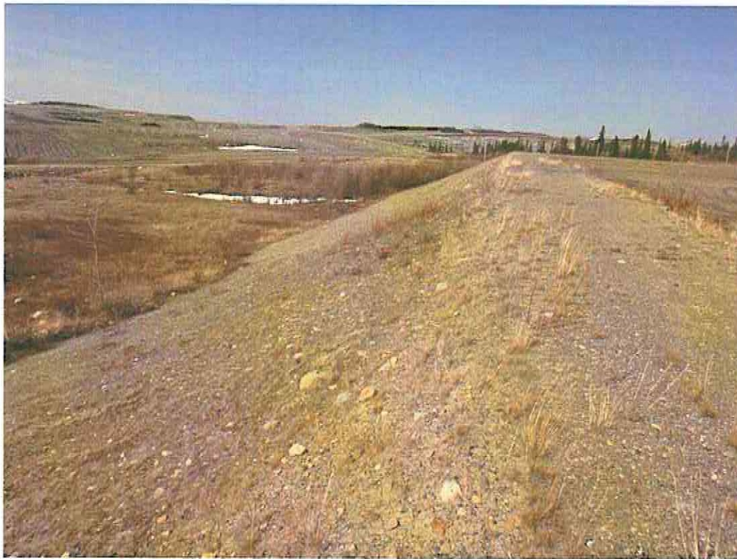
Photo 35: Downstream Slope of Sludge Pond Embankment
