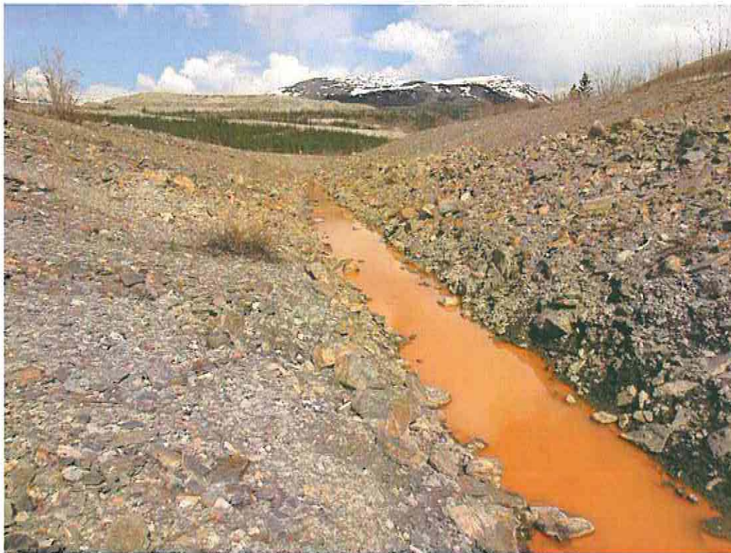
Photo 7: Seepage Collection Ditch at Nose of Vangorda Waste Rock Dump.
