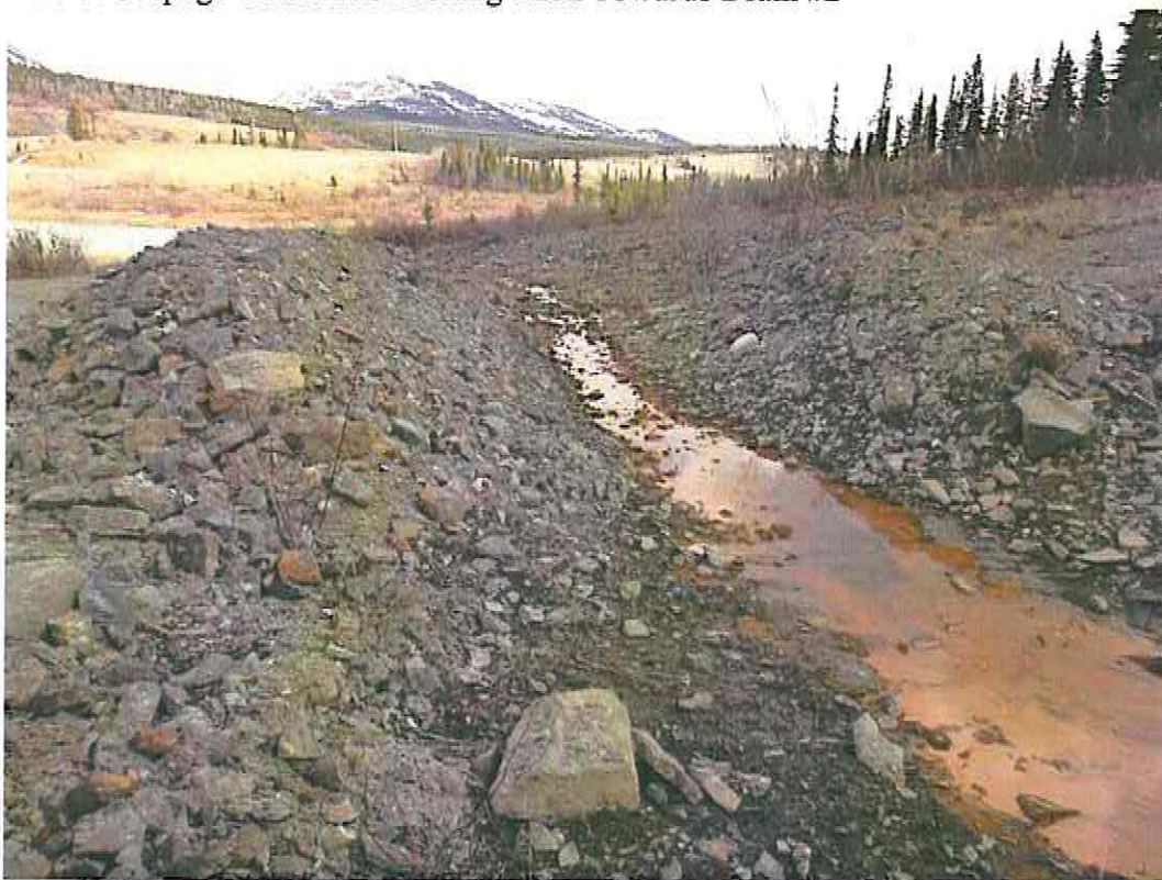
Photo 6: Seepage Collection Ditch Looking Downstream Towards LCP
