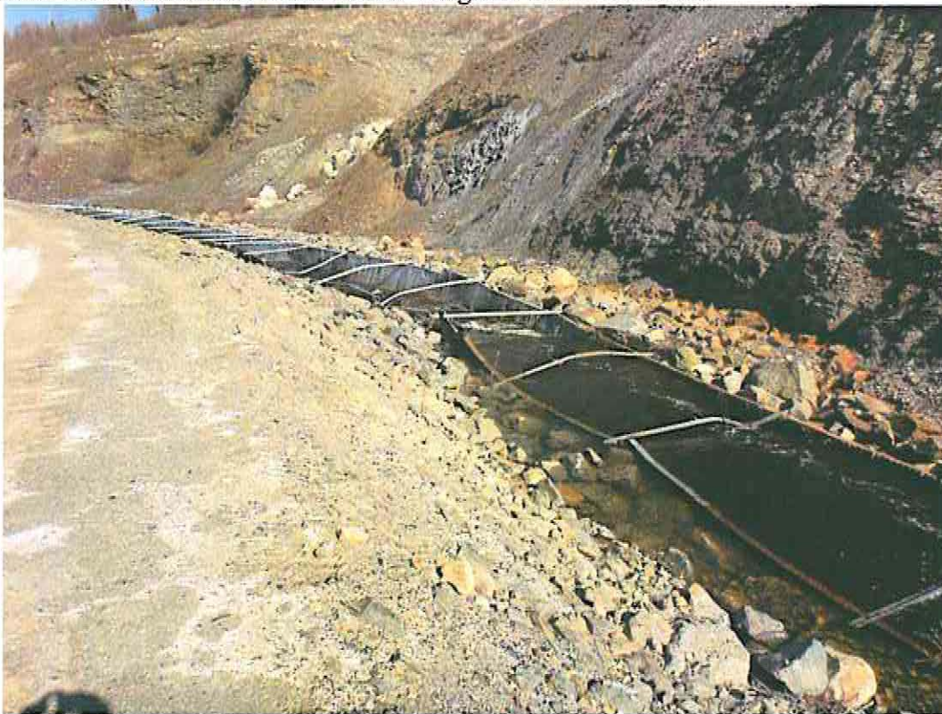
Photo 16: Vangorda Creek Diversion
