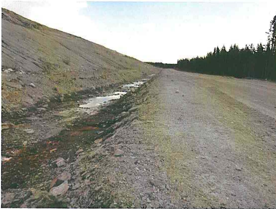
Photo 5: Seepage Collection Looking Back Towards Drain #2
