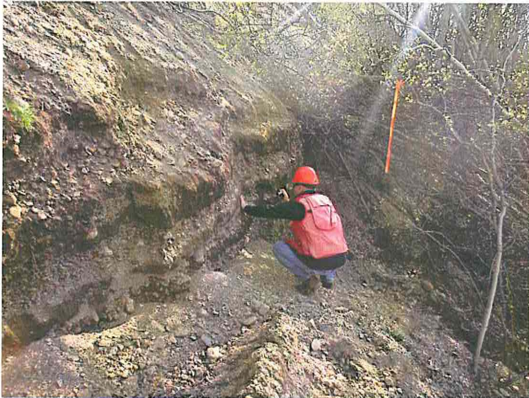
Photo 32: Seepage Zone Below Moose Pond
