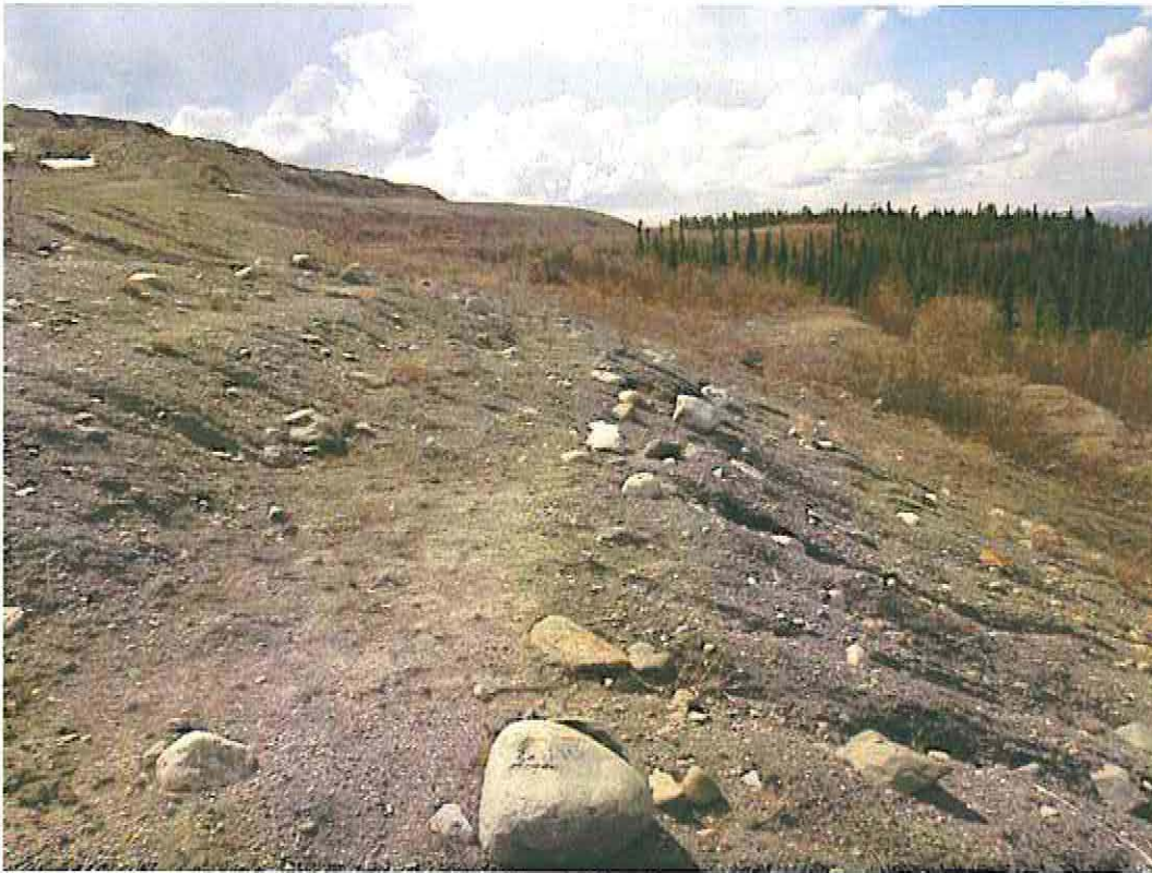
Photo 11: Downstream Face of Little Creek Pond
