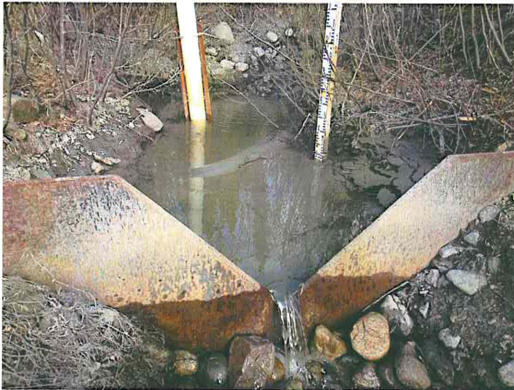
Photo 28: V-notch Weir on Main Stem of Grum Creek
