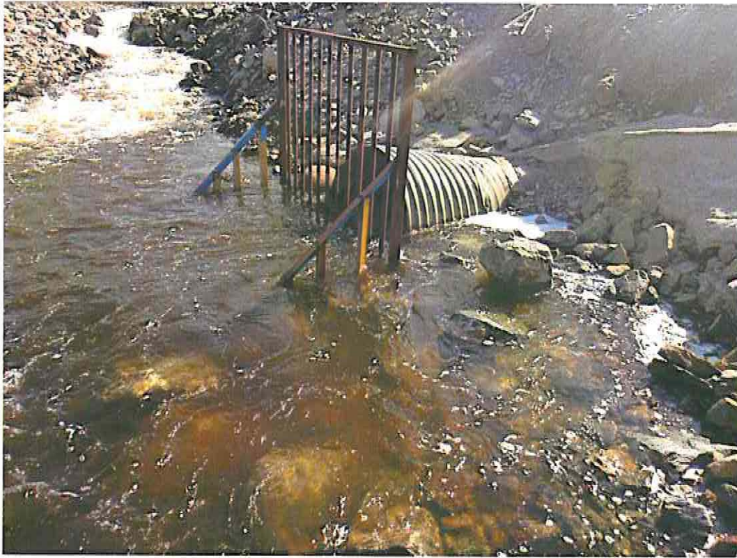
Photo 19: Plunge Pool at Base of Vangorda Creek Diversion
