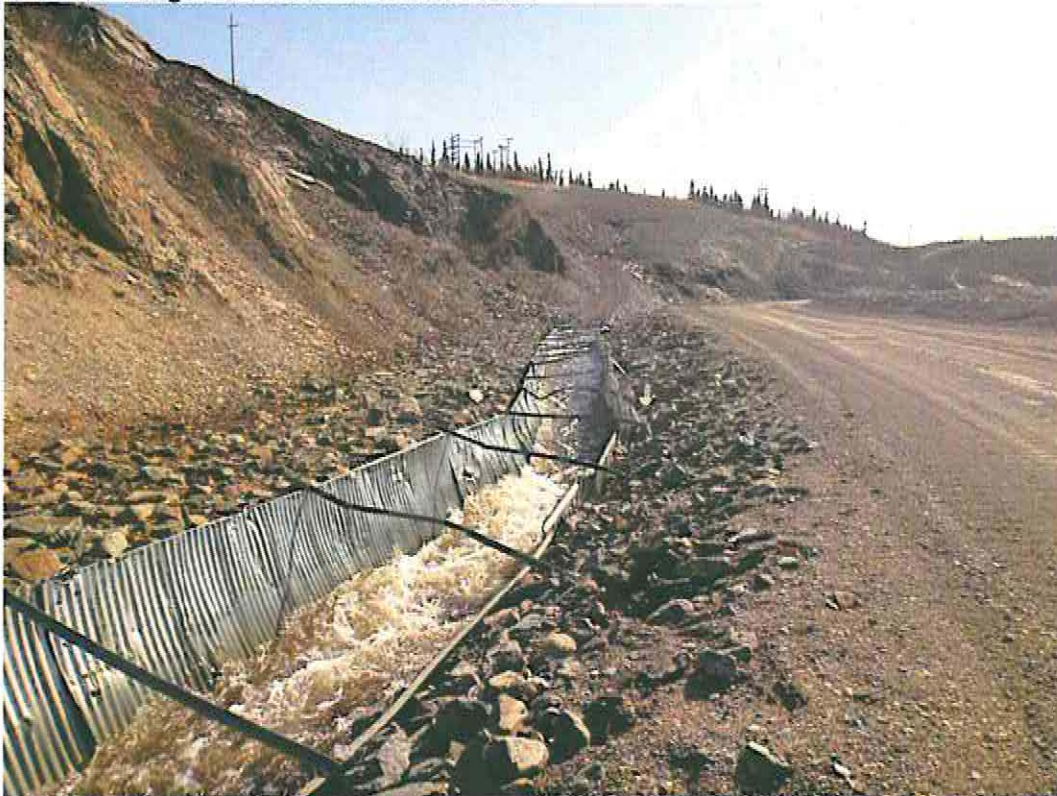
Photo 18: Vangorda Creek Diversion
