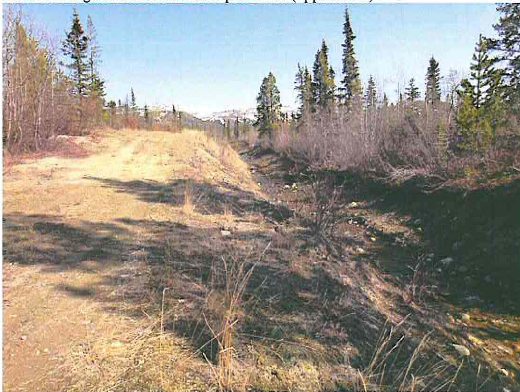
Photo 22: Vangorda Pit North Interceptor Ditch (lower reach)
