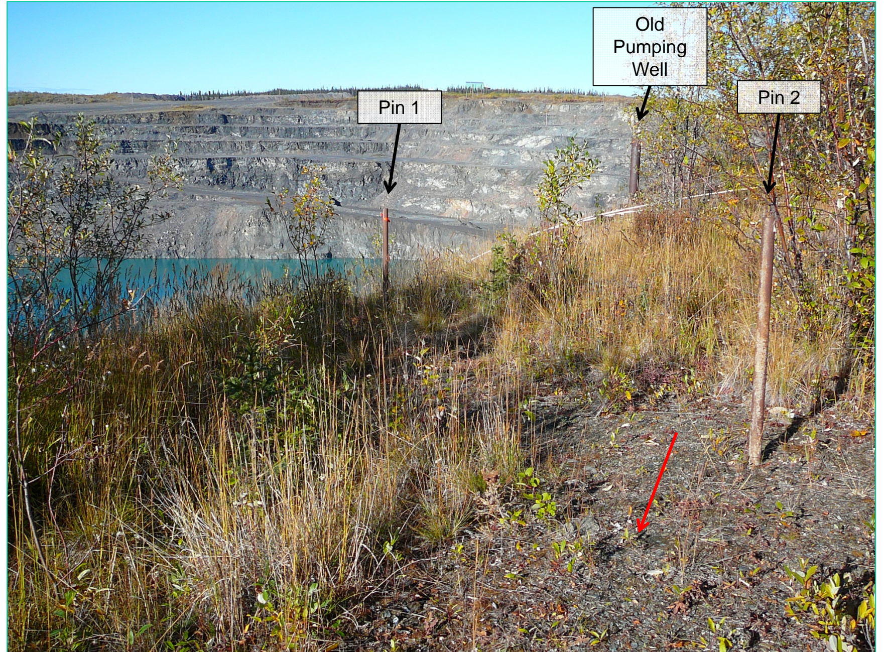
Photograph D-9 Grum Pit recent crack, located across the second pin from the crest in the North Array. Approximate location indicated by red arrow. View looking west.
