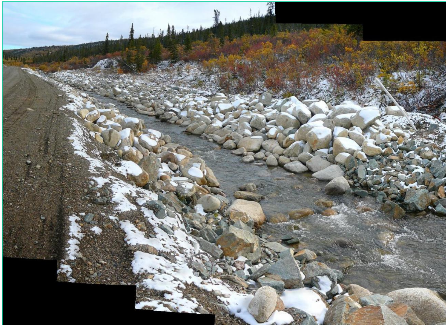
Photograph A-8 Faro Creek Diversion Channel. View looking northwest.
