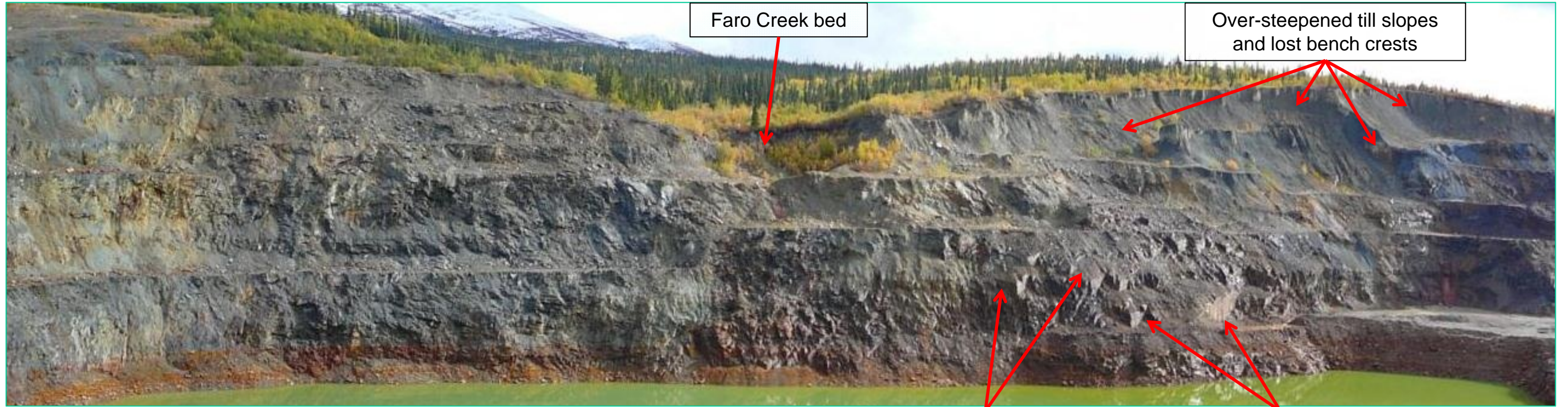
Photograph E-18 Vangorda Pit northeast wall. View looking northeast.
