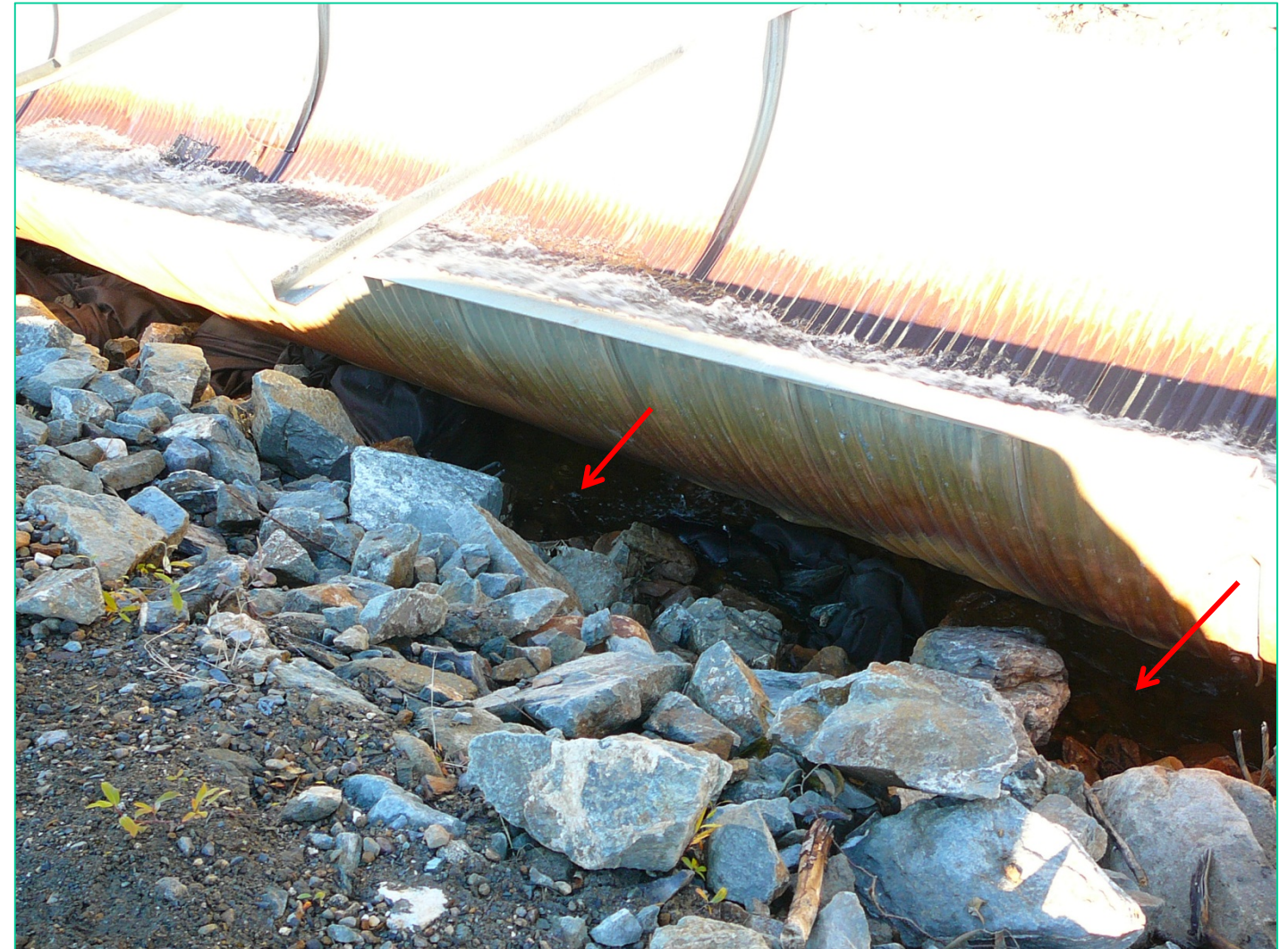
Photograph E-10 Vangorda Pit – Water flowing in channel beneath flume indicated by red arrows.
