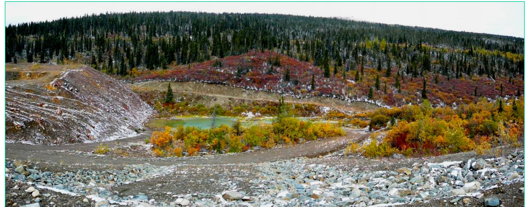
Photograph A-7 Faro Pit – North Instability Zone. Pond of water to the north of the North Instability Zone. This water drains into a creek, which drains into the pit to the north of the North Instability Zone.
