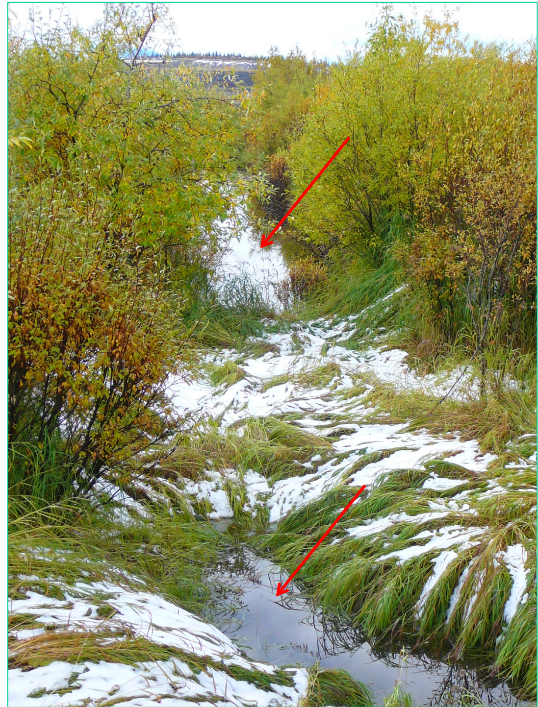
Photograph D-13 Grum Pit – areas of ponded water behind crest, in vegetated area. View looking west.
