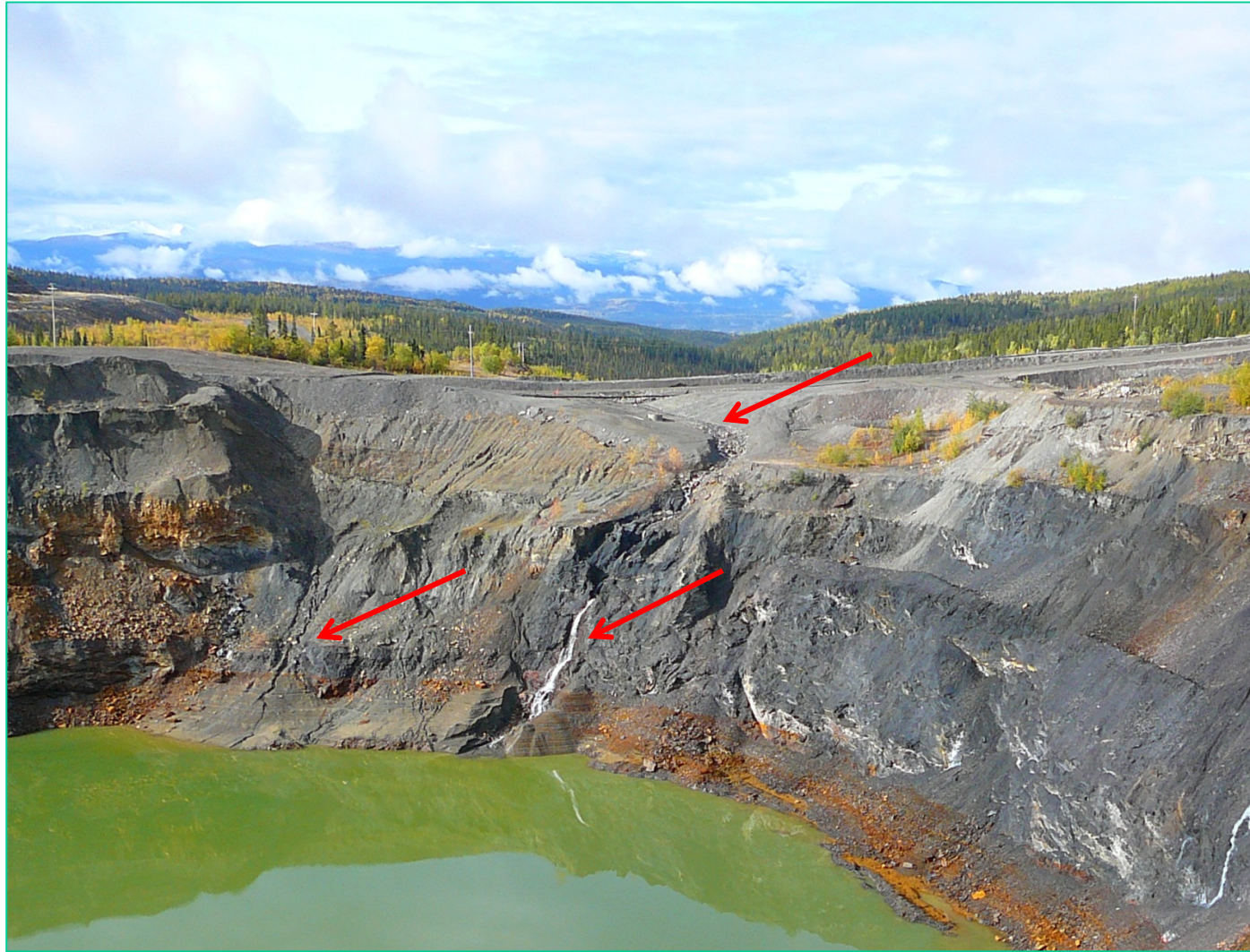
Photograph E-14 Vangorda Pit – Water flowing into pit in northwest corner.
