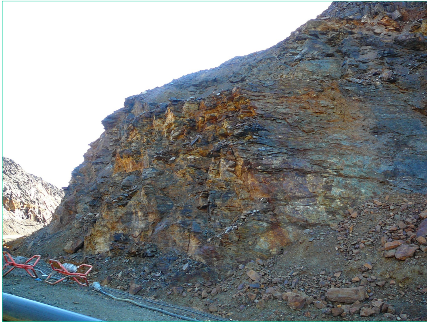
Photograph E-5 Vangorda Pit – Mapping Station 3. View looking south.
