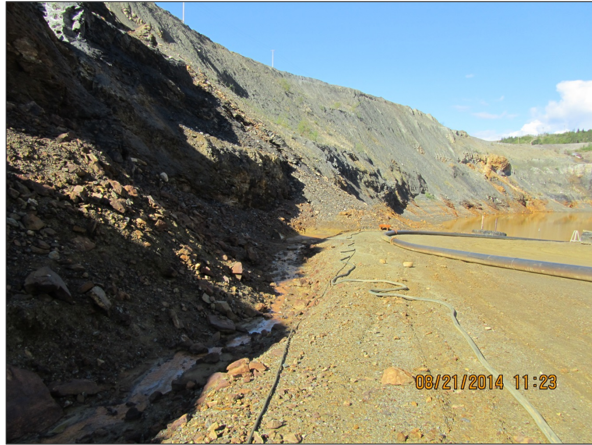
CABLES AT TOE OF SLOPE
