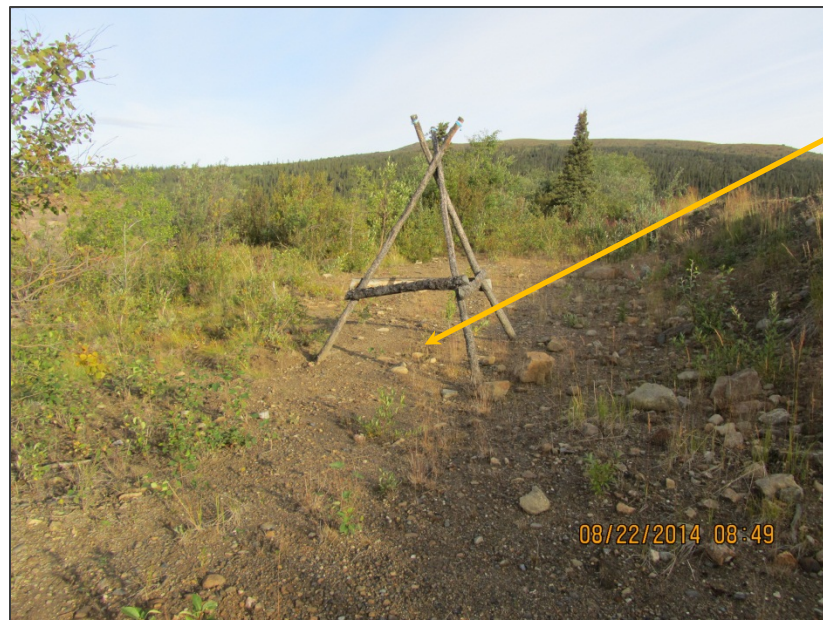
15342 STRUCTURE IN GOOD CONDITION
