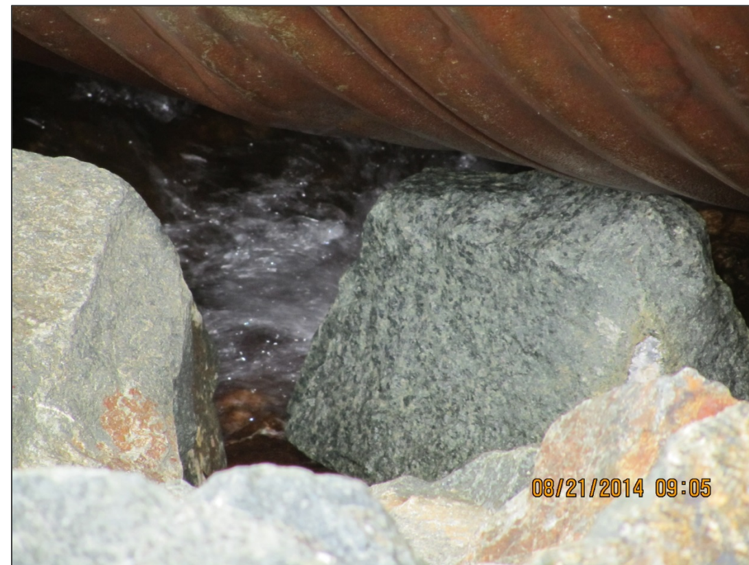
WATER FLOWING BENEATH VANGORDA FLUME
