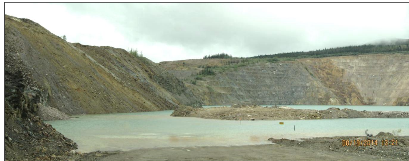
NO BERM AT END OF ZONE 2 ACCESS ROAD
