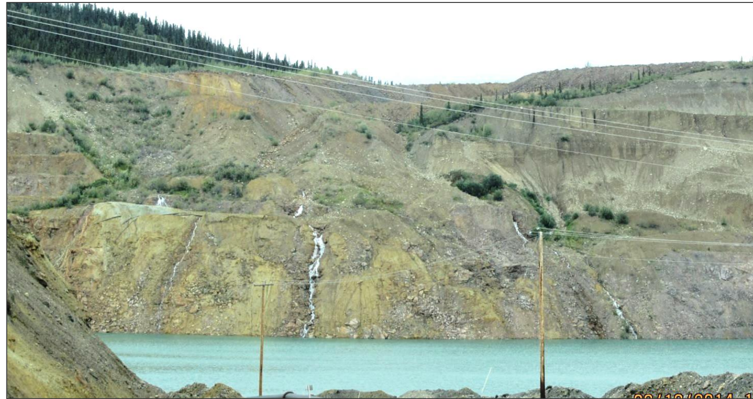
SEEPAGE AND SURFACE RUNOFF
