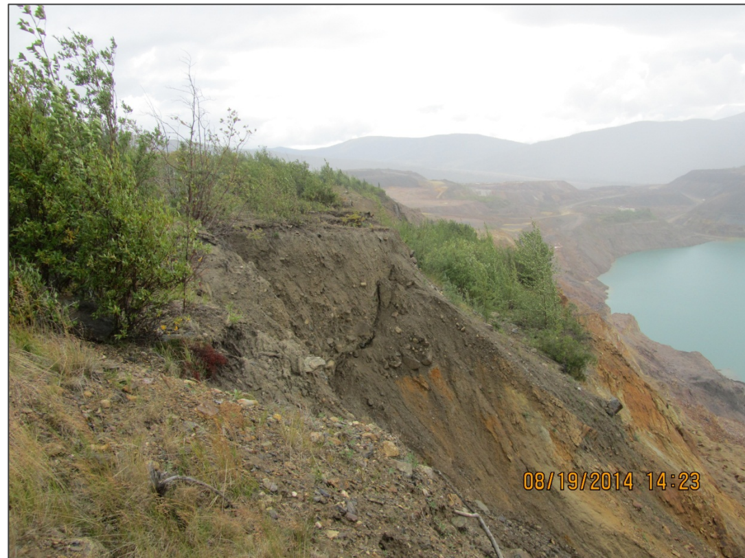
BACKSCARP SLUMPING
