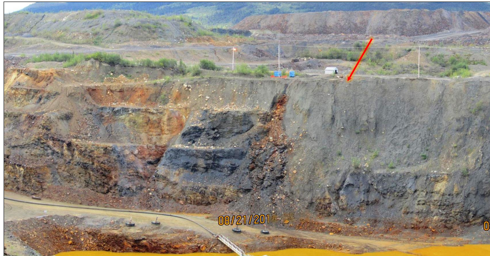
EMERGENCY DISCHARGE ON SOUTHWEST WALL
