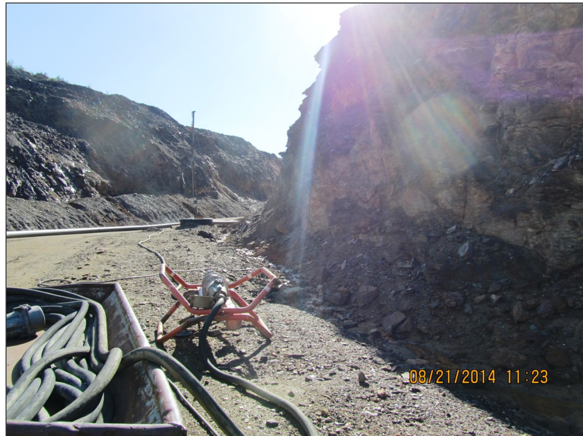
EQUIPMENT NEAR SLOPE
