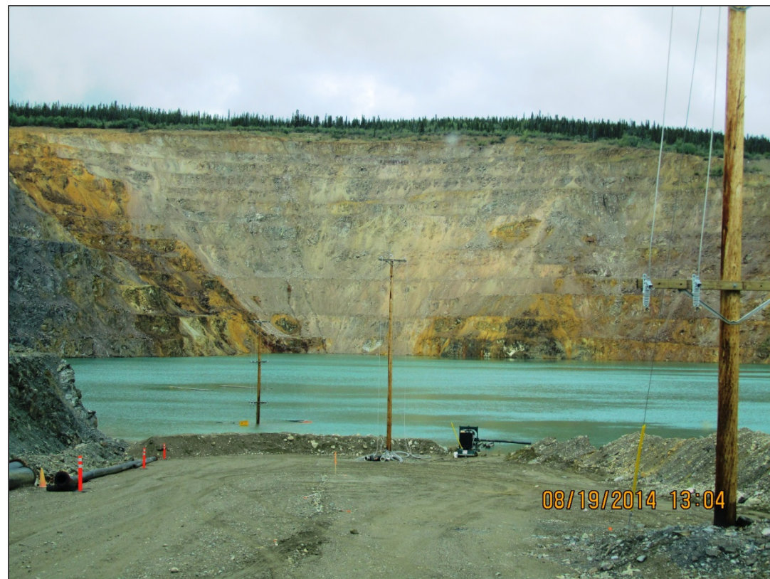
BERM AT END OF WEST ACCESS ROAD
