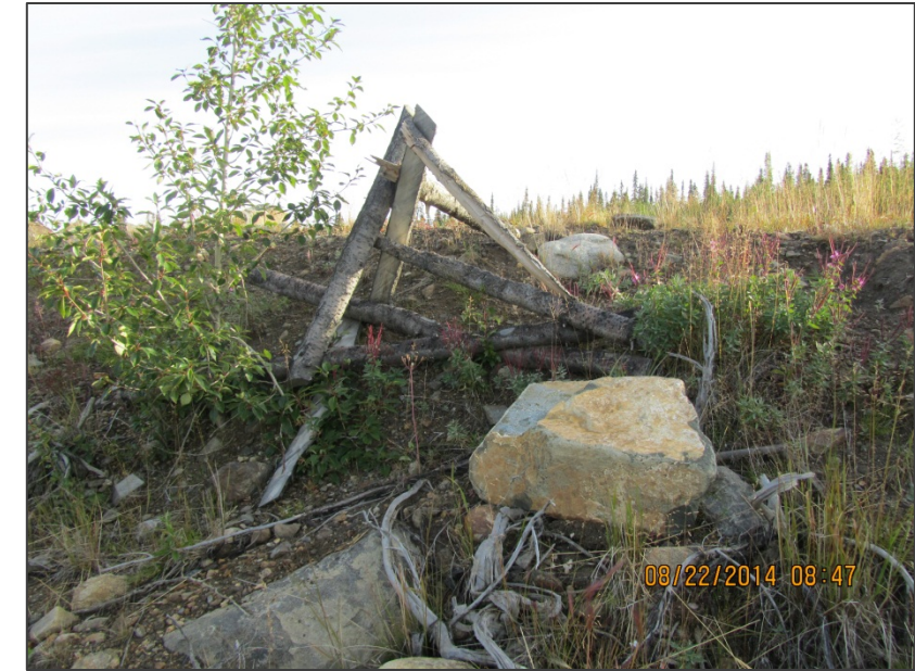
15742? COULD NOT FIND TAG OR PIN, AND STRUCTURE IS COLLAPSED
