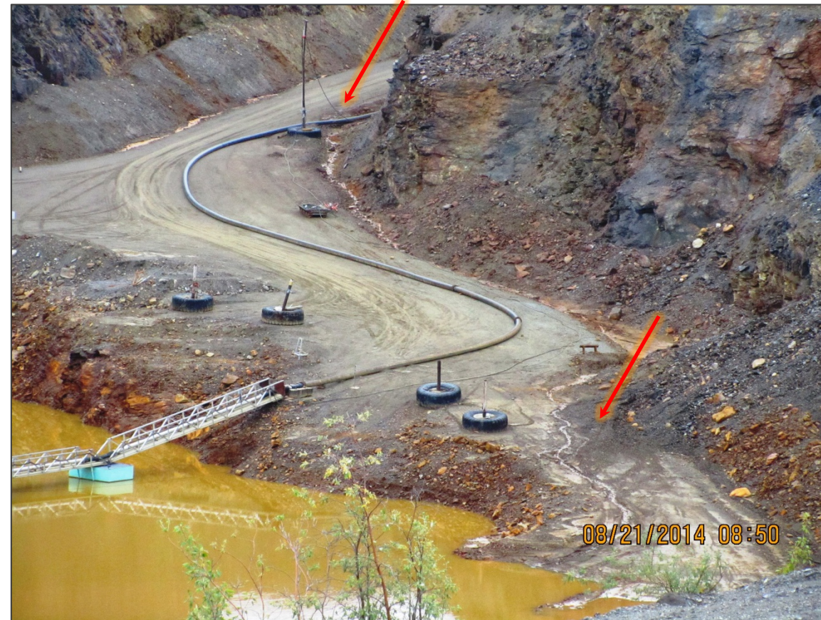
POWER POLE AND CABLES NEAR SLOPE, AREA WITH NO BERM OR DITCH
