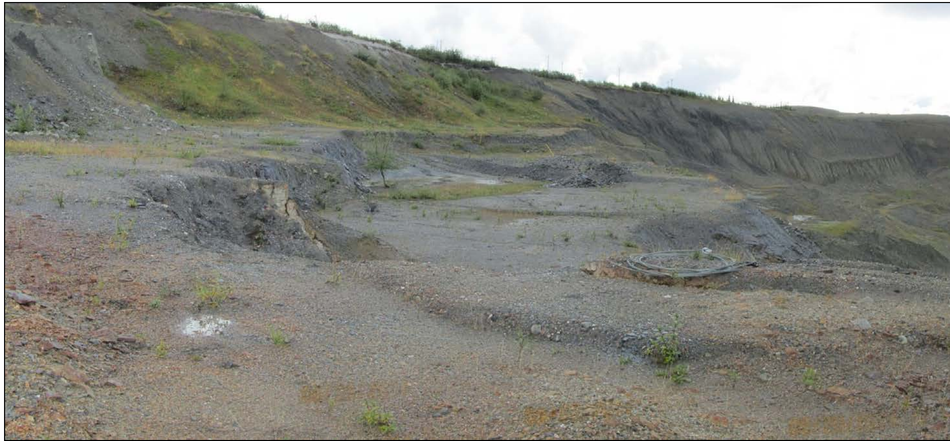
2014 PHOTOGRAPH OF ROCK BENCH TO THE NORTH OF THE INSTABILITY ZONE, EAST WALL, VIEW LOOKING SOUTH
