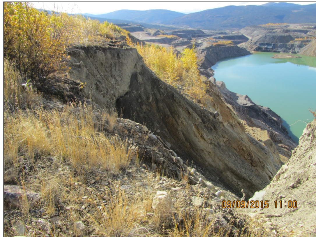
BACKSCARP SLUMPING
