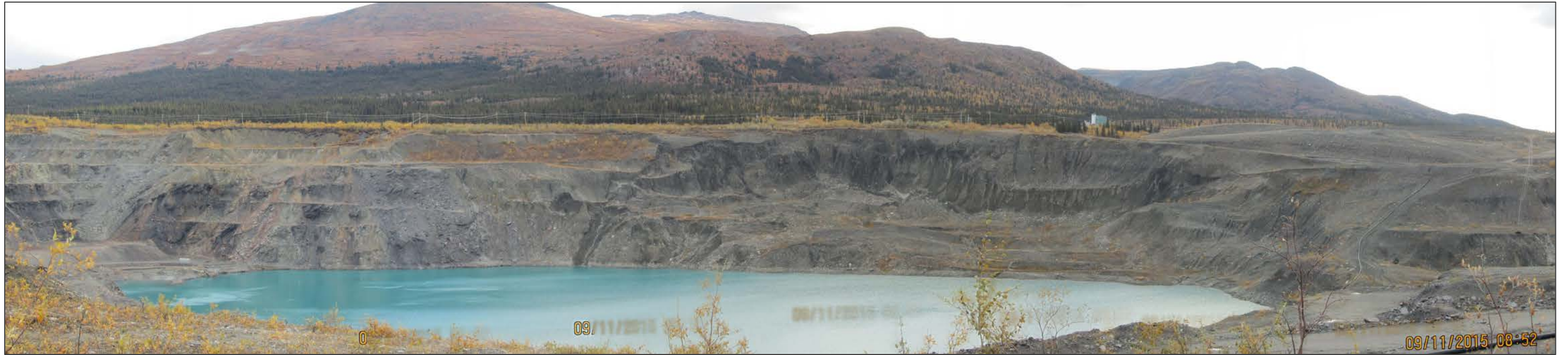
EAST WALL AND INSTABILITY ZONE, VIEW LOOKING EAST
