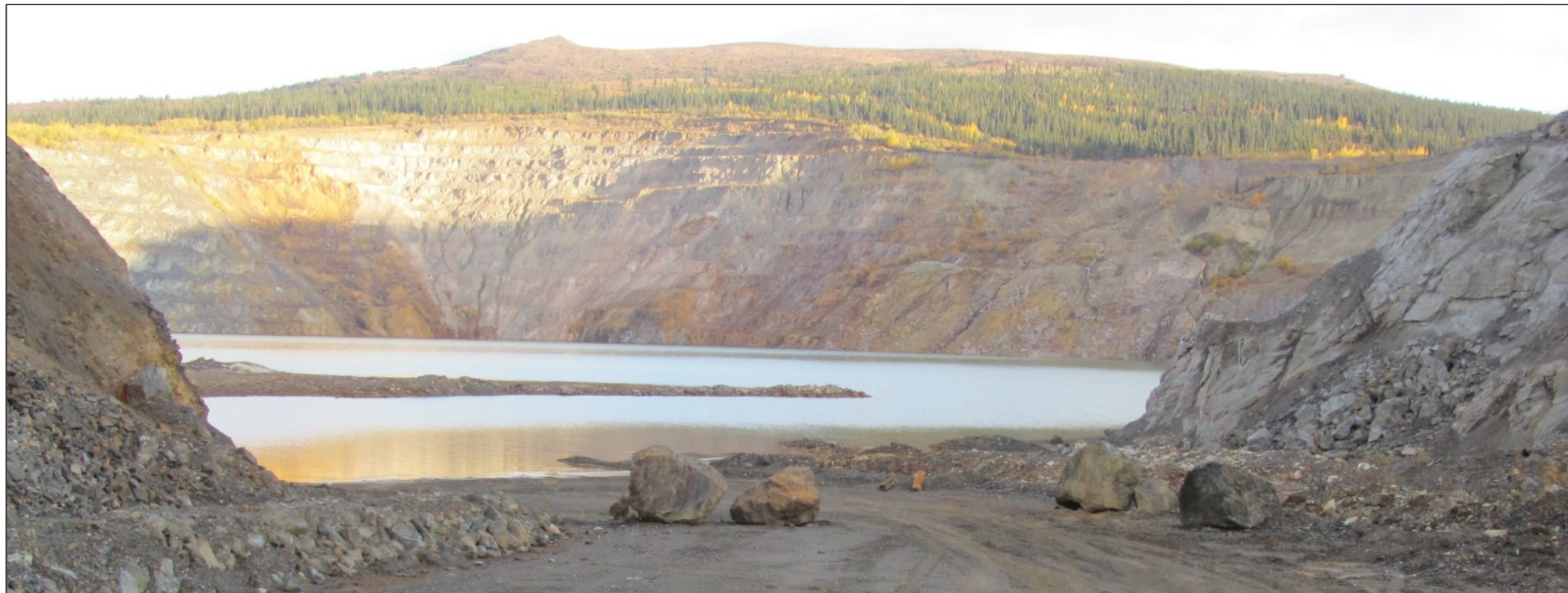
BOULDERS AT END OF ZONE 2 ACCESS ROAD, SOUTH SIDE OF PIT, VIEW LOOKING NORTH
