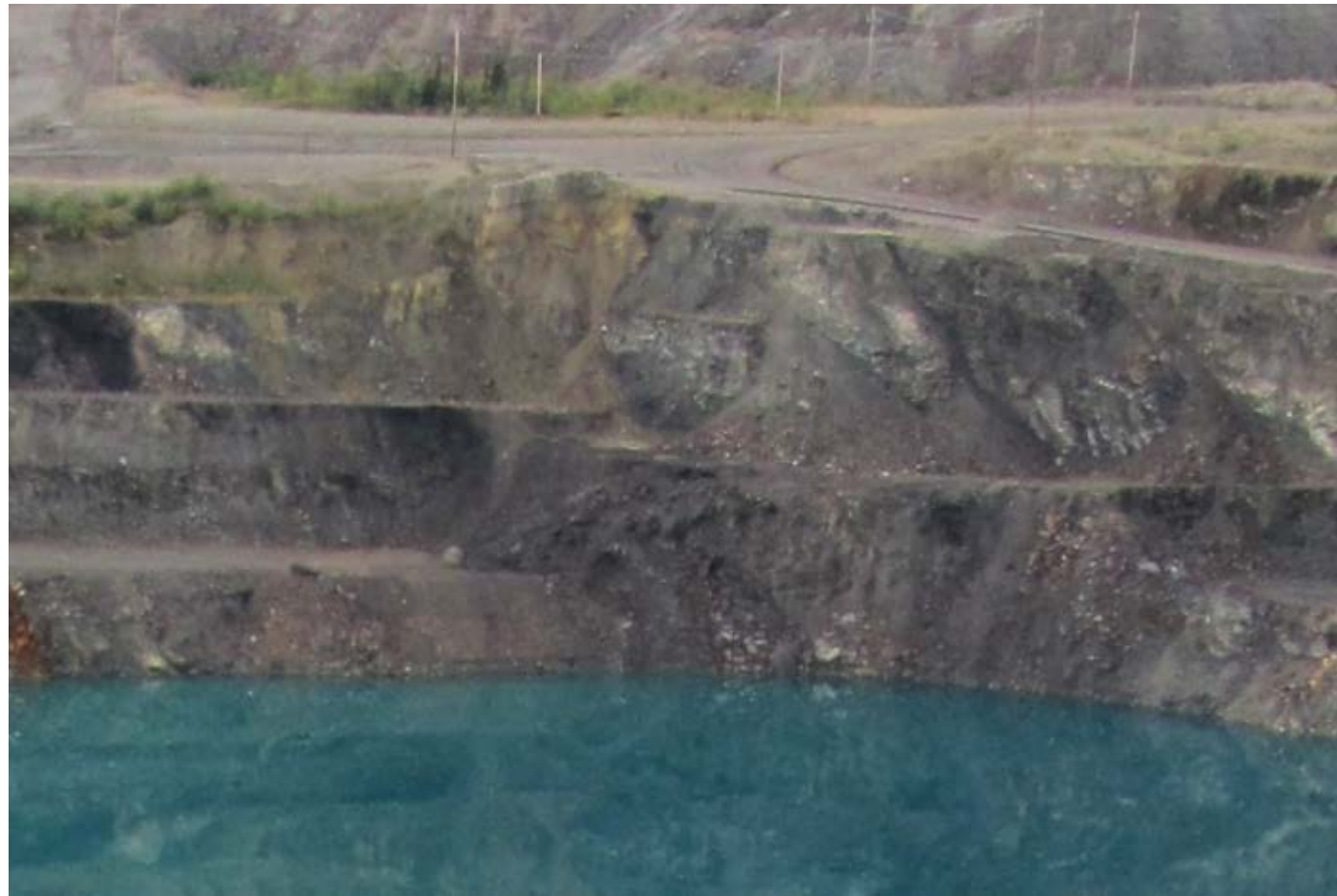
2014 PHOTOGRAPH OF ROCK SLOPE IN SOUTHWEST CORNER OF GRUM PIT. VIEW LOOKING SOUTHWEST.
