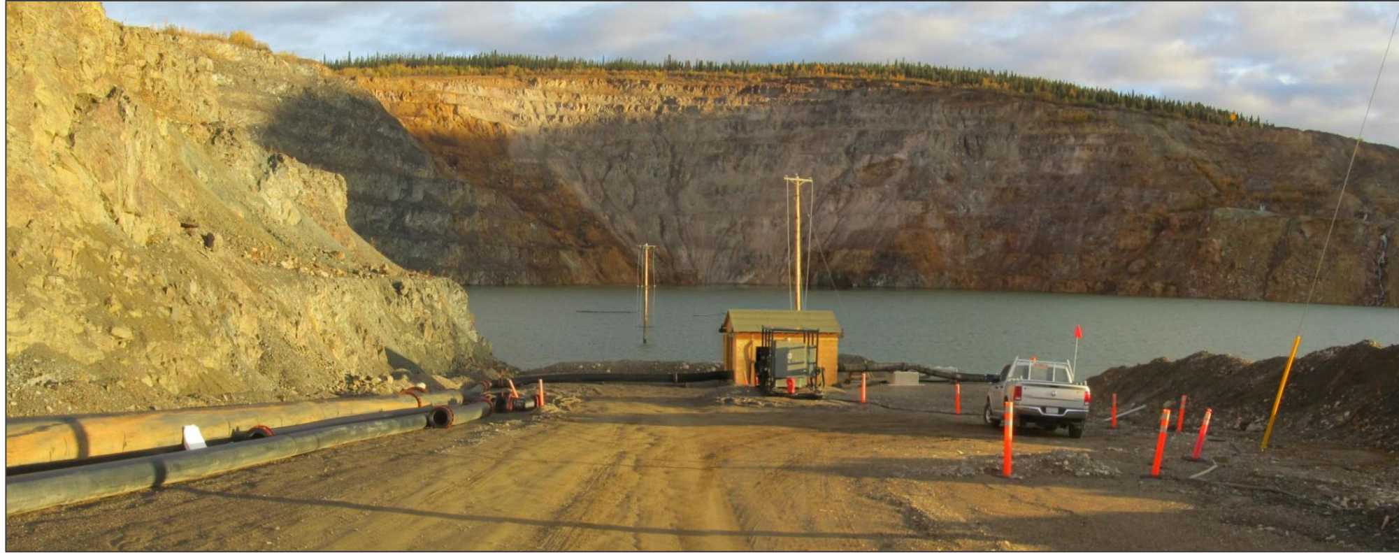
BERM AT END OF WEST ACCESS ROAD, WEST SIDE OF PIT, VIEW LOOKING NORTH
