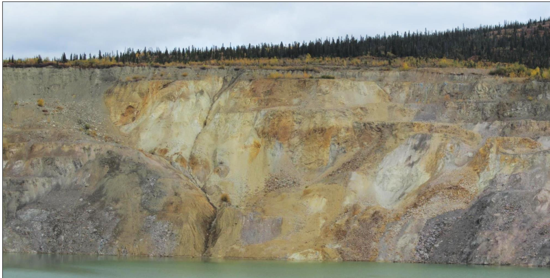
2015 PHOTOGRAPH OF NORTH INSTABILITY ZONE, VIEW LOOKING EAST
