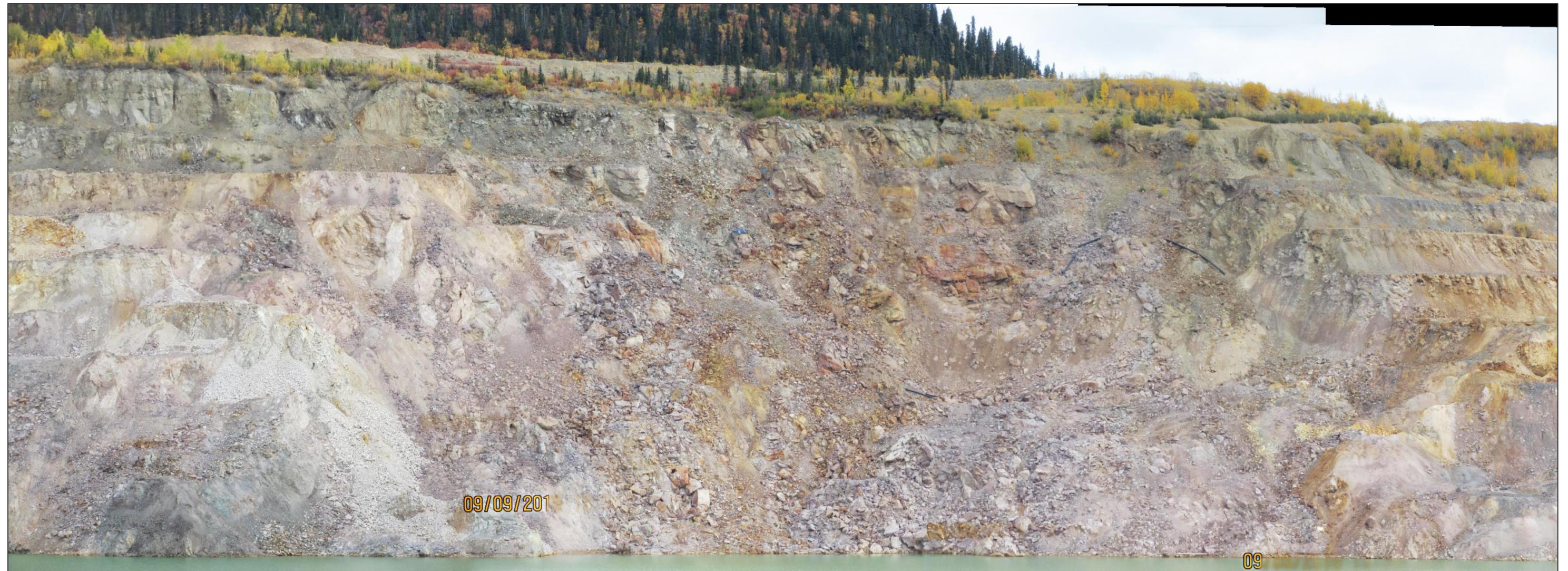
SOUTH INSTABILITY ZONE, EAST WALL, VIEW LOOKING SOUTHEAST
