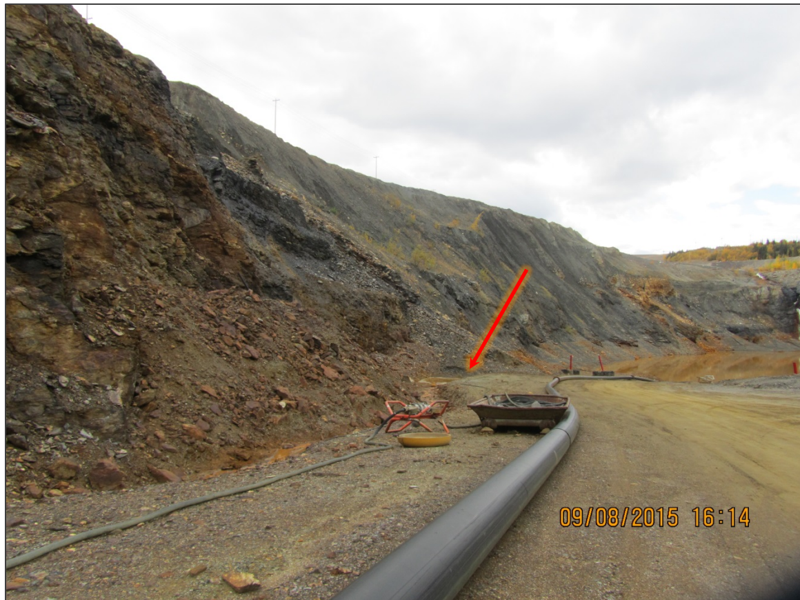
DITCH SERVES AS ROCKFALL CATCHMENT ON EAST SIDE OF ACCESS ROAD, VIEW LOOKING NORTH
