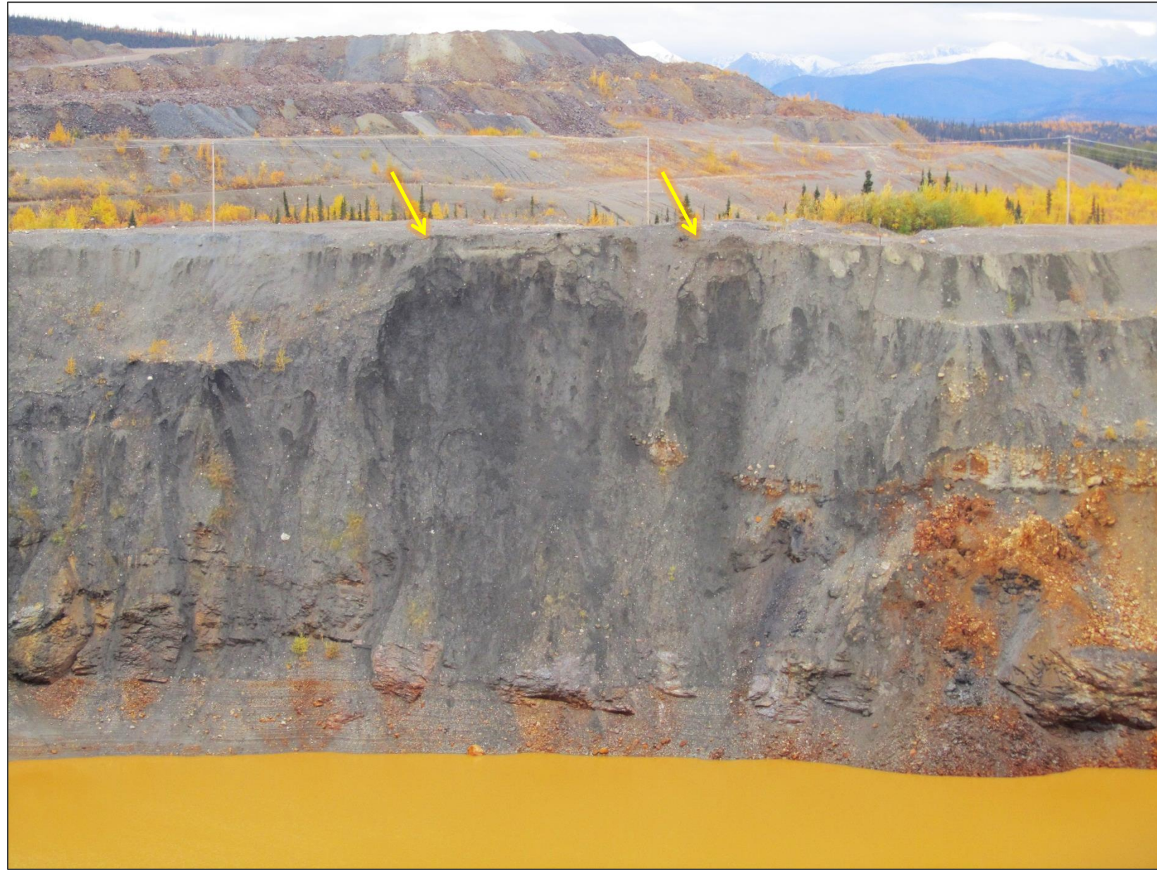
NORTH SIDE OF WEST WALL, VIEW LOOKING WEST ARROWS INDICATE RECENTLY SLUMPED AREAS
