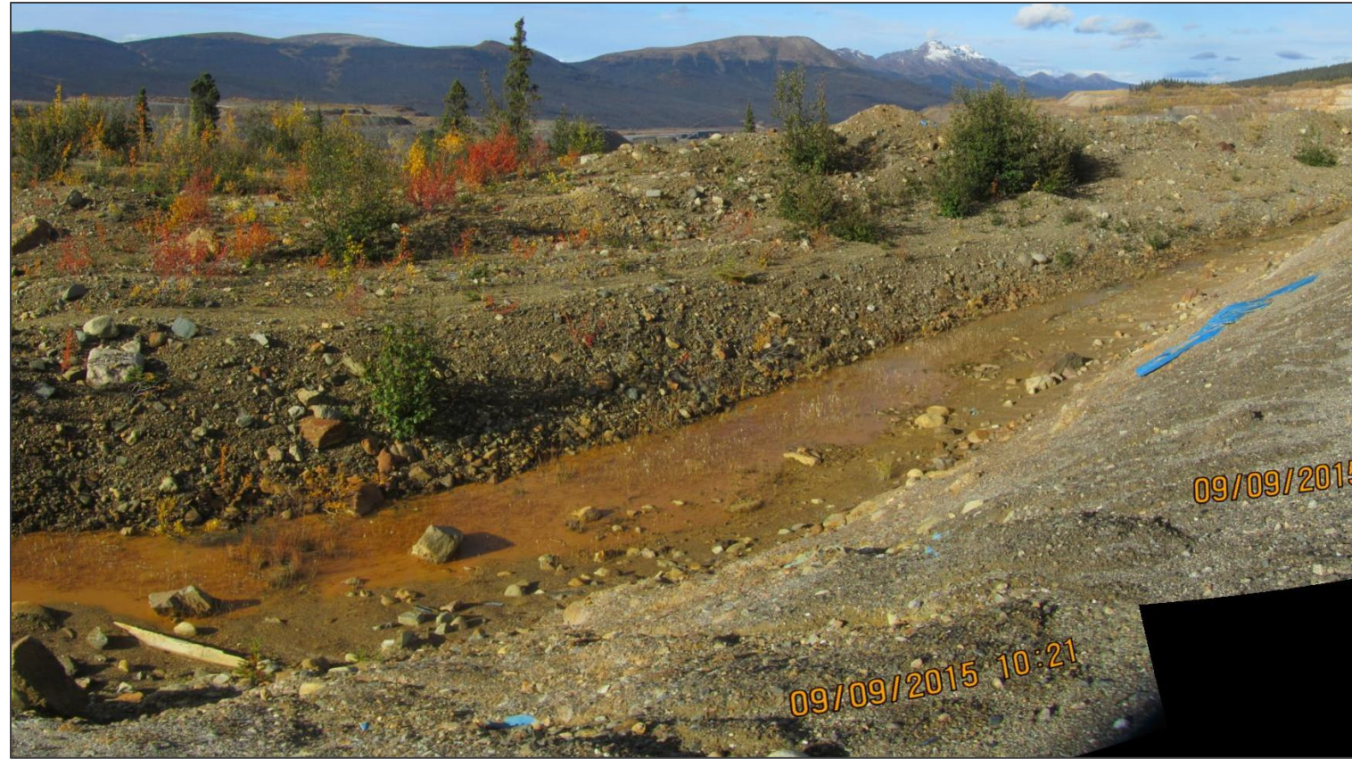
BERM AT CREST OF EAST WALL, ON WEST SIDE OF ROAD, VIEW LOOKING NORTHWEST
