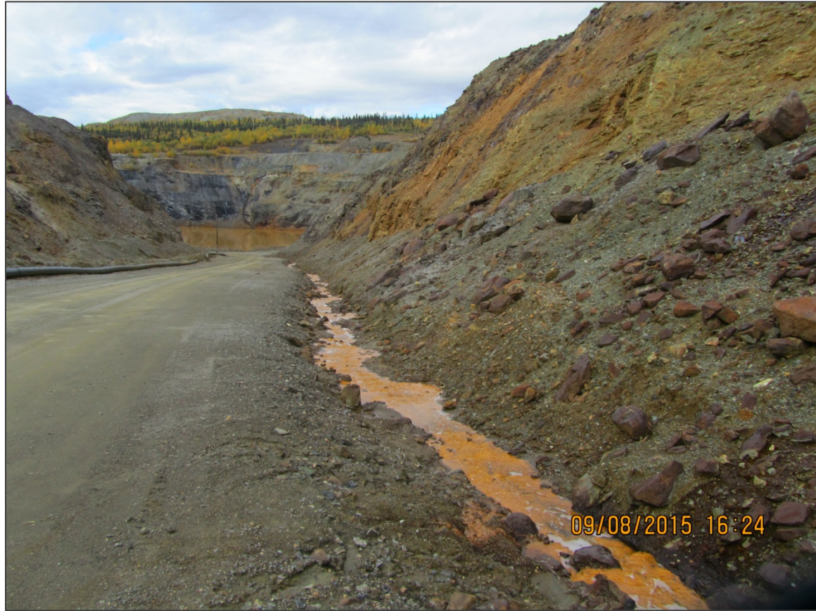
DITCH SERVES AS ROCKFALL CATCHMENT ON EAST SIDE OF ACCESS ROAD, VIEW LOOKING NORTH
