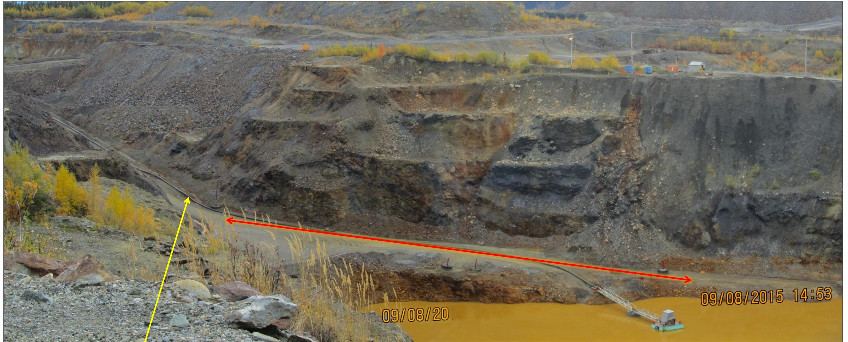
IN-PIT ACCESS ROAD, SOUTH SIDE OF PIT, VIEW LOOKING SOUTHWEST
