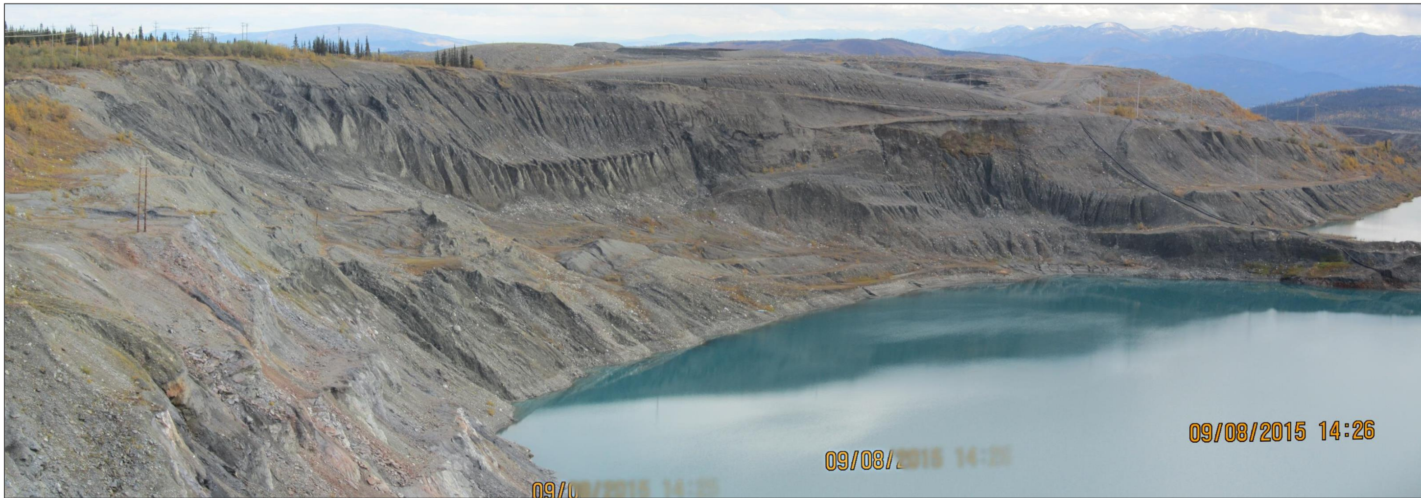
INSTABILITY ZONE, VIEW LOOKING SOUTHEAST
