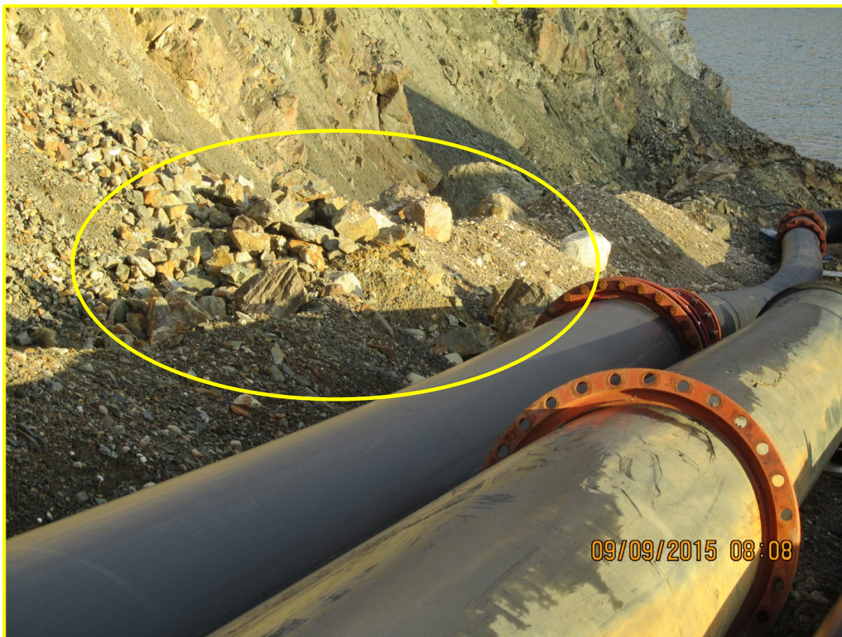
REMOVE MATERIAL BEHIND BERM TO RE-ESTABLISH ROCKFALL CATCHMENT
