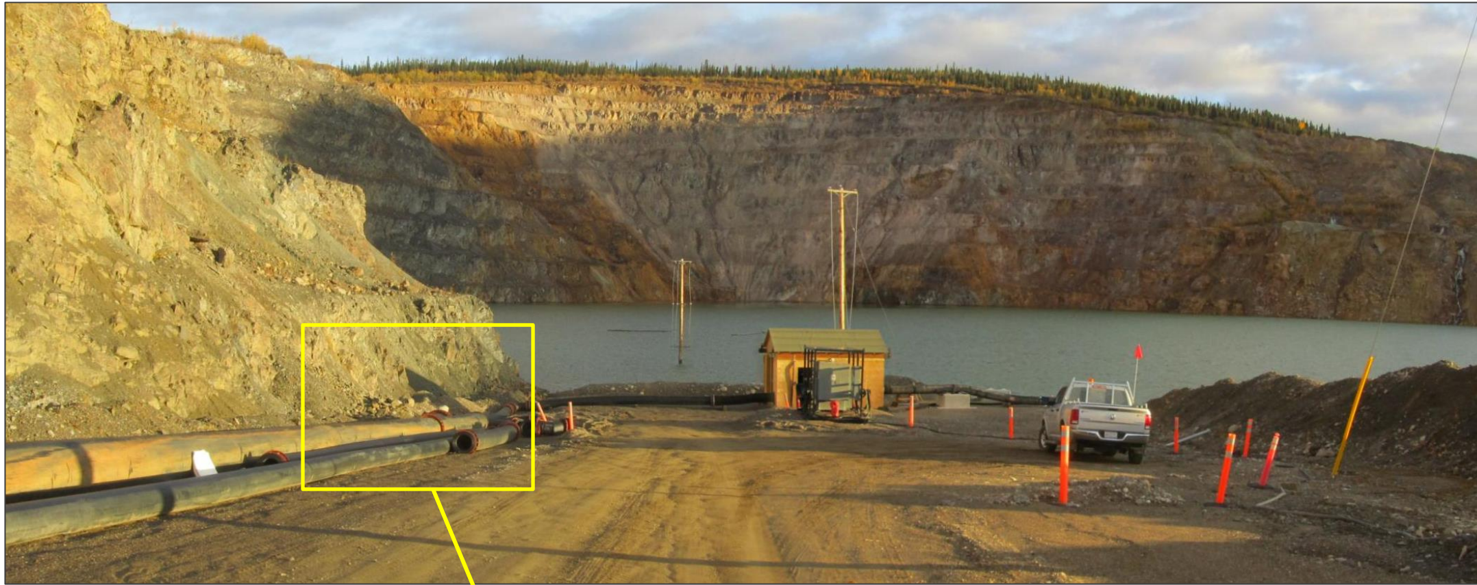
WEST ACCESS ROAD, WEST SIDE OF PIT, VIEW LOOKING NORTH
