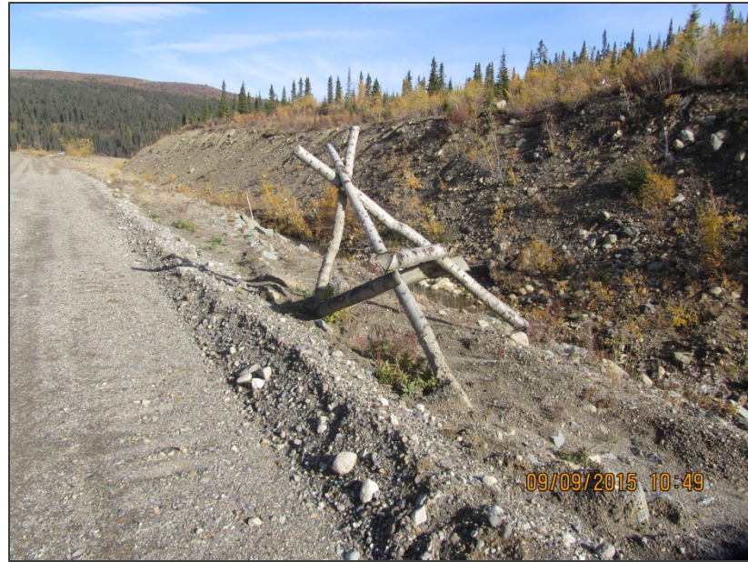
PIN 13908 – STRUCTURE STILL STANDING, BUT COULD NOT FIND PIN
