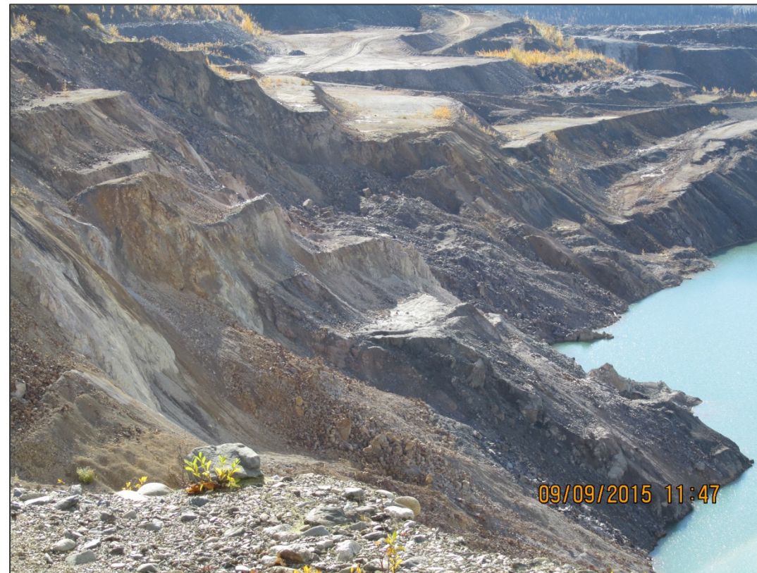
RAVELING ON BENCHES
