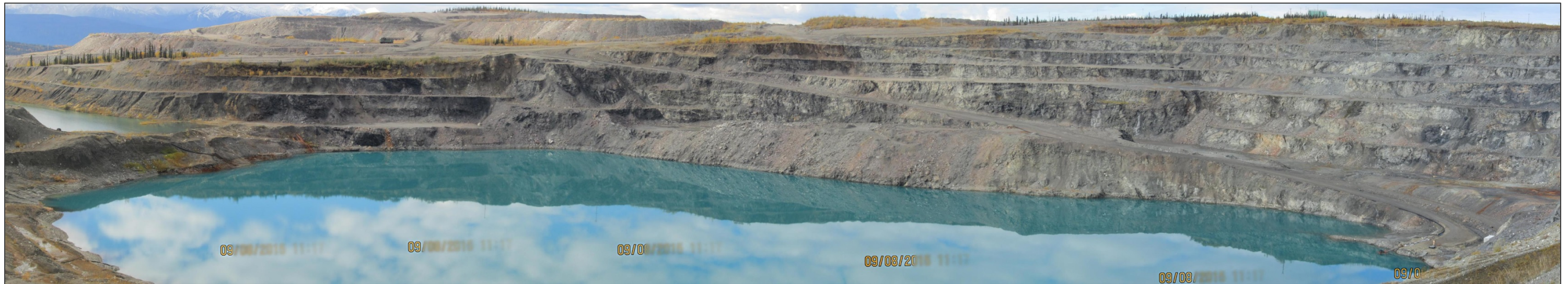
WEST AND SOUTH WALL
