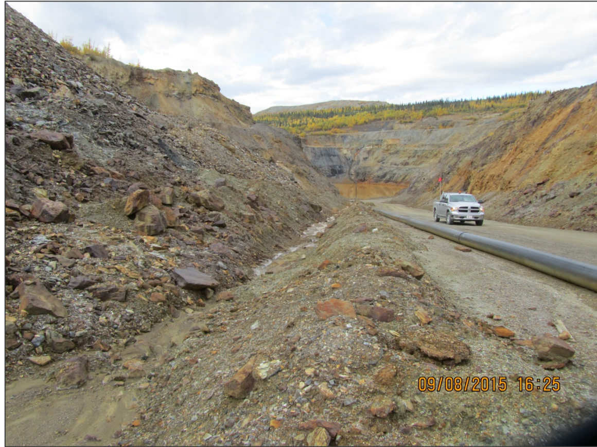
BERM ON UPPER PART OF ACCESS ROAD, WEST SIDE, VIEW LOOKING NORTH
