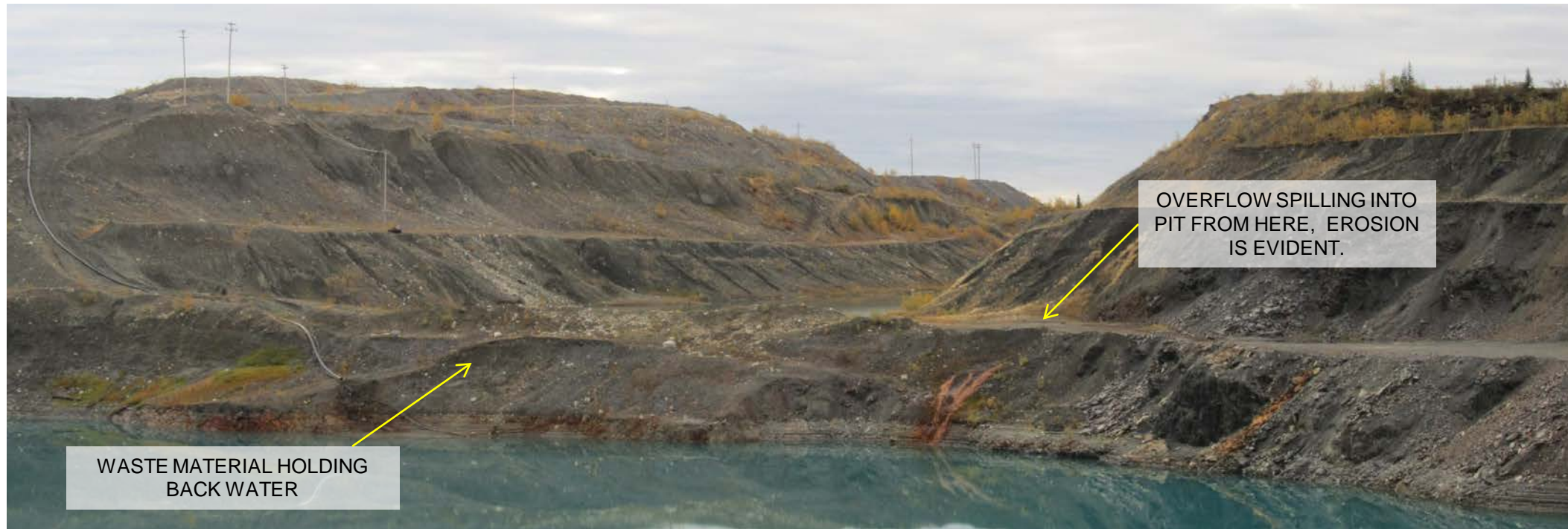
GRUM SLOT CUT, VIEW LOOKING SOUTH
