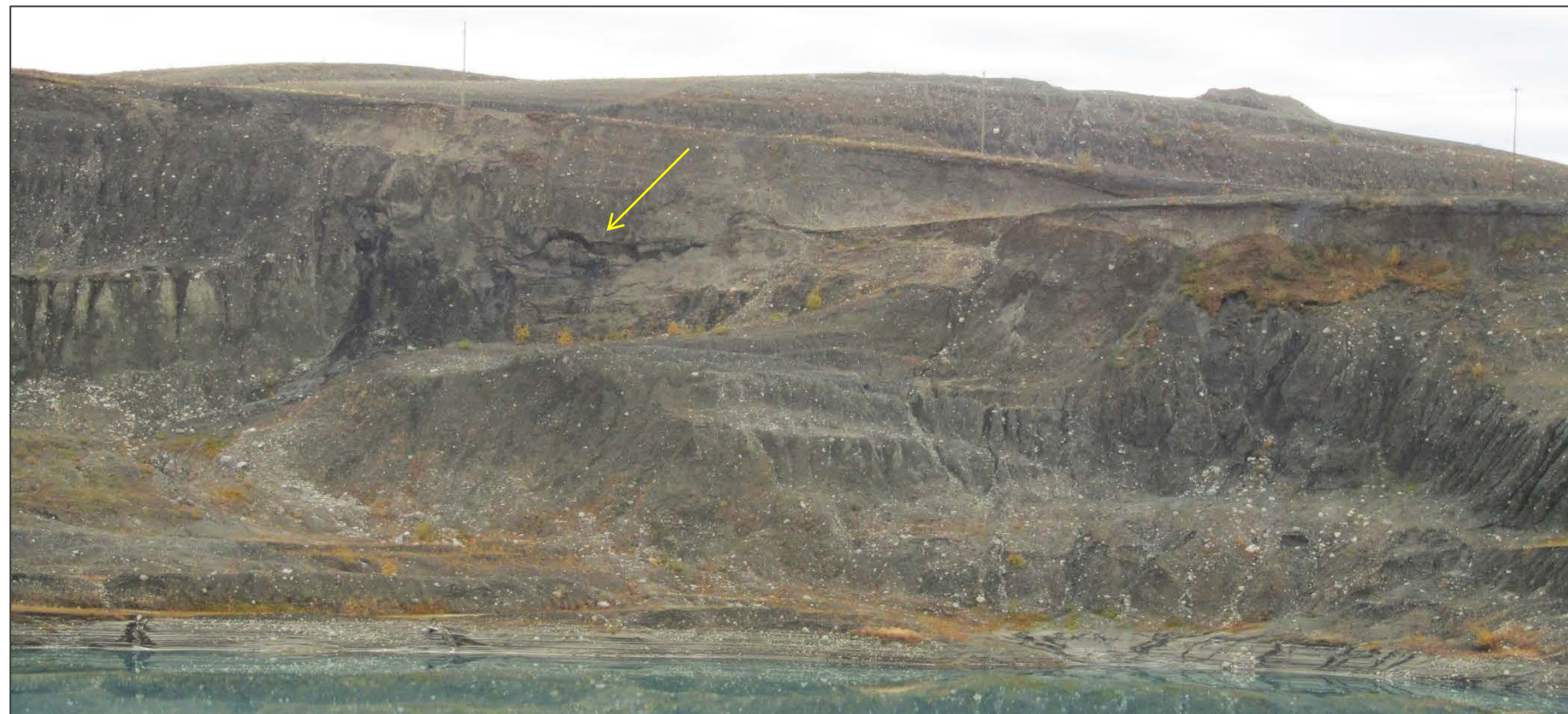
2015 PHOTOGRAPH OF INSTABILITY ZONE, VIEW LOOKING EAST
