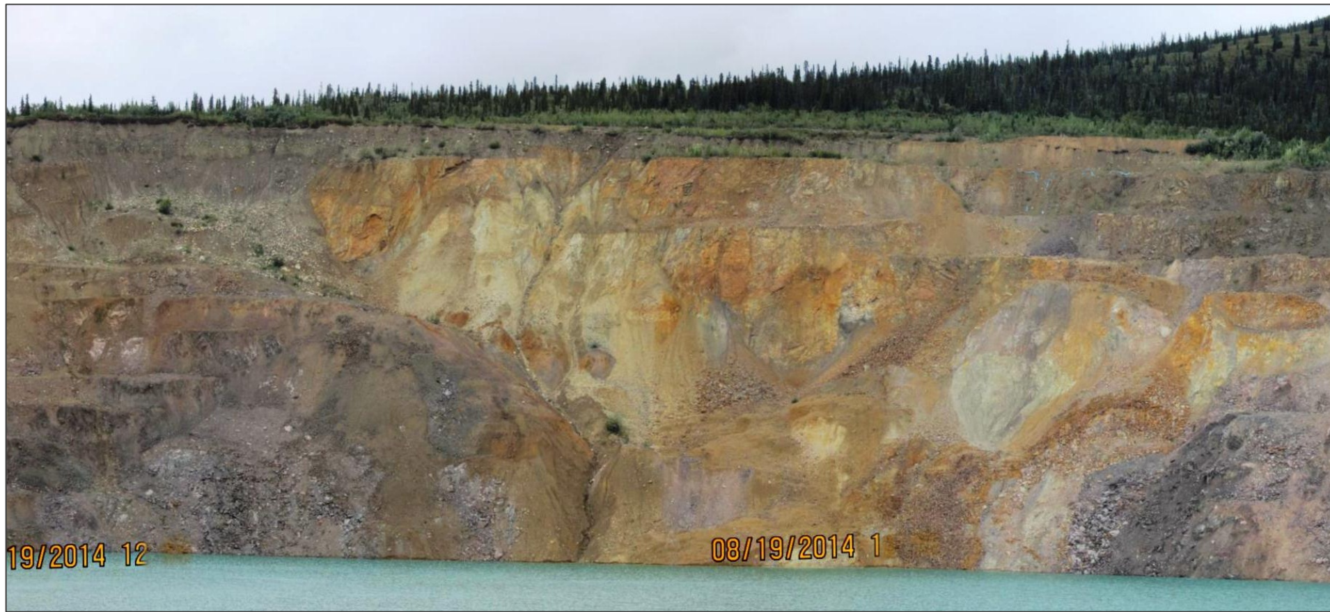
2014 PHOTOGRAPH OF NORTH INSTABILITY ZONE, VIEW LOOKING EAST
