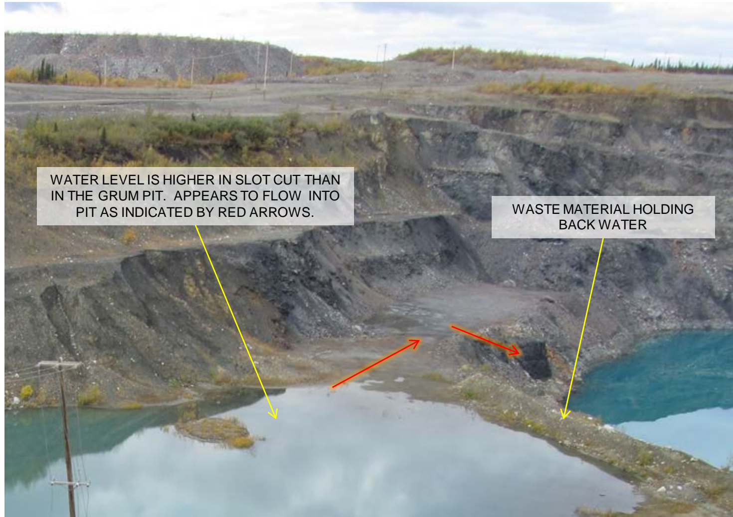
GRUM SLOT CUT, VIEW LOOKING WEST
