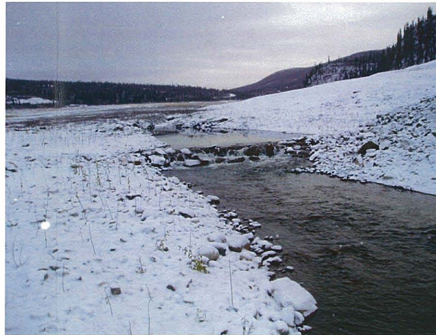
September: Shows the first water flowing over the inlet structure during normal flow period.
