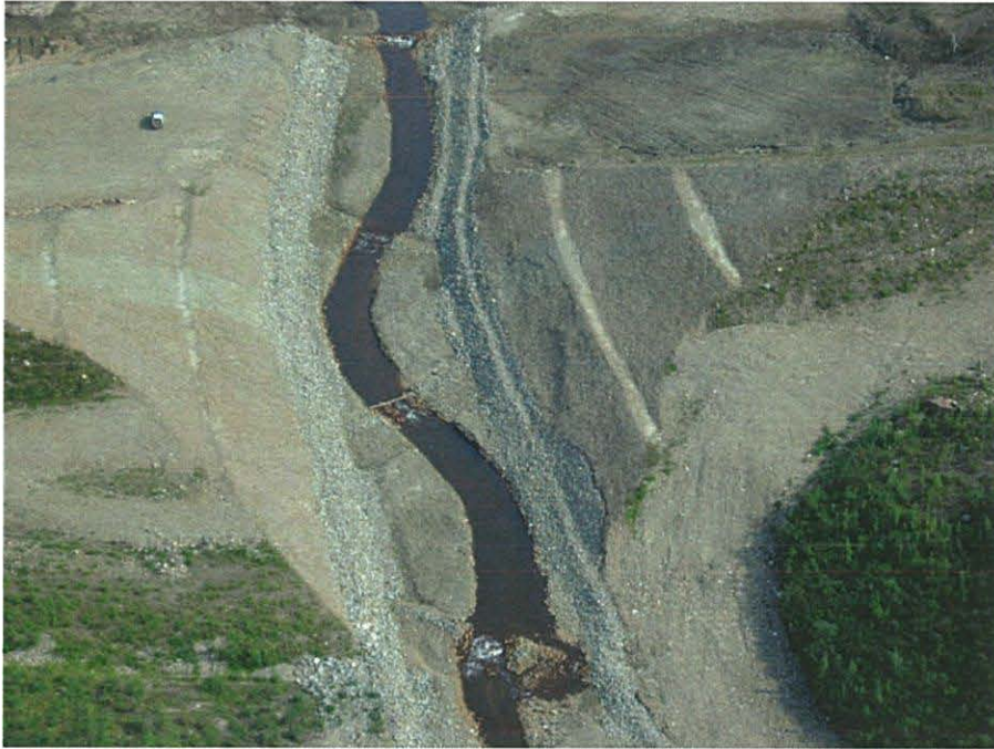
Photo 21: Aerial view of the constructed channel within the breach.
