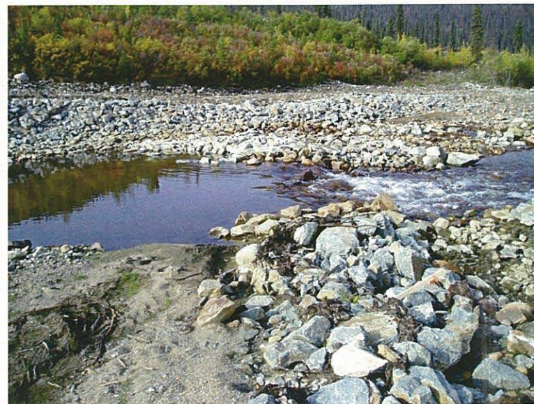
September: Shows a view of the left side of Riffle 3 following the repairs. Note the riprap placed to match the riprap elevation elsewhere.
