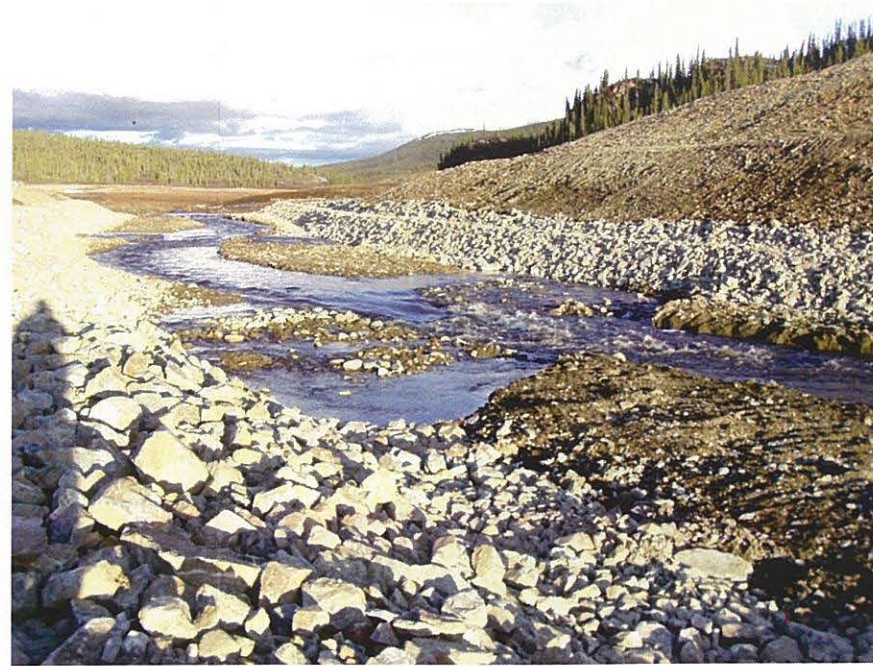
May: Shows water flowing over Riffle 2 during freshet period. Again, some erosion of the soil above the rock of the riffle has been eroded.
