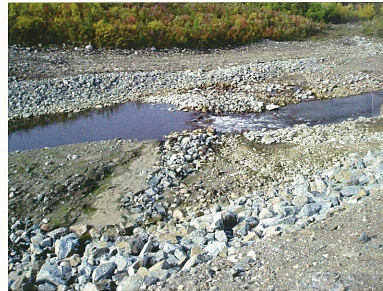
September: Shows an overview of the repaired Riffle 3. The newly placed riprap on the left side of the floodplain is high enough that the majority of the water is flowing in the centre of the channel.
