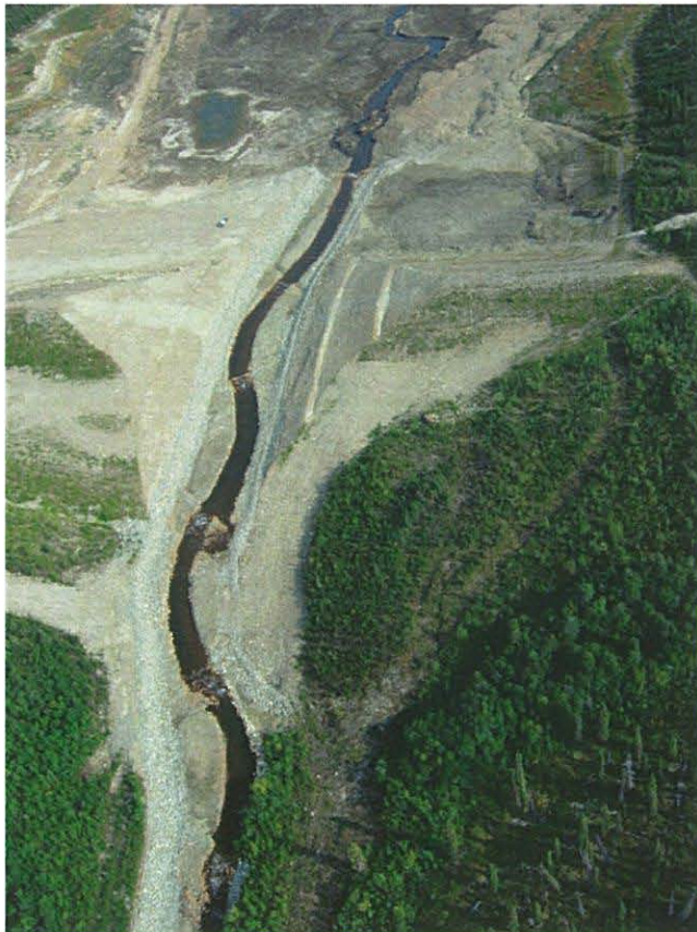
Photo 20: Aerial view of the constructed channel through the breach.
