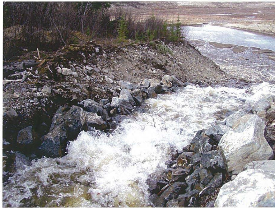
May: Shows a view, looking downstream at the water flowing across the repair portion of K8 creek.
