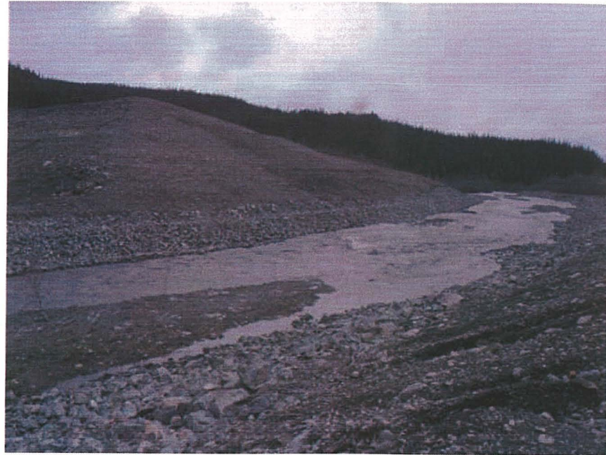
May: Flow in the channel and flood plain during the peak freshet flow of 2005.
