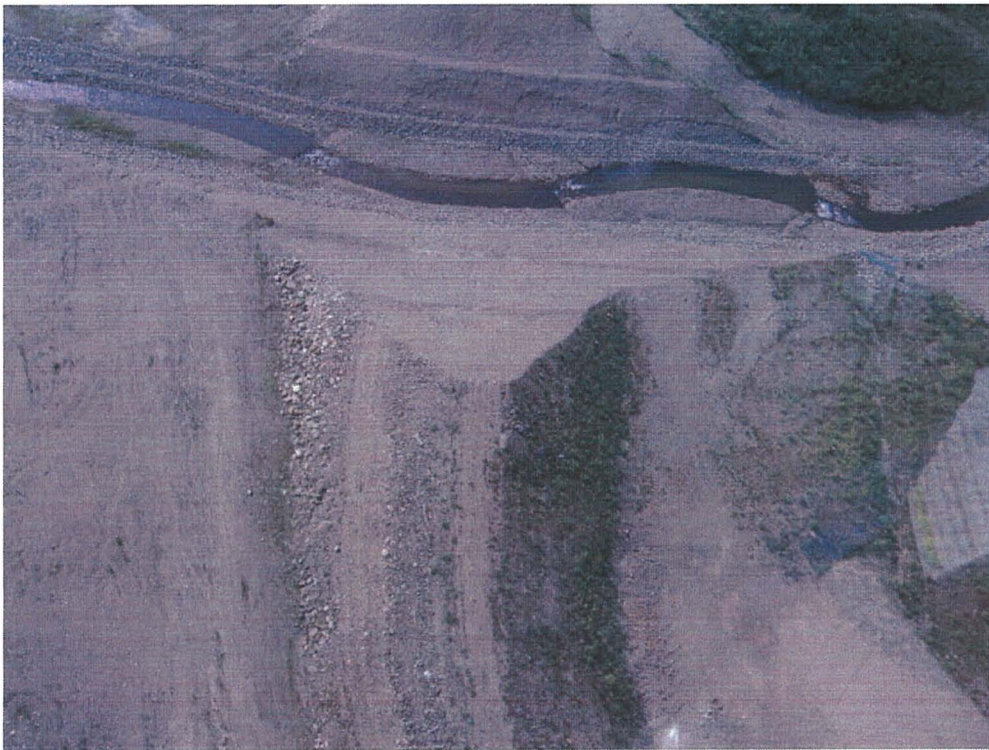
Photo #12: The constructed channel within the breach, August, 2005
