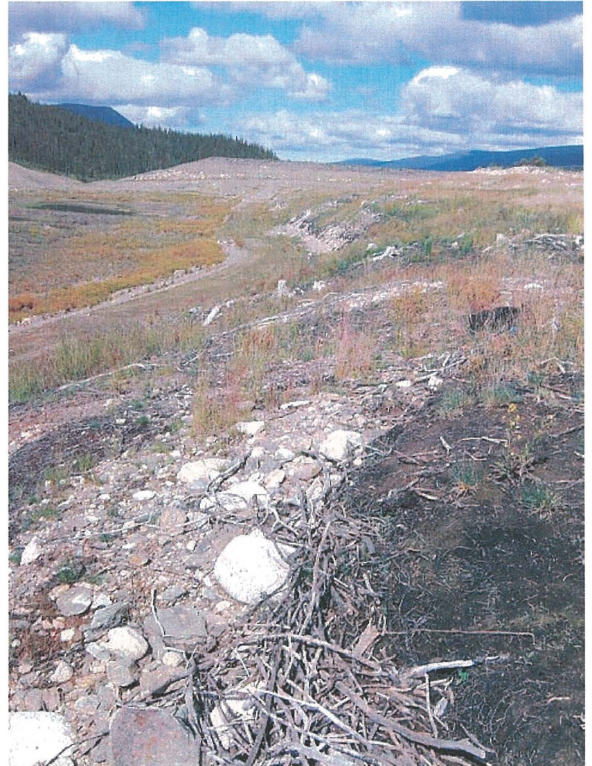
Photo #4 : Facing west towards breached dam through Phase II, Phase I in upper right.
