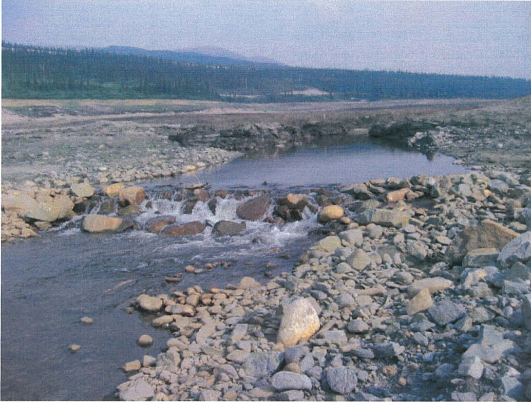
Photo #15: Inlet structure at the upstream margin of the newly created channel and start of Reach #4, August 2004.
