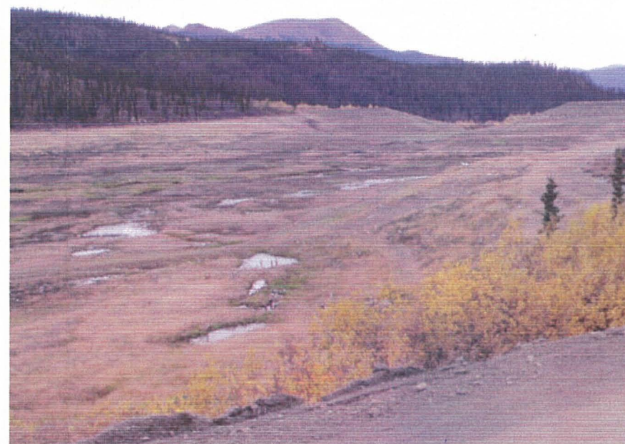
September: A general view of the former reservoir bottom and the upstream side of the Fresh Water Supply Dam breach.
