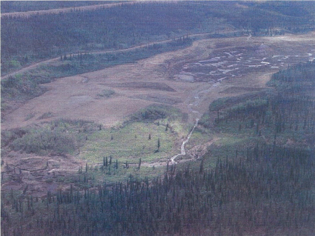
Photo # 14: The dam has been breached and dewatering has occurred. Summer 2004.
