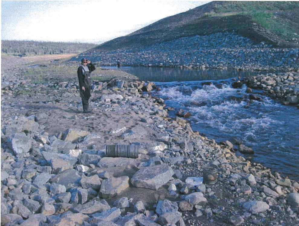
Photo #19: The downstream end of the breach, August 2005.
