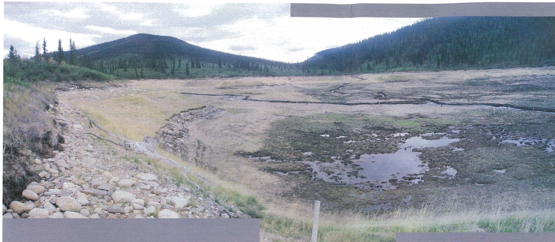
May: Shows a panoramic showing the condition of the vegetation and the two tributaries at the upstream end of the reservoir. The early phases of re-vegetation performed in the upper part of the former reservoir appears to be performing better than the later (lower) re-vegetation efforts.
