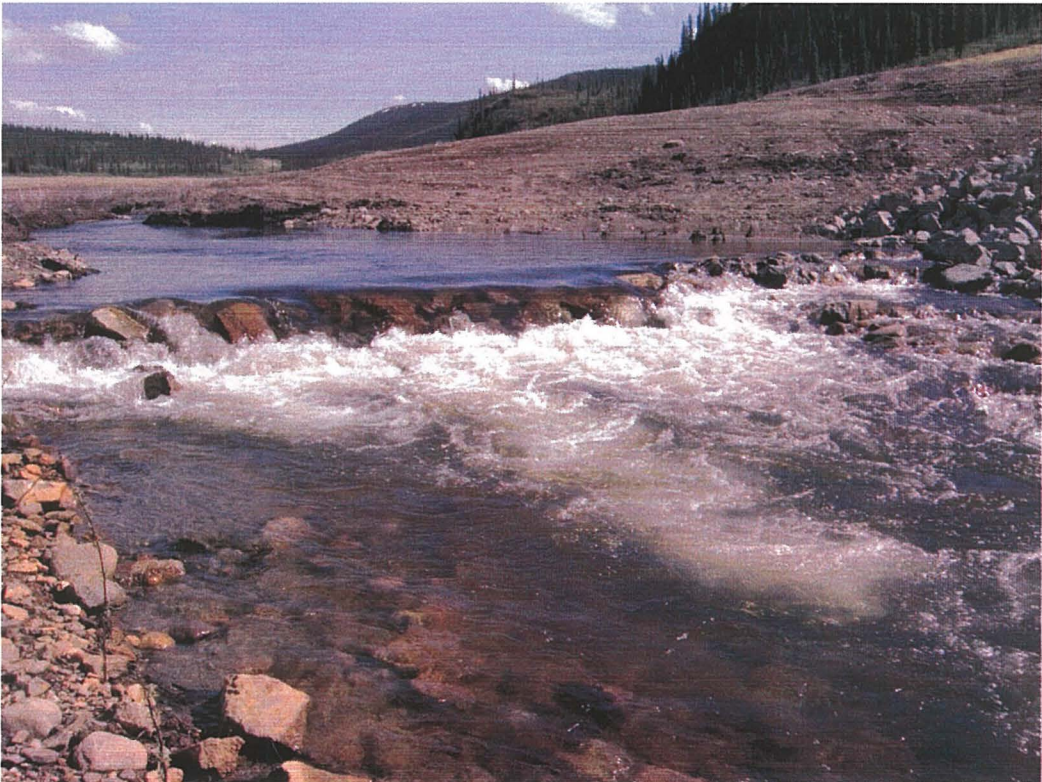
Photo #14: The inlet structure at the upstream margin of the breach during June flows, 2005.
