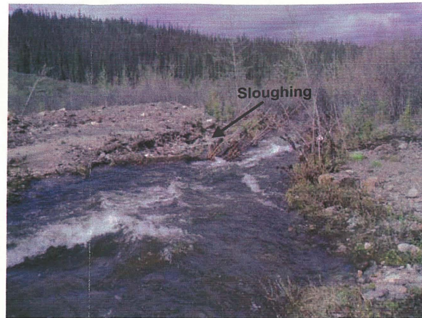
May: Erosion on left bank immediately downstream of the limit of the 2003 construction.
