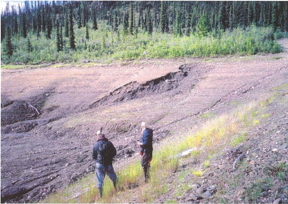
Photo #5: Eroded gully formed on south west side of reservoir.
