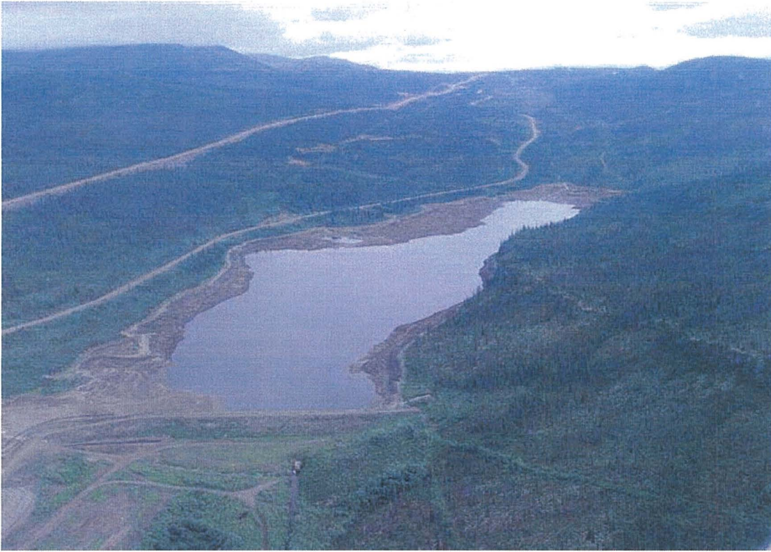
Photo # 13: Freshwater Reservoir prior to breaching. Draw down has occurred to at least the Phase I level. Summer 2003.
