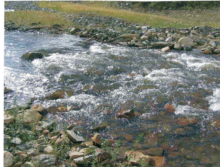
June 2007: Riffle 4 is shown here. This riffle has experienced some riprap movement which has lengthened the riffle and made it less distinct. No remedial action is recommended.
