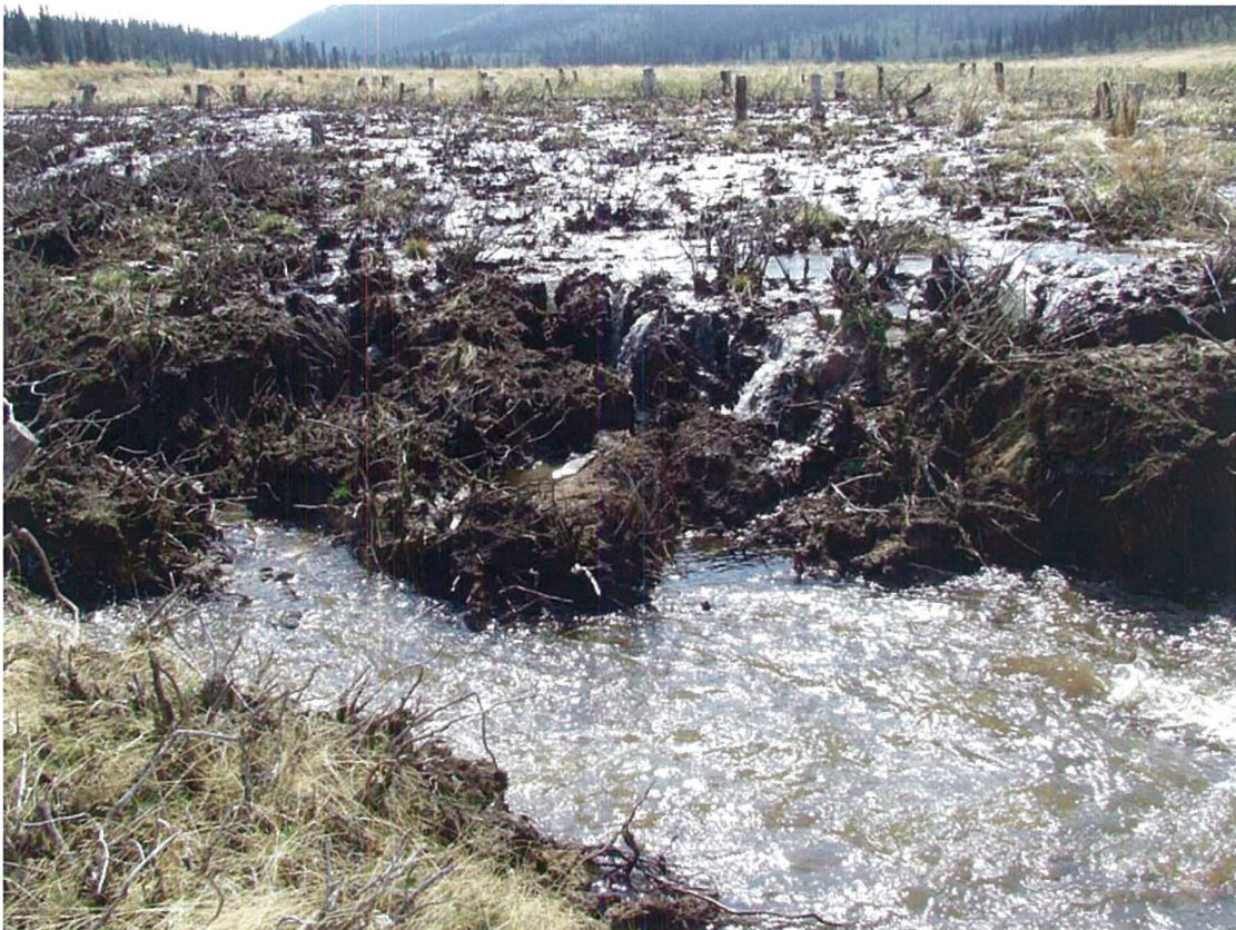
Photo #4: Retrogressive erosion of the North Tributary over and through loose soils and silt of the valley floor. June 5, 2007.
