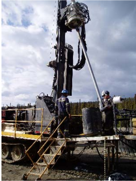
Photograph 1. Sonic drill rig extracting the core at BH05-02
