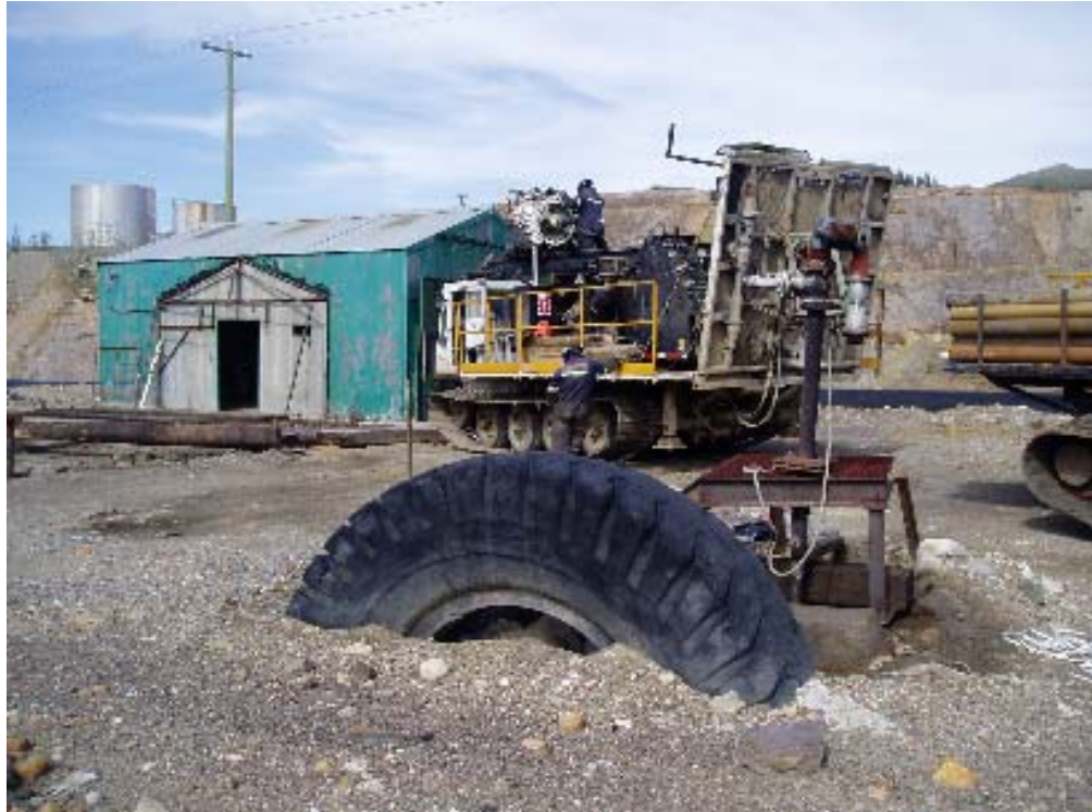
Photograph 3. Setting up to drill at BH05-8 at the Faro Lube Shack
