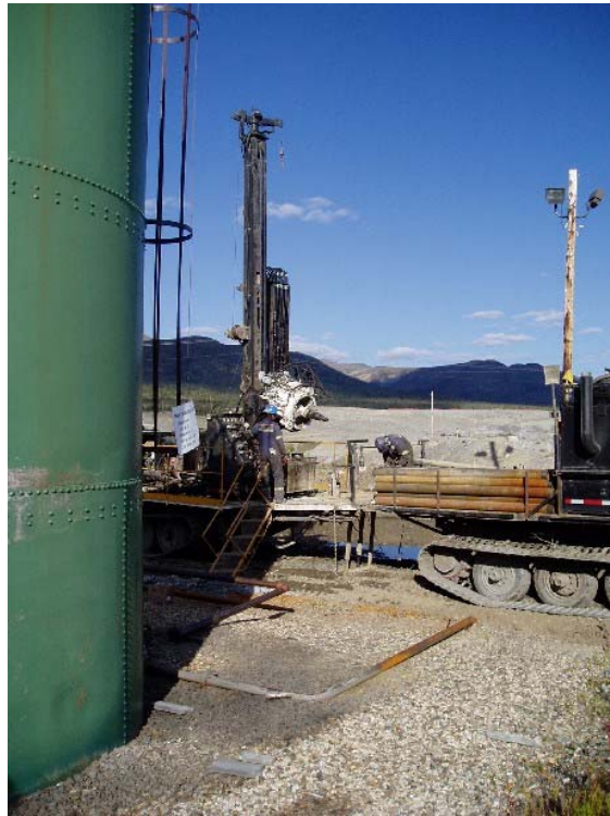
Photograph 6. Drilling BH05-20 inside the bermed Vangorda Tank Farm
