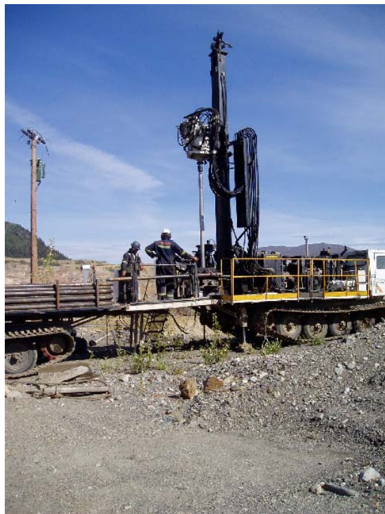
Photograph 4. Drilling BH05-11 at the Faro Tank Farm
