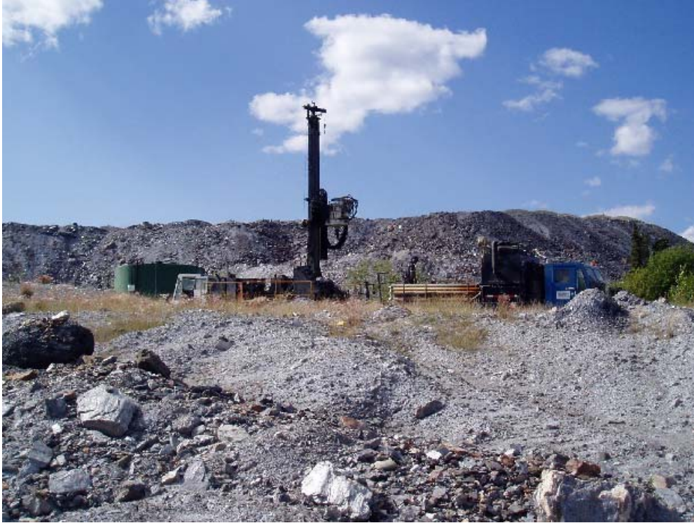
Photograph 5. Drilling BH05-19 adjacent to the Vangorda Tank Farm
