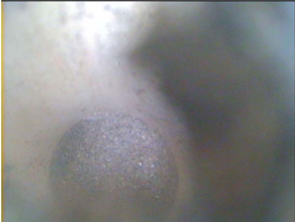
Photograph 1. X24B-96 – Sand heave at 3.69 m (photo from July 2005)
