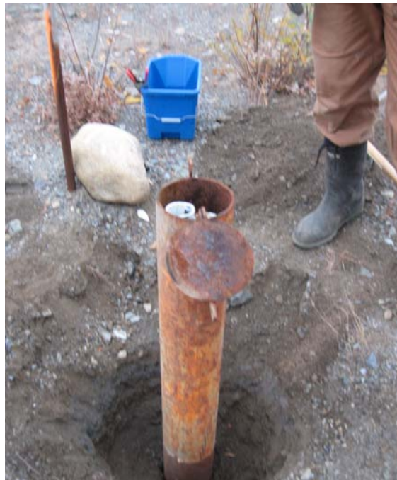
Photograph 16. P01-01 A,B during rehabilitation, well stick-up was shortened, protective steel casing was installed, ground was leveled. (Sept. 2006). New stick-ups from ground surface are : P01-01A = 0.74 m , P01-01B = 0.65 m)
