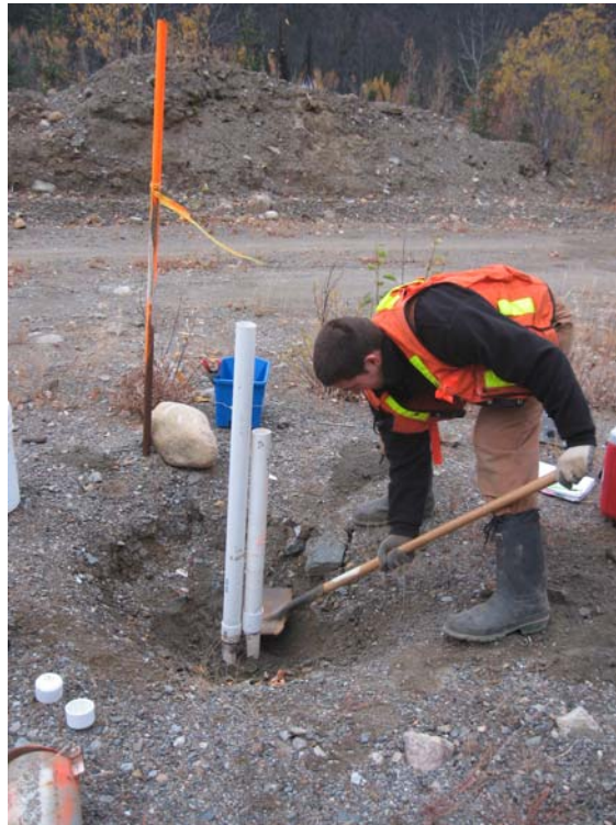
Photograph 15. Well P01-01 A,B during rehabilitation. 0.30 m was cut from stickup at P01-01B.
