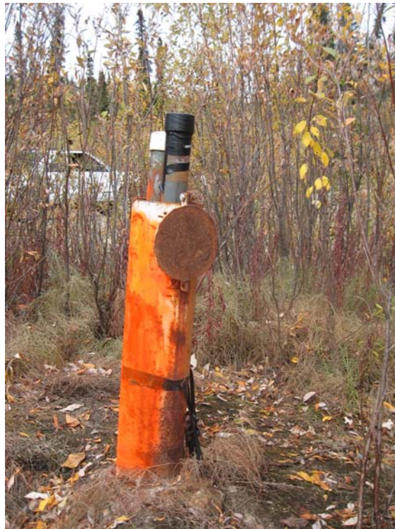
Photograph 2. Protective casing and nested wells at P96-9A/B. Wells and steel casing are tilted.
