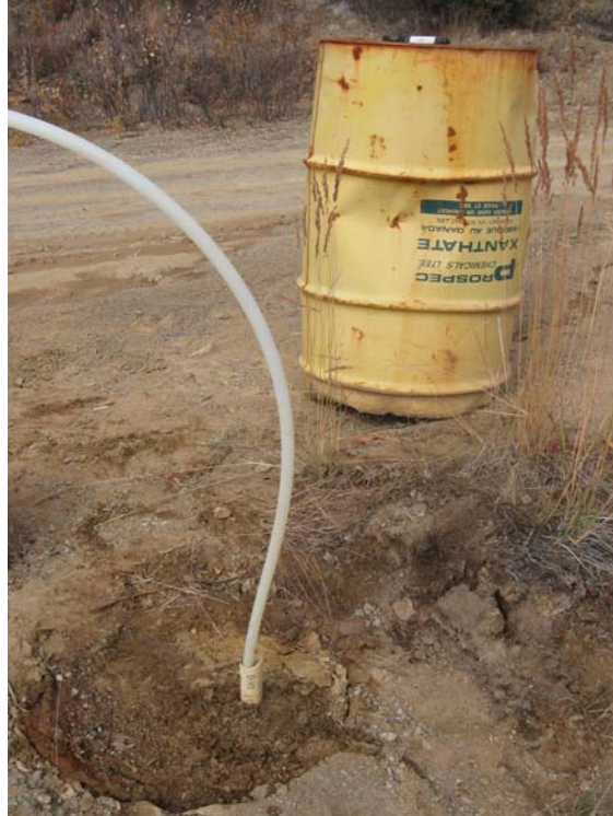
Photograph 5. Well BH11 broken at ground surface (September, 2006)
