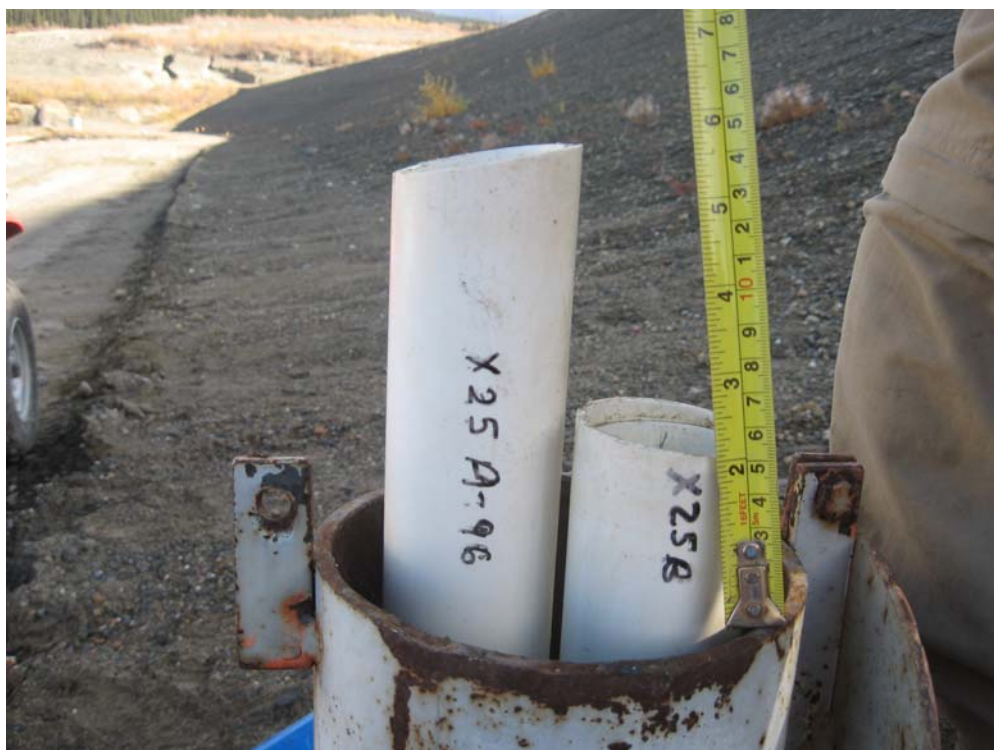
Photograph 1. Wells X25-96 prior to shortening the stickup (Sept. 21, 2006).
