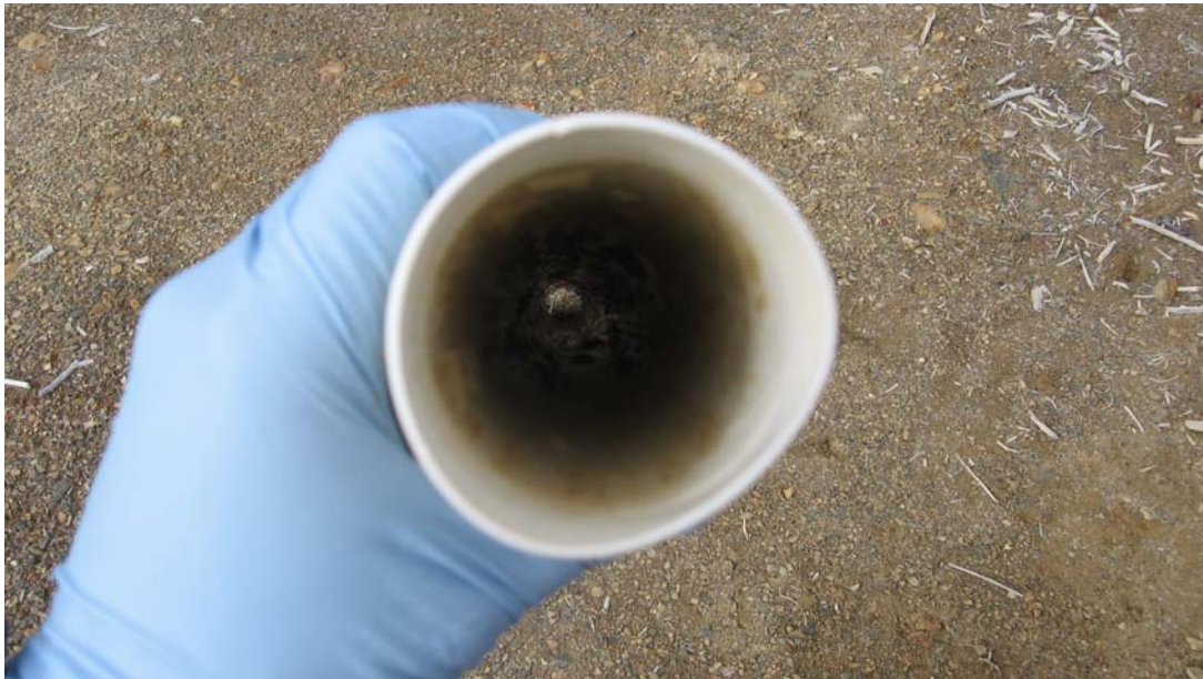
Photograph 7. Top section of well casing at BH7D after it was removed from ground. Joint is no longer circular and appears to have been strained
