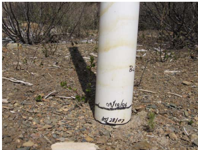
Photograph 1. Evidence of frost-jacking at BH7S over winter 2006-2007.
