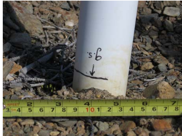
Photograph 3. Ground surface (g.s.) representing September 2006 ground elevation at BH6.
