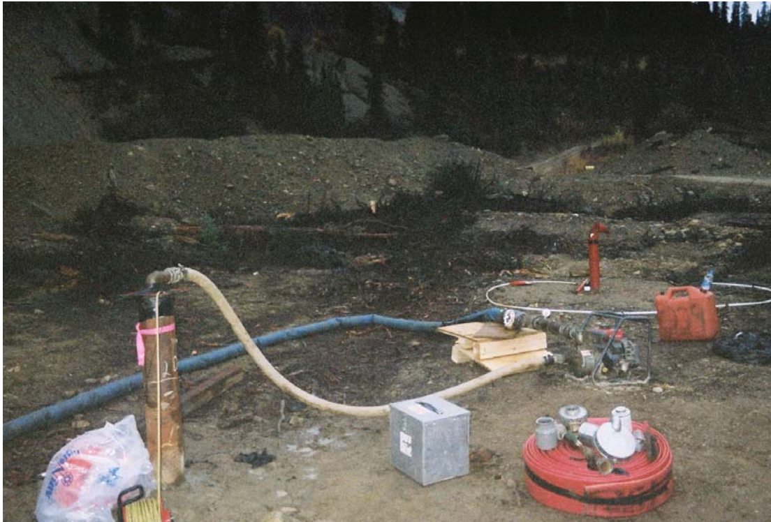
Photo 3: Setup for 24 hour Pumping Test at PW-3
