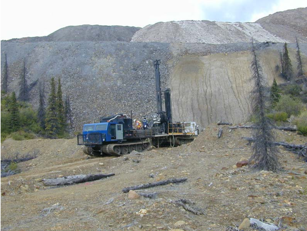
Photo 1: Sonic Drill Rig set up in Zone 2 Outwash Area (at BH05-01)
