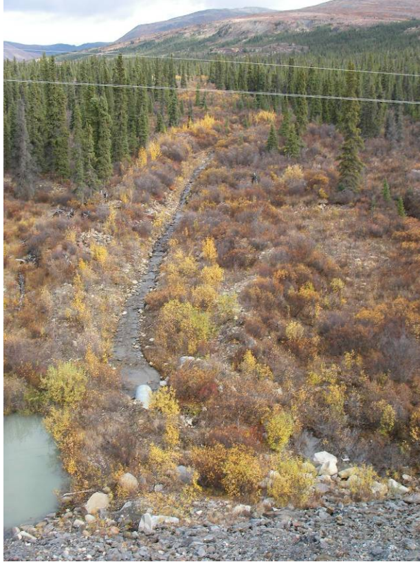
Photo 25: Area upstream of inlet to HR-5 (Sept. 16, 2007).
