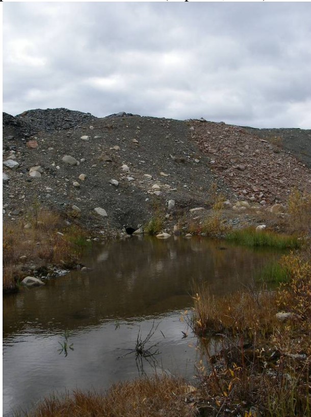
Photo 34: View of partially buried corrugated pipe at inlet to HR-7 (Sept. 16, 2007).
