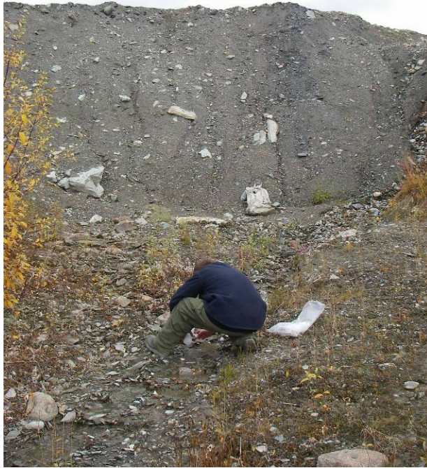
Photo 31: Diffuse drainage at downstream toe area of HR-6 (July 7, 2008).
