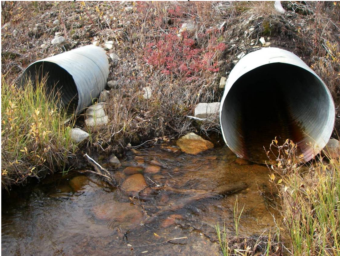
Photo 18: Corrugated pipes at inlet of HR-3 (Sept. 16, 2007).
