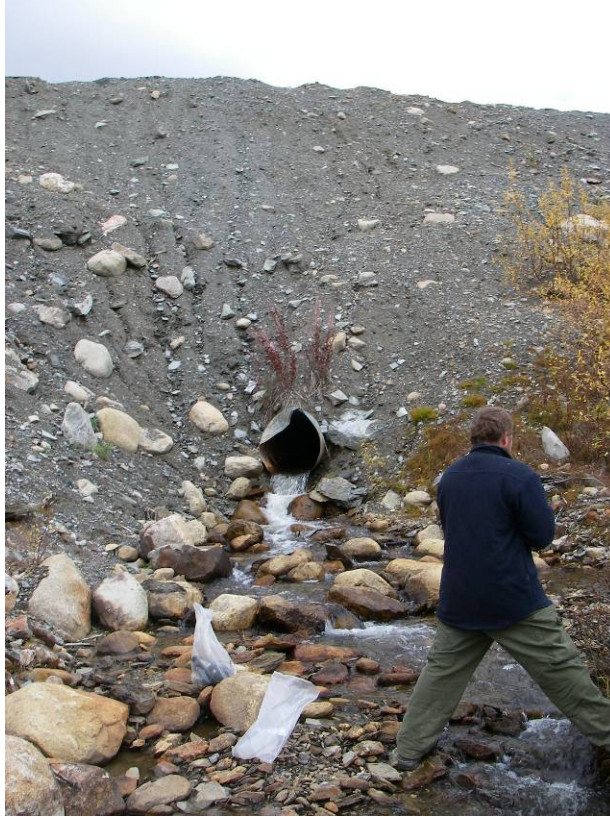
Photo 35: Discharge from corrugated pipe at outlet of HR-7 (Sept. 16, 2007).
