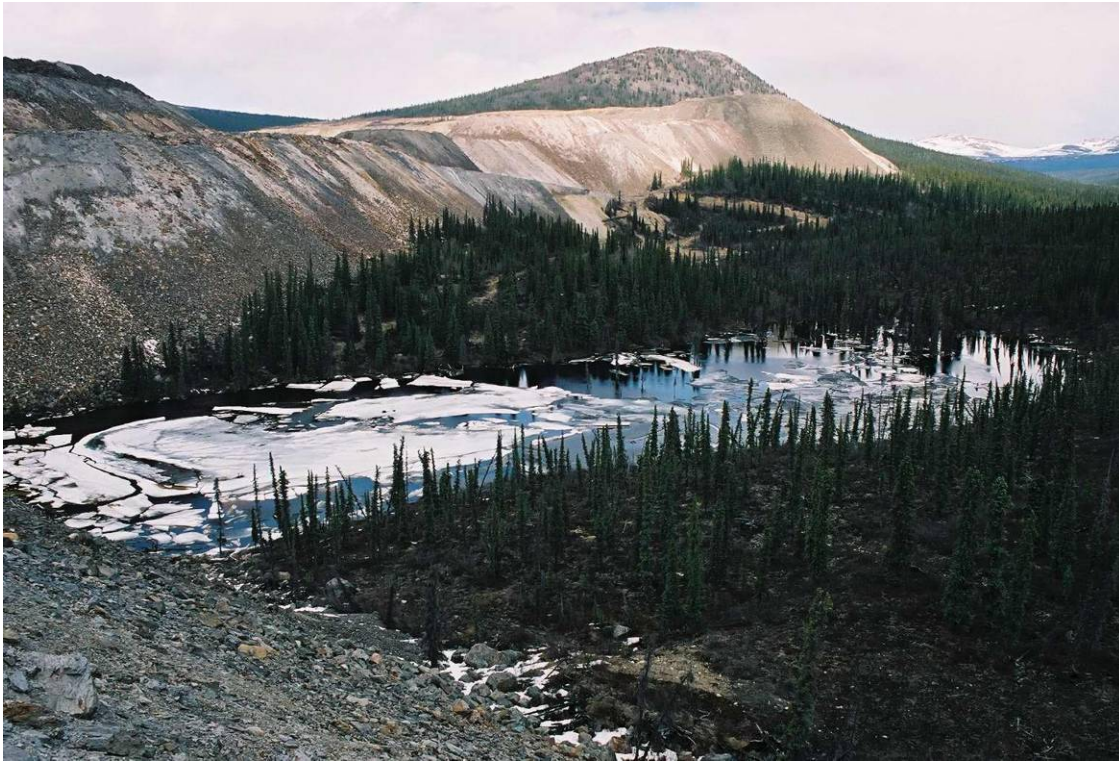
Photo 1: RC drainage, showing water ponded upstream of the Rock Drain (May 24, 2004).
