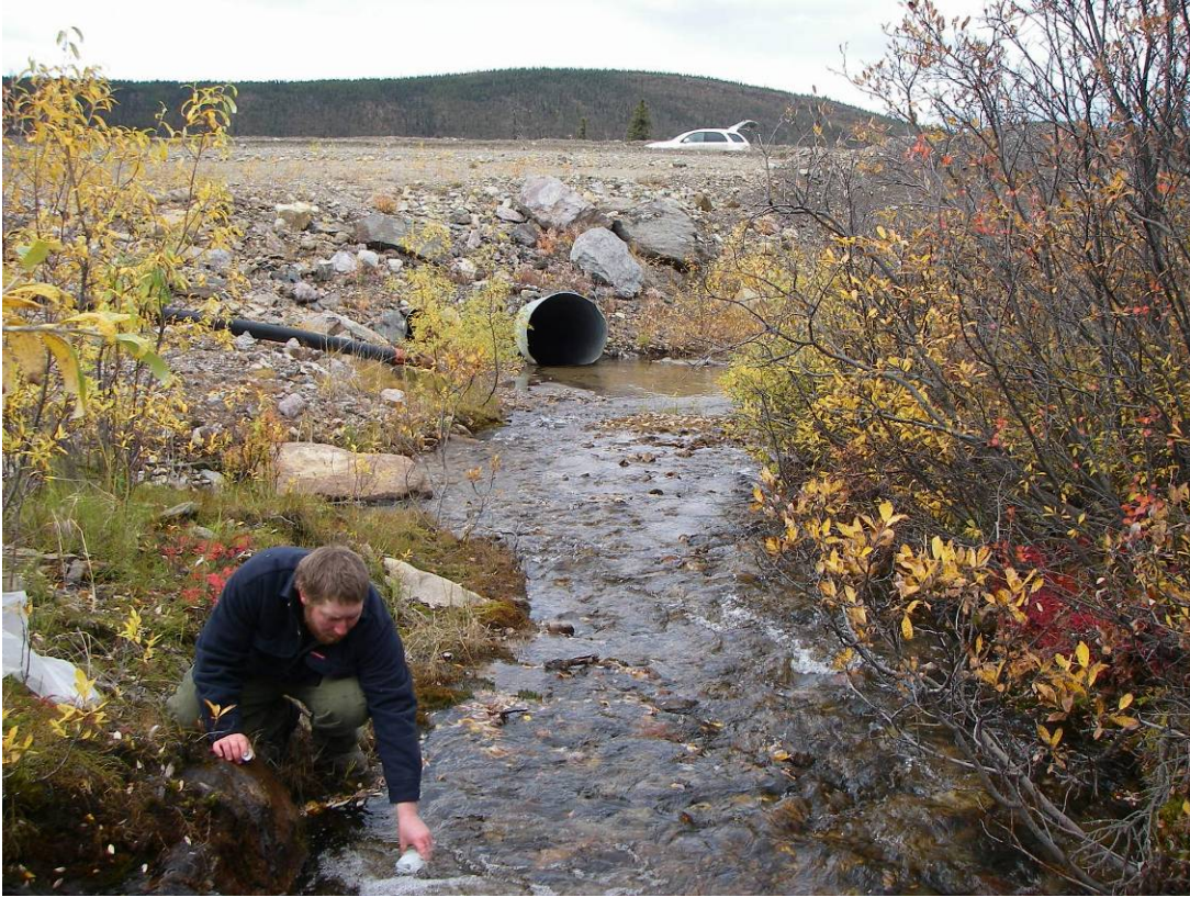
Photo 13: Looking towards two corrugated pipes at inlet of HR-2 (Sept. 16, 2007).
