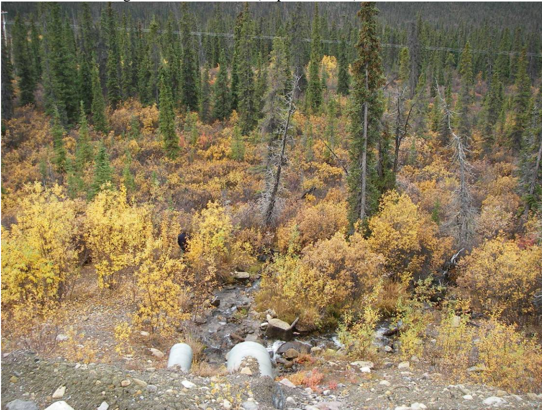
Photo 16: View away from Haul Road on downstream side of HR-2 (Sept. 16, 2007).
