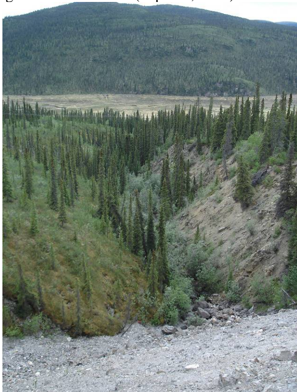
Photo 40: View away from Haul Road at downstream side of HR-8 (Sept. 16, 2007).
