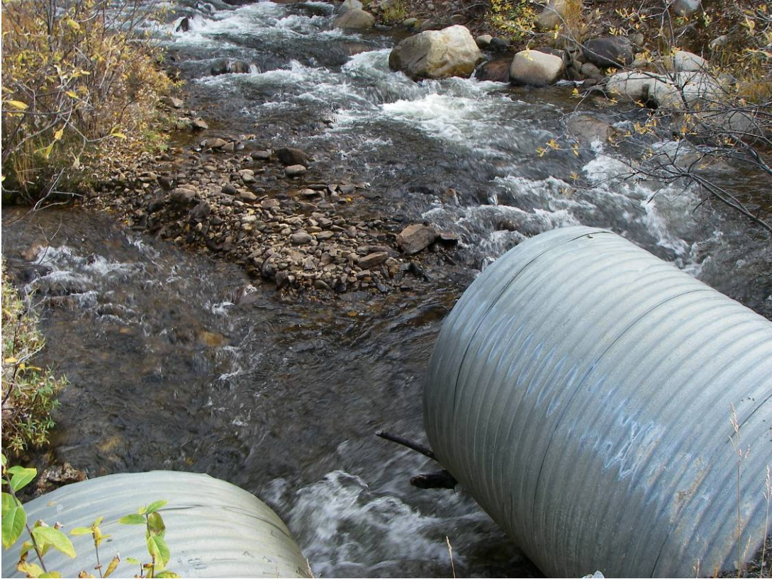
Photo 21: Area upstream of inlet to HR-4 (Sept. 16, 2007).
