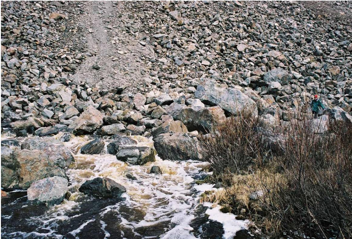
Photo 3: RC drainage showing water discharging from the Rock Drain (May 24, 2004).
