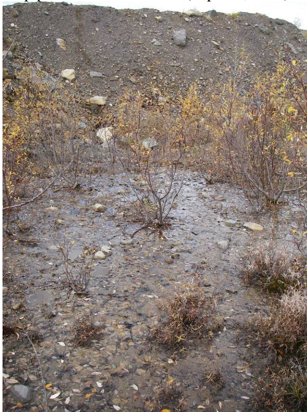
Photo 10: Diffuse drainage at downstream toe area of HR-1 (July 7, 2008).
