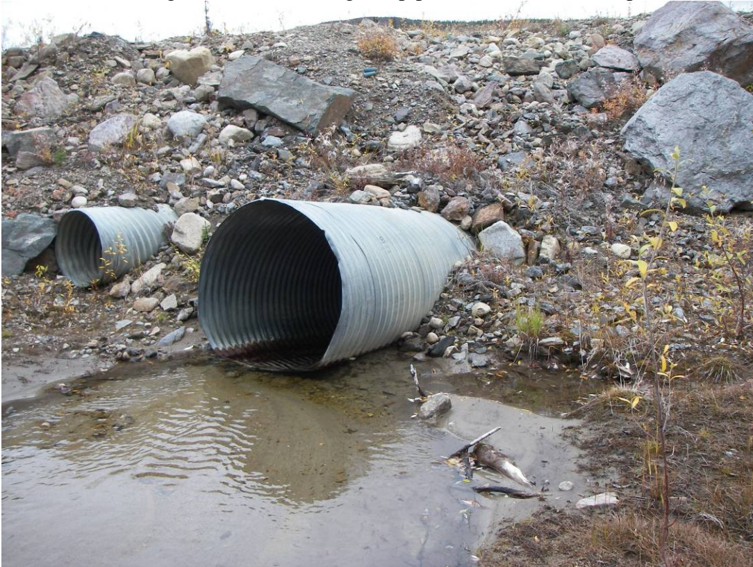
Photo 14: Corrugated pipes at inlet of HR-2 (Sept. 16, 2007).
