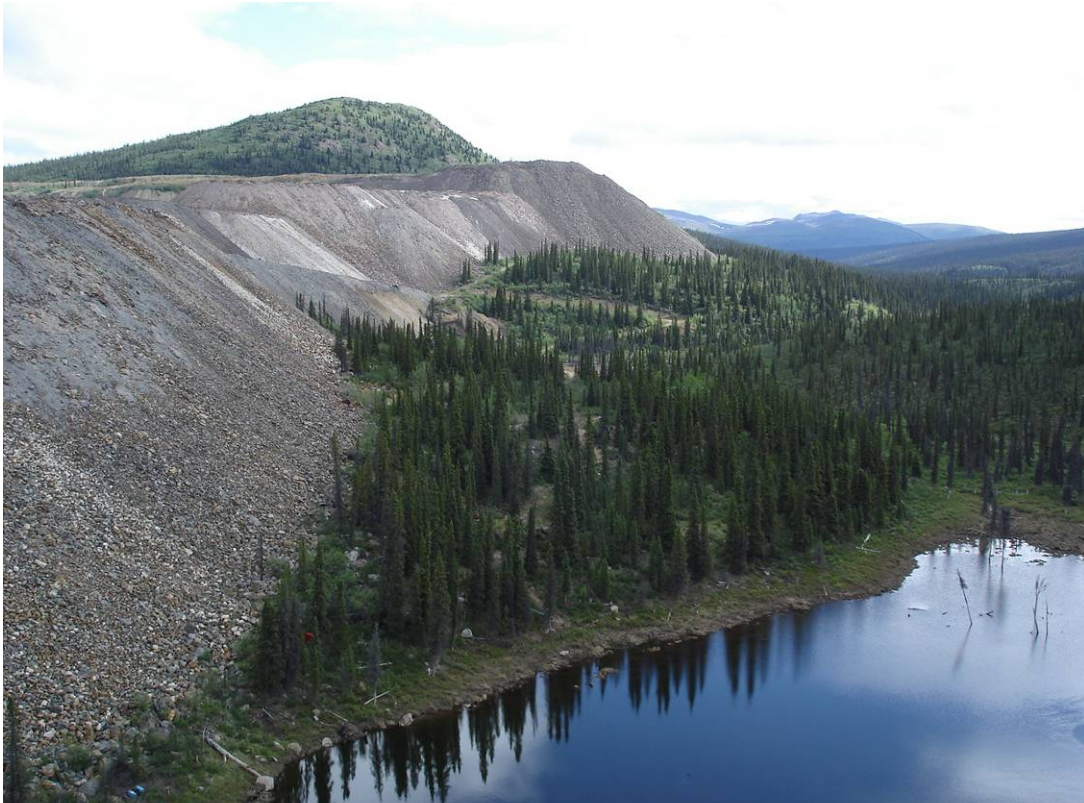
Photo 5: Water ponded upstream of the Rock Drain (June 22, 2006).
