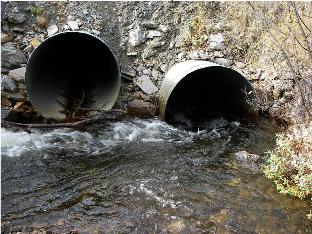
Photo 22: Corrugated pipes at inlet to HR-4 (Sept. 16, 2007).
