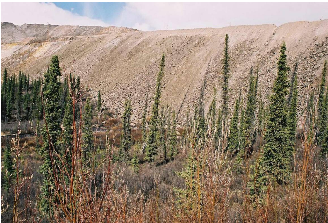
Photo 2: RC drainage area showing downstream face of the Haul Road (May 24, 2004).
