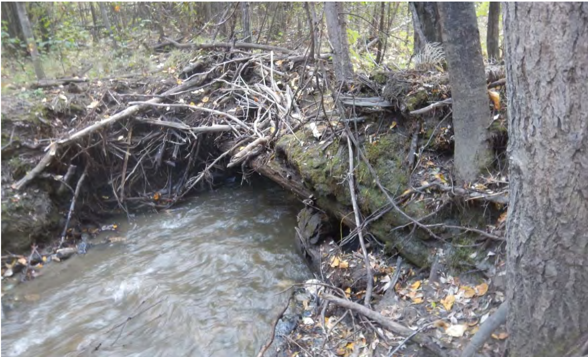
Eagle Creek Photo 2: An old bridge crossing that parallels the existing road still spans Eagle Creek.
