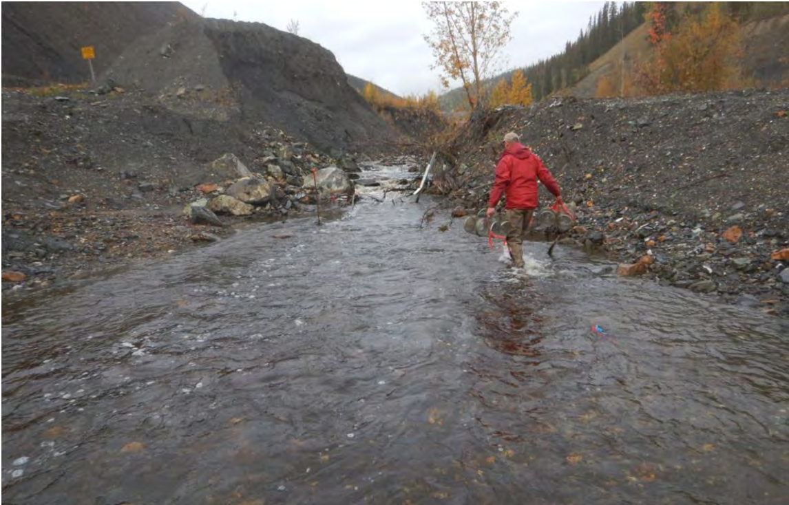
CCE1 Photo 3: Looking upstream towards Hudgeon Lake during September 2016. The shifting waste rock piles and unconsolidated banks of the creek are very obvious in this photo.
