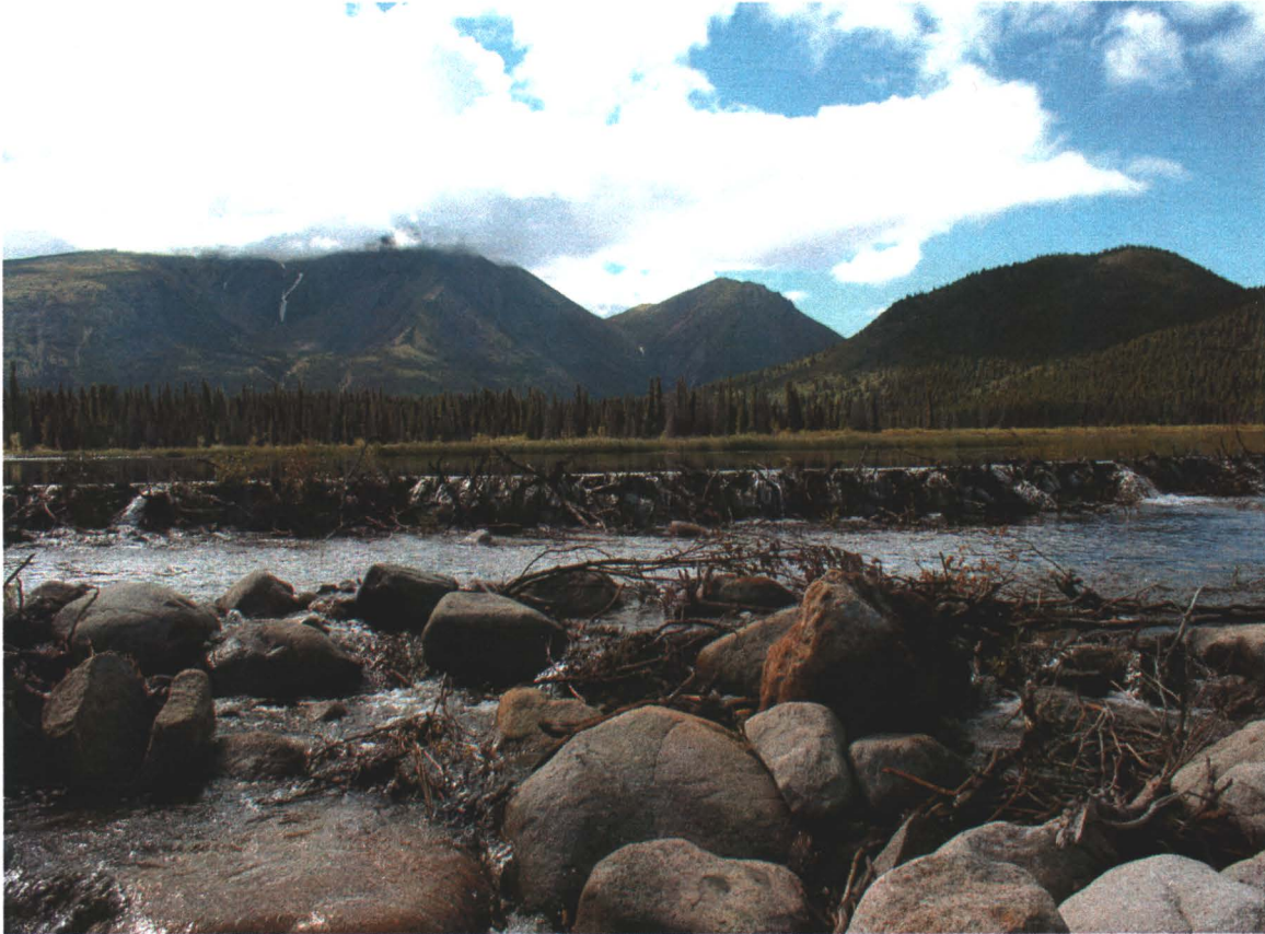
Photo 1: Beaver Dam near the Spillway
