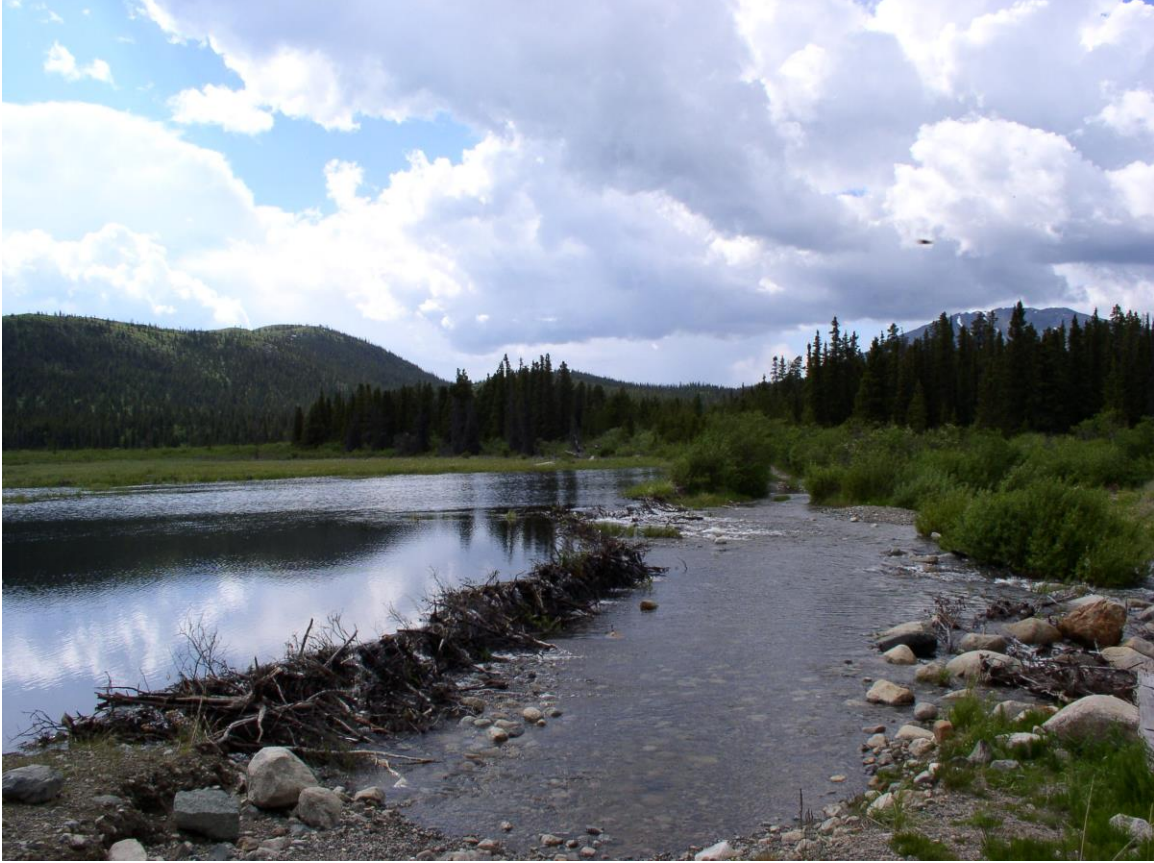
Photo 2: Beaver Dam near the Spillway
