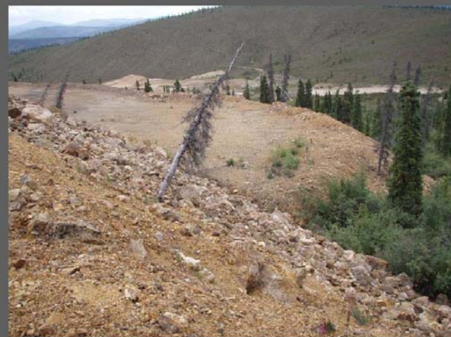
Photo 4e Examples of the surface condition of slopes and platforms of the waste rock pile
