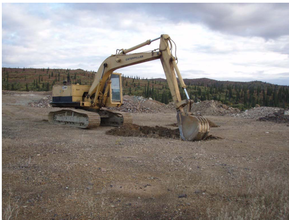
Photo 5d Test pit excavation, pit TP-1 on the Northwest Pile.
