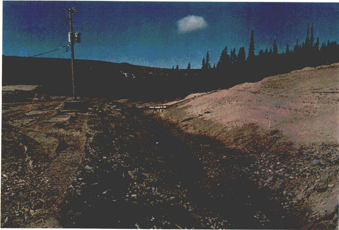
Photograph 13 North Diversion Ditch - looking west (pipelines crossings in background).
