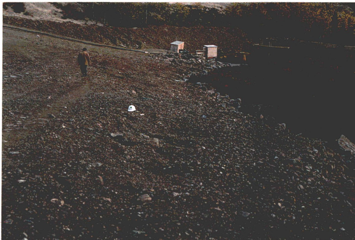
Photograph 6 Downstream Slope of Buttress Berm - looking downward towards Seepage Recovery Pond.
