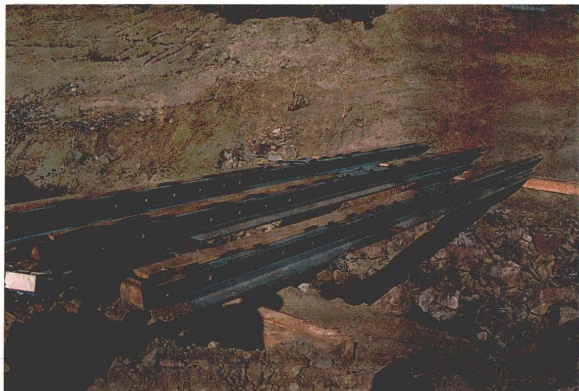
Photograph 12 Bridge construction in progress - across North Diversion Ditch.
