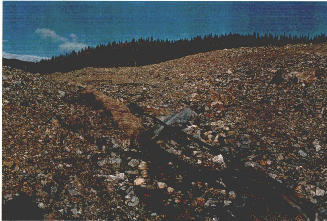
Photograph 11 Emergency Spillway Channel - upper segment (used also for conveying water from North Diversion Ditch).
