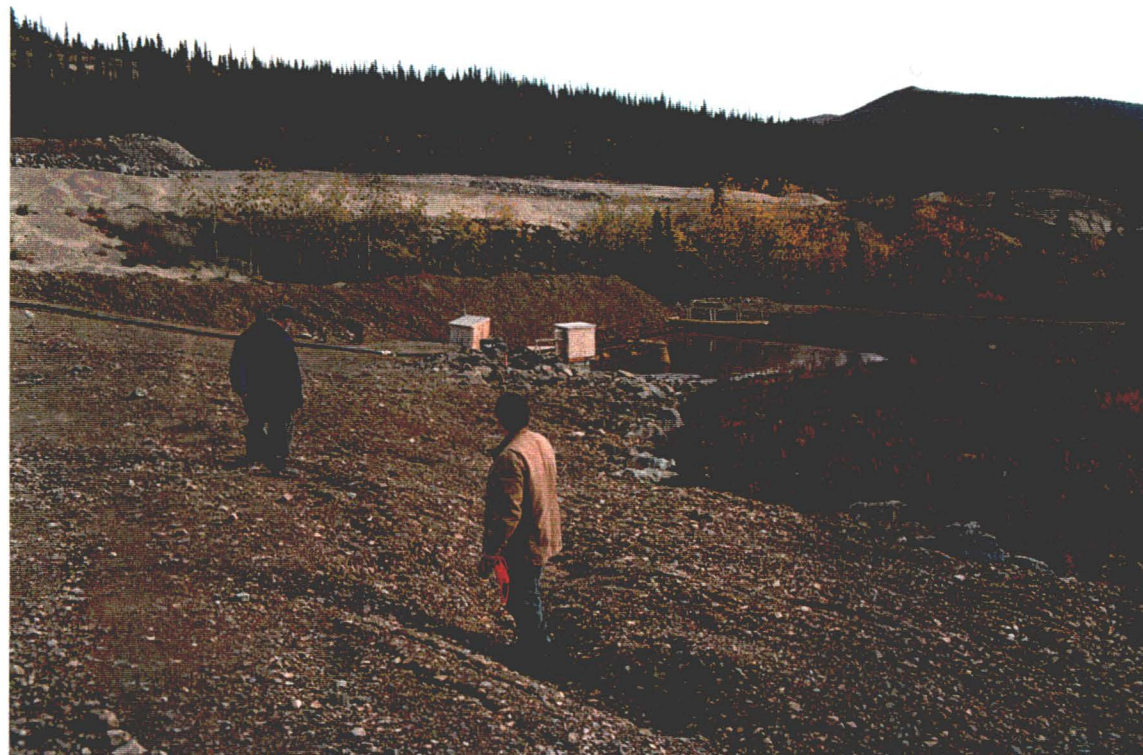
Photograph 7 Close-up of local depressions on buttress berm slope.
