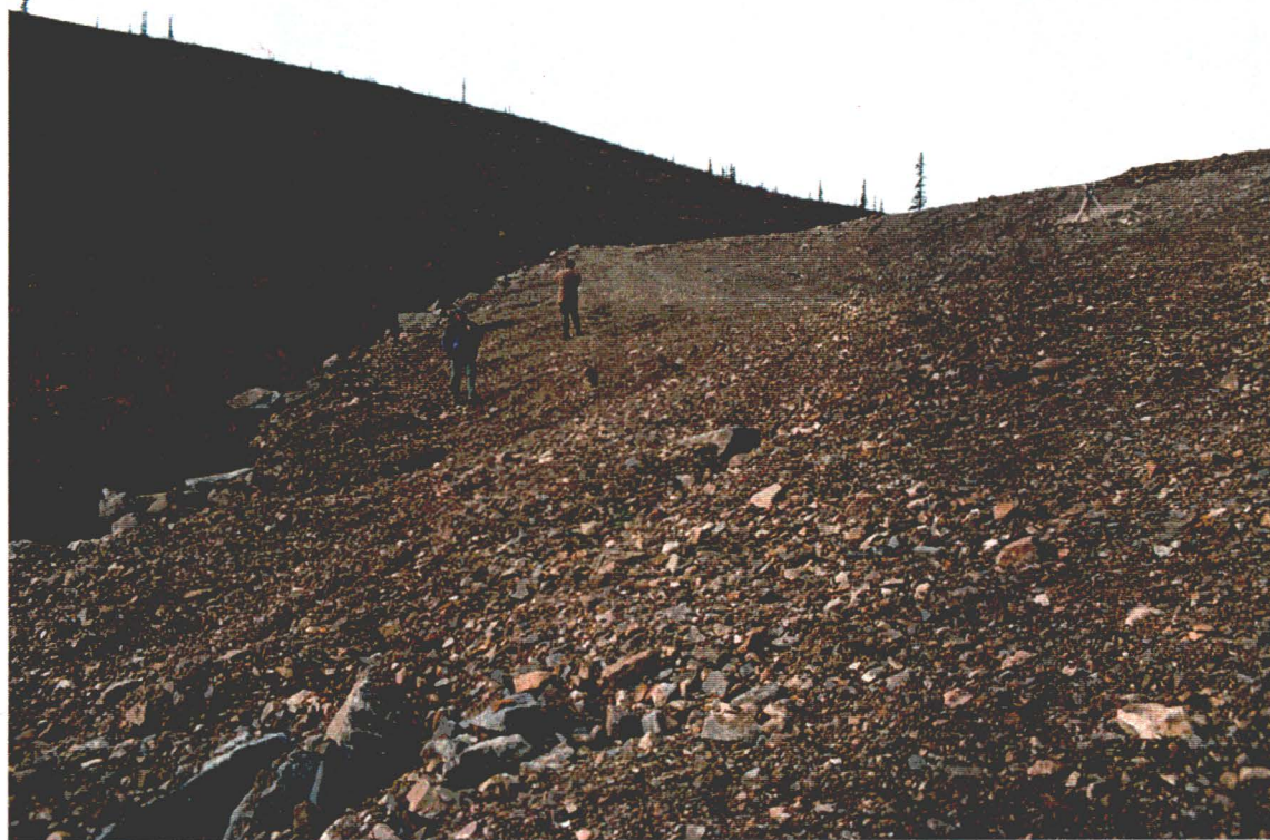
Photograph 5 Downstream Slope of Buttress Berm - looking upward towards south abutment.
