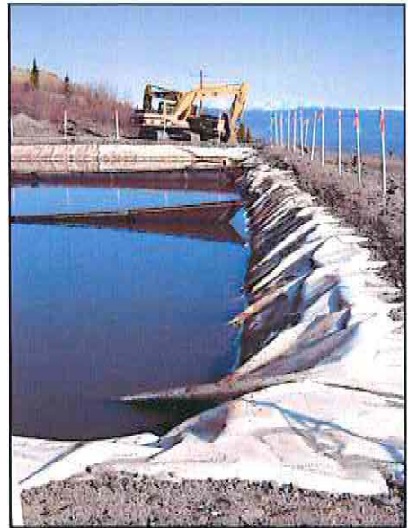
Plate 11 - Baffles installed in Galkeno 300 Settling Pond
