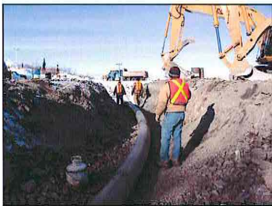
Plate 10 - Installation of pipe from Galkeno 300 adit to treatment pond
