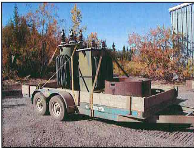
Plate 20 - Transformers being transported to storage area
