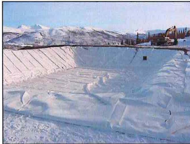
Plate 9 – Installation of Galkeno 300 Settling Pond
