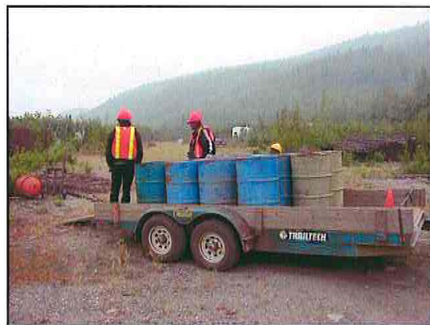
Plate 21 – Ewing employees moving waste hydrocarbon drums to bermed storage area
