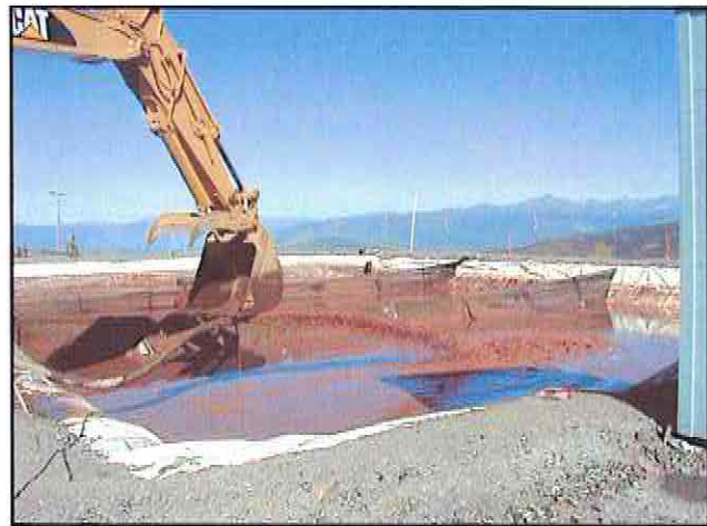
Plate 5 - De-sludging the Galkeno 300 treatment pond
