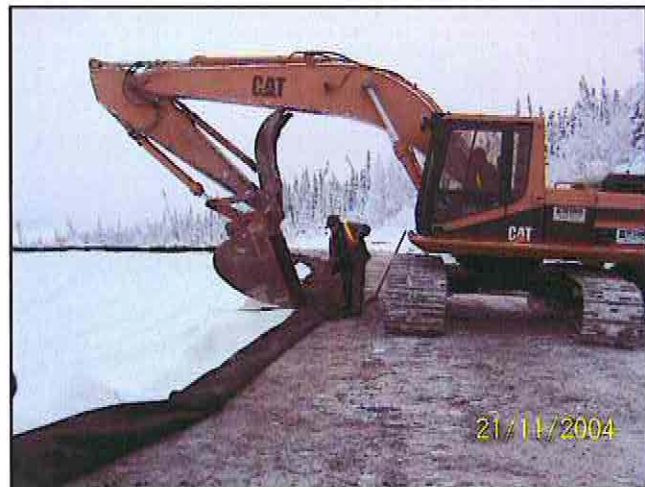
Plate 8 – Galkeno 900 treatment pond liner installation
