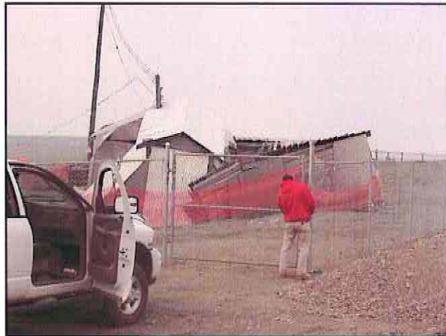
Plate 15 - Newly installed security fence surrounding partially-collapsed Shamrock 'J' Raise structure
