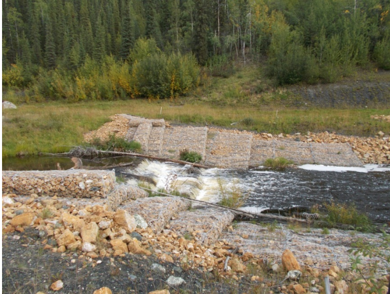
Photo 24: DS1 looking north.
