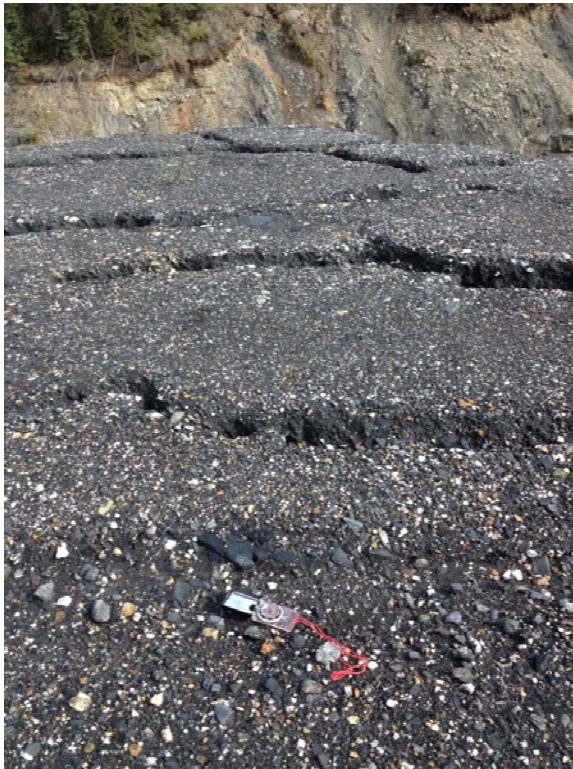
Photo 13: Decommissioned access road east of DS4 looking north.
