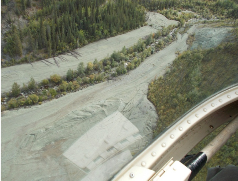
Photo 58: Tailings slope and Wolverine Creek looking southeast.
