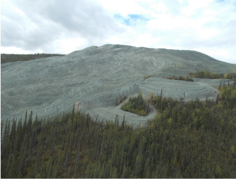
Photo 62: Tailings slope looking southwest.
