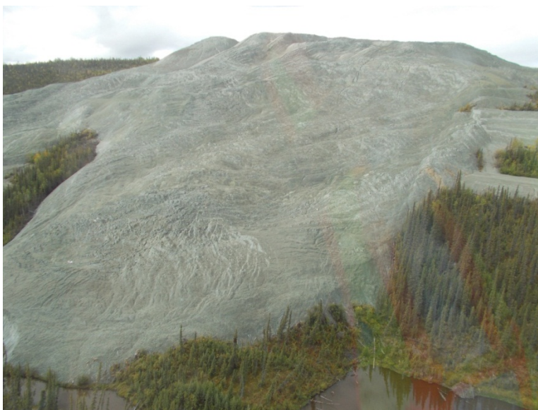
Photo 61: Tailings slope looking west.
