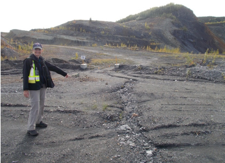
Photo 2: Access Road north of Porcupine Pit looking south.
