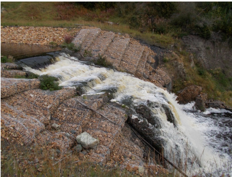
Photo 33: DS4 looking north.
