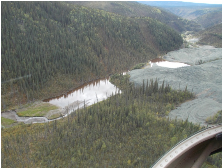
Photo 81: Wolverine Creek tailings ponds looking southeast.
