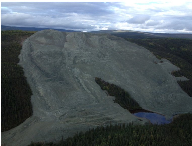
Photo 63: Tailings slope and tailings pond looking west.
