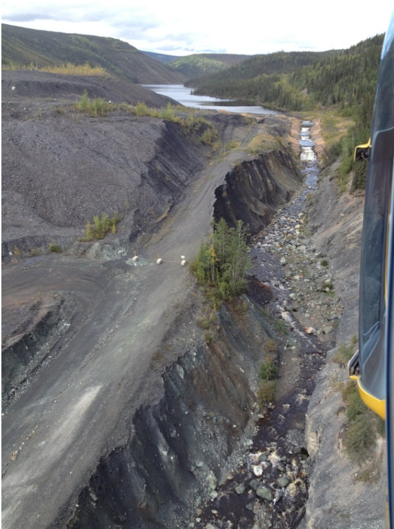
Photo 11: Decommissioned access road and Clinton Creek east of DS4 looking west.
