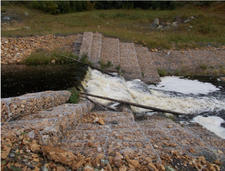
Photo 28: DS3 looking north.
