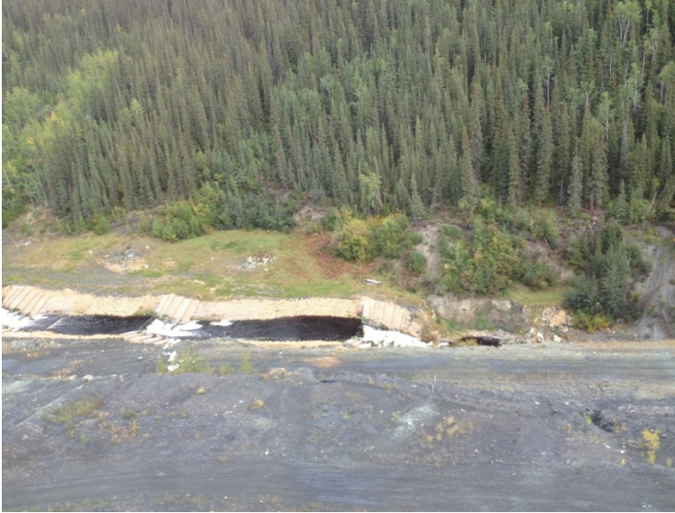
Photo 46: Drop structures looking north.
