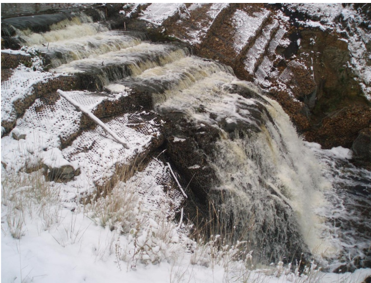
Photo 41: DS4 in 2013 looking north.
