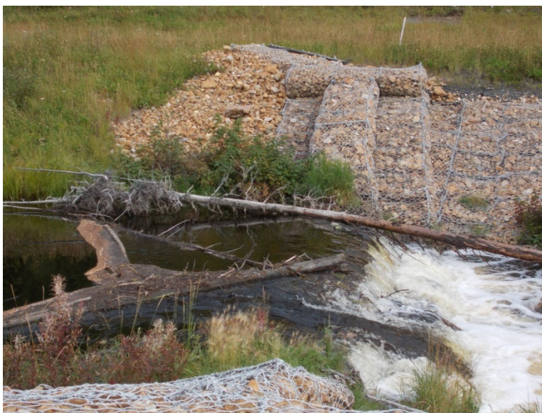
Photo 25: DS1 looking north.
