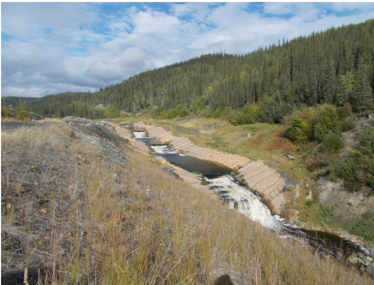
Photo 43: Drop structures looking northwest.
