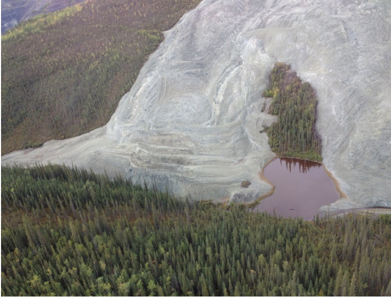
Photo 64: Tailings slope and tailings pond looking west.
