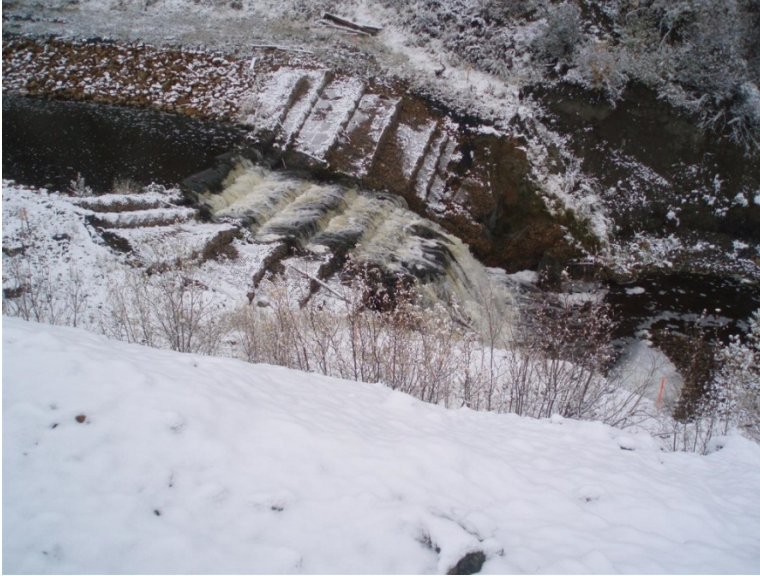
Photo 42: DS4 in 2013 looking north.
