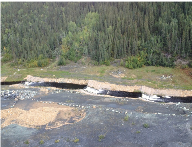
Photo 45: Drop structures looking north.
