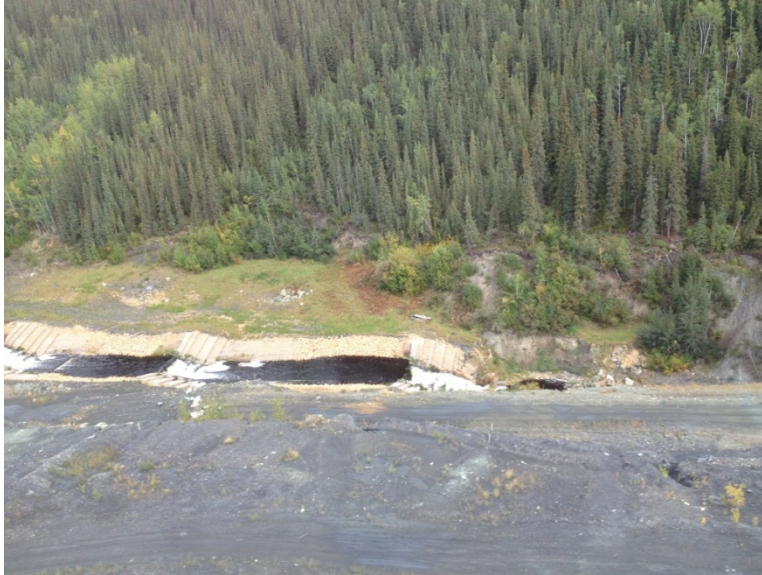
Photo 46: Drop structures looking north.
