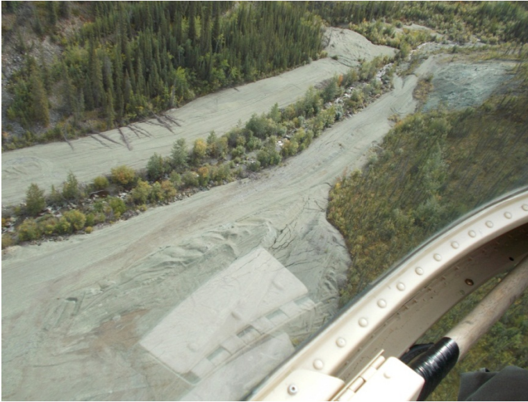
Photo 58: Tailings slope and Wolverine Creek looking southeast.
