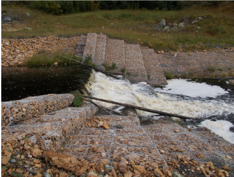
Photo 28: DS3 looking north.
