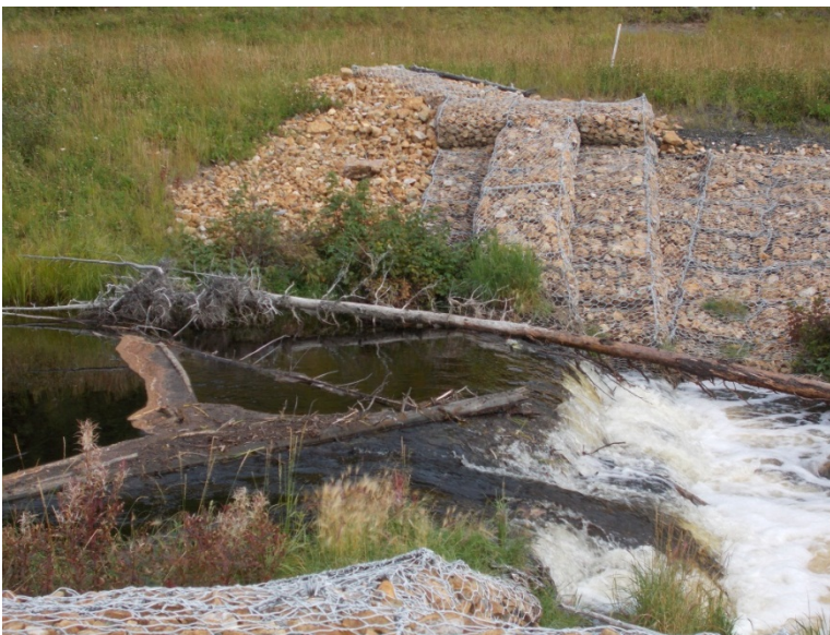
Photo 25: DS1 looking north.
