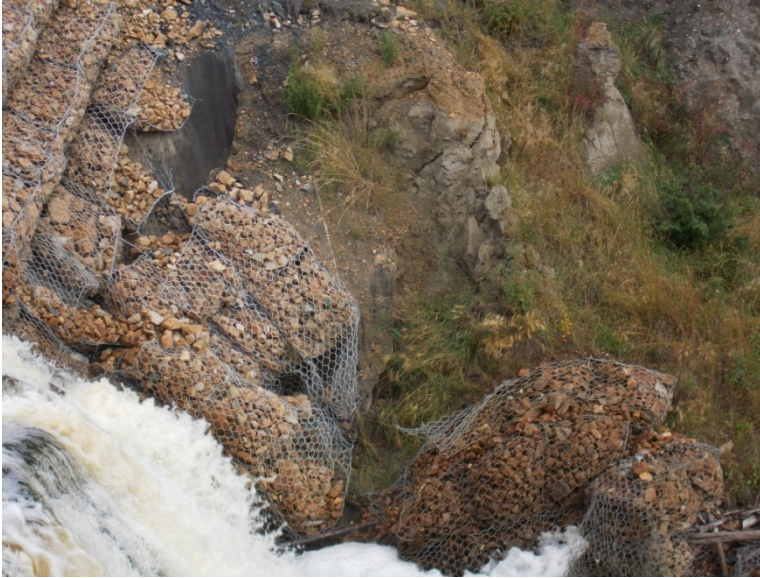
Photo 34: DS4 looking north.
