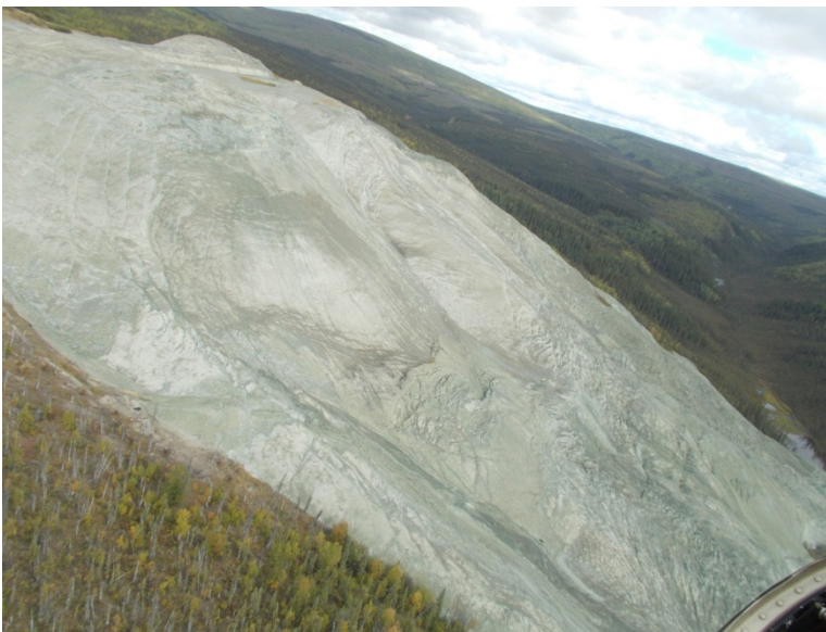
Photo 55: Tailings slope looking north.
