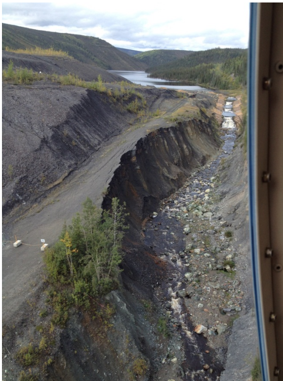
Photo 8: Decommissioned access road and Clinton Creek east of DS4 looking west.
