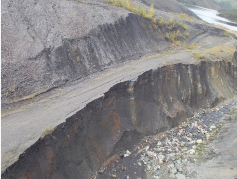
Photo 9: Decommissioned access road east of DS4 looking southwest.
