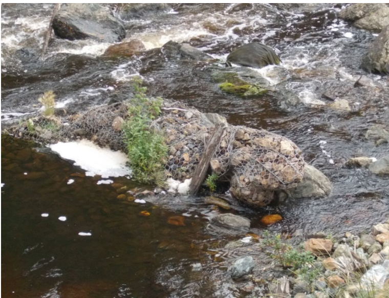
Photo 35: Failed gabion basket downstream (east) of DS4.
