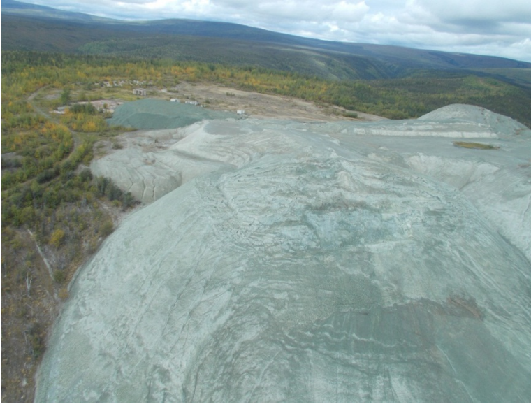
Photo 56: Tailings slope looking west.
