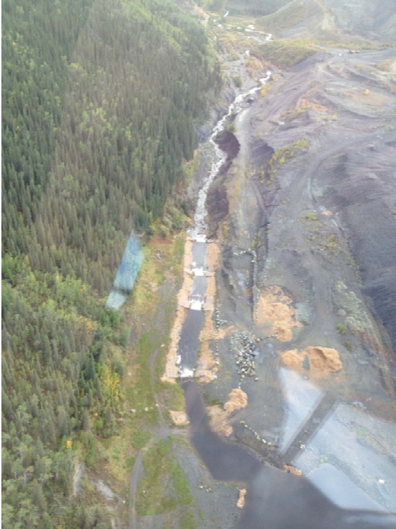
Photo 44: Drop structures looking east.
