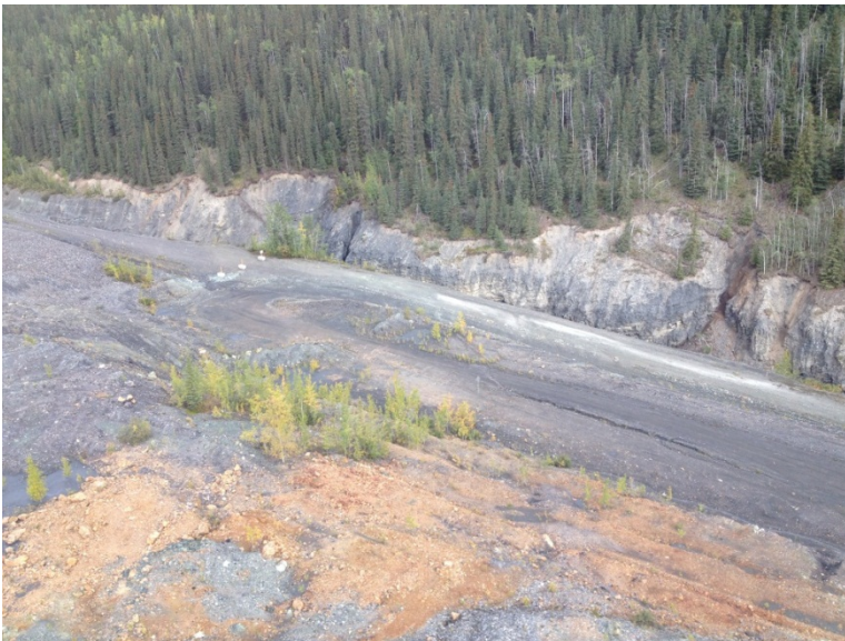
Photo 21: Access road north of Snowshoe Pit looking northwest.
