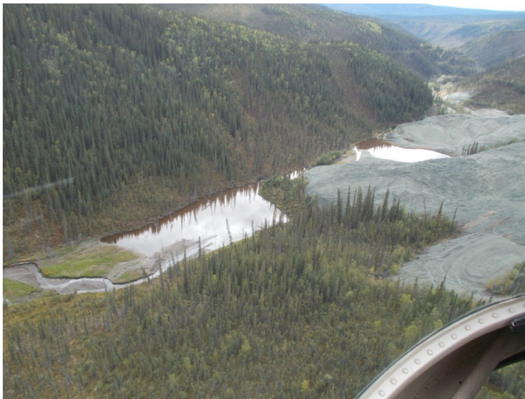
Photo 81: Wolverine Creek tailings ponds looking southeast.
