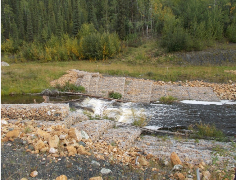
Photo 24: DS1 looking north.
