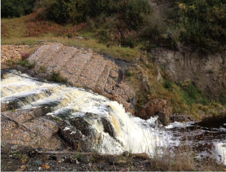
Photo 38: DS4 looking north.
