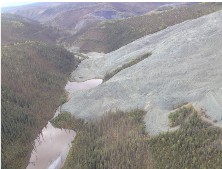
Photo 65: Tailings slope and tailings pond looking south.
