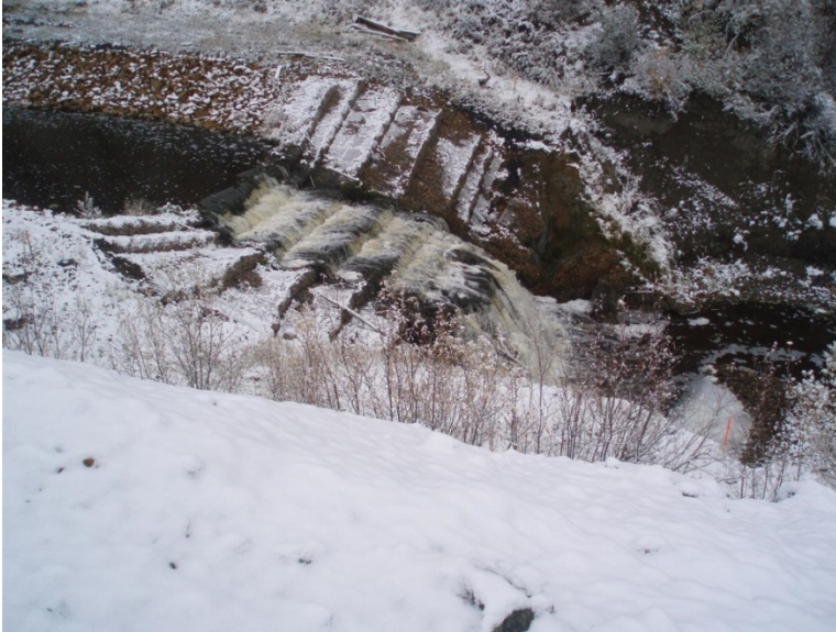
Photo 42: DS4 in 2013 looking north.
