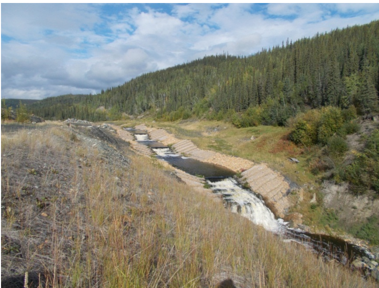
Photo 43: Drop structures looking northwest.
