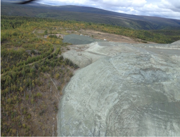
Photo 66: Tailings slope looking southwest.
