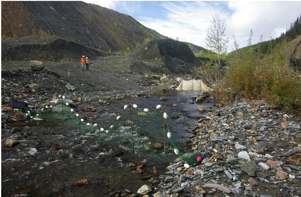
Photo 1: View of the isolated and salvaged area at the Clinton Creek ford crossing location, showing the reduced isolation area. Photo taken August 10, 2015.
