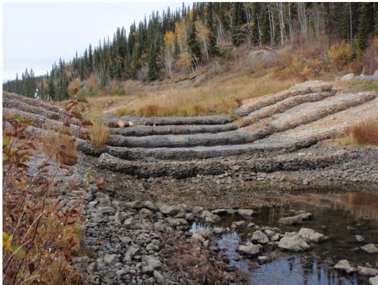
Photo 22: Drop Structure No. 1 looking northwest.
