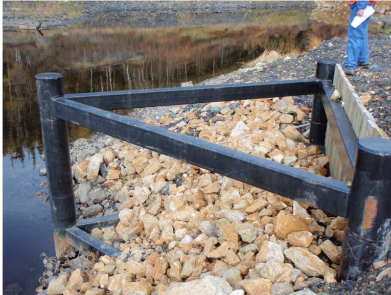
Photo 17: Hudgeon Lake south abutment looking northeast.
