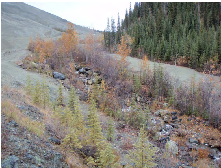
Photo 52: Wolverine Creek rock lined channel looking northwest.
