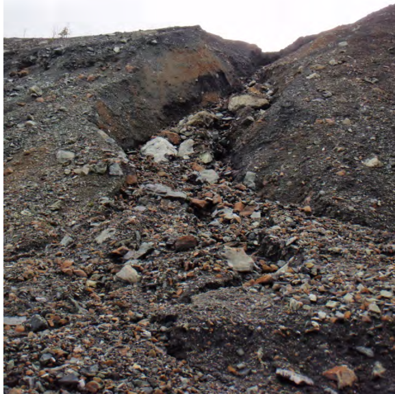
Photo 42: Clinton Creek Waste Rock Pile slope erosion near Ford Crossing No. 1 looking south.
