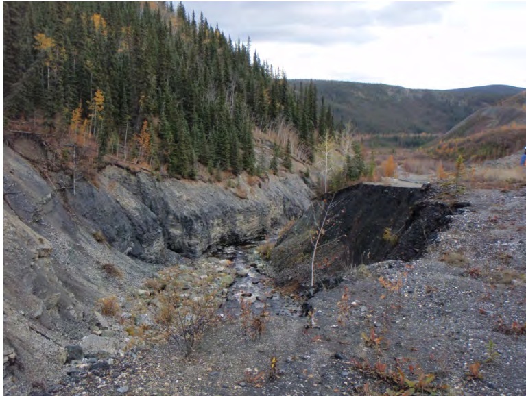
Photo 11: Closed portion of access road embankment looking east.
