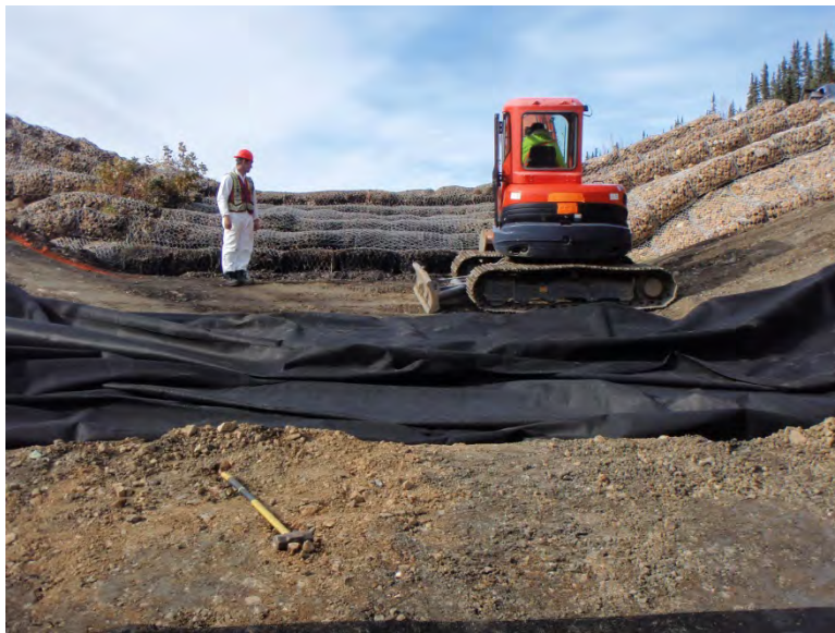
Photo 28: Drop Structure No. 4 transition to revetment chute looking west.
