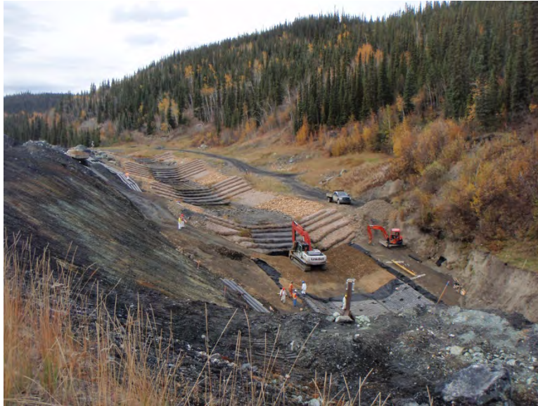
Photo 21: All drop structures looking northwest.
