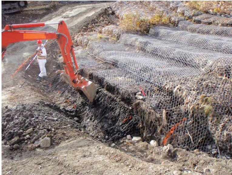
Photo 29: Drop Structure No. 4 transition to revetment chute looking southwest.
