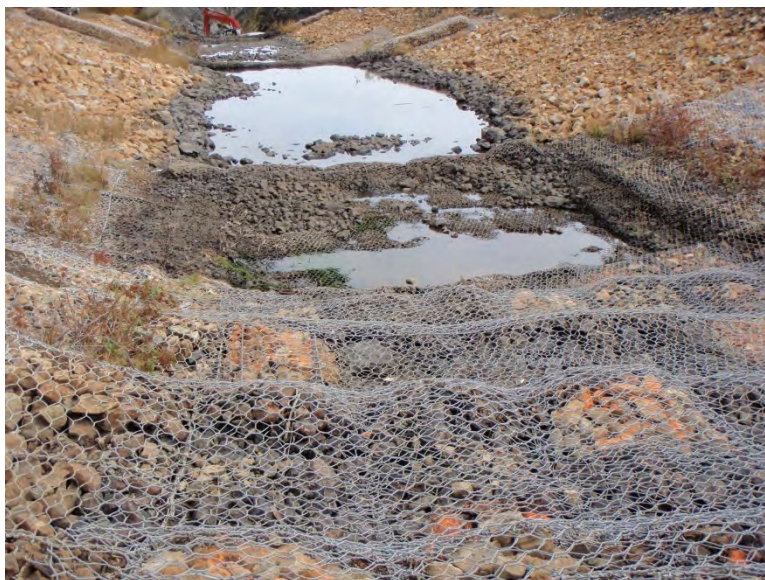
Photo 24: Drop Structure No. 2 downstream pool looking east.
