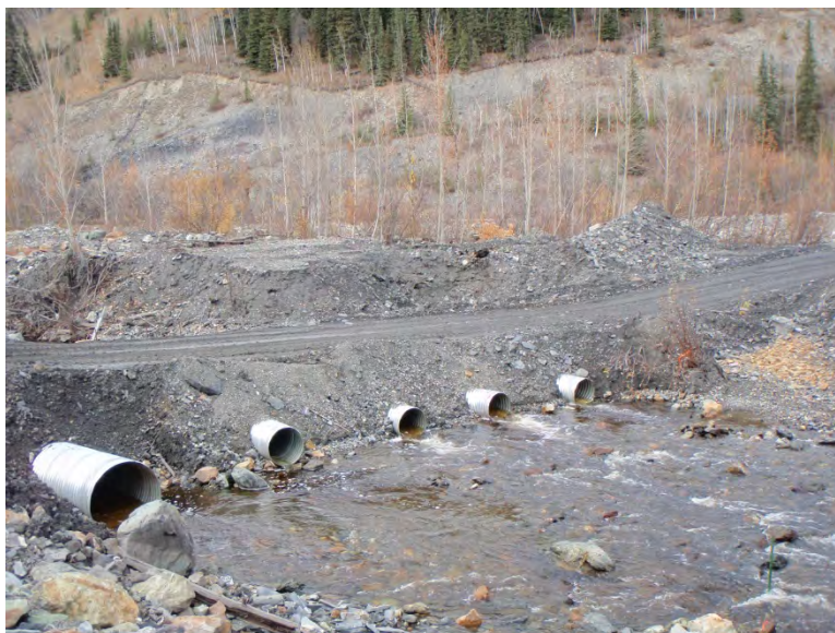
Photo 4: Downstream side of Ford Crossing No. 1 temporary infrastructure looking northwest.
