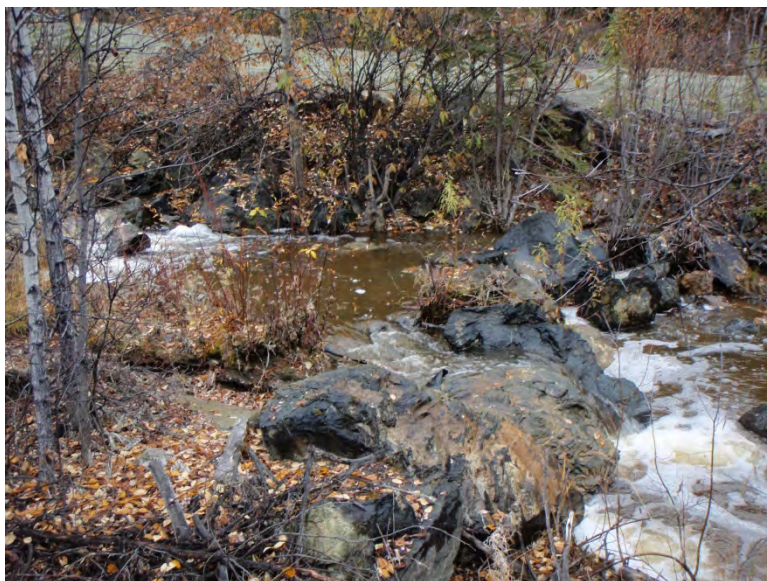
Photo 54: Wolverine Creek rock weir looking east.
