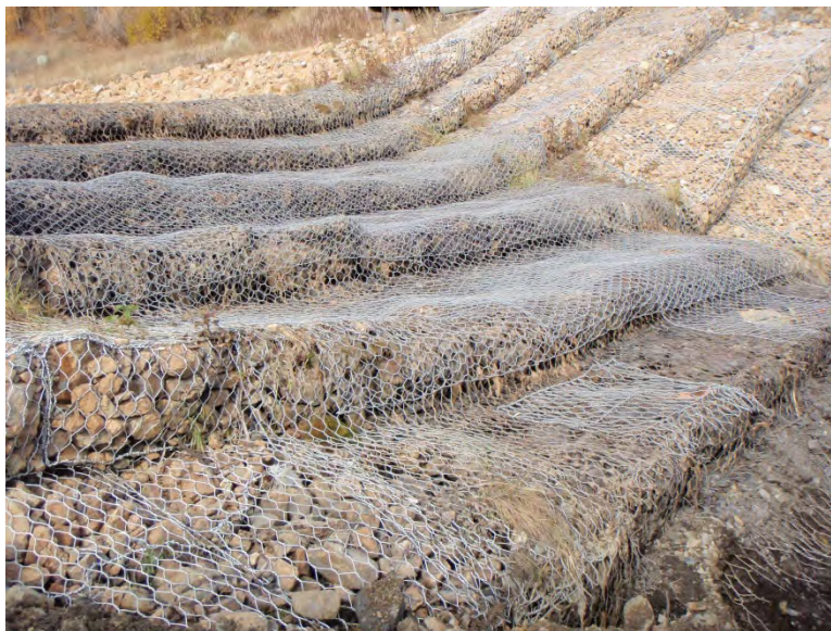
Photo 31: Additional mesh installed at Drop Structure No. 4.
