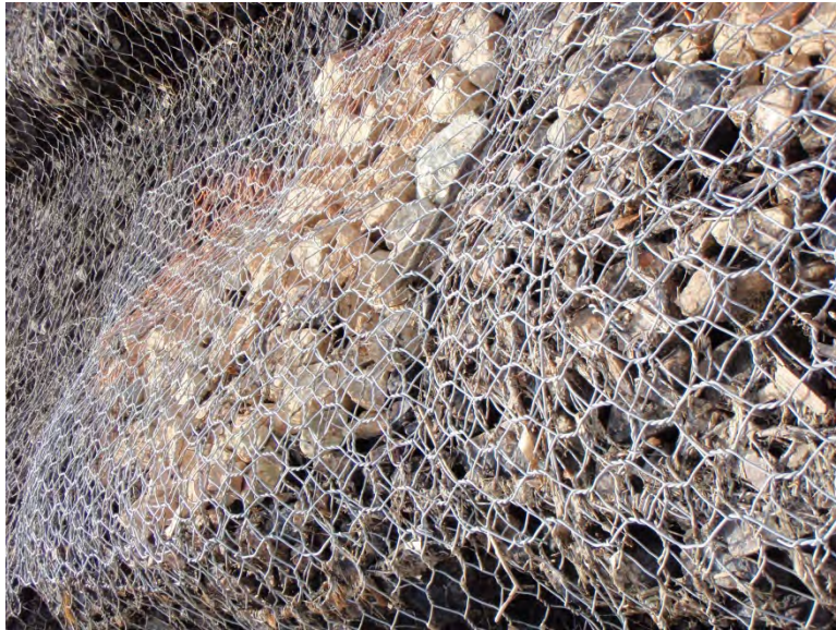
Photo 27: Repaired drop structure gabion basket looking southwest.
