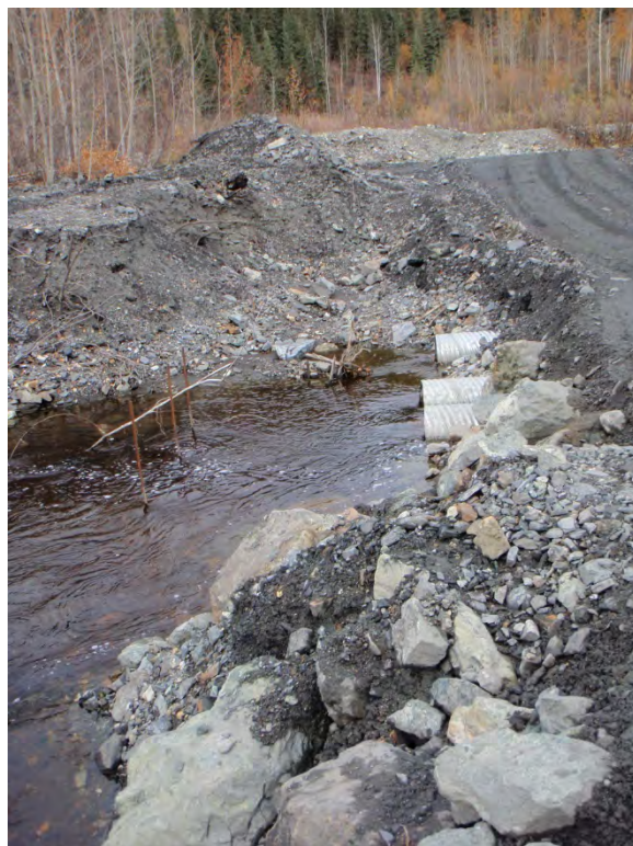
Photo 5: Upstream side of Ford Crossing No. 1 temporary infrastructure looking north.
