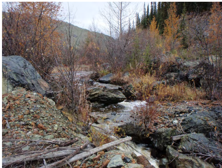
Photo 55: Wolverine Creek rock weir looking northwest.
