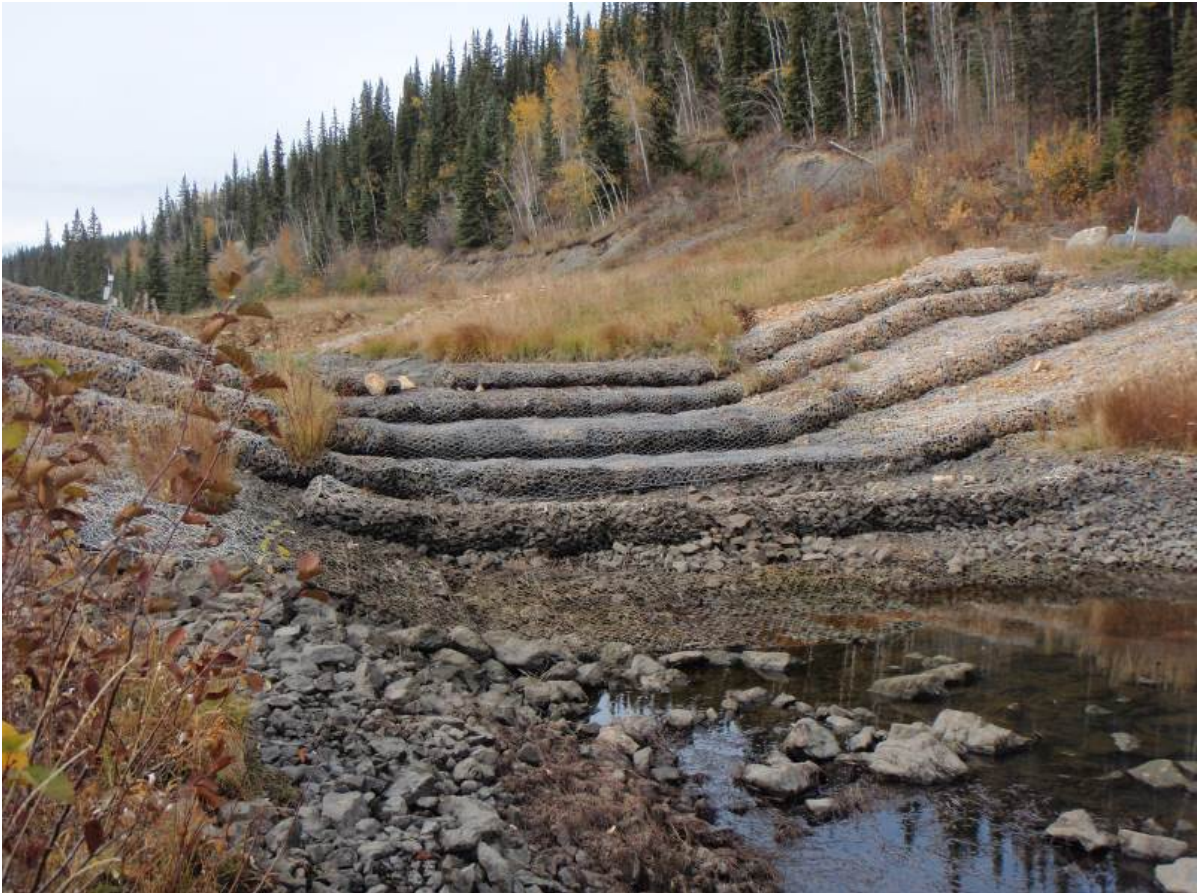
Photo B Drop Structure No. 1 Looking West (Upstream)
