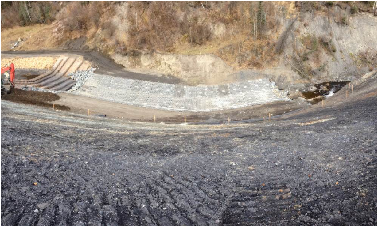
Photo C Repaired Drop Structure No. 4 Looking North
