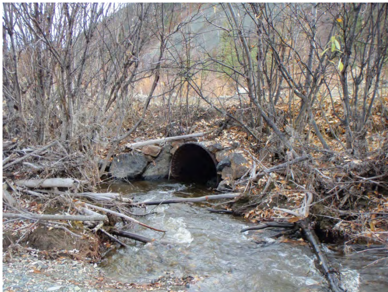
Photo 48: Wolverine Creek culvert inlet looking southeast.
