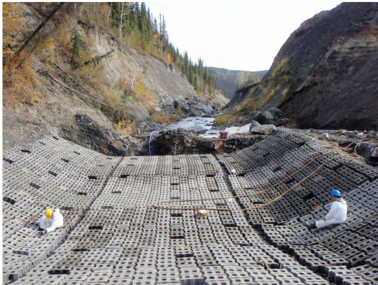
Photo 30: Drop Structure No. 4 revetment chute looking east.
