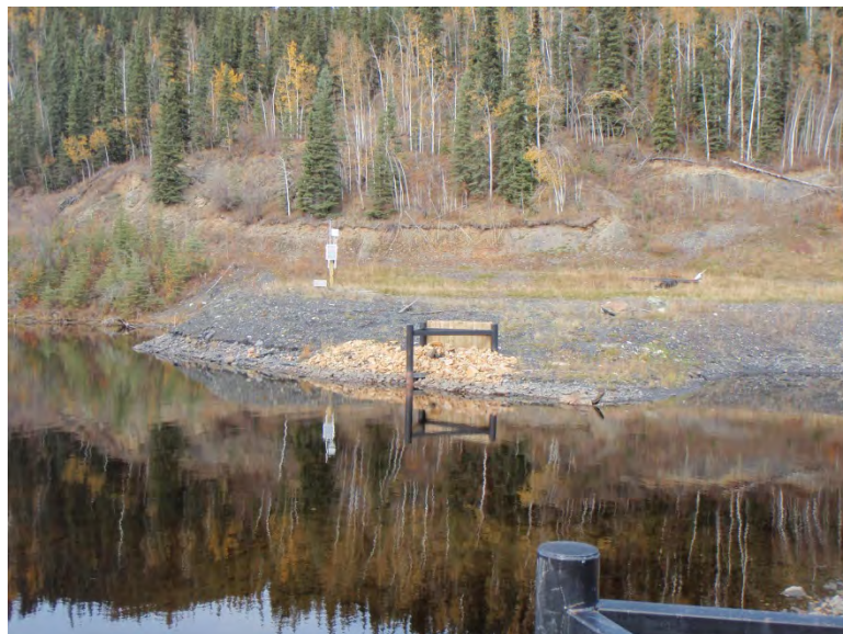
Photo 16: Hudgeon Lake north abutment looking north.
