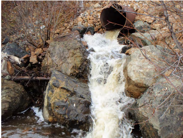
Photo 47: Wolverine Creek culvert outlet at confluence with Clinton Creek looking northwest.
