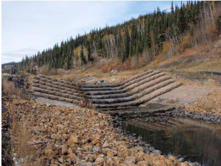
Photo 23: Drop Structure No. 2 looking northwest.
