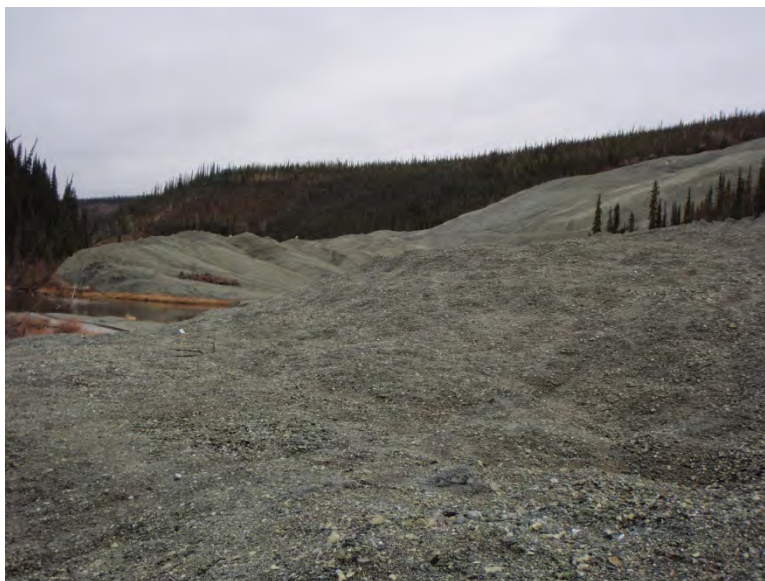
Photo 70: Bottom of Wolverine Creek Tailings Pile south lobe looking south.
