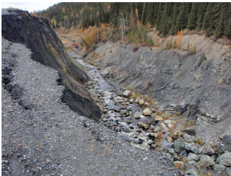
Photo 14: Closed portion of access road top of bank looking west.
