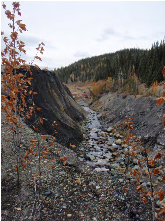
Photo 10: Closed portion of access road embankment looking west.
