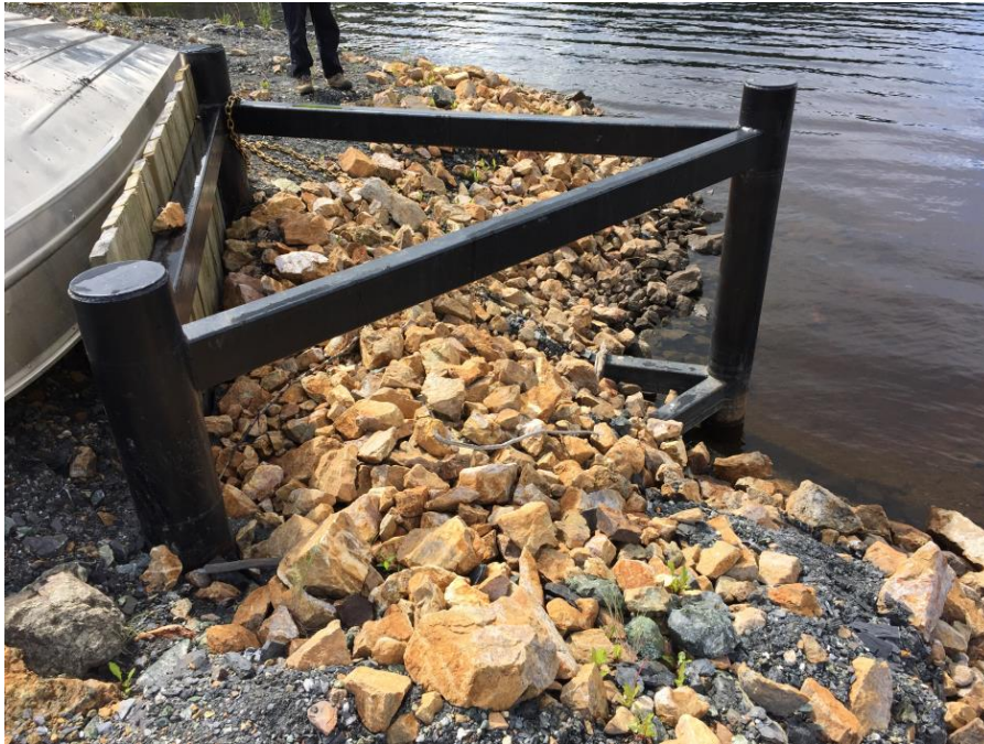
Photo 14 South Boom Abutment, looking west
