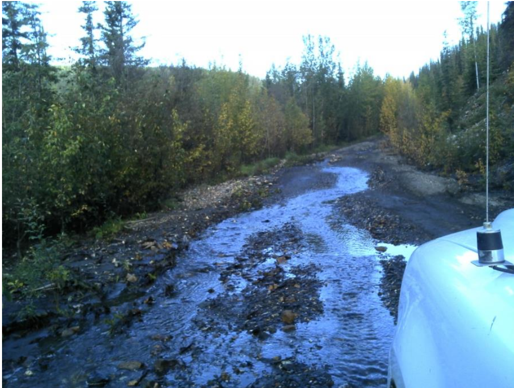
Photo B Clinton Creek Site Access Road – Erosion (August 29, 2016)
