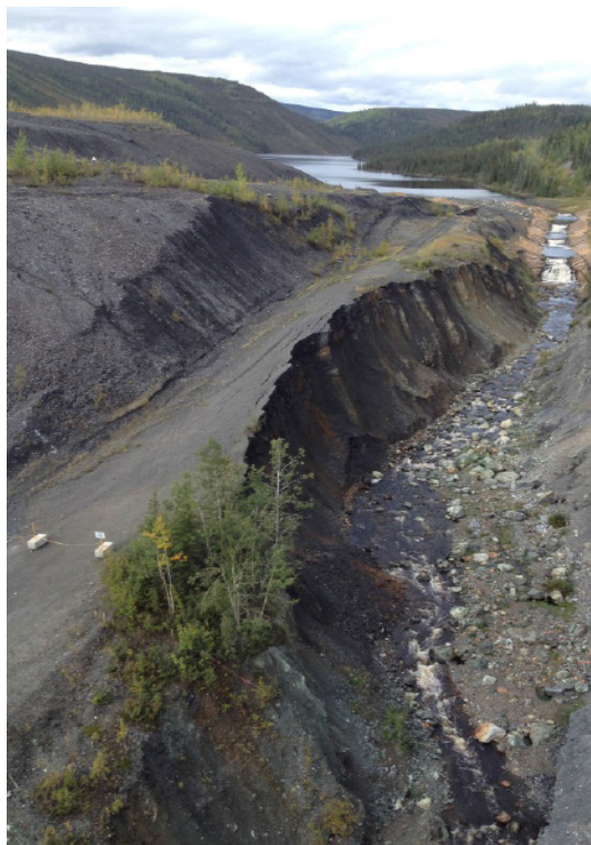
Figure E Decommissioned access road and Clinton Creek east of DS4 looking west (left) and potential deep seated failure mechanism (right)
