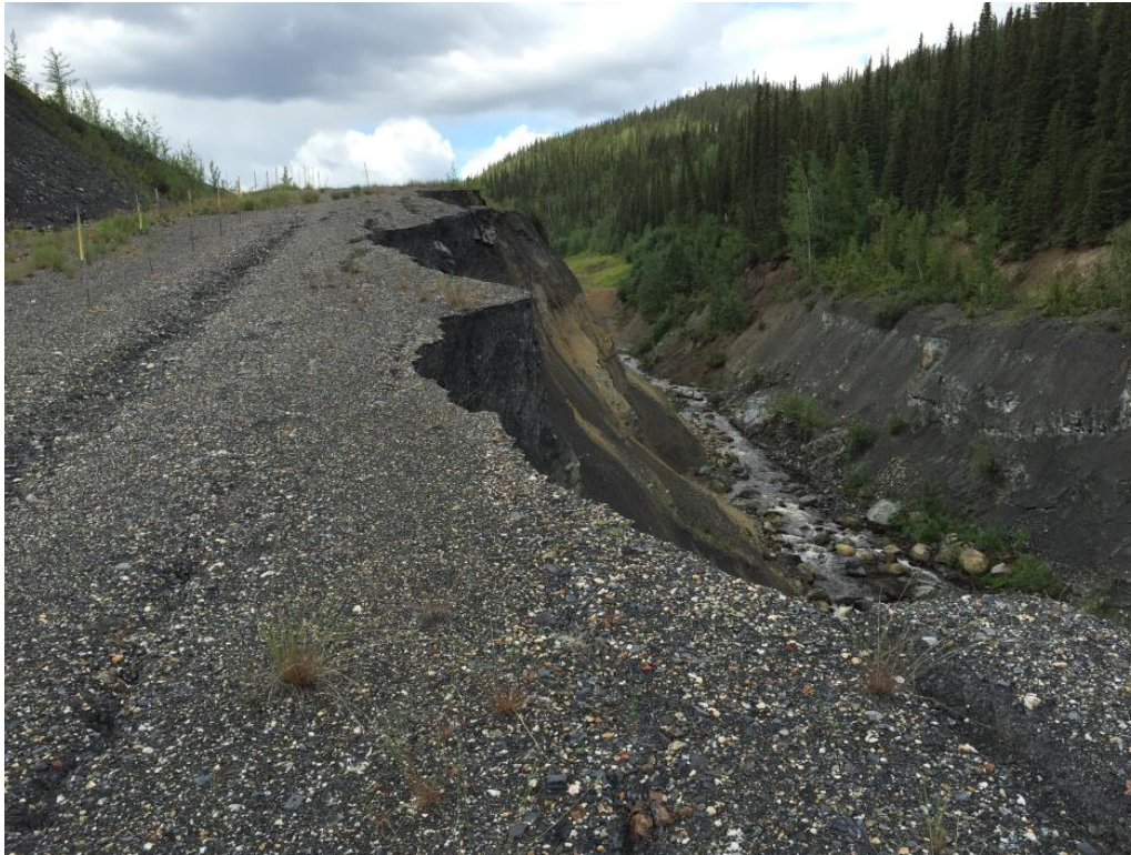
Photo C Closed Section of Clinton Creek Site Access Road – Looking West (June, 2016)
