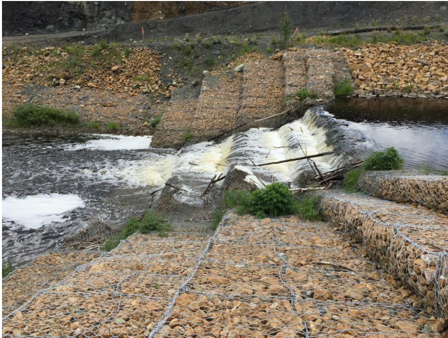
Photo 19 Drop Structure 3, looking south
