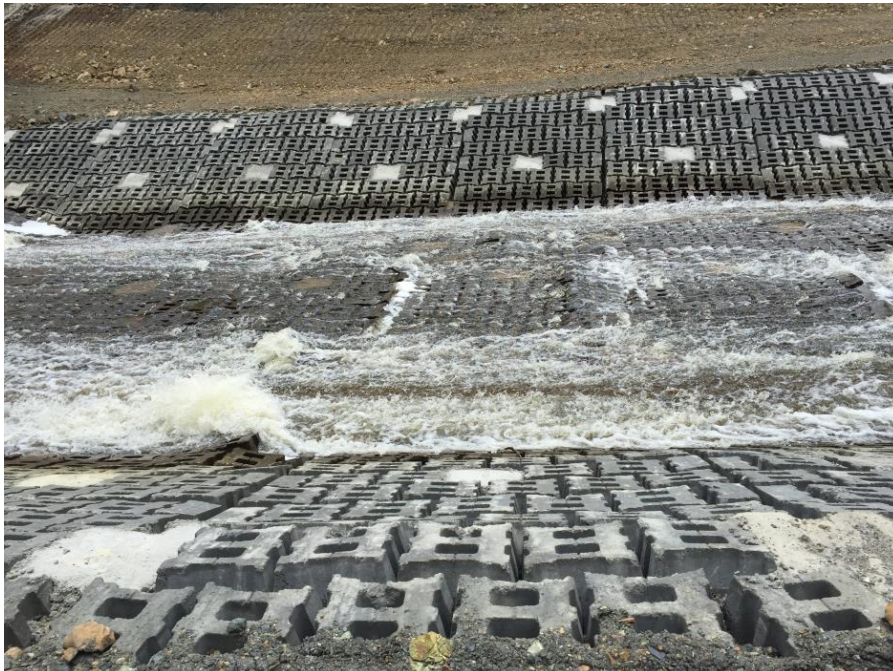
Photo 23 DS4 Repair – ACB Channel looking south at Mats 6, 7, 8 and 9 from top
