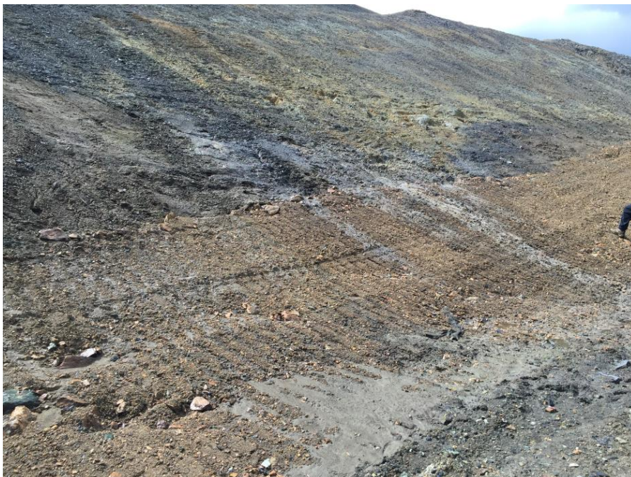
Photo 34 Groundwater Seep at 2015 permafrost location (Slope south of DS4)
