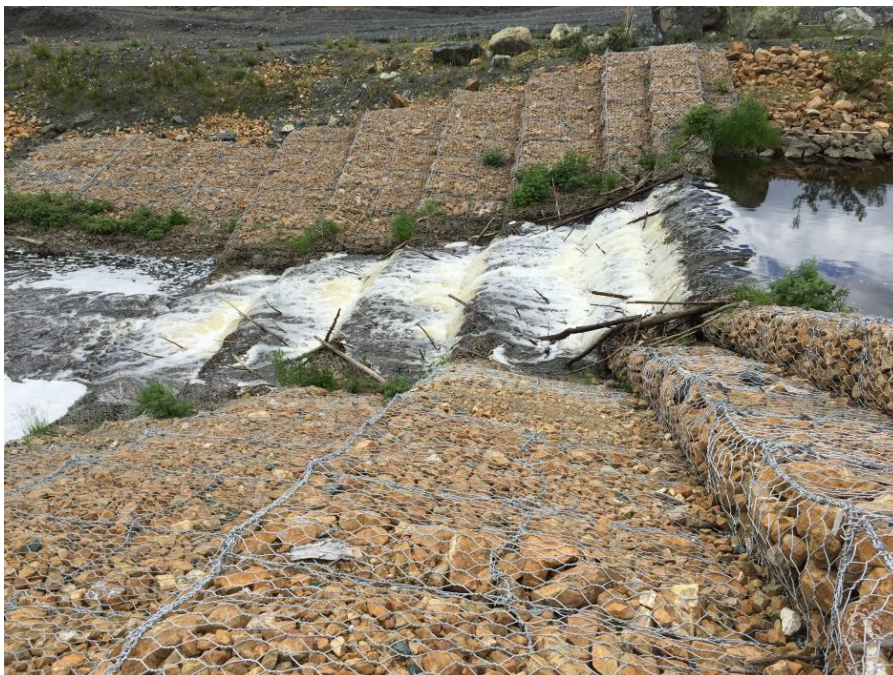
Photo 18 Drop Structure 2, looking south
