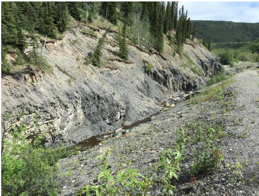
Photo 30 Between closed road and Fording No. 1, looking downstream – failed slope encroaching on creek
