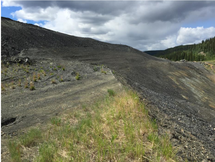
Photo 33 Stabilized Slope south of DS4, looking west
