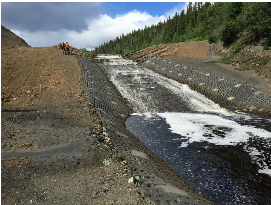
Photo 21 DS4 Repair – ACB Channel looking west
