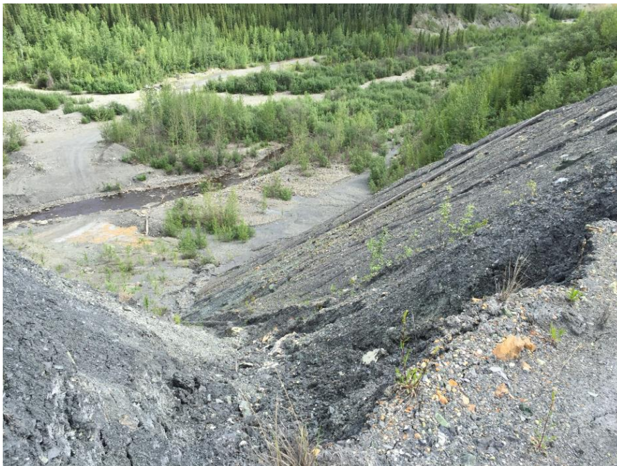
Photo 36 Erosion of slope south of Fording No. 1, delta of eroded sediment
