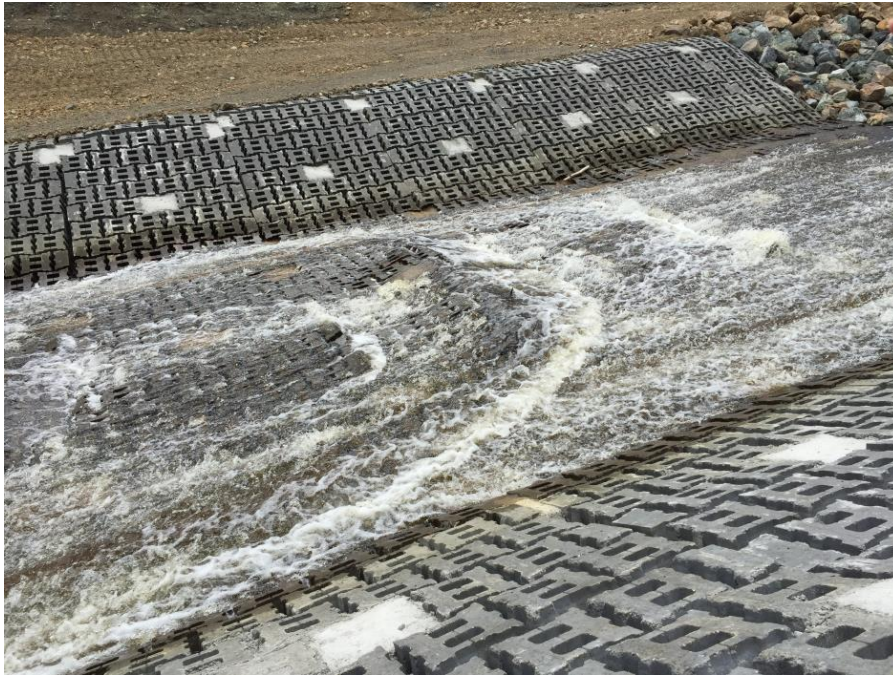
Photo 22 DS4 Repair – ACB Channel looking south at Mats 4, 5 and 6 from top
