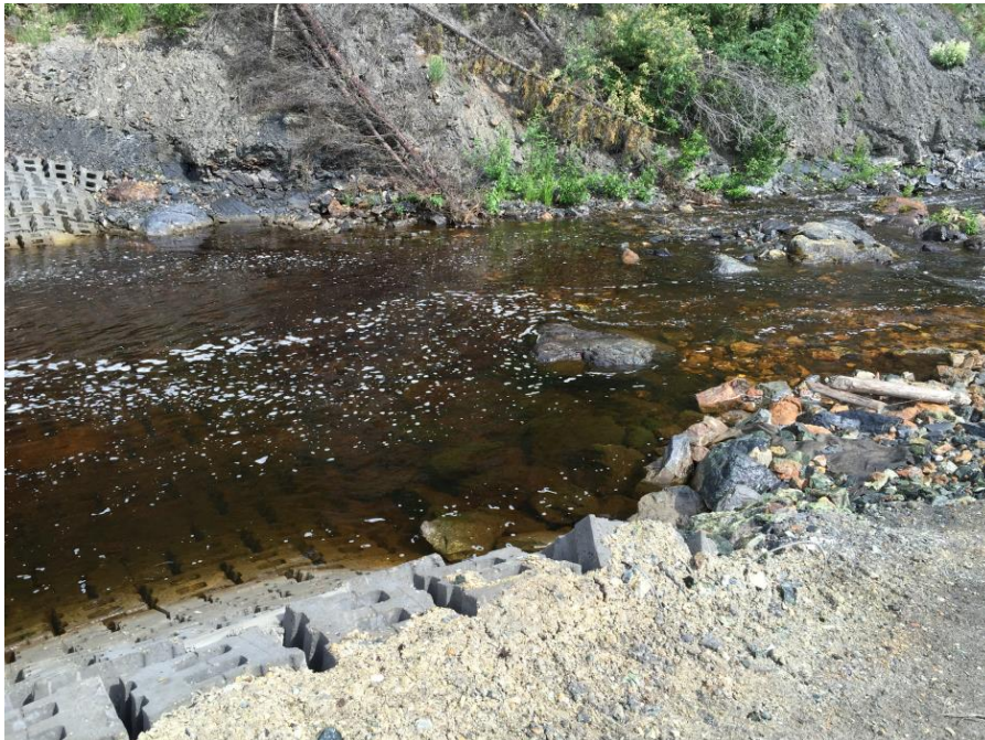
Photo 25 DS4 Repair – ACB channel looking north at outlet
