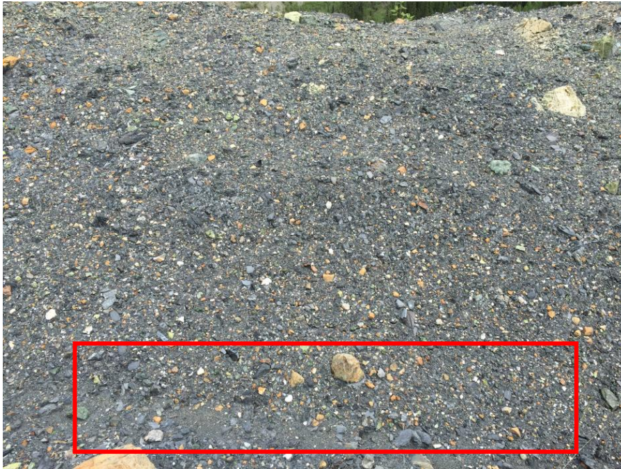
Photo 35 Cracks in soil at crest of slope south of Fording No. 1
