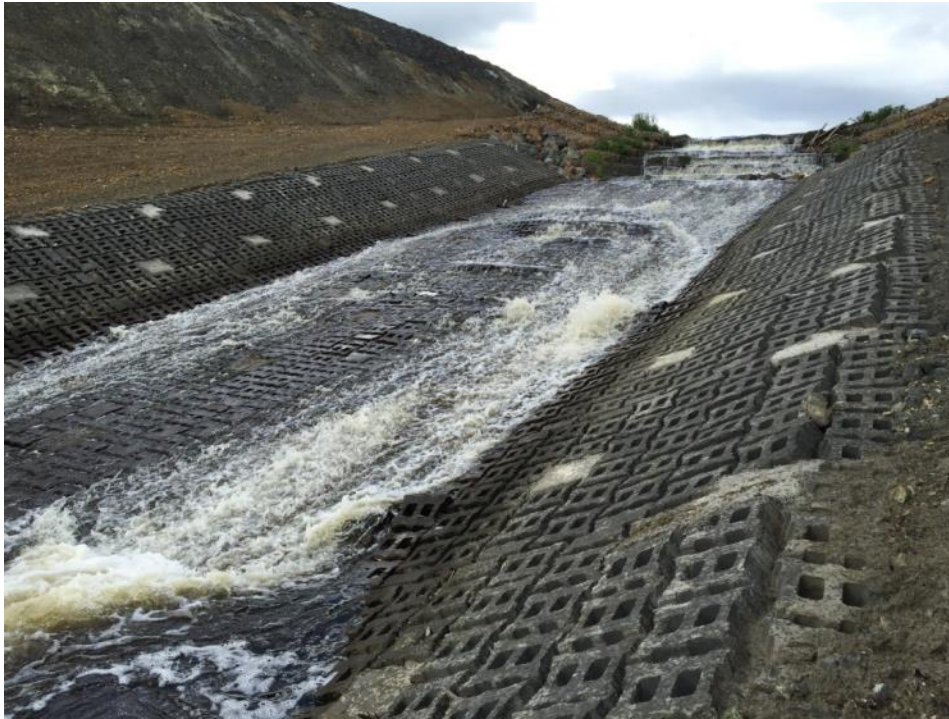
Photo E Drop Structure 4 ACB Channel, looking southwest (June 21, 2016)
