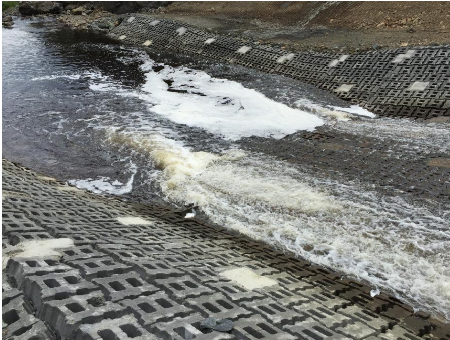
Photo 24 DS4 Repair – ACB Channel looking southeast at Stilling Basin
