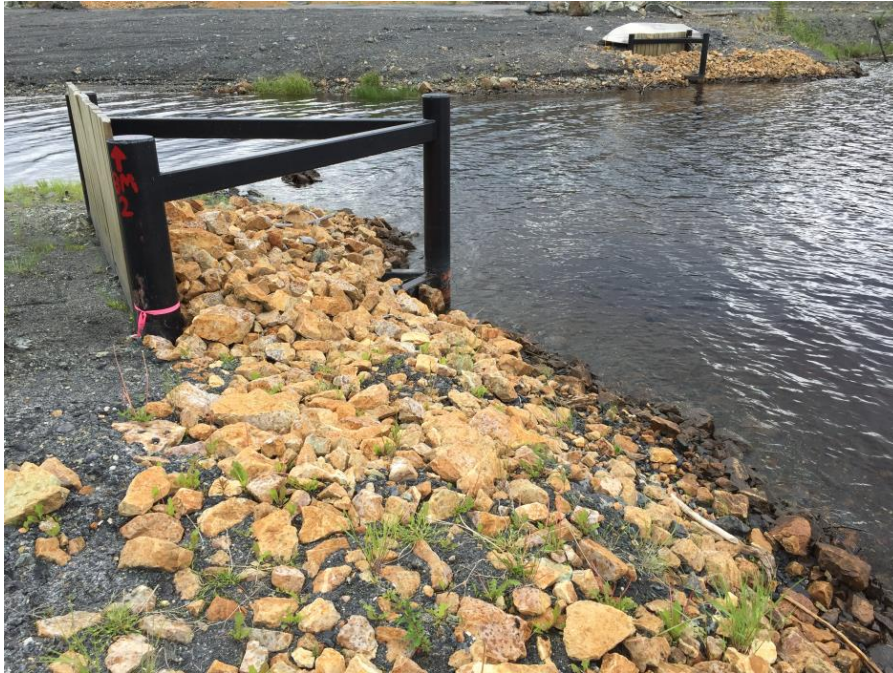
Photo 12 North Boom Abutment, looking south
