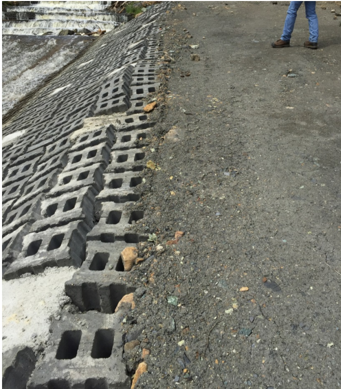
Photo 26 DS4 repair – ACB channel Anchor Trench
