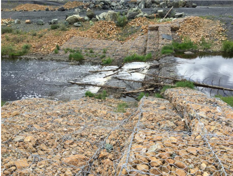
Photo 17 Drop Structure 1, looking south
