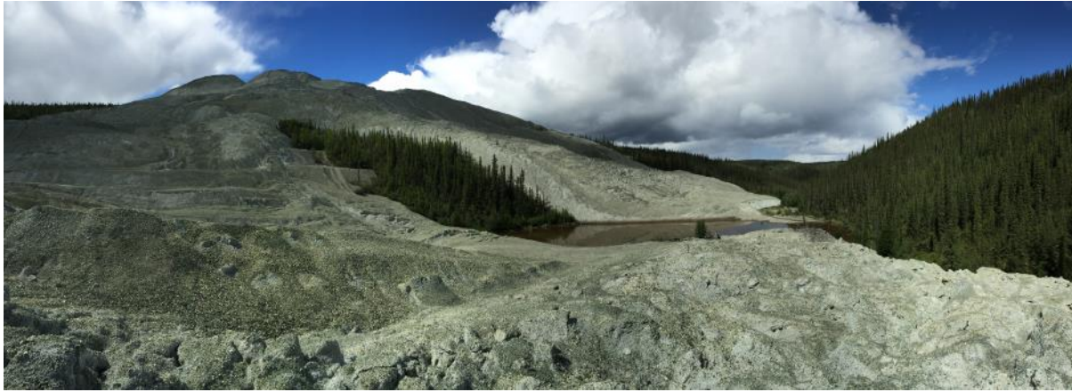
Photo 42 Tailings Pile Panorama from base of slope
