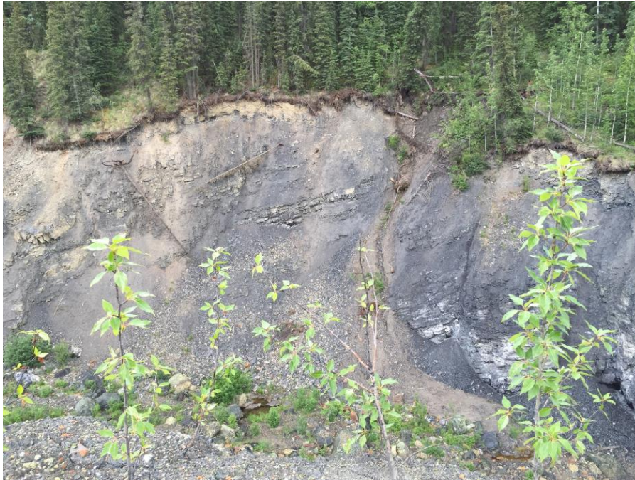
Photo 29 Minor Slope Failure, looking north
