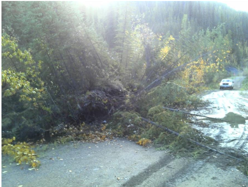
Photo A Clinton Creek Site Access Road – Landslide (August 29, 2016)
