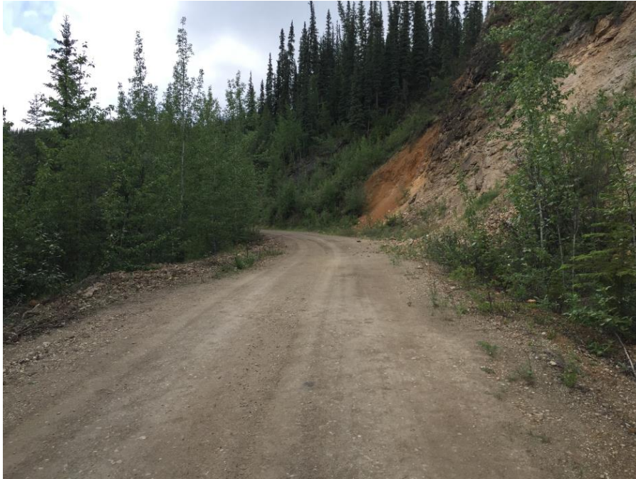
Photo 2 Typical Road Conditions
