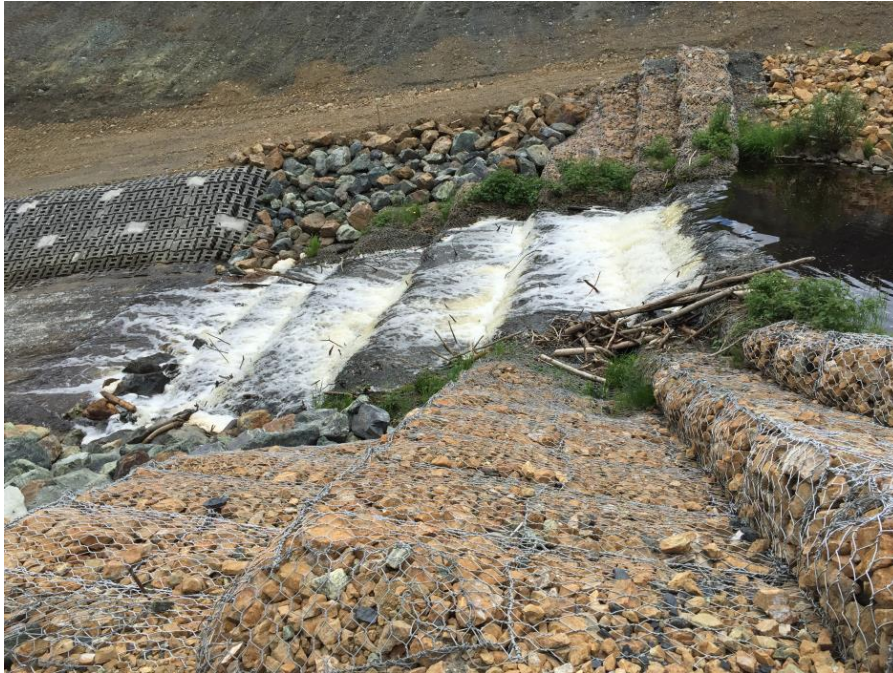
Photo 20 Drop Structure 4, looking south
