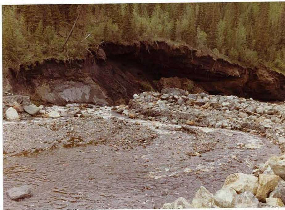
Photo 4: Detailed view of upstream weir section; note the height of breached bank relative the weir height and driftwood position.
