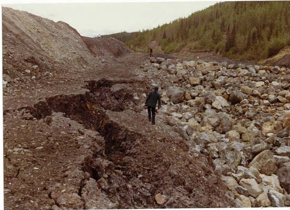
Photo 5: Sloughing of the undercut dump at the weir section.
