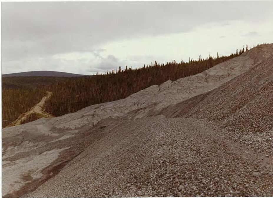
Photo 11: View of disturbances affecting the upper section of the south lobe.
