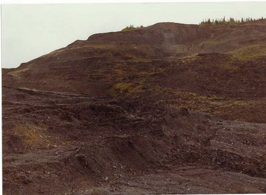
Photo 2: Continuing subsidence within the central portion of the dump.
