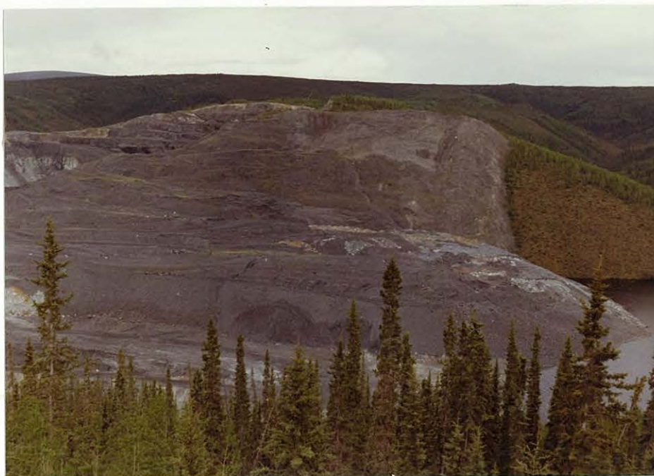
Photo 1: Clinton Creek Waste Dump.
