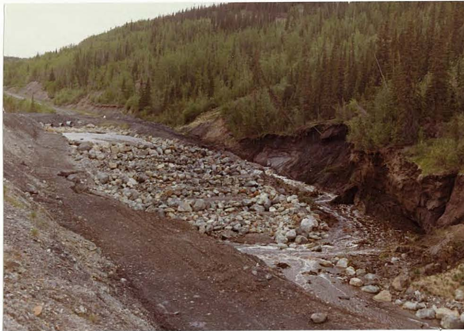
Photo 3: Clinton Creek weir system; stream bypassing the system and undercutting the bank.
