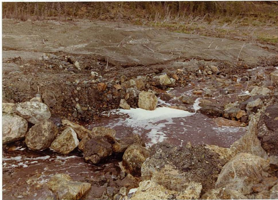
Photo 18: Reconstructed bottom weirs and rock apron below the weir floodway.
