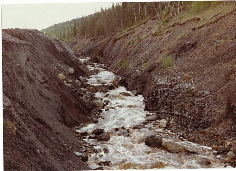
Photo 7: Downstream segment of Clinton Creek channel cut through waste dump and into the bedrock.
