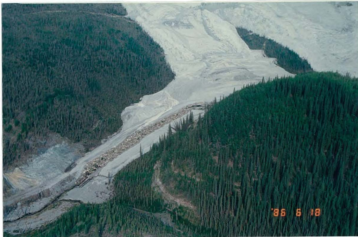
Photo 12: Rock lined outfall channel is dry. A new channel is developing along the east side of the valley fill.
