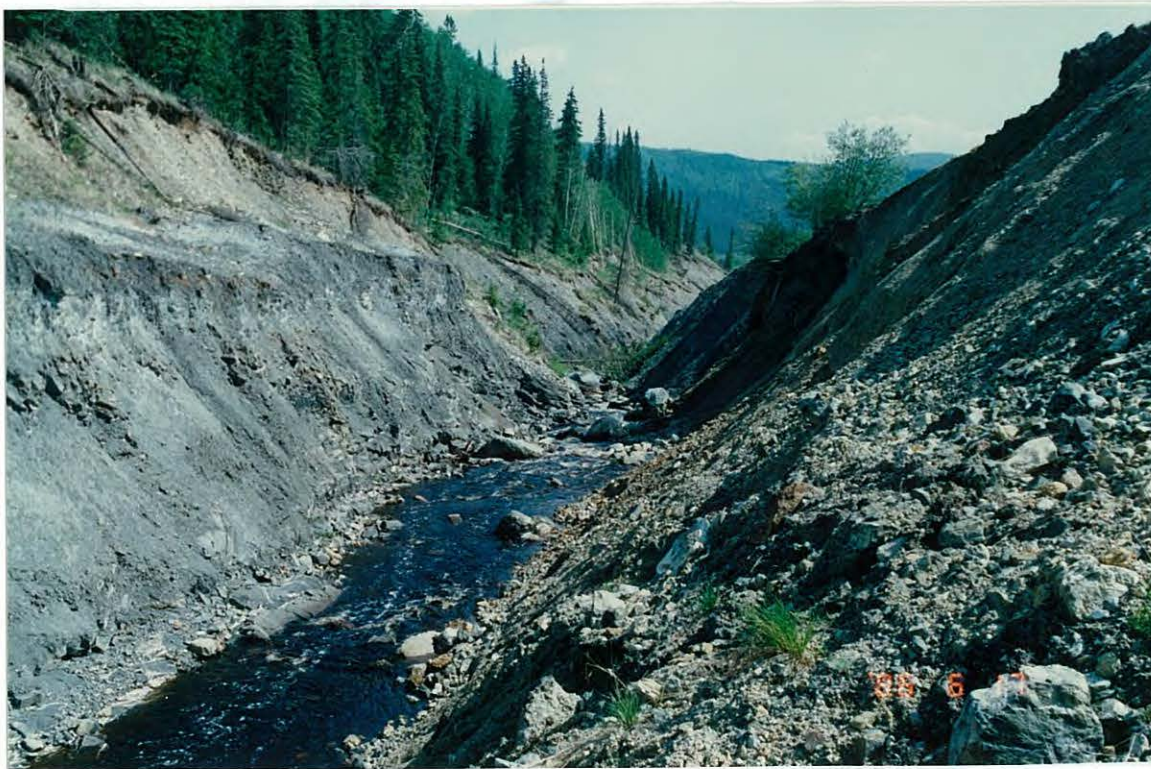
Photo 6: Oversteepened channel banks.
