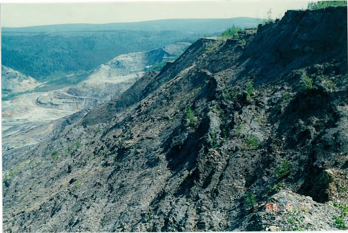
Photo 3: Fresh cracks in the headscarp of the waste dump confirm recent movements.
