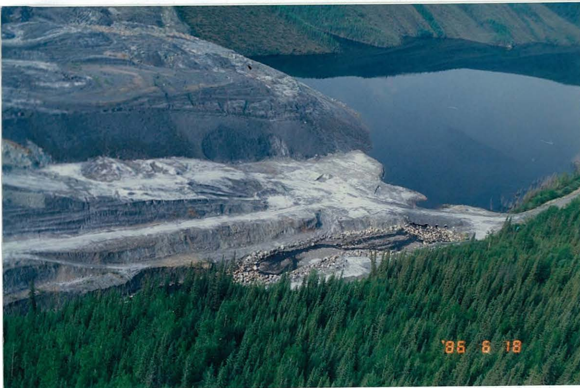
Photo 2: Upstream face of the dump and outfall from the lake.
