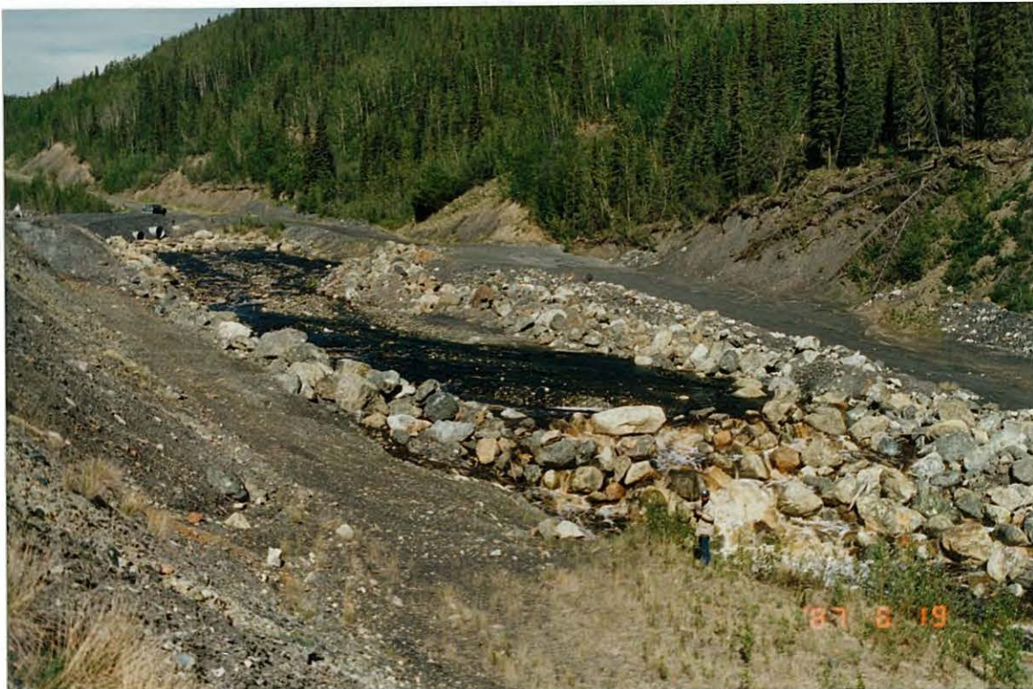
Photo 4: Lake outfall, armoured banks and drop weir did not change since 1986.
