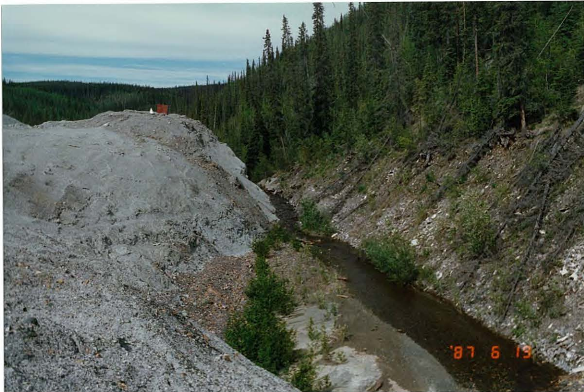
Photo 12: Build-up of material in the toe area of the south tailings pile and squeezing of the Wolverine Creek channel.
