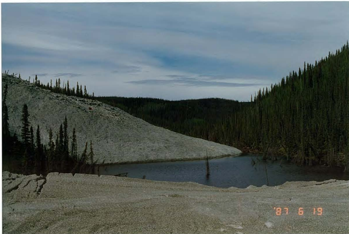
Photo 17: The toe area of the north pile is flatter than it was in 1986 and advanced only slightly towards the east valley wall.
