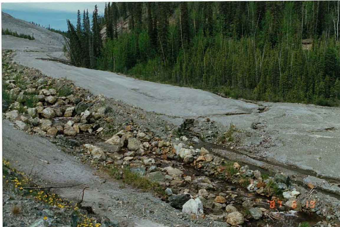
Photo 19: Junction of armoured and newly developed channels.
