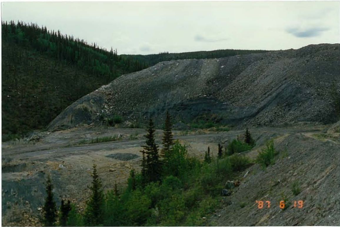
Photo 10: The downstream section of the Porcupine Dump. The underflow is discharged above the toe of the dump, apparently following more permeable materials within the waste. Surface drainage channel is on the left.
