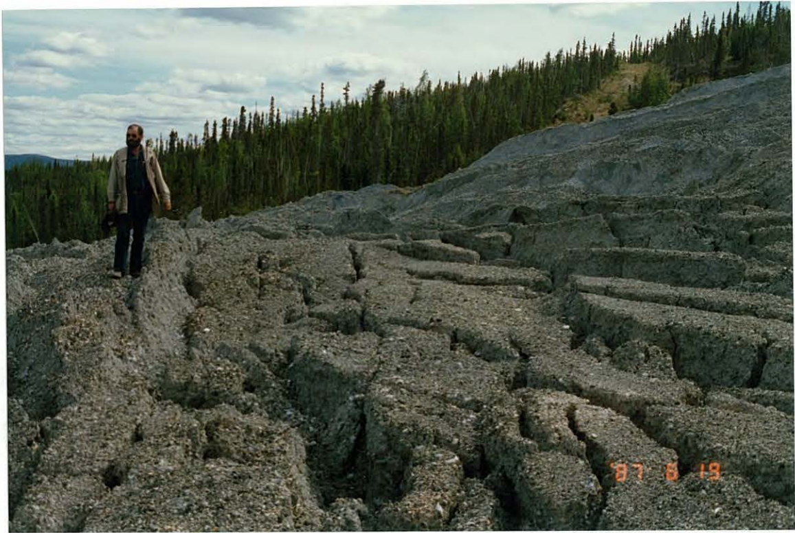
Photo 14: Middle sector of the south tailings pile shows fresh and deep tension cracks.
