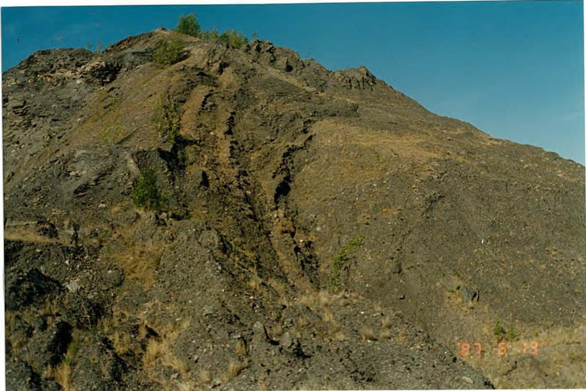
Photo 1: Fresh scarps outline the uppermost sector of the Clinton Creek Dump. No significant change in slump characteristics since 1986.
