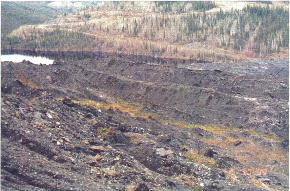
Photo 5: Prominent slide ridges parallel the toe of the hillside in the western segment of the dump.
