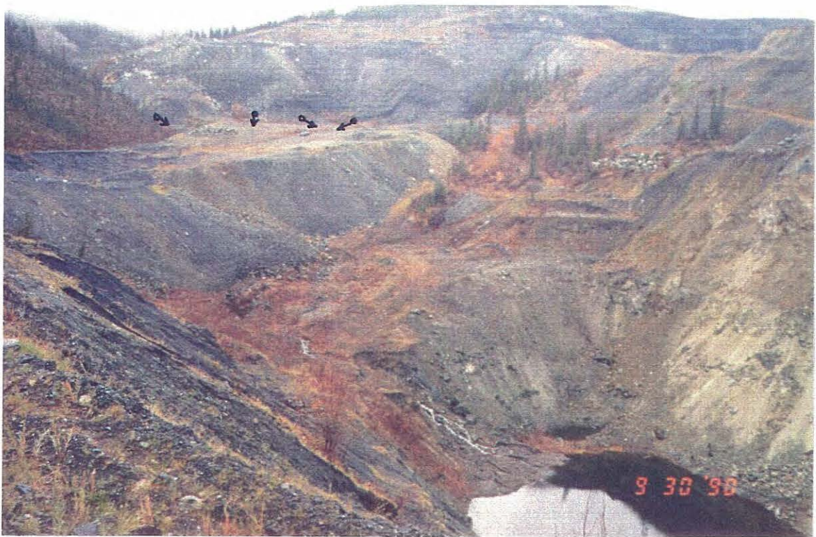
Photo 14: Underground flow is discharged at several locations from the northern toe of the Porcupine dump. This seepage apparently contributes to the instability of the dump on the left.
