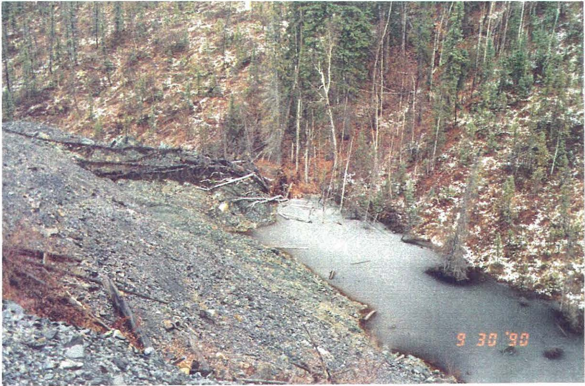
Photo 12: Eastern lobe of the pond formed by the sliding Porcupine dump appears to be narrower than in 1988. Refer to photo 12 of the 1988 report.
