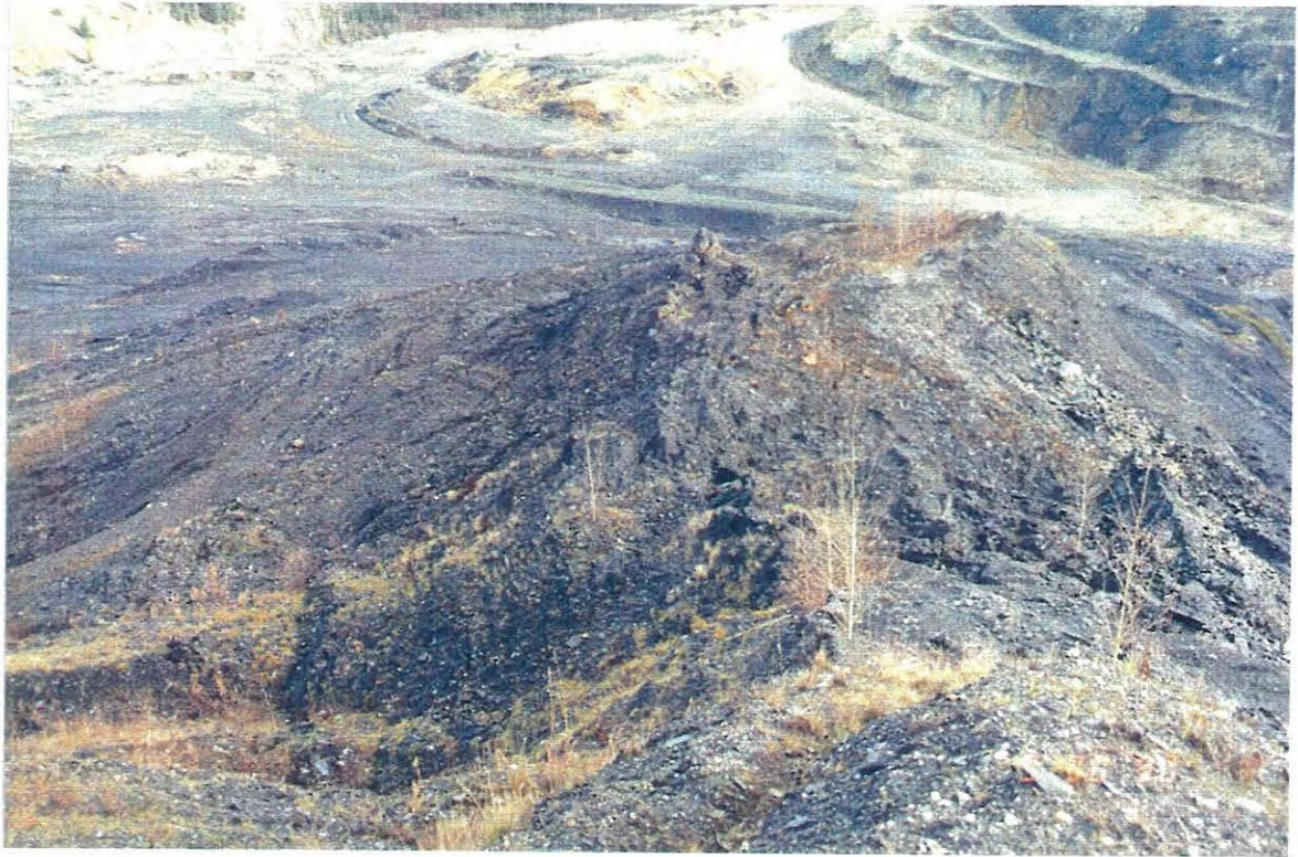
Photo 3: Unstable ridge bordering the north wall of the Porcupine pit. Refer to Photo 2 of the 1988 report.
