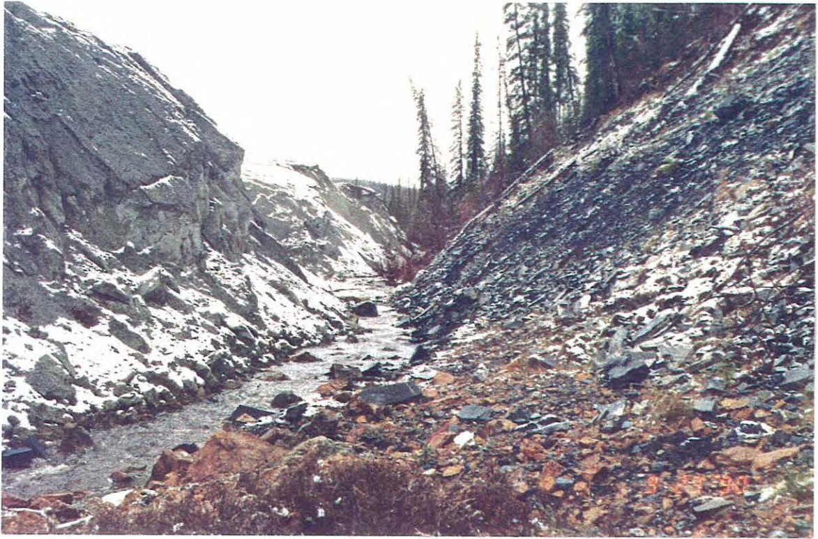
Photo 19: View of the outlet channel through the south lobe. Refer to photos 20 and 21 of the 1988 report.
