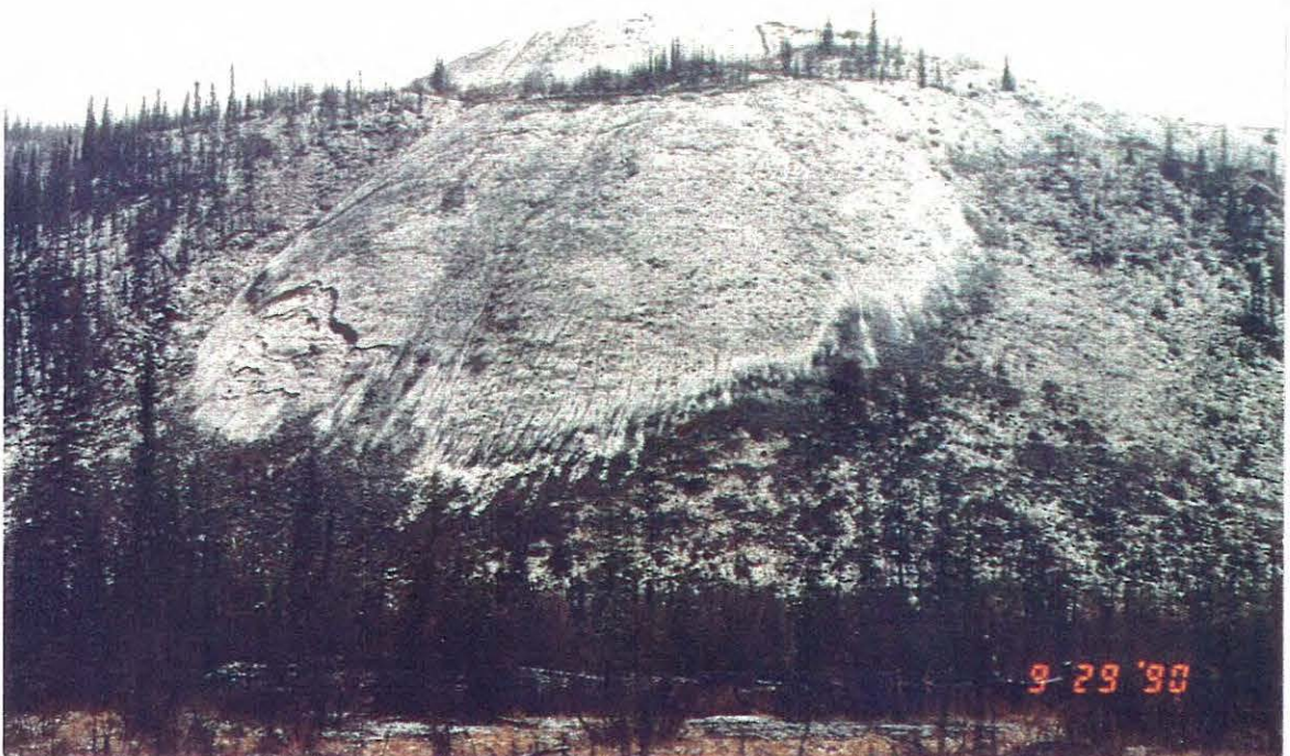
Photo 15: View of the Snowshoe waste dump. Fresh cracks exist along the crest of the dump and at its toe.
