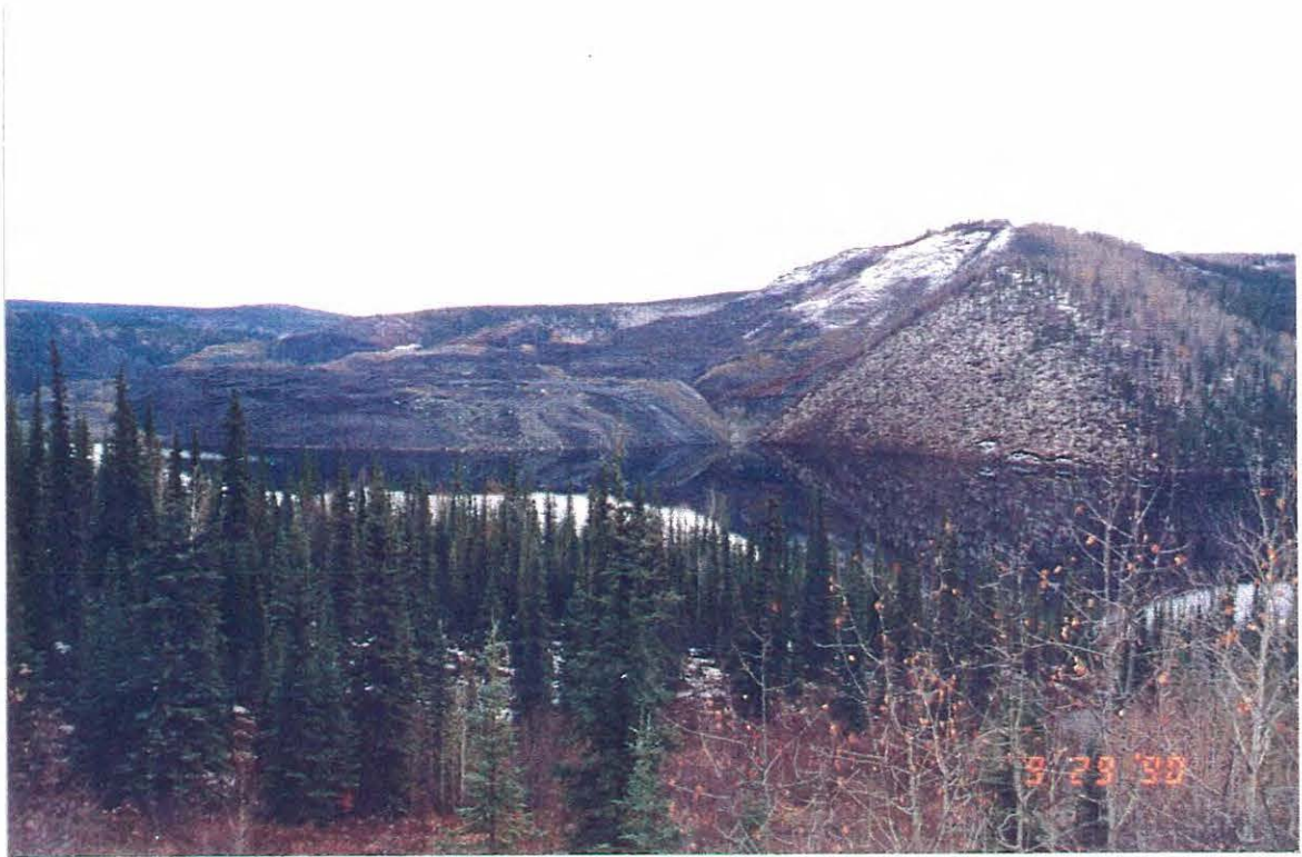
Photo 1: View of the Clinton Creek waste dump. Note small slumps along the lake shore upstream from the dump.
