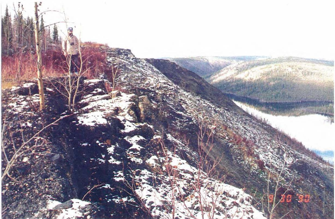
Photo 2: Fresh cracks along the waste dump headscarp.
