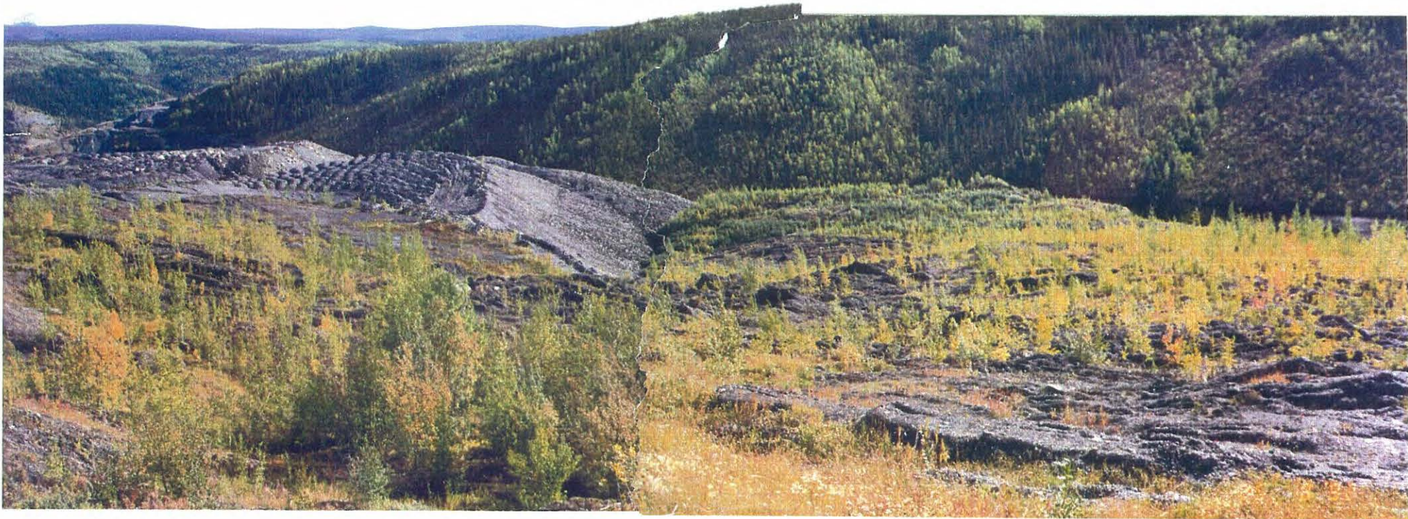
Photo 11: Oblique view of the Porcupine Creek waste dump, looking north. Movement of the dump is well illustrated by fresh fissures and scarps, widespread along the headscarp and throughout the southern dump segment.
