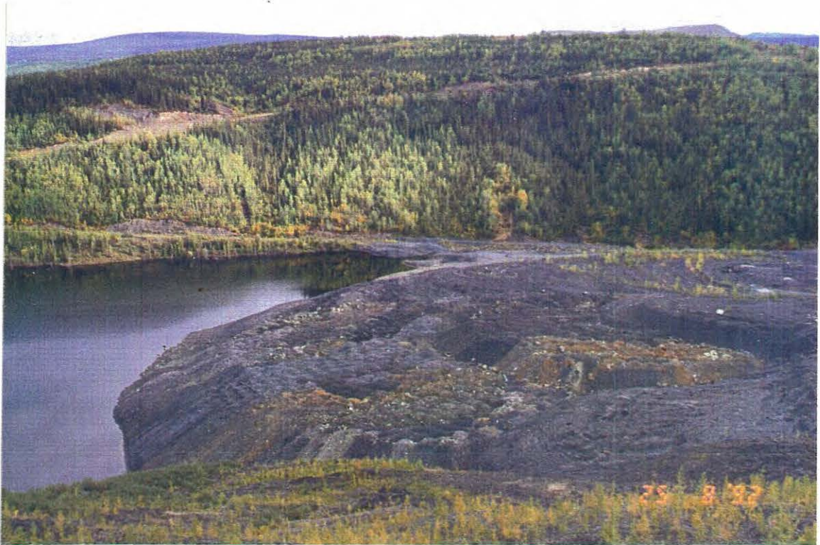
Photo 5: View of the Clinton Creek waste dump forming the valley plug. Hudgeon Lake outlet in background.
