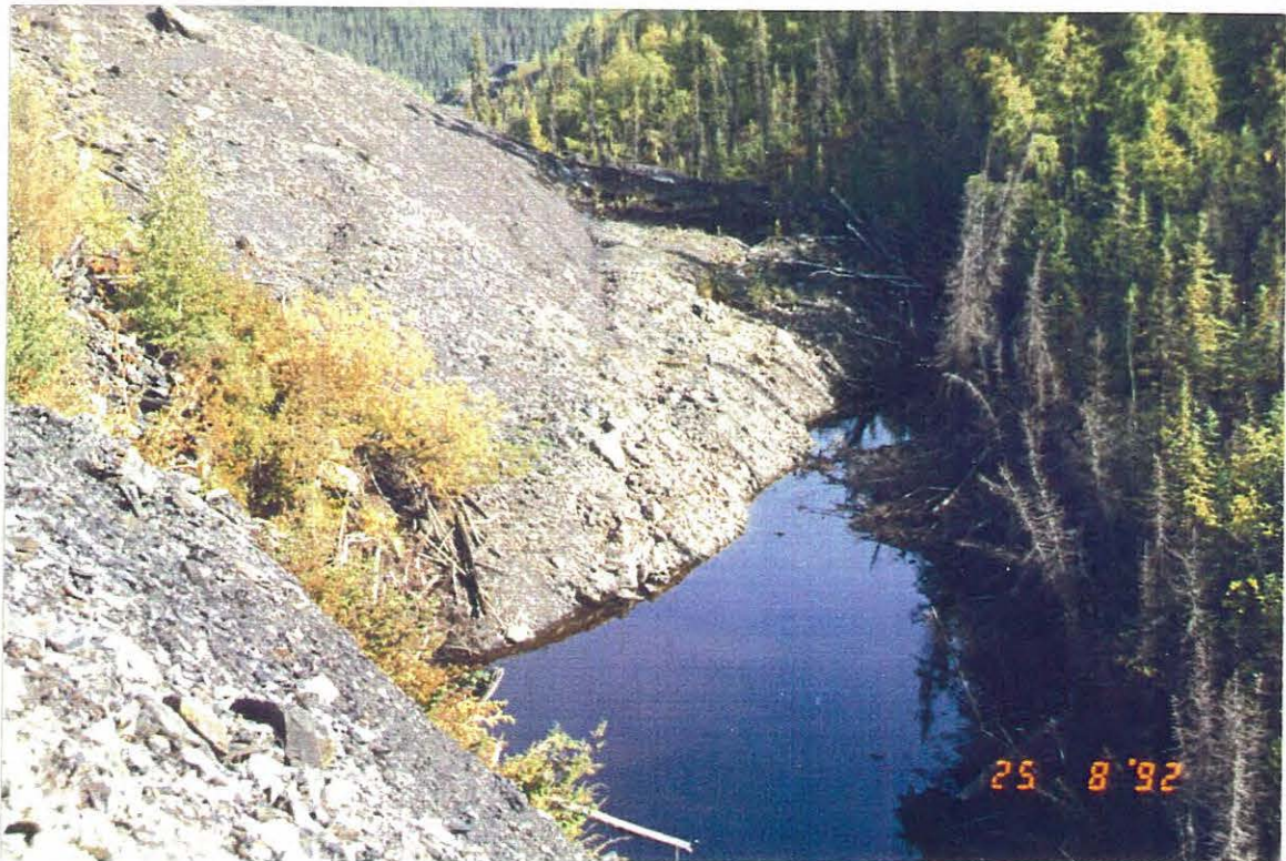
Photo 13: Original valley blockage has been widened as a result of ongoing ground and dump movement.
