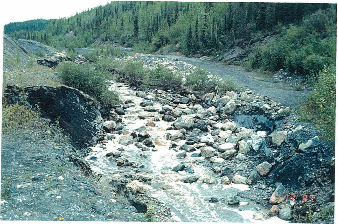
Photo 7: Armoured channel and control weir was destroyed during the 1997 flood event. Compare with Photo 7/90 and Photos 5 and 6 of the 1988 report.
