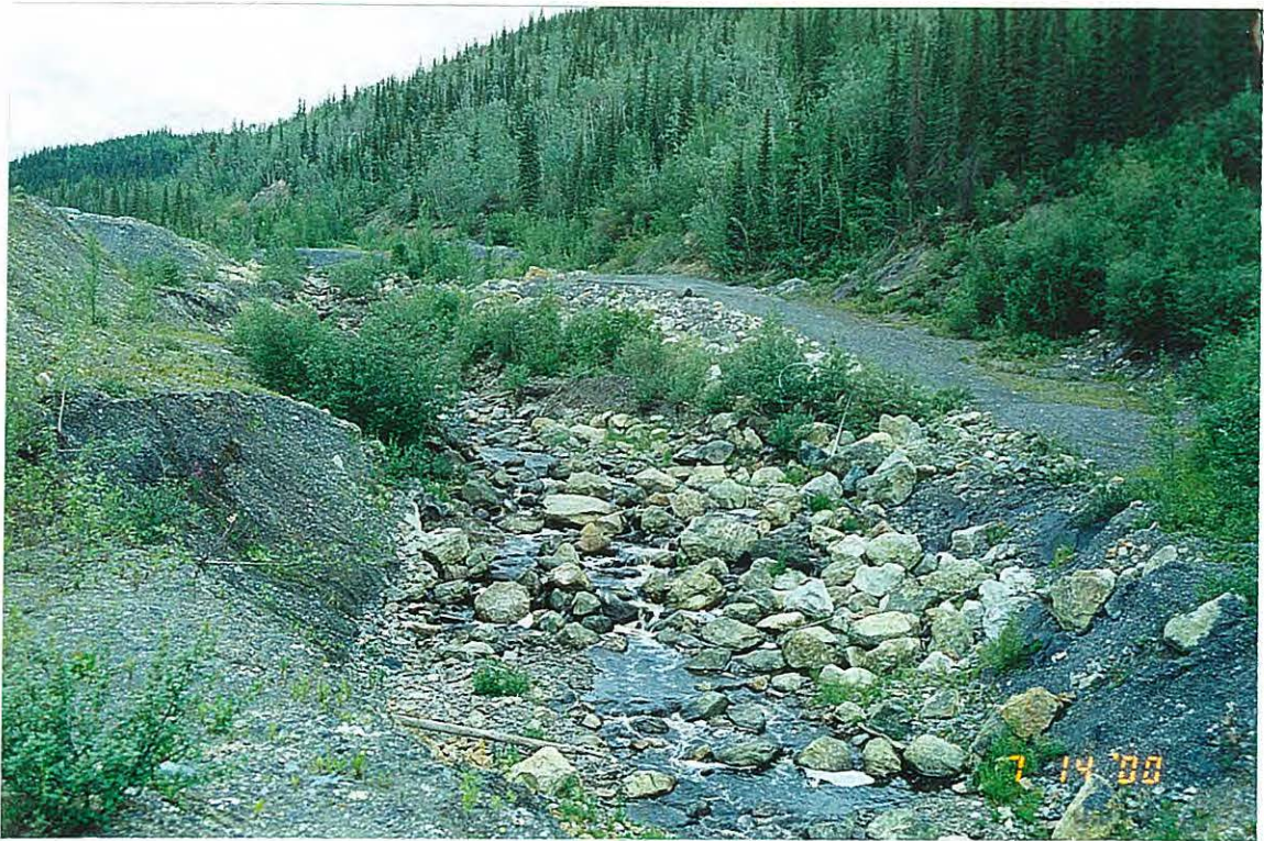
Photo 5: View of former rock weir and increased lateral erosion of both channel banks.
