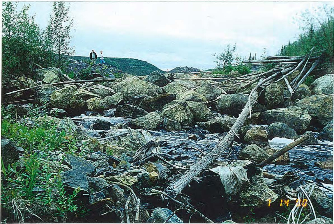
Photo 1: Looking upstream at the rip-rap segment of the Hudgeon Lake outlet. The left side appears to sag relative to the right side.
