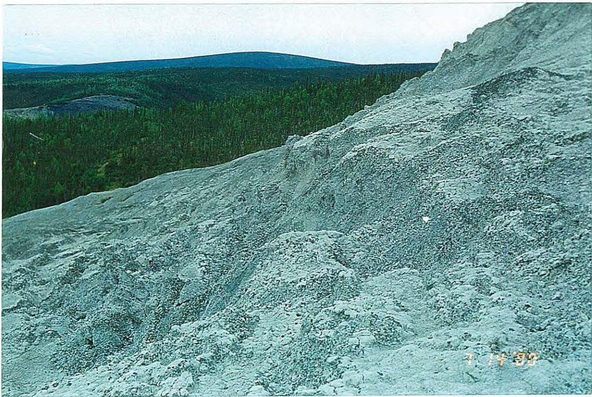
Photo 7: Wolverine Creek tailings pile. View of one of several active headscarps.
