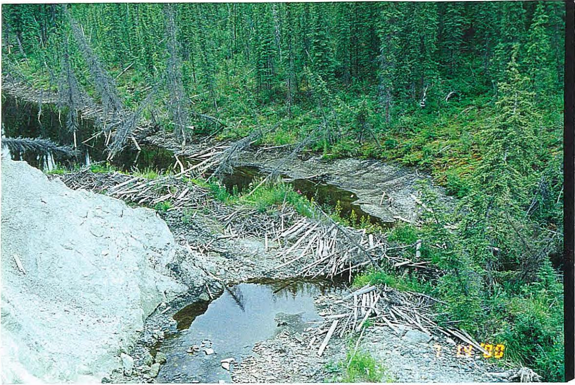
Photo 9: View of the beaver dam located at the upstream edge of the south tailings pile, uplifted by ongoing ground movements.
