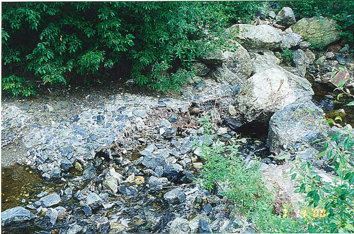
Photo 11: View of the Wolverine Creek lowermost rock weir, currently dislodged. Note the channel erosion.
