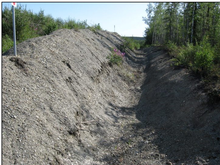
Figure 51 Ditch and Berm at WP 359
