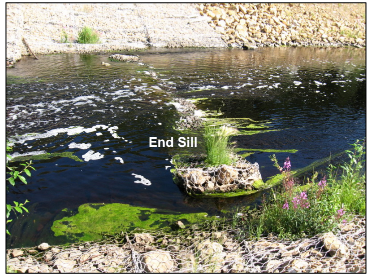
Figure 39 DS #1 End Sill in July 2009, view N
