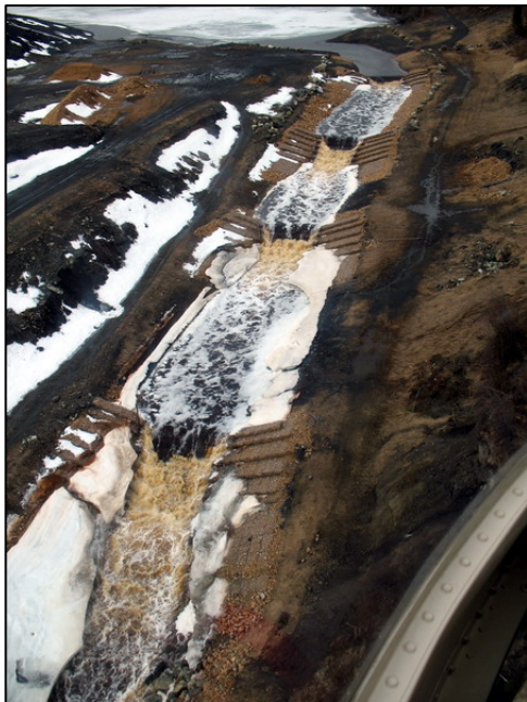
Figure 15 Gabion Drop Structures in May 2009 (DS # 2 on Right Hand Side Photo)
