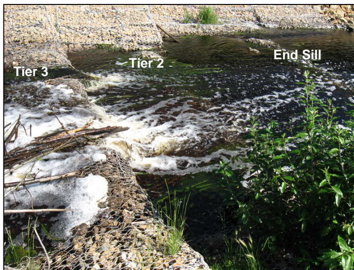
Figure 38 DS #1 Tier 2 and 3 & End Sill in July 2009, view N
