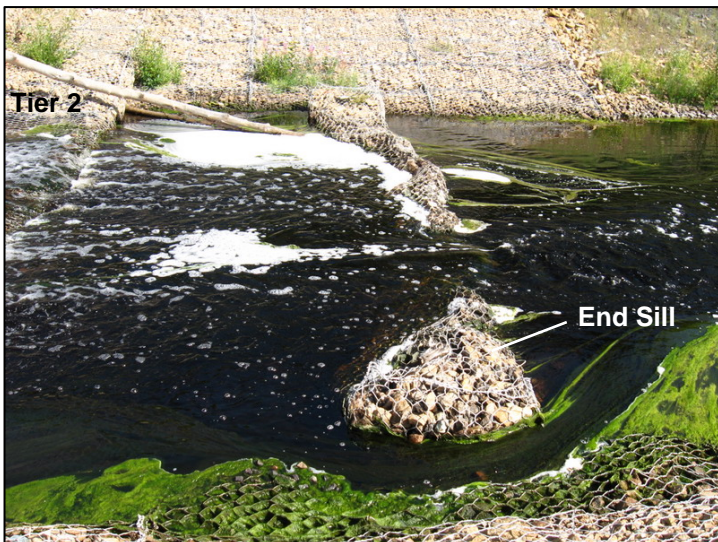
Figure 27 DS #3 End Sill in 2009, view N
