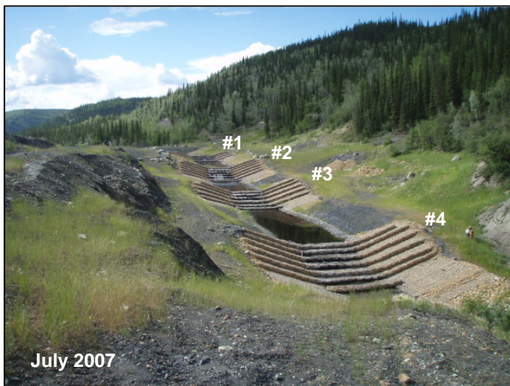
Figure 14 Gabion Drop Structures in 2007 (left) and From WP 346 in 2009 (right), view U/S
