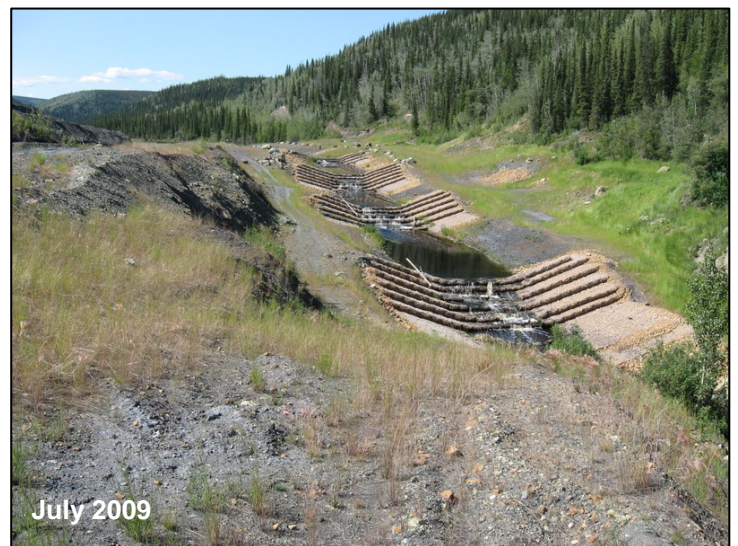
Figure 14 Gabion Drop Structures in 2007 (left) and From WP 346 in 2009 (right), view U/S
