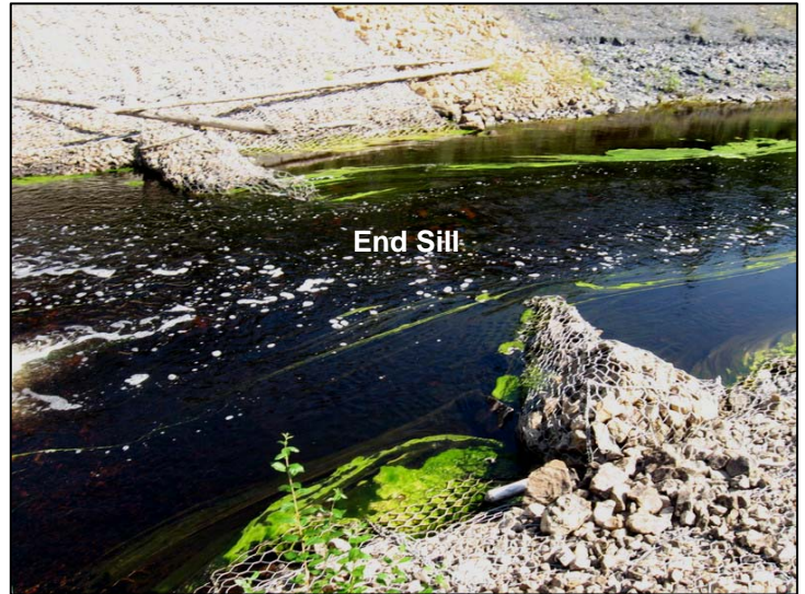
Figure 33 DS #2 End Sill in 2009, view N
