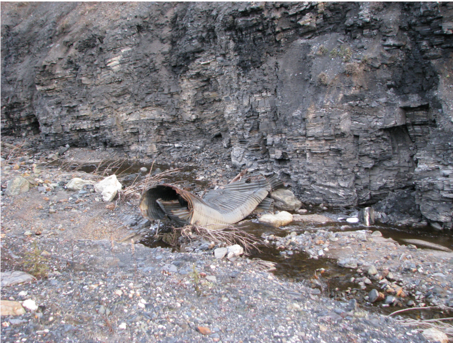
Old culvert in canyon below gabion drop structures.
