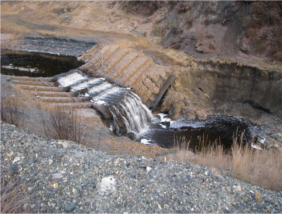
Lower drop structure Oct 7, 2010
