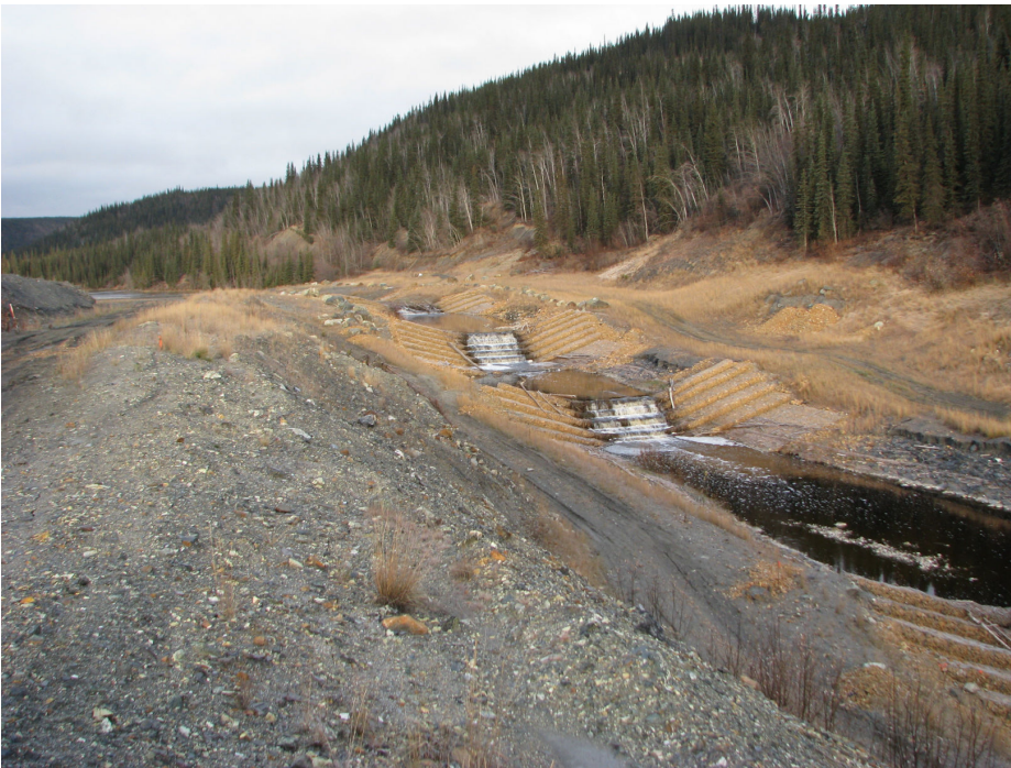
Upper three drop structures
