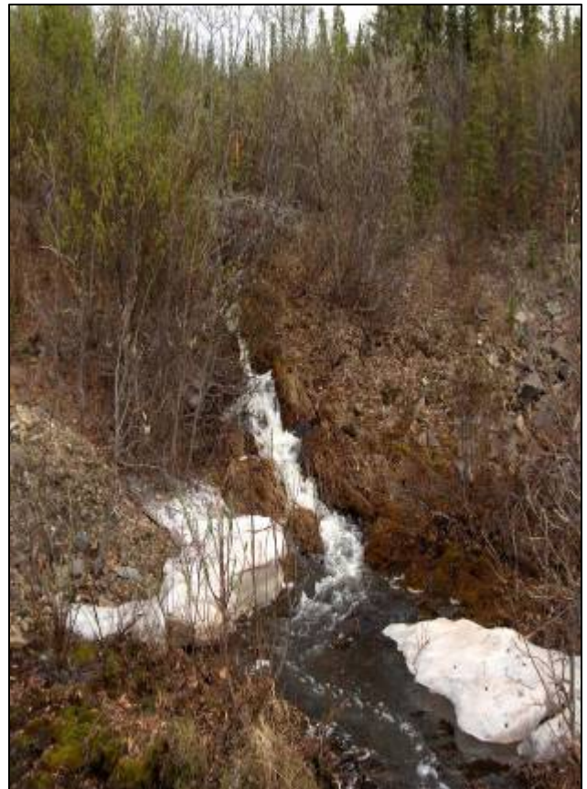
Plate 11: Bermingham discharge upstream of Calumet Drive culvert
