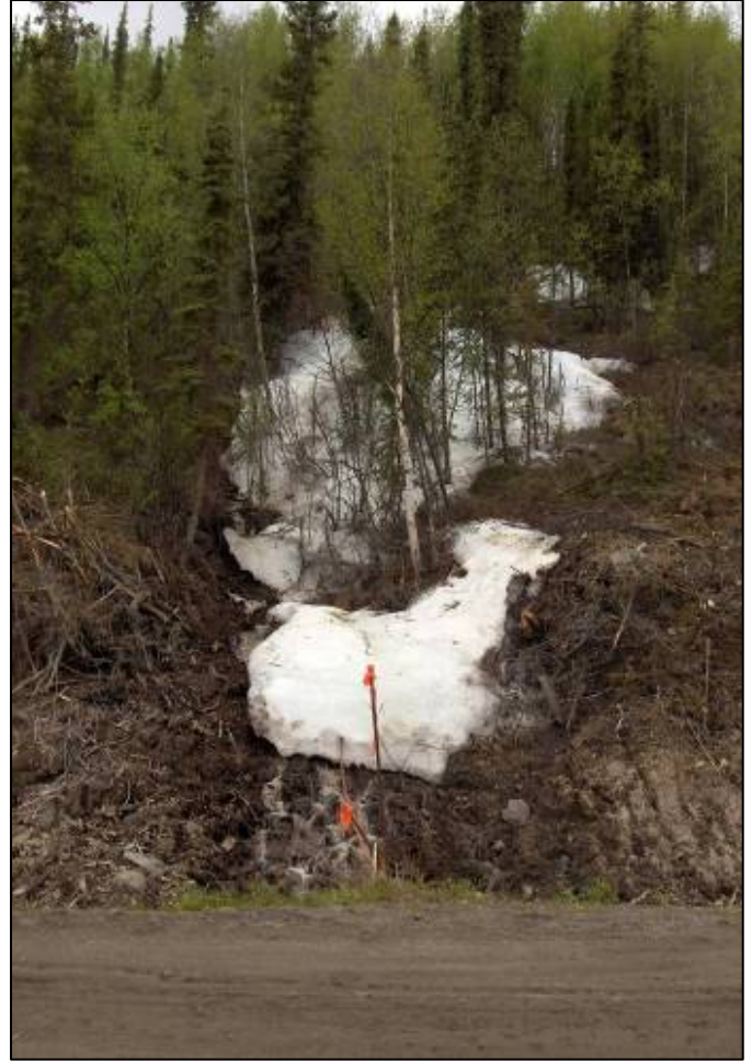
Plate 21: Galkeno 300 discharge at Silver Trail Highway
