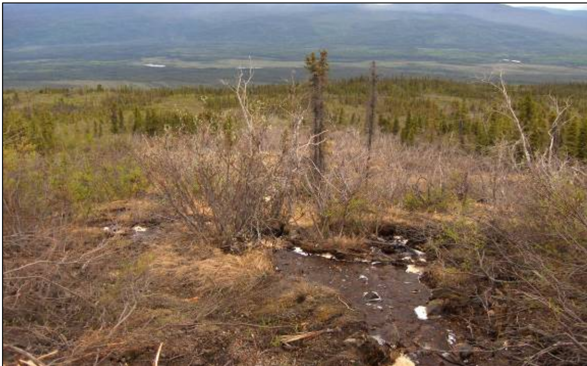
Plate 16: Ruby discharge down gradient of Calumet Drive culvert
