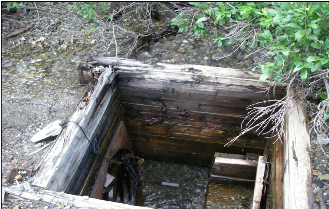
Plate 29: Sadie Ladue flow from adit through culvert
