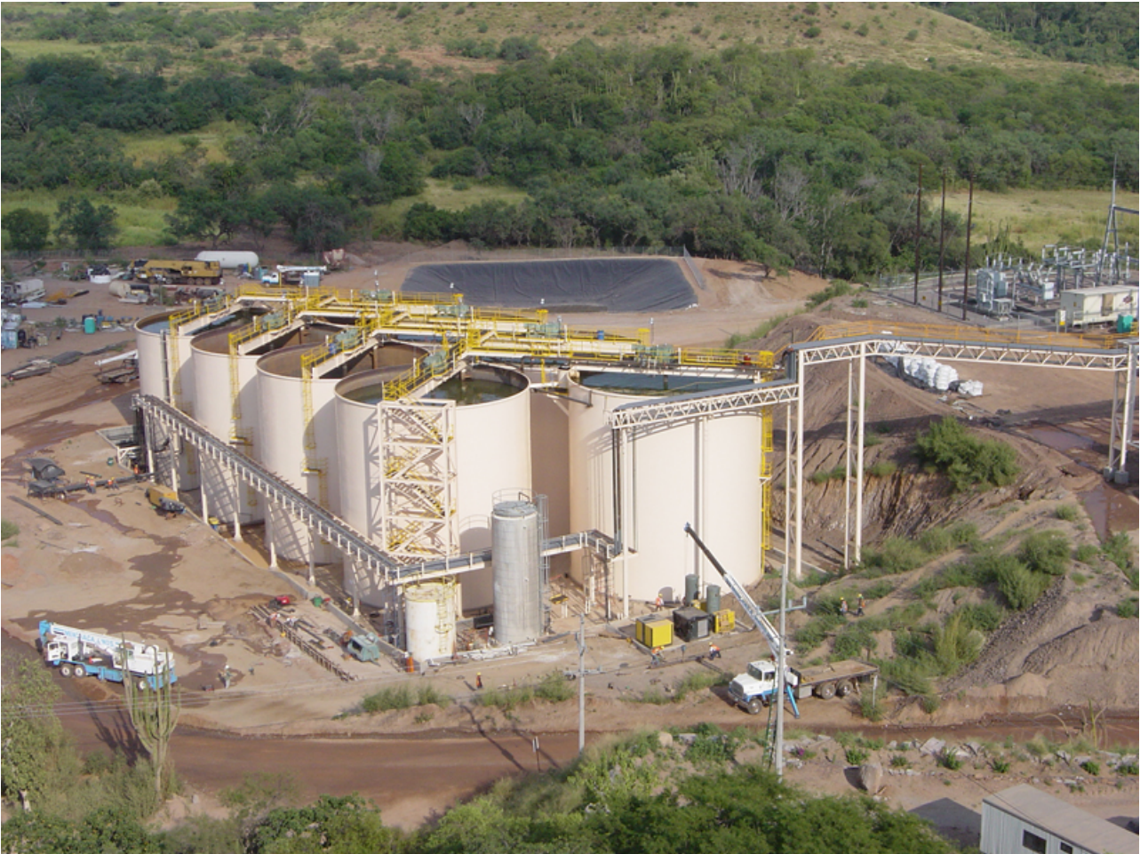
FIGURE 5. EXAMPLE OF CIP/CIL SILVER RECOVERY CIRCUIT
