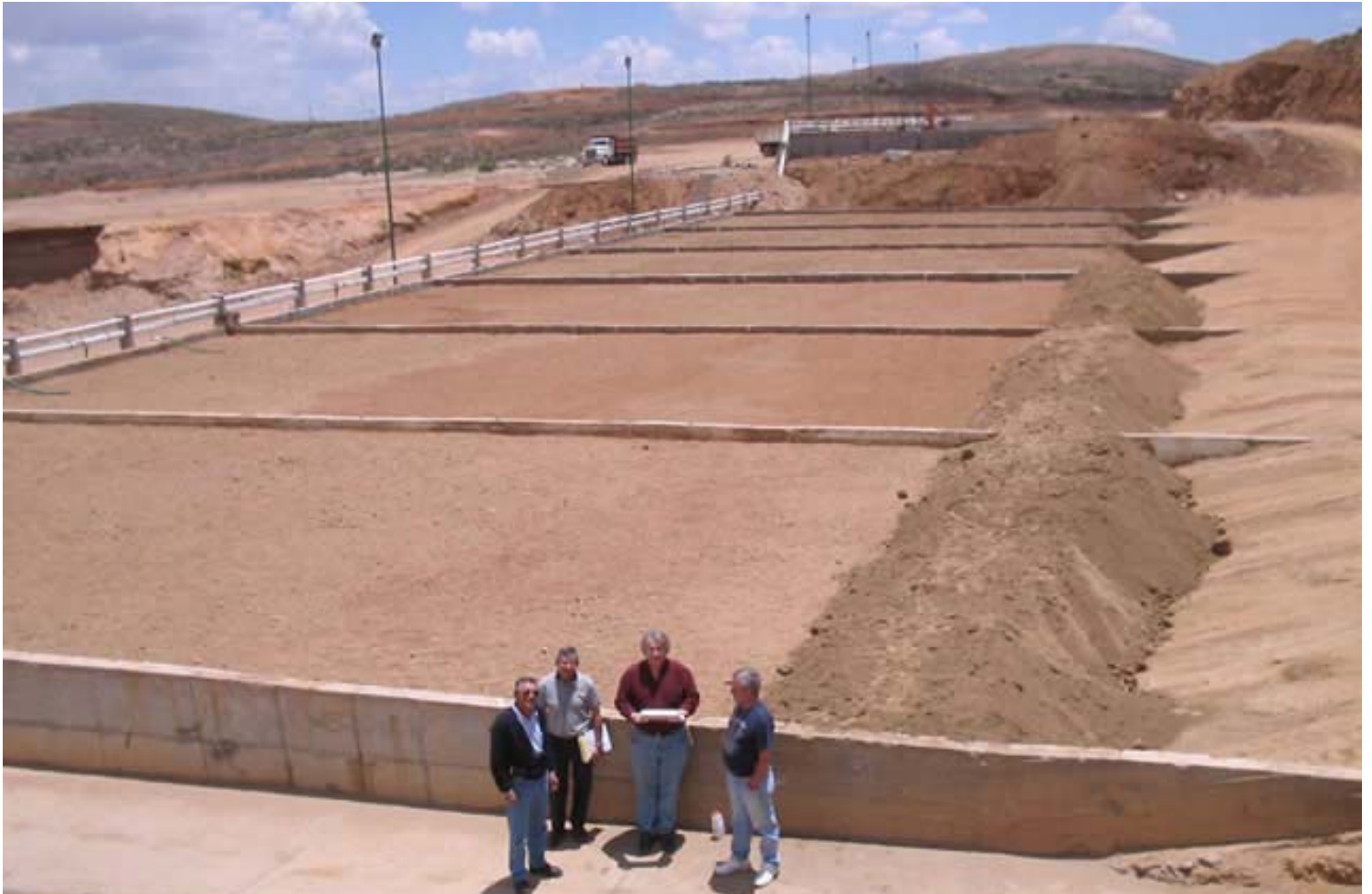
FIGURE 4. EXAMPLE OF TAILINGS VAT LEACH SYSTEM
