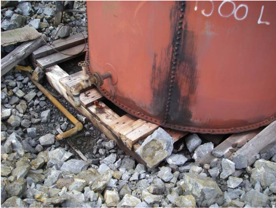
Photo #11: AST and surface staining at Husky
