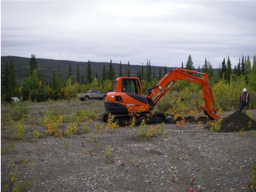
Photo #23: Test pit excavation for potential LTF near CBC tower
