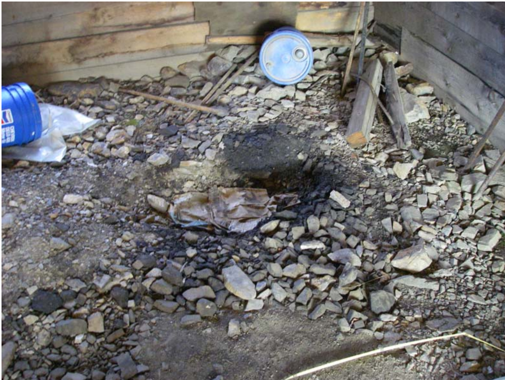
Photo #20: Inside Runer building
