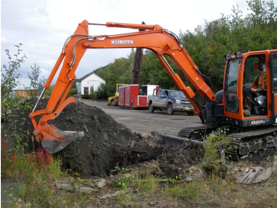
Photo #7: Test pit for potential LTF location in sawmill yard
