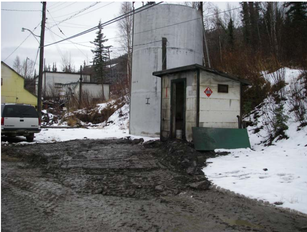
Photo #8: Fuel storage area #4
