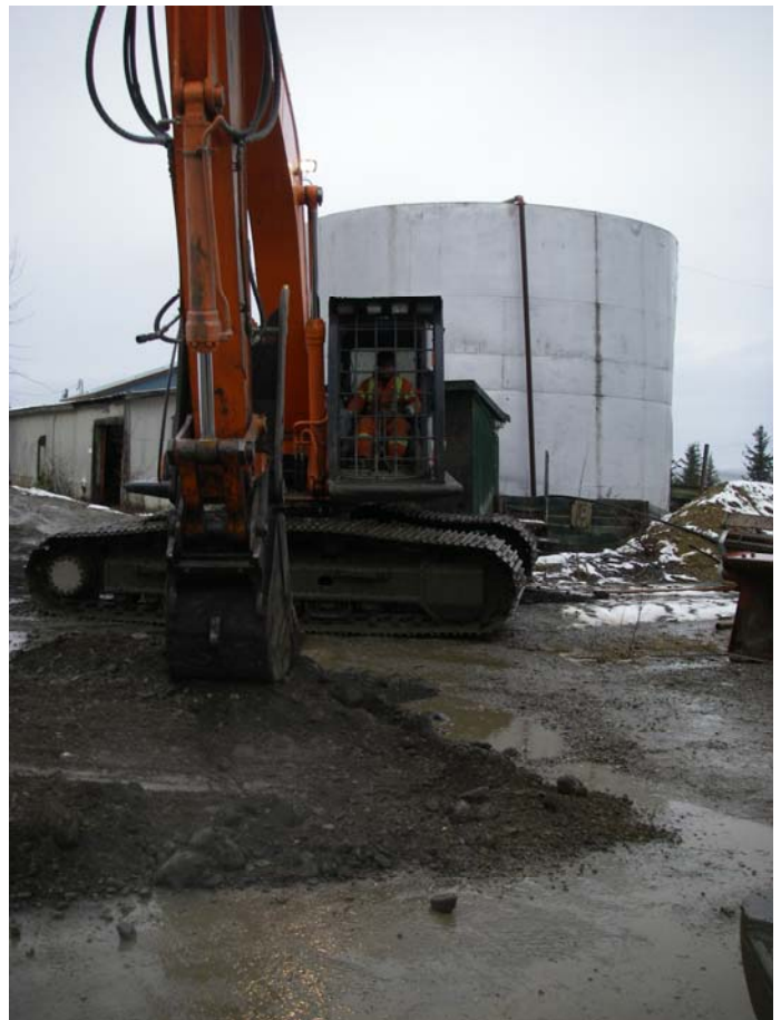
Photo #14: Test pit at fuel storage area #3
