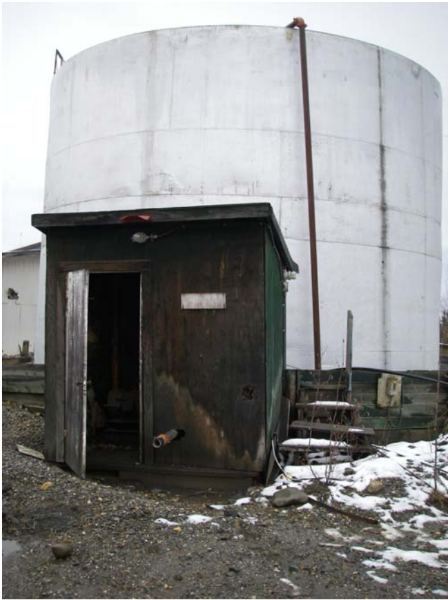
Photo #13: Fuel storage area #3
