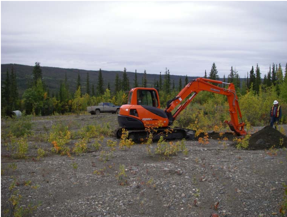
Photo #9: Test pit excavation for potential landfill near CBC tower
