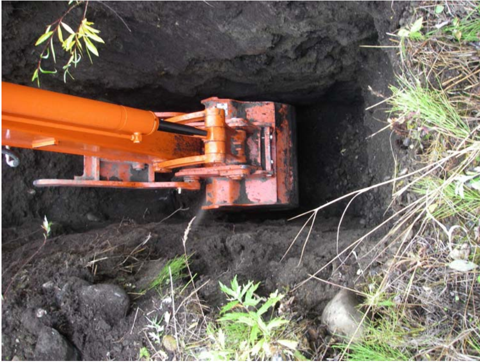
Photo #5: Test pit excavation 4 m deep below Elsa old dump site
