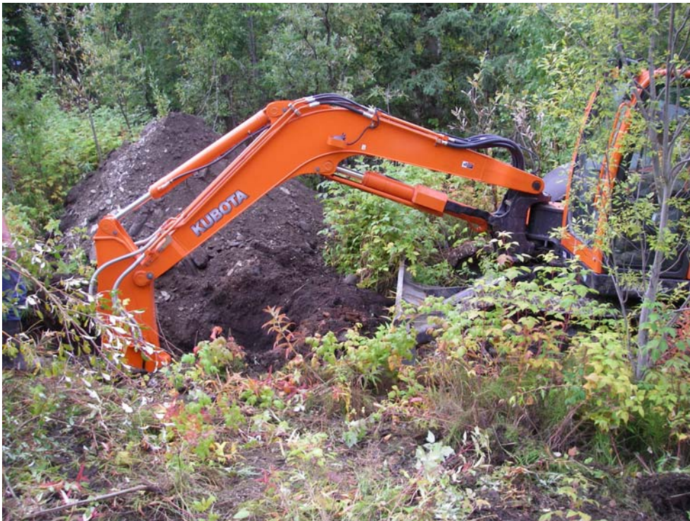
Photo #4: Test pit excavation below the Elsa old dump site
