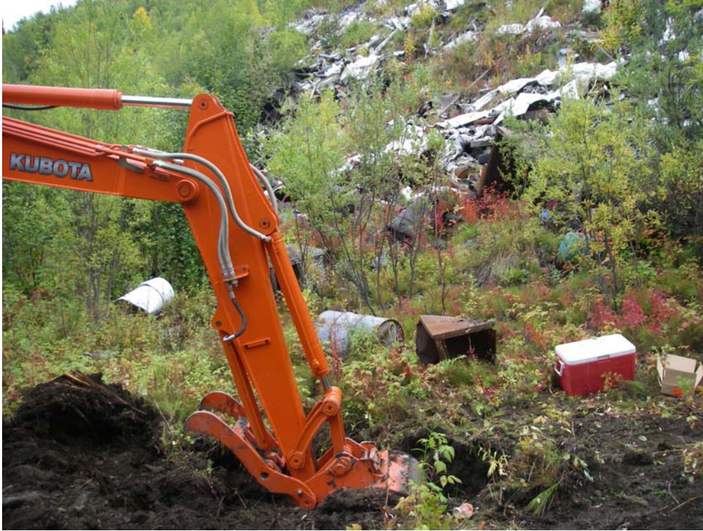
Photo #3: Test pit excavation below Elsa old dump site
