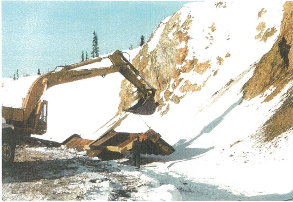
(February 18, 2001) Placing truck canopies over flume in front of Zone 1.
