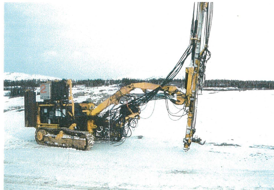
(February 12, 2001) Atlas - Copco track mounted pneumatic drill rig for blast holes
