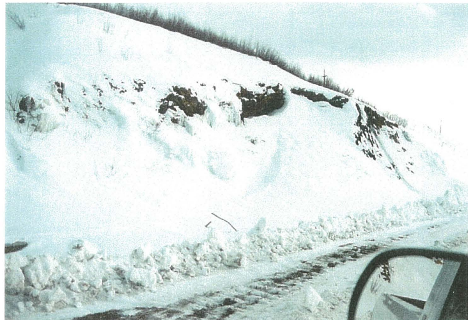
(February 12, 2001) Zone 4 area prior to start of work.
