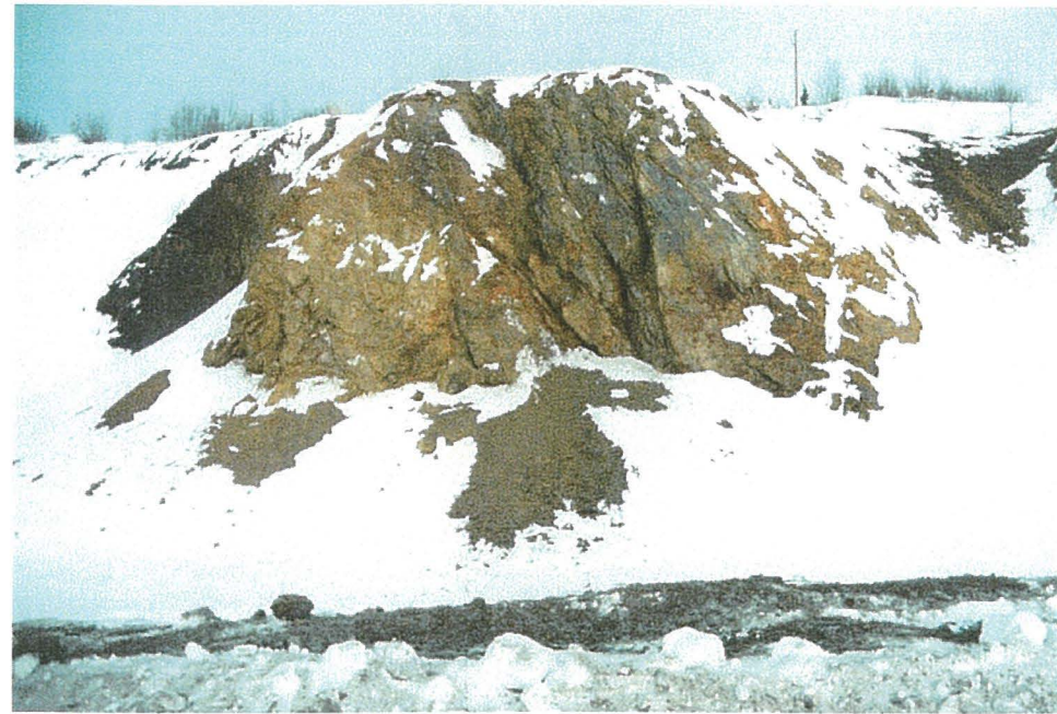
(February 12, 2001) Bedrock knob at downstream end of Zone 1, previously recommend for rock bolting. (Prior to start of work).
