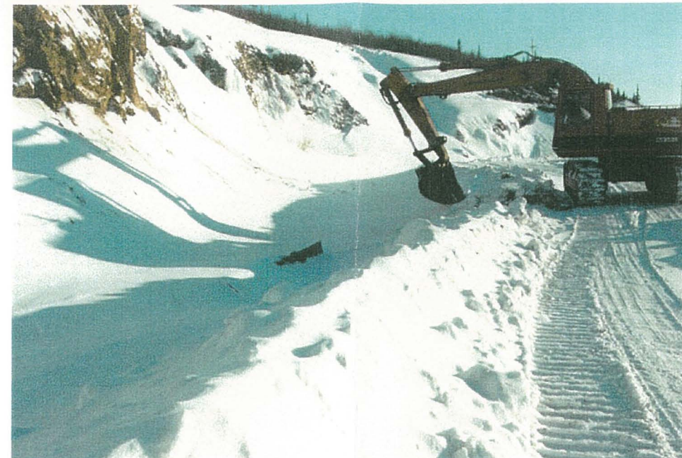
(February 14, 2001) Removing snow in front of Zone 1 for flume protection.
