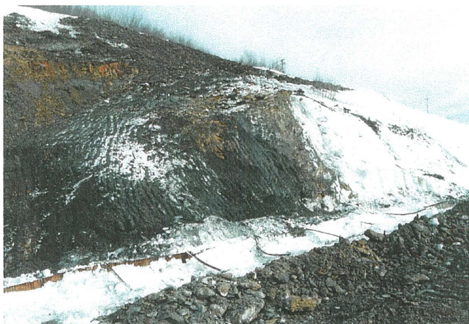
(February 25 2001) Final Slope after trimming and scaling in Zone 4.
