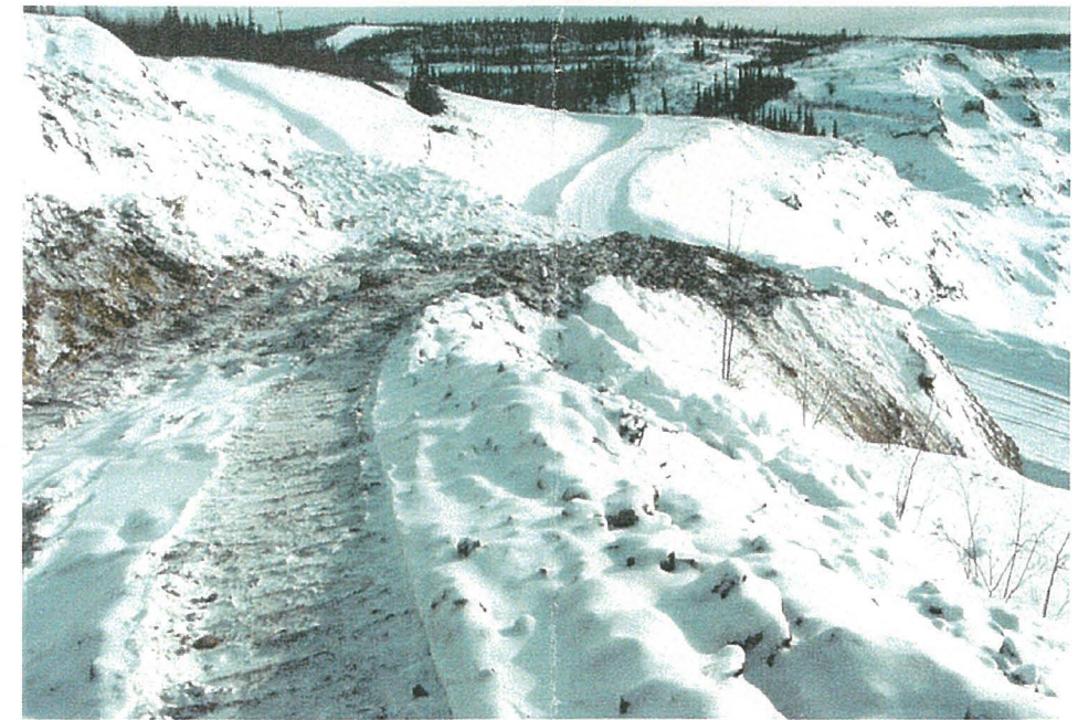
(February 13, 2001) Completed access to top of Zone 1 area ready for drilling.
