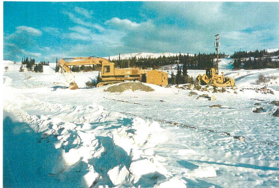
(February 12, 2001) Golden Hill Equipment at lay down area at Vangorda Flume
