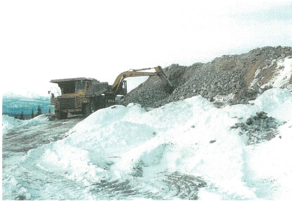
(February 15, 2001) Excavating and hauling riprap at quarry.
