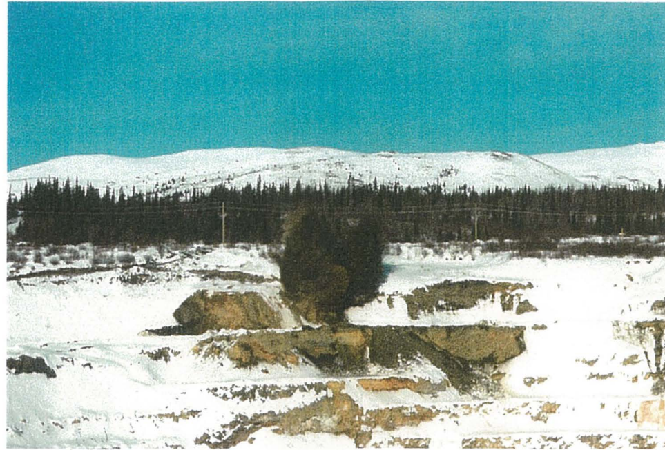
(February 20, 2001) Blast - Zone 1 area.
