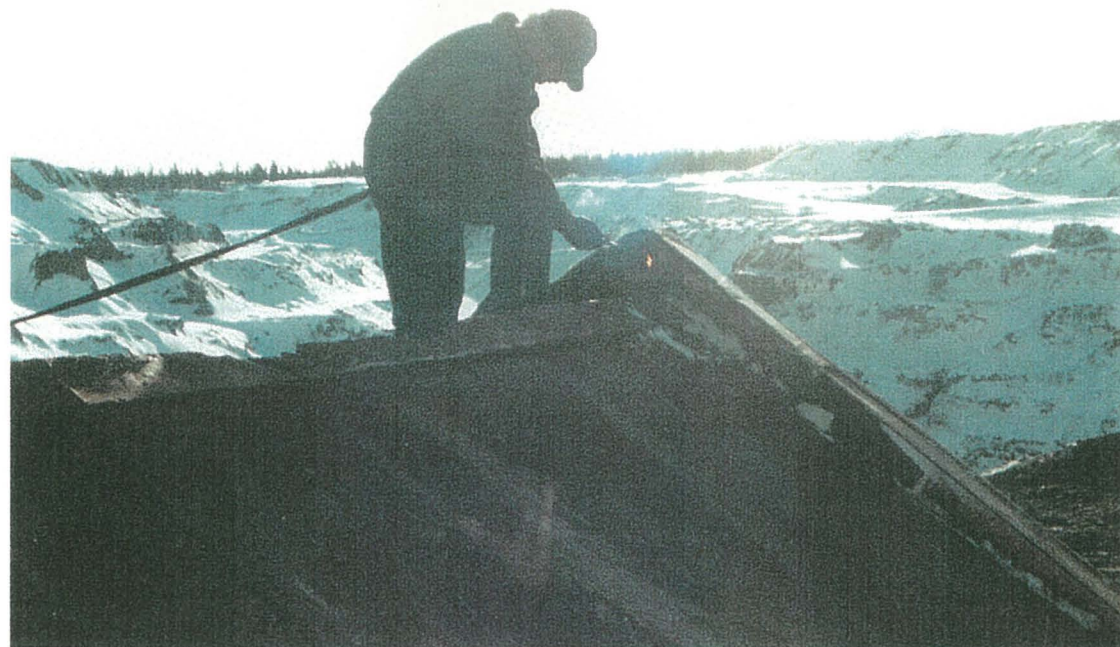
(February 18, 2001) Torch cutting holes in truck canopies for lifting eyes.
