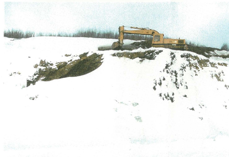
(February 13, 2001) Cutting access road to top of Zone 4 for drill.
