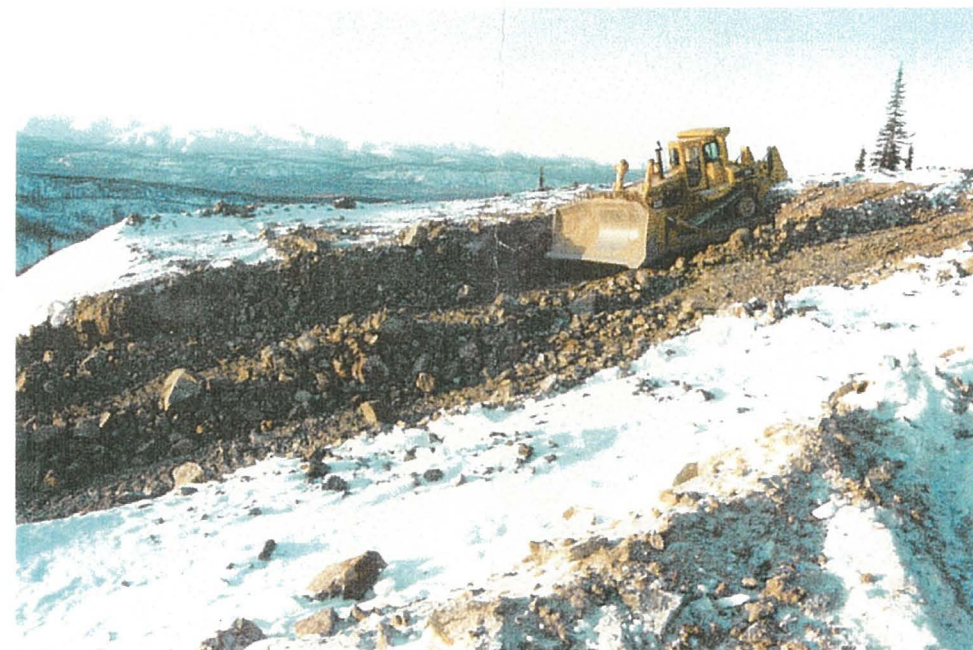
(February 14, 2001) Cat D9N ripping blasted riprap in quarry.
