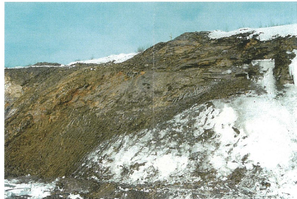
(February 25, 2001) Zone 1 area completed trimming and scaling.
