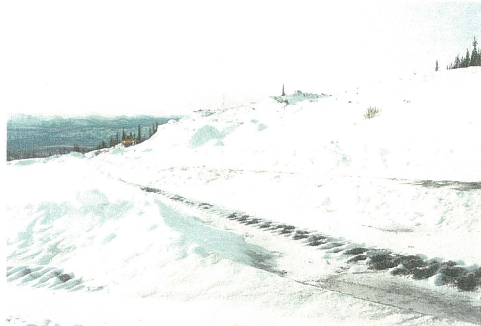
(February 13, 2001) Cleaning snow from access road to riprap quarry.
