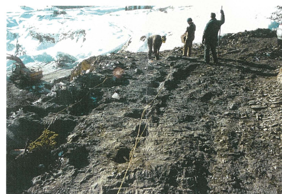
(February 20, 2001) Loading blast holes Zone 1.
