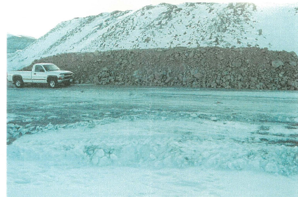
(February 18, 2001) Completed stockpile - 1204 m 3 volume.
