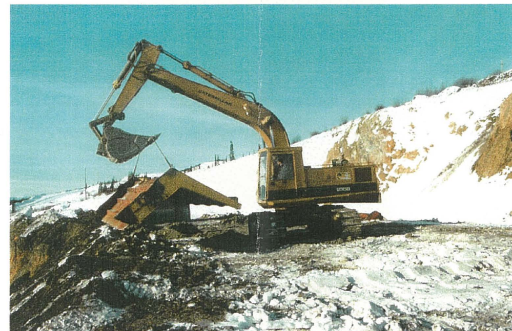
(February 18, 2001) Lifting truck canopies with Cat 235 backhoe.
