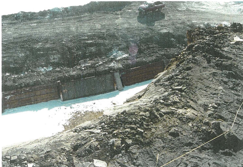
(February 25, 2001) Completed scaling of downstream end of Zone 1 area.
