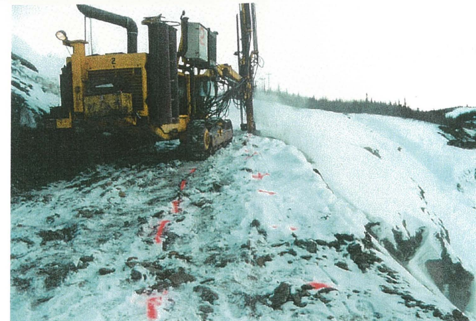
(February 17, 2001) Drilling blast holes in Zone 1.
