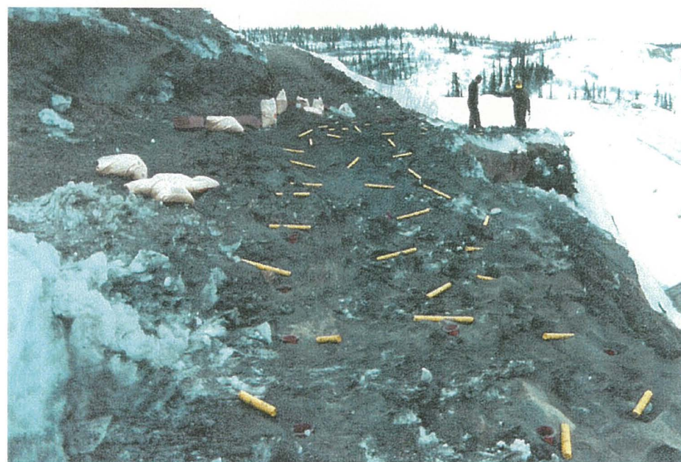
(February 21, 2001) Loading drill holes Zone 4 area.
