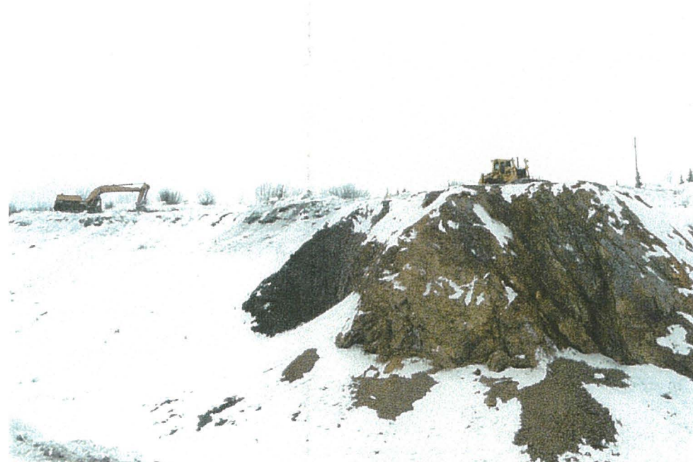
(February 13, 2001) Excavating access road to top of Zone 1.
