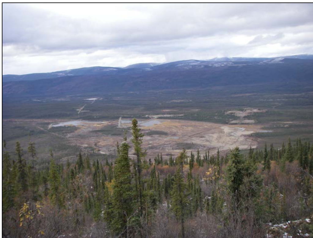
Photo 1. View of the Elsa tailings facilities, looking northwest.
