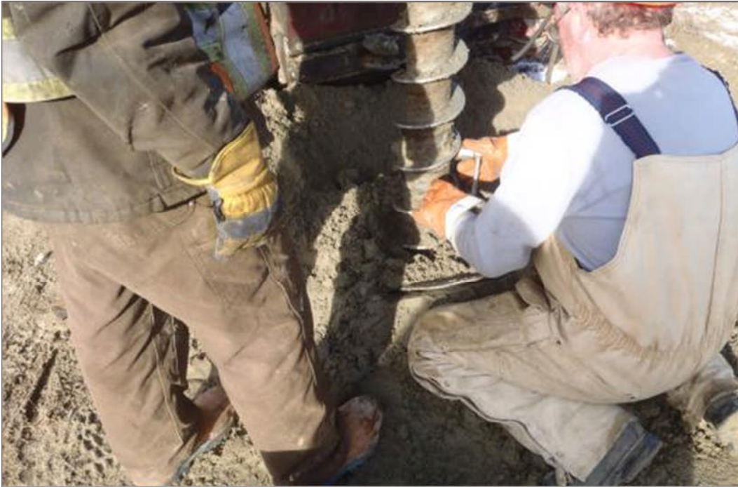
Photo 5: Frozen sand encountered in BH01, BH02, and BH04 (October 3, 2012)
