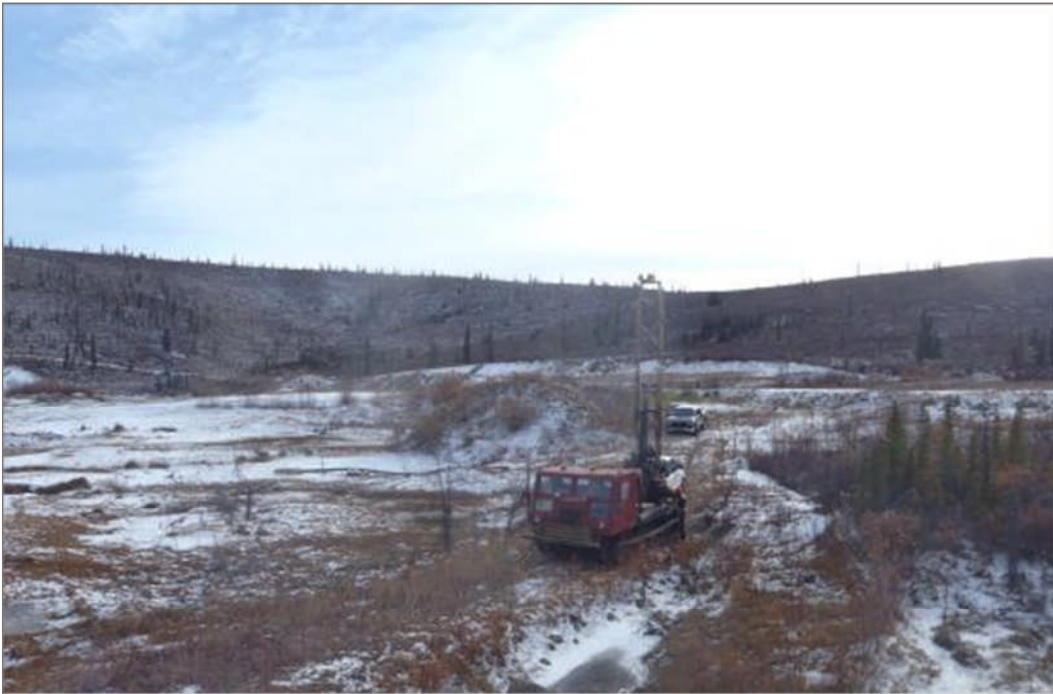
Photo 2: Drilling BH03 Facing south (October 2, 2012)
