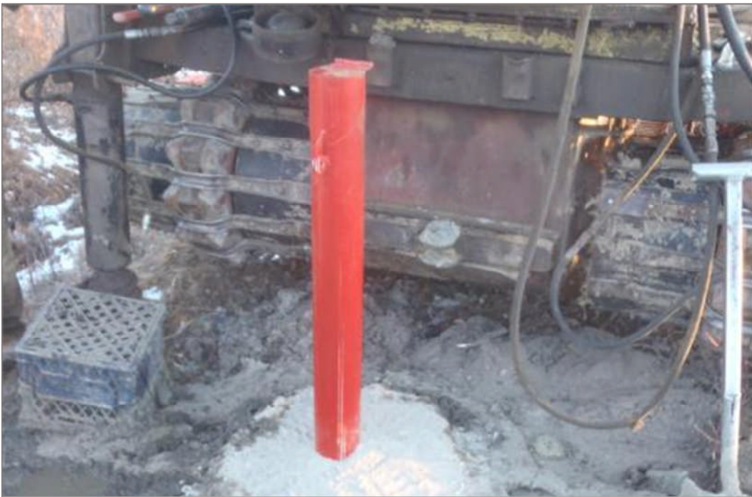
Photo 6: Typical completed installation (October 2, 2012)
