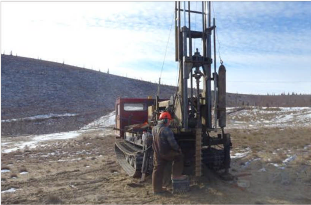
Photo 4: Drilling BH04 Facing south (October 3, 2012)
