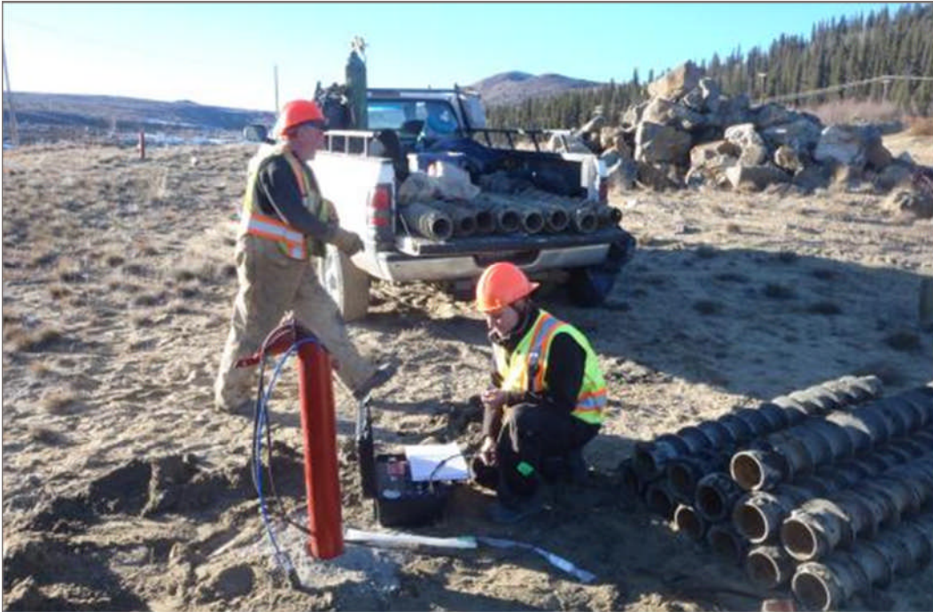
Photo 7: Collecting initial readings from piezometers in BH04 Facing west (October 3, 2012)
