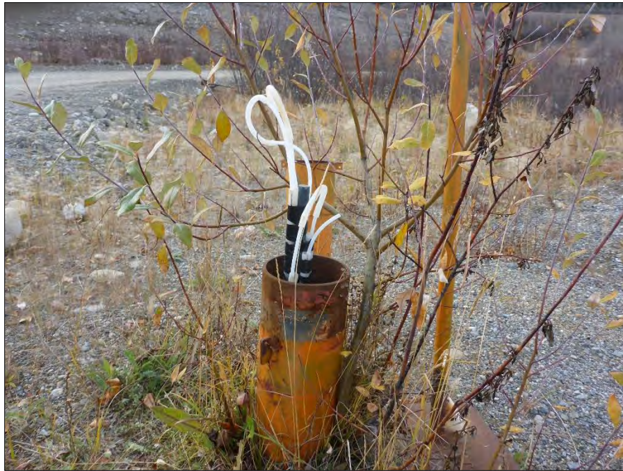
Photo 27: View of well P05-01, includes depths 01, 02, 03, 04, and 05. Photo taken on September 23 rd , 2016.
