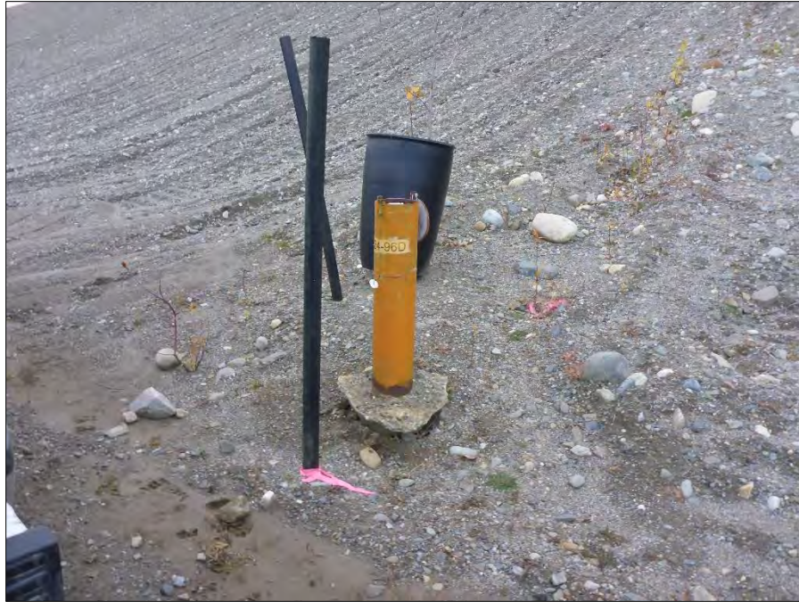
Photo 67: View of well X24-96D. Photo taken on September 23 rd , 2016.
